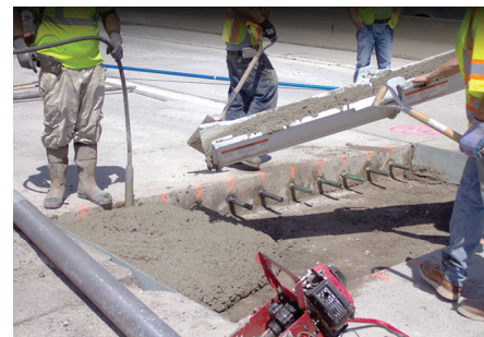
ACPA, used with permission Figure 10. Full-depth repair
