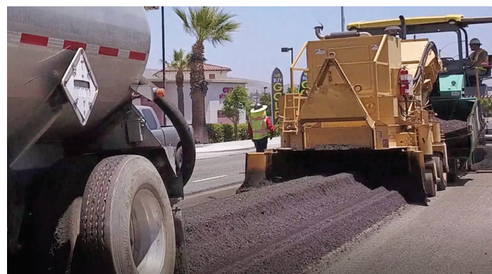
Figure 3. Cold in-place recycling
