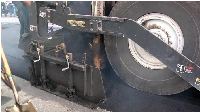
National Center for Pavement Preservation Figure 7. Thin hot-mix asphalt overlay
