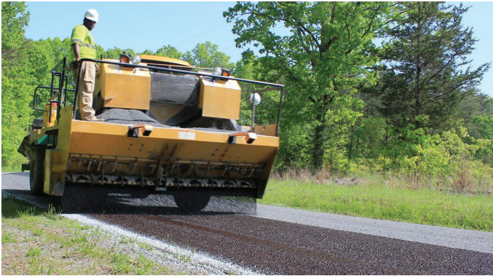
Slurry Pavers, Inc. Figure 6. Chip sealing
