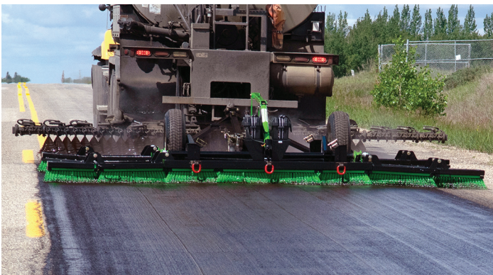
Saskatchewan Ministry of Highways and Infrastructure Figure 8. Scrub sealing
