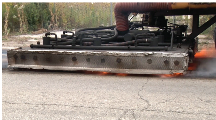
Figure 2. Hot in-place recycling
