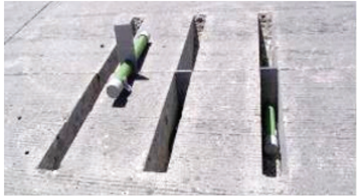
ACPA Figure 10. Dowel bar retrofit
