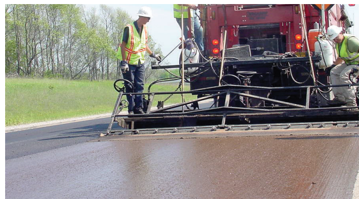
Figure 4. Micro surfacing
