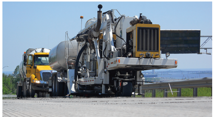
International Grooving and Grinding Association Figure 11. Diamond grinding
