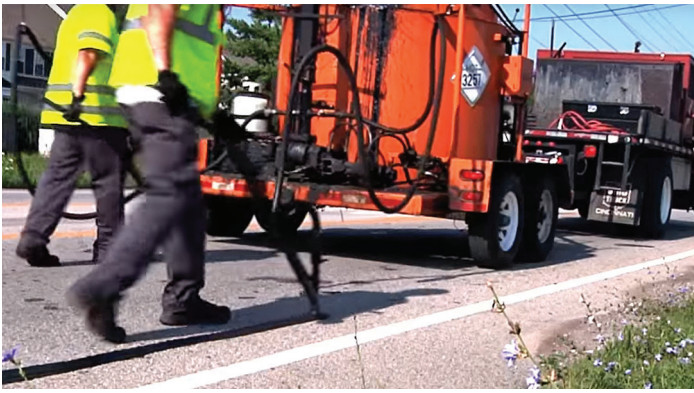
National Center for Pavement Preservation Figure 5. Crack sealing
