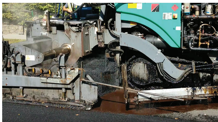
Figure 1. Ultrathin bonded wearing course
