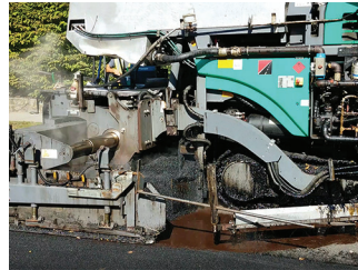
All States Materials Group Figure 3. Ultrathin bonded wearing course
