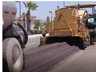
Pavement Recycling Systems Figure 5. Cold in-place recycling
