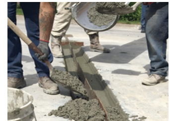
ACPA Figure 6. Partial-depth repair
