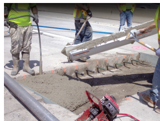
ACPA Figure 7. Full-depth repair
