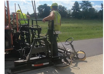
Strawser Construction Inc. Figure 4. Cape sealing
