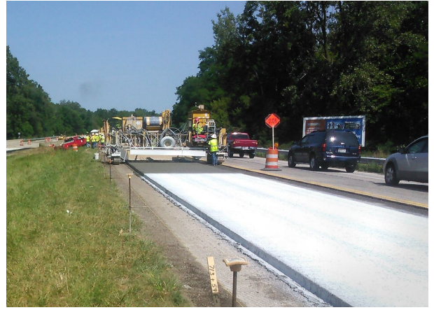
Crews install a concrete overlay. Source: FHWA
