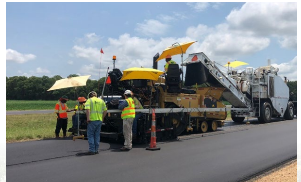
Crews install an asphalt overlay. Source: National Asphalt Pavement Association
