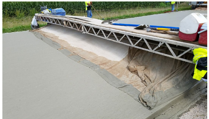
Concrete overlay Source: FHWA
