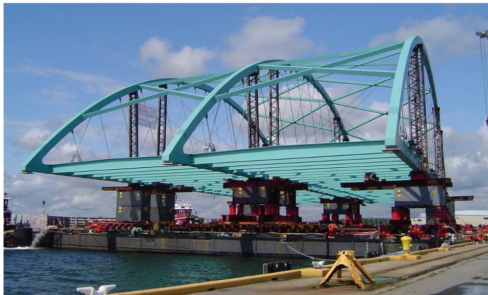
Figure 2.4.1-3 SPMT Bridge Move in Rhode Island
