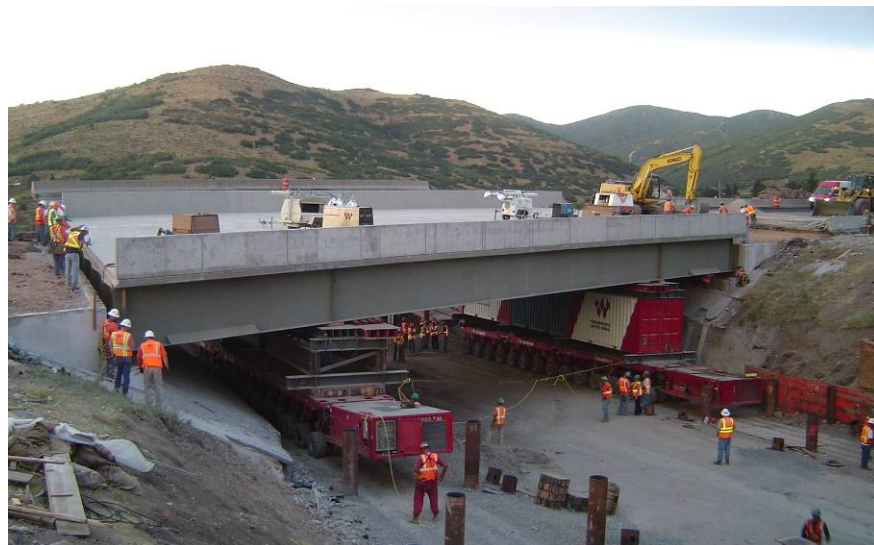
Figure 2.6.1.2-1 Superstructure Installation Using SPMTs
