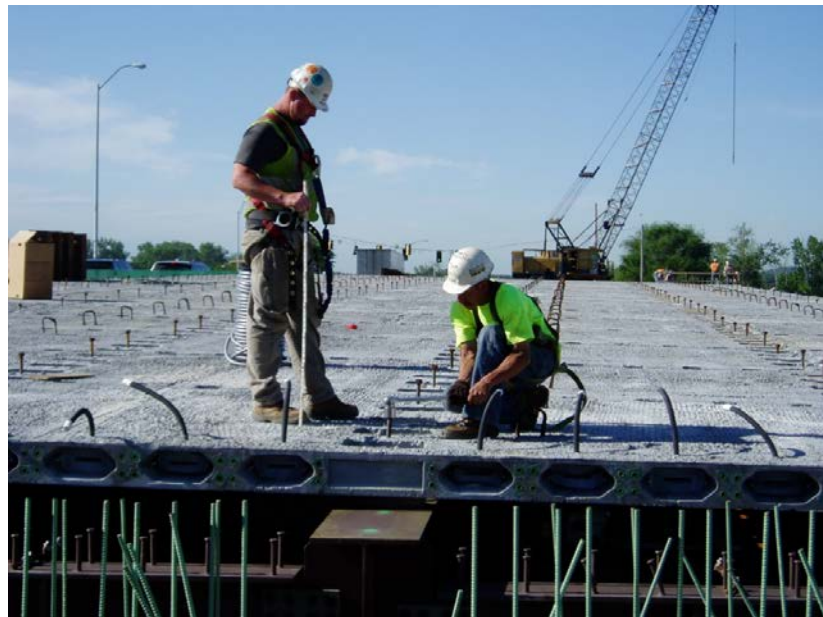
Figure 5.2.3.1-2 Precast Full Depth Deck Leveling System
