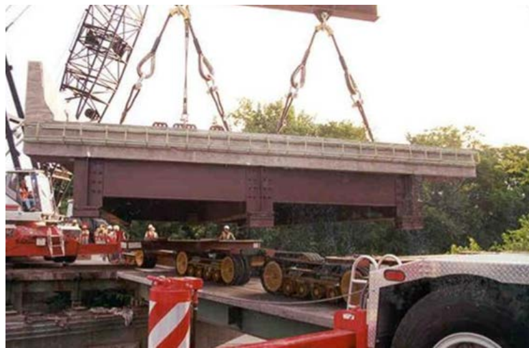
Figure 2.3.1-3 Modular Steel Superstructure Element Installation James River Bridge, Richmond, VA
