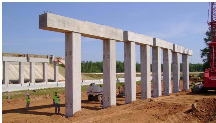
Figure 5.3.1.1-3 Precast Open Frame Pier Bent
