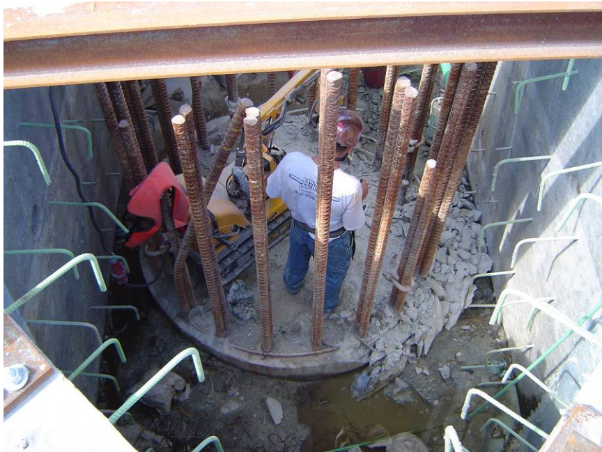
Figure 5.4.3.3-1 Precast Concrete Pier Box Cofferdam Top photo: Exterior View Bottom Photo: Interior View (source: Cardi Corporation)
