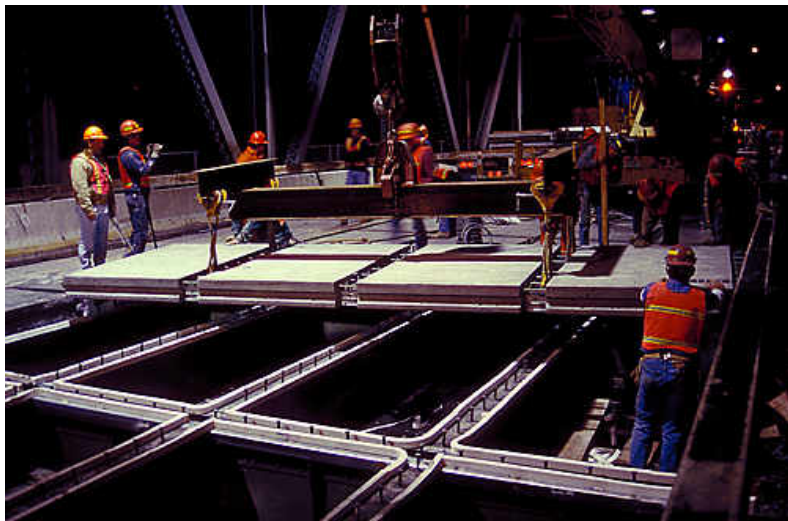
Figure 5.2.3.2.2-2 Exodermic Deck Installation (source: D.S. Brown Company)
