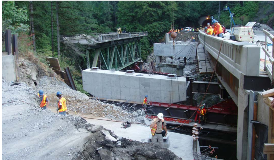
Figure 2.4.3-2 Lateral Bridge Slide in Oregon
