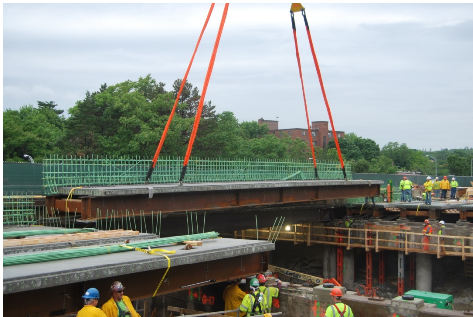
Figure 2.3.1-5 I-93 Superstructure Replacement Construction
