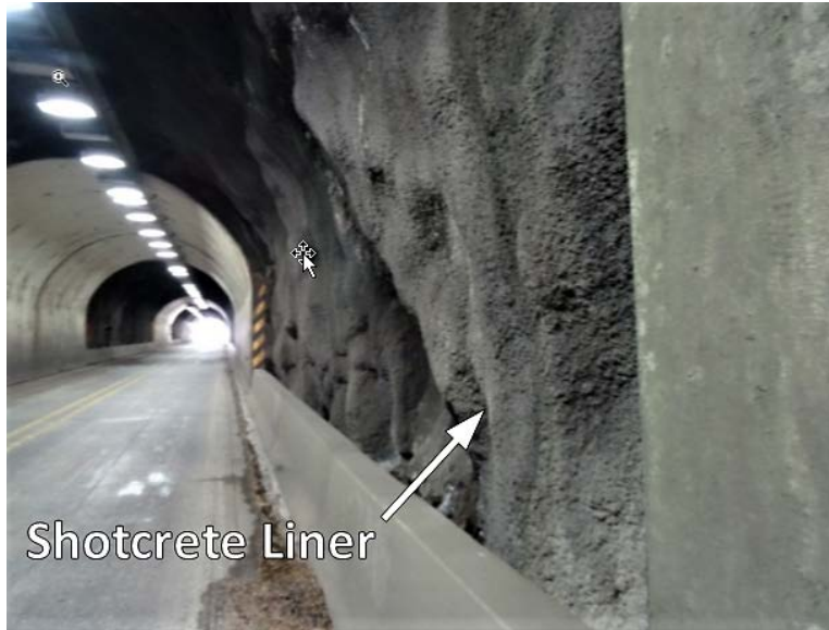
Figure 5. Photo. Shotcrete tunnel liner.
