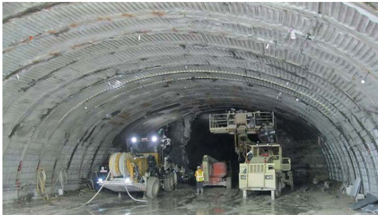
Figure 6. Photo. Steel ribbed tunnel liner.
