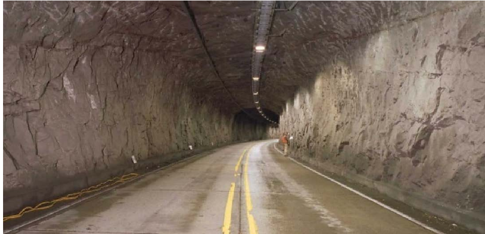
Figure 4. Photo. Unlined rock tunnel.
