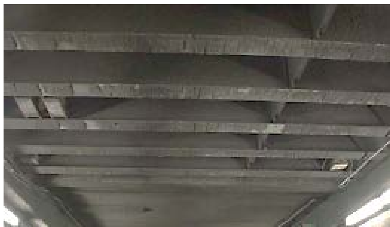
Figure 18. Photo. Girder-supported roof.
