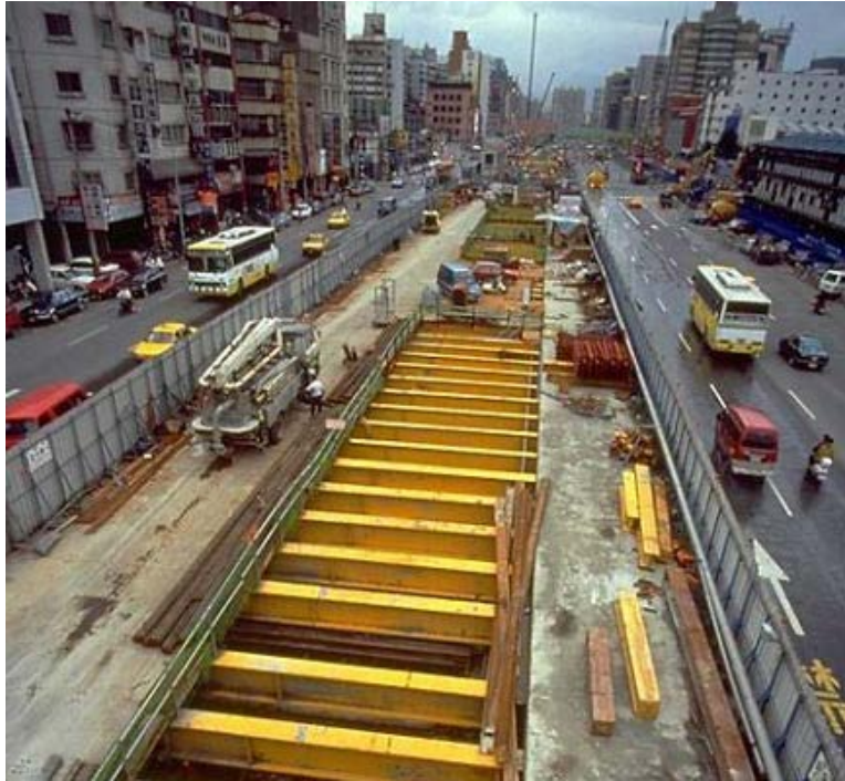
Figure 9. Photo. Braced slurry wall tunnel construction.
