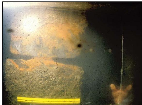
Figure 3-27 H-pile Corrosion Below Concrete Encasement
