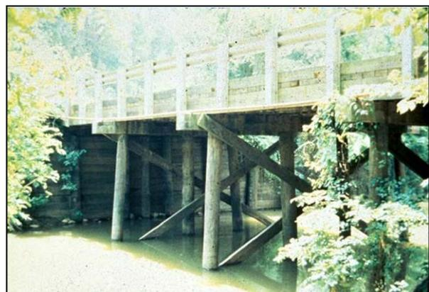
Figure 3-3 Timber Pile Bents and Timber Pile Abutment
