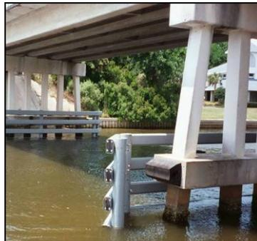
Figure 3-8 Composite Pile and Wale Fender System
