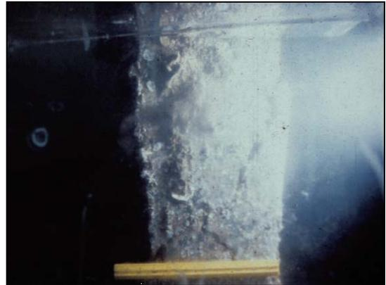
Figure 3-21 Cracked Concrete Pile
