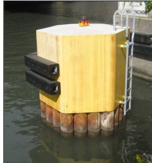
Figure 3-16 Steel Pipe Pile Dolphin with Concrete Cap
