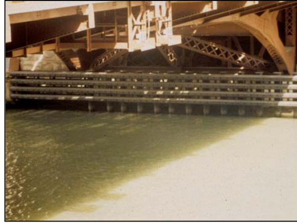
Figure 3-18 Pile Supported Fender System
