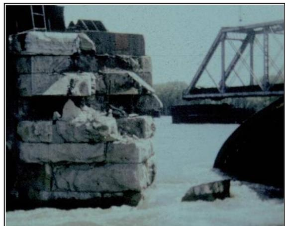
Figure 3-41 Vessel Damage
