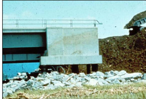
Figure 3-4 Exposed Timber Piles at Scoured Abutment
