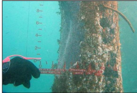
Figure 4-14 Graphic Scale with Location Shown
