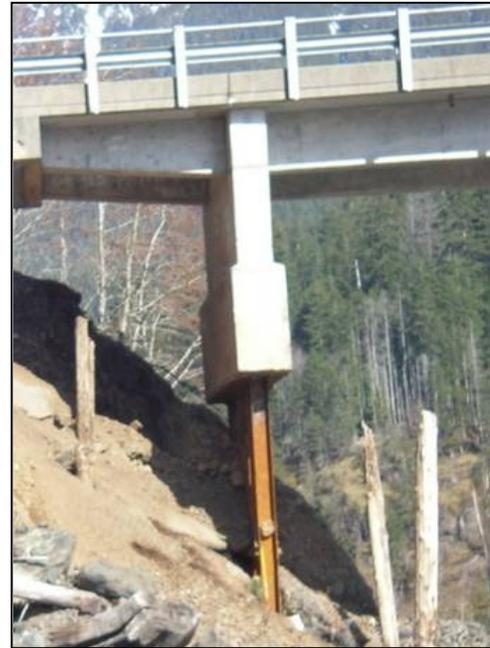
Figure 3-6 Concrete Pier Supported by Steel H-Piles
