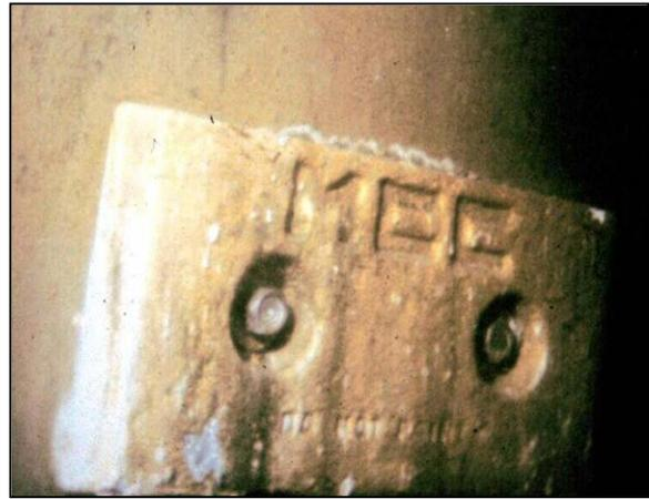
Figure 3-33 Sacrificial Anode on Steel Pipe Pile
