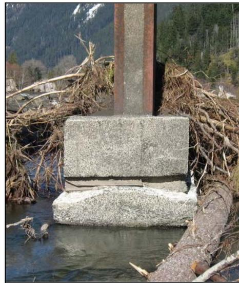
Figure 3-14 Foundation Seal Under Pier Exposed by Scour
