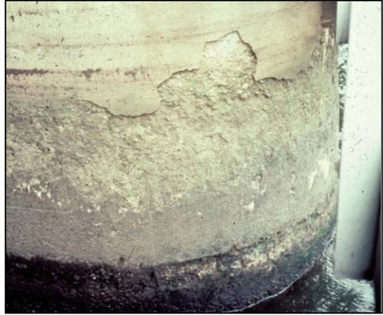
Figure 3-22 Scaling of Pier at Waterline
