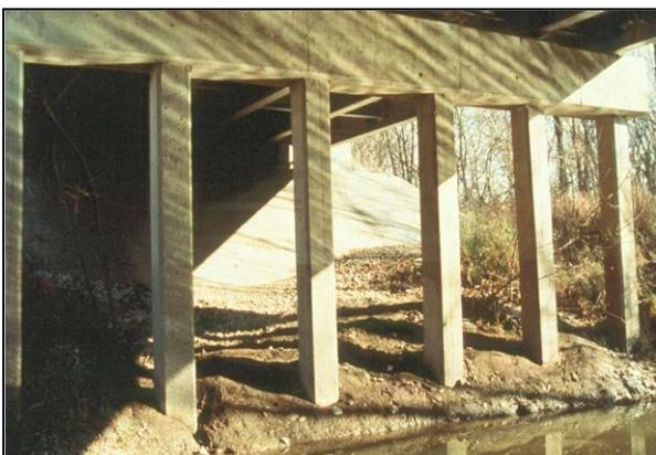
Figure 3-2 Concrete Pile Bent at Low Water
