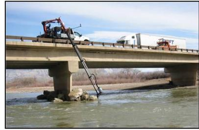
Figure 6-18 Transducer on Articulated Head
