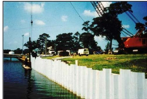
Figure 3-9 Composite Sheet Piling
