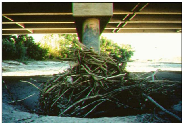
Figure 6-9 Debris Increasing Width of Pier
