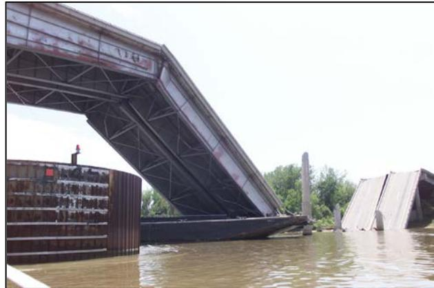
Figure 1-6 Vessel Impact Damage at I-40 Bridge over Arkansas River, Oklahoma (2002)
