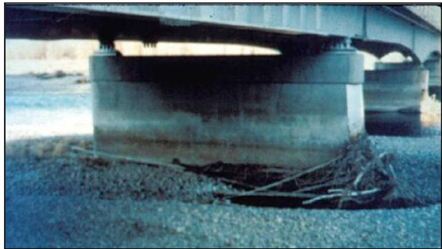
Figure 6-8 Upstream Scour Hole and Debris with Downstream Deposition of Material Shown in Dry
