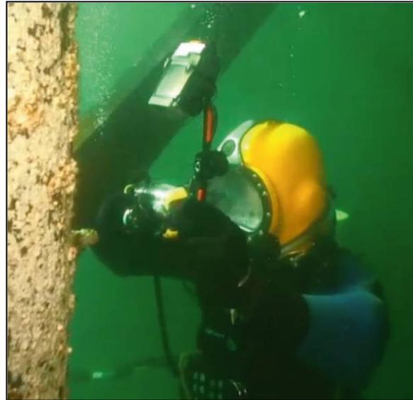
Figure 4-13 Underwater Camera and Strobe Unit
