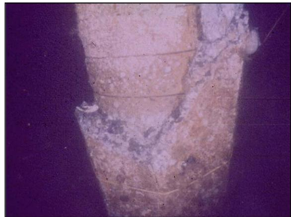
Figure 3-25 Pile Damaged by Delayed Ettringite Formation
