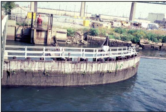
Figure 3-19 Timber Shear Fence
