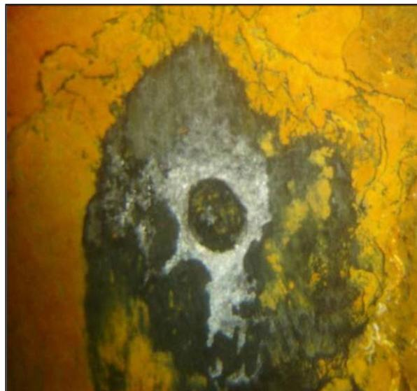
Figure 3-29 Steel Sheet Pile with MIC
