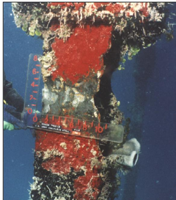
Figure 1-3 Level II Cleaning of a Steel H-Pile
