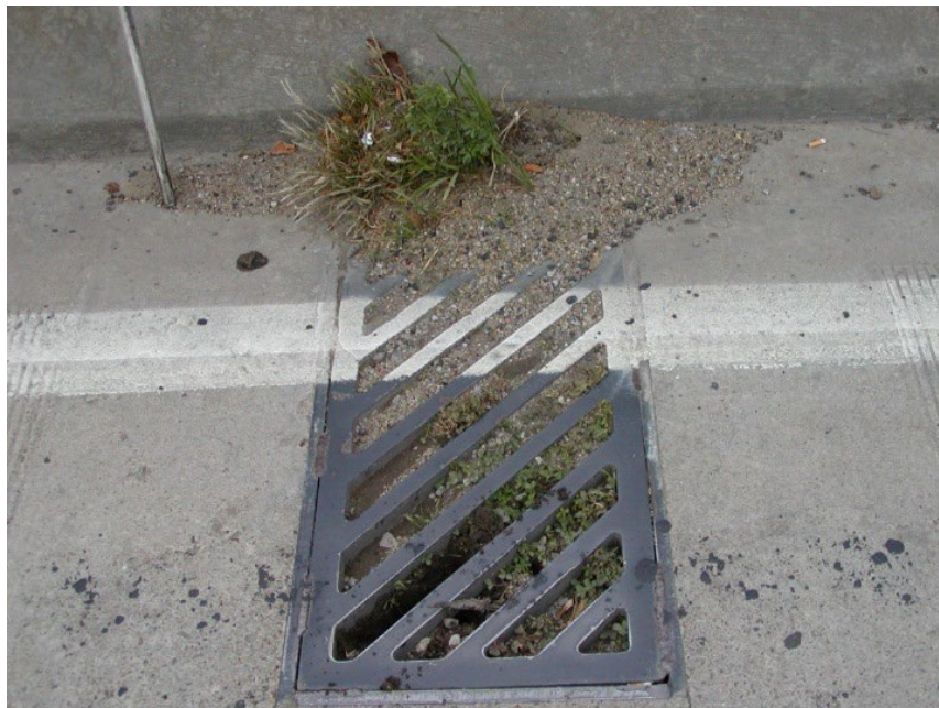
Figure 8.5.31 Clogged Scupper
