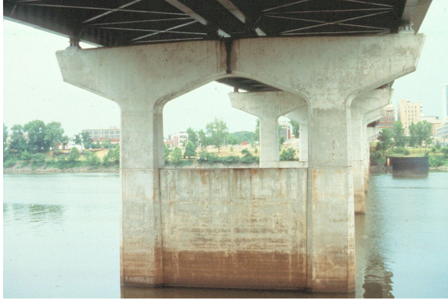
Figure 14.2.53 Cantilevered Piers Joined by a Web Wall
