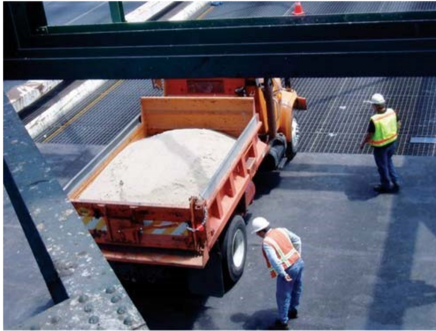
Figure 8.4.5 Use of Truck for Visual Inspection of FRP Deck
