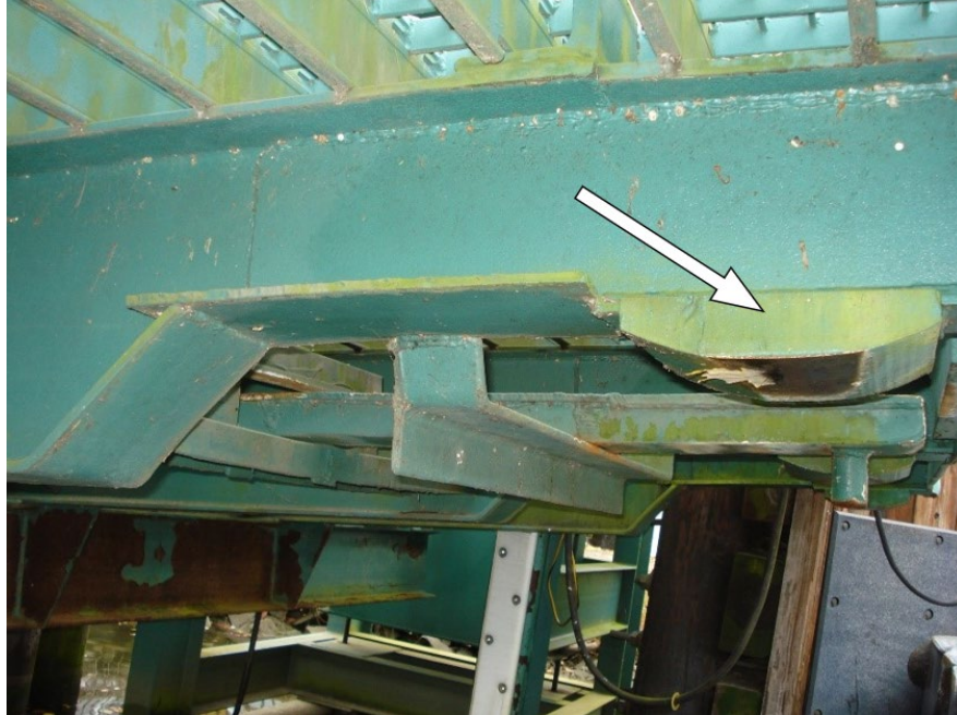
Figure 5.5.4 Fixed Shoe Bearing
