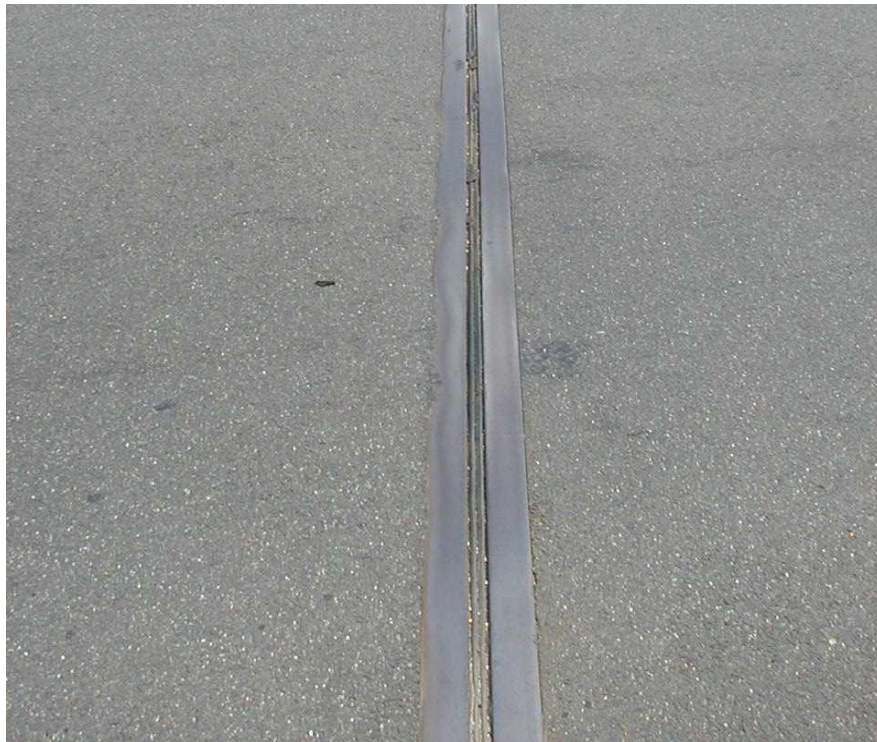
Figure 4.1.40 Top View of an Armored Compression Seal in Place
