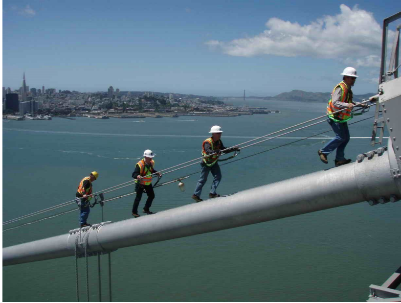
Figure 2.5.21 Handrail on Suspension Bridge
