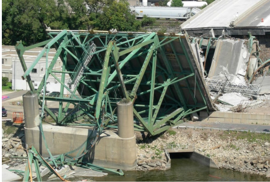
Figure 10.5.4 I-35W Mississippi River Bridge Collapse
