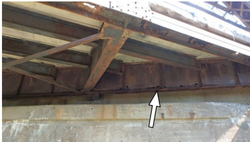
Figure 10.4.27 Corroded Floorbeam
