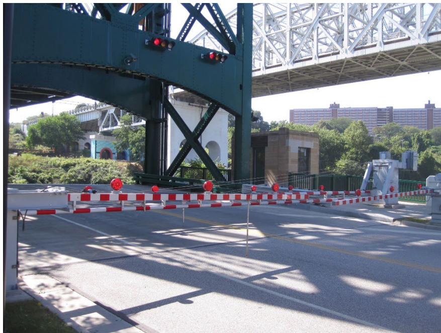
Figure 12.3.2 Movable Bridge Traffic Control Gate
