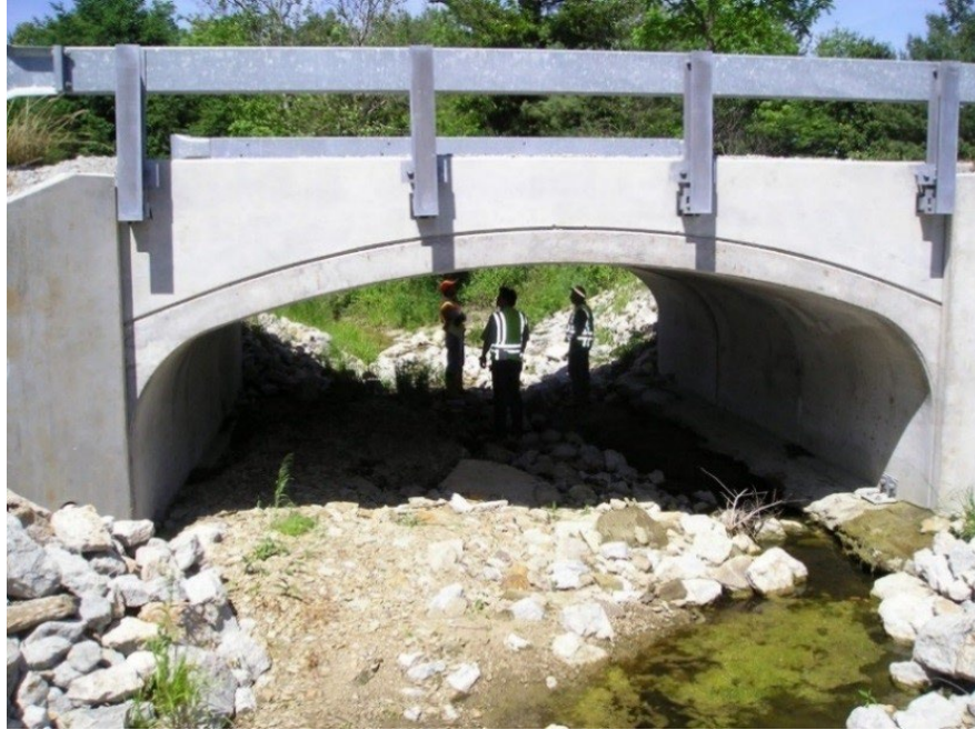
Figure 4.2.6 Precast Frame Culvert
