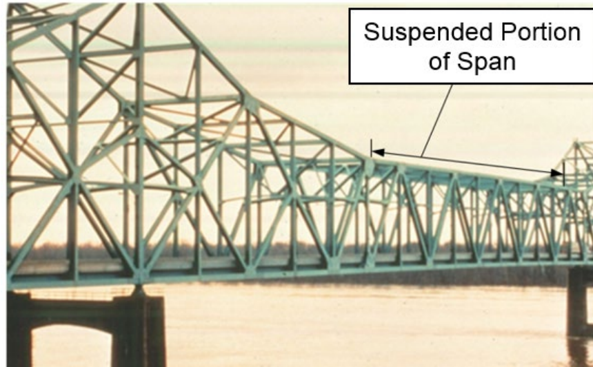
Figure 10.1.38 Cantilever Through Truss
