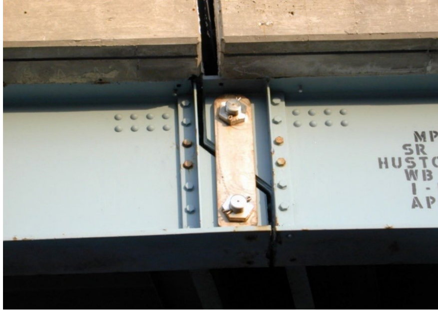
Figure 10.1.84 Stainless Steel Pin-and-Hanger Assembly Retrofit
