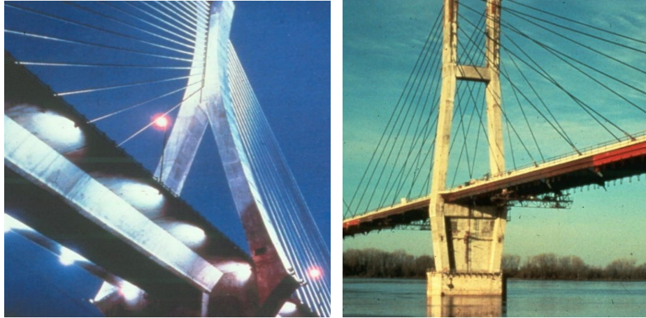
Figure 5.2.28 Single and Double Vertical Plane Cable System
