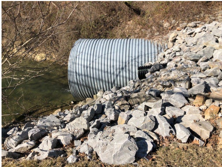
Figure 15.5.20 Flexible Culvert Projection
