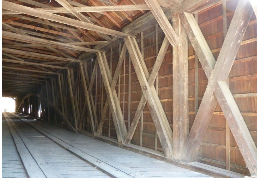
Figure 11.2.4 Inside View of Covered Bridge Showing Truss Members
