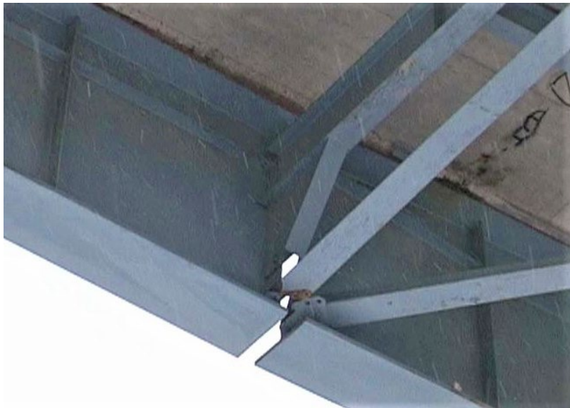
Figure 10.5.8 Fractured Girder
