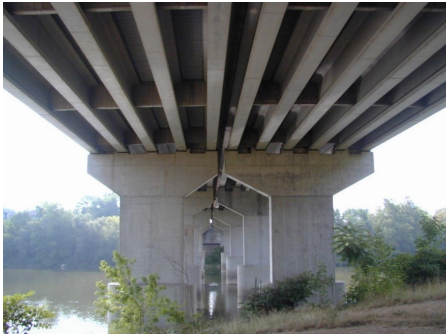
Figure 4.1.83 Pier Walls with Cantilever or Hammerhead Caps
