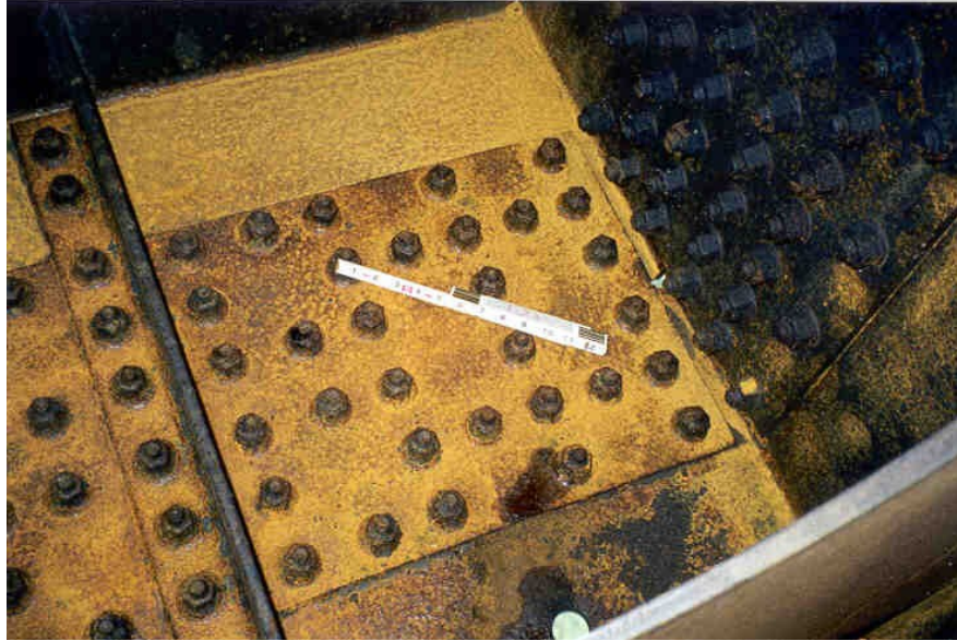
Figure 7.2.6 Yellow Orange - Early Development of the Oxide Film (Patina)
