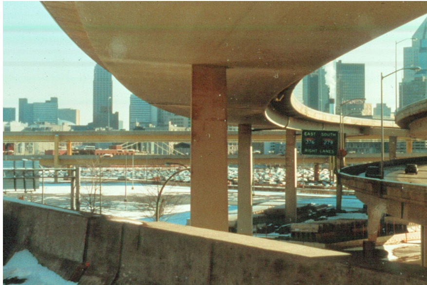
Figure 10.1.16 Single Box Girders
