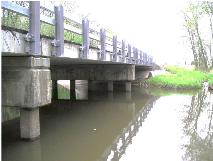
Figure 9.1.31 Typical Prestressed Slab Beam Bridge
