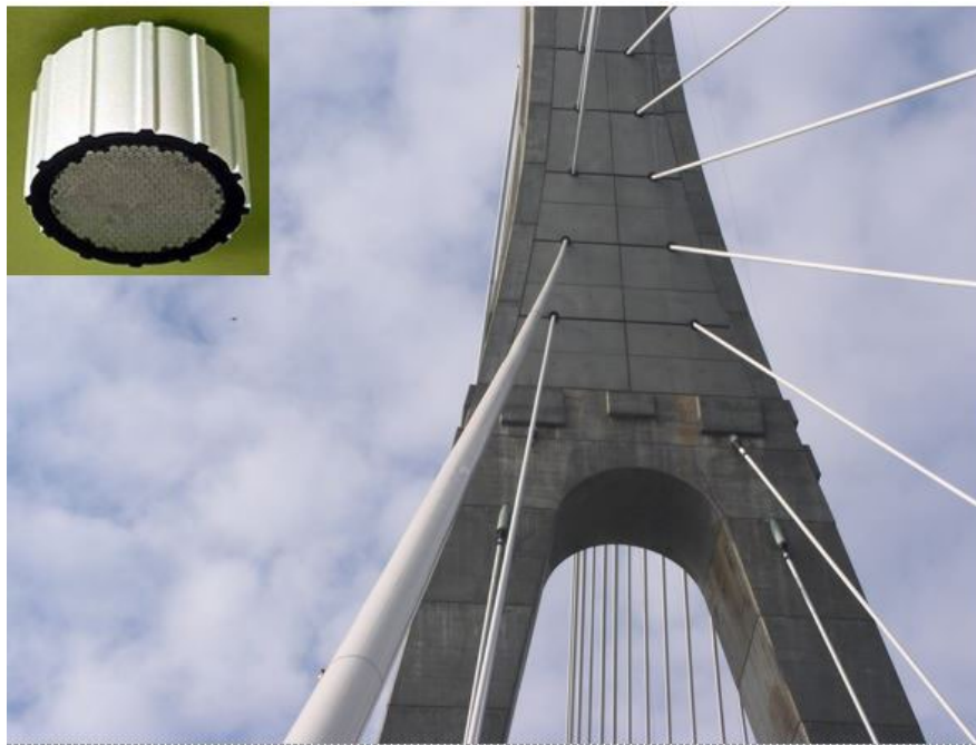
Figure 7.2.1 Steel Cables with Close-up of Cable Cross-Section showing Individual Wires
