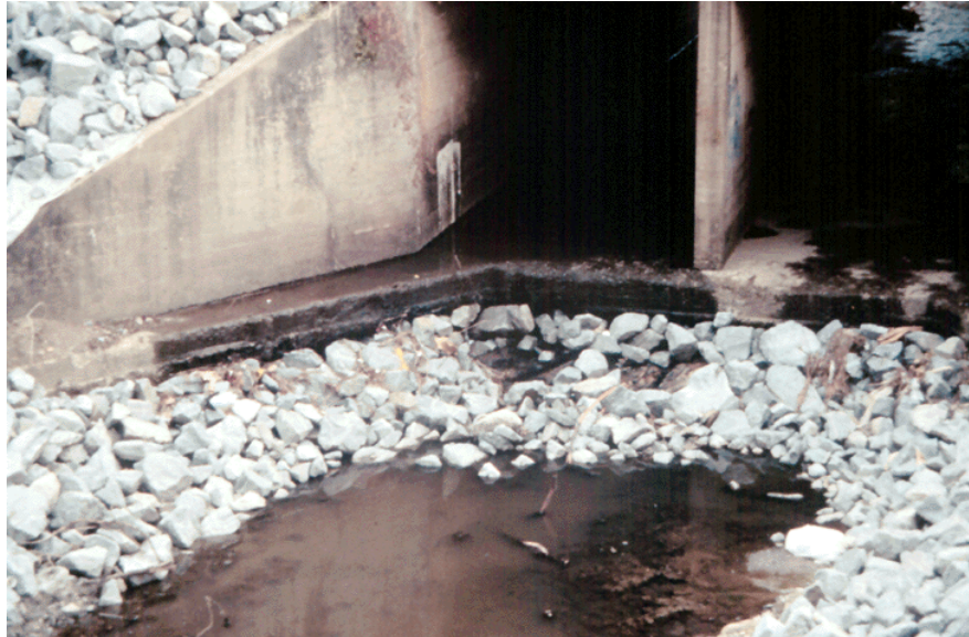
Figure 16.1.39 Failed Riprap
