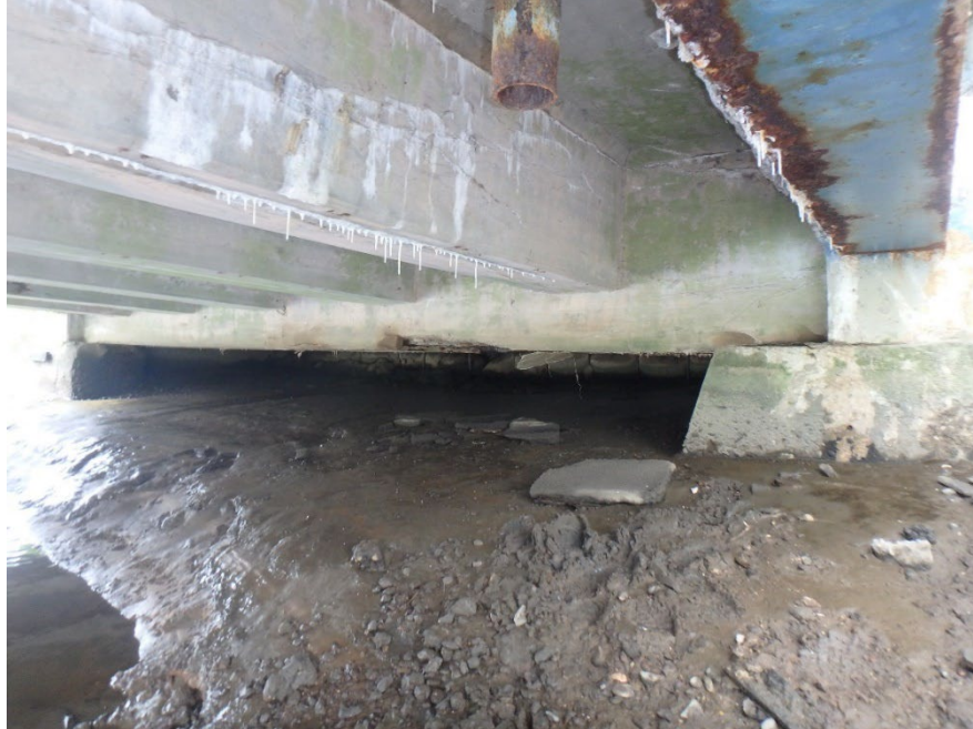
Figure 4.1.77 Spill Through or Open Abutment
