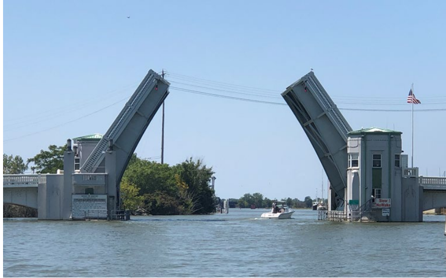
Figure 5.3.6 Double-Leaf Bascule Bridge in the Open Position
