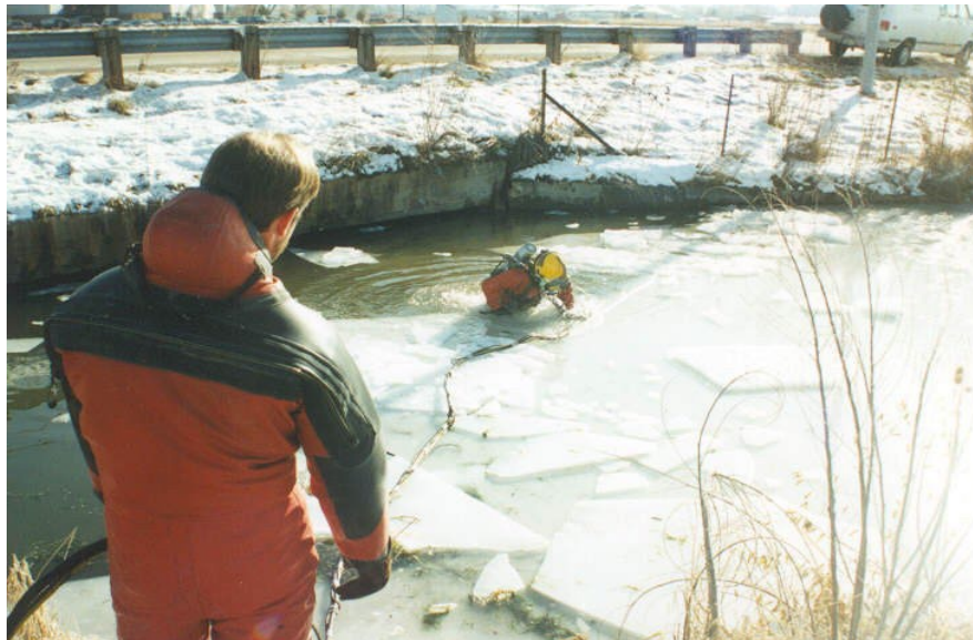
Figure 16.2.10 Inspection of Culvert with Limited Freeboard and Ice cover
