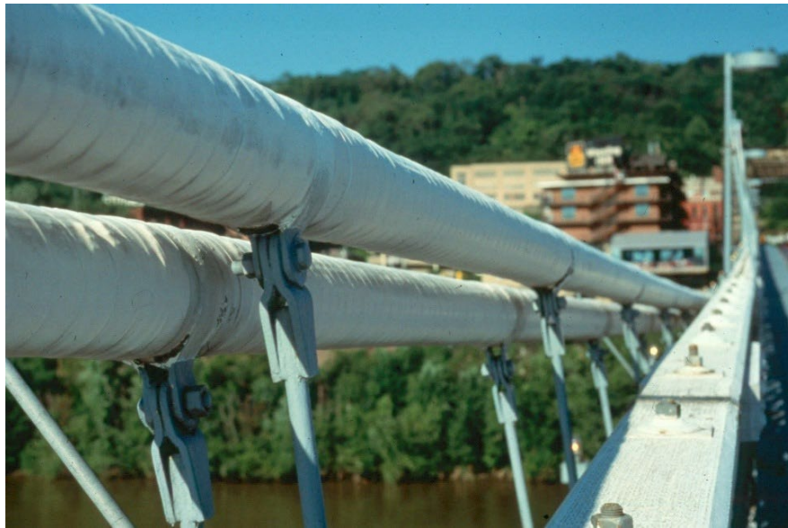
Figure 5.2.9 Cable Wrapping on Older Suspension Bridge
