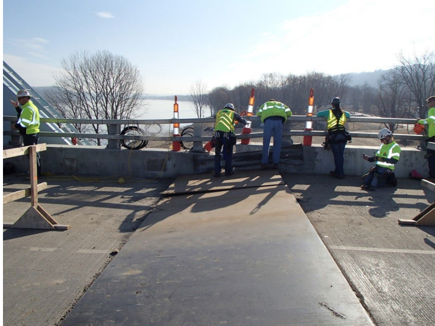
Figure 16.1.37 Superstructure Misalignment
