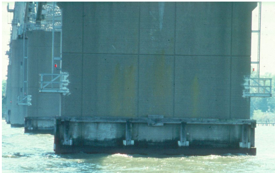
Figure 14.2.65 Steel Fender
