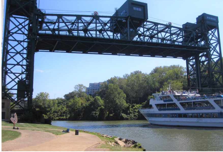
Figure 5.3.15 Span-Drive Vertical Lift Bridge
