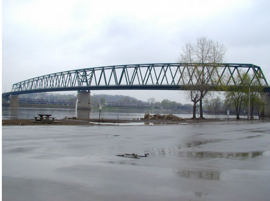
Figure 4.1.52 Through Truss Bridge
