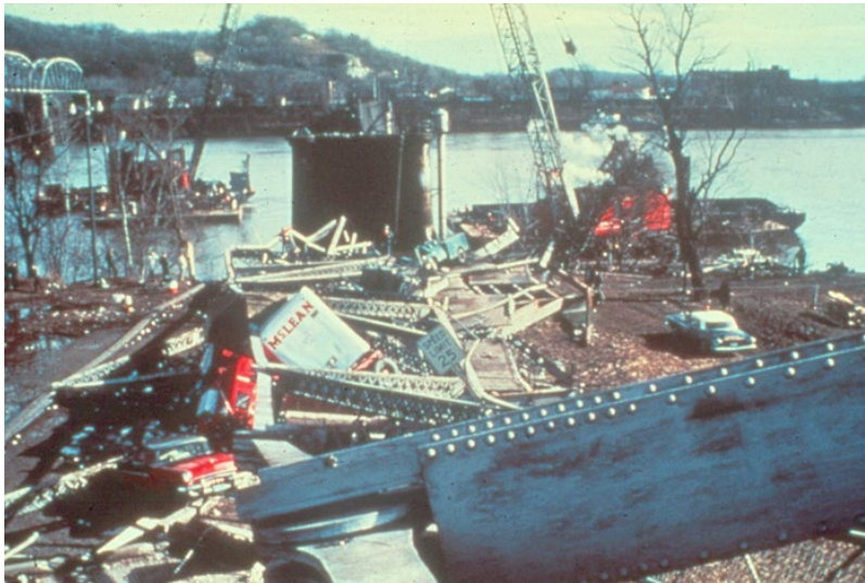
Figure 1.1.1 Silver Bridge Failure, 1967
