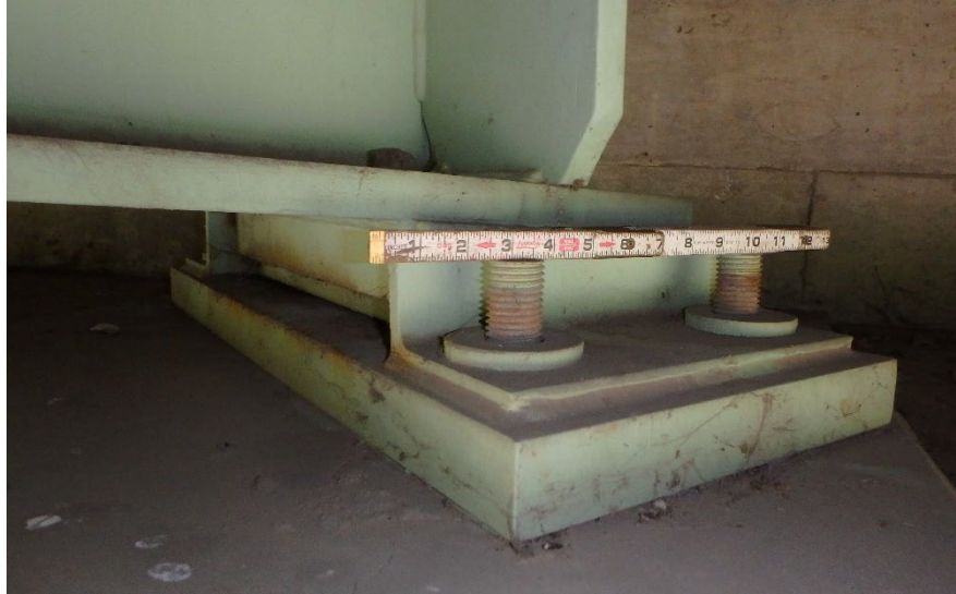
Figure 13.3.1 Lubricated Steel Plate Bearing
