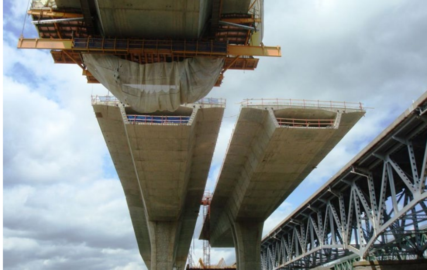
Figure 7.1.8 Post-tensioned Concrete Segmental Box Girders
