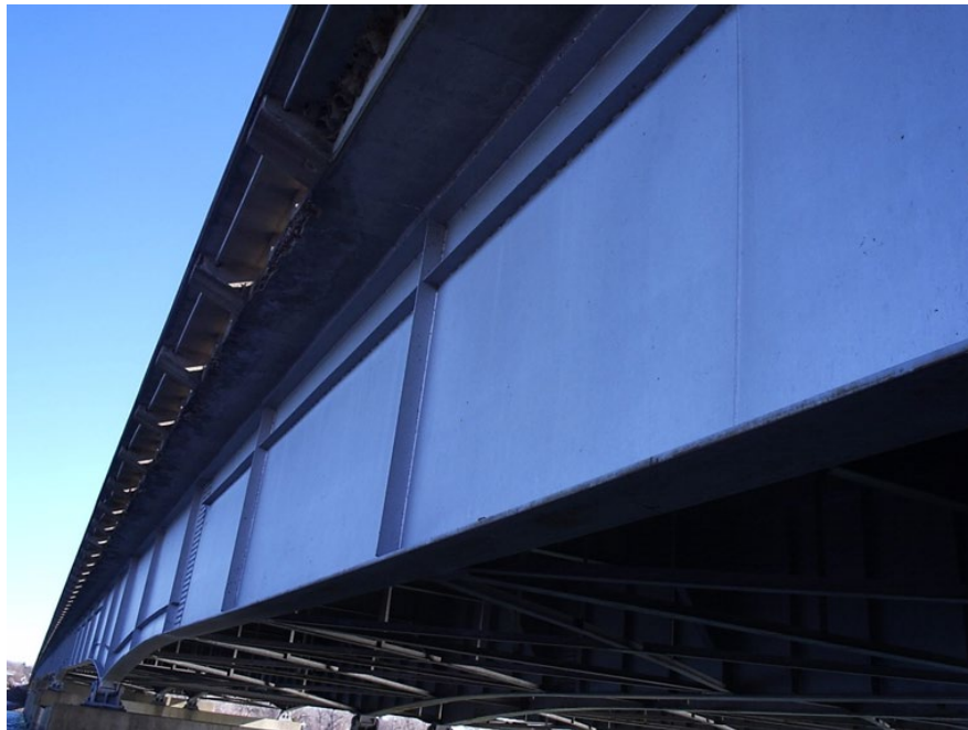
Figure 7.2.3 Welded I-Girder
