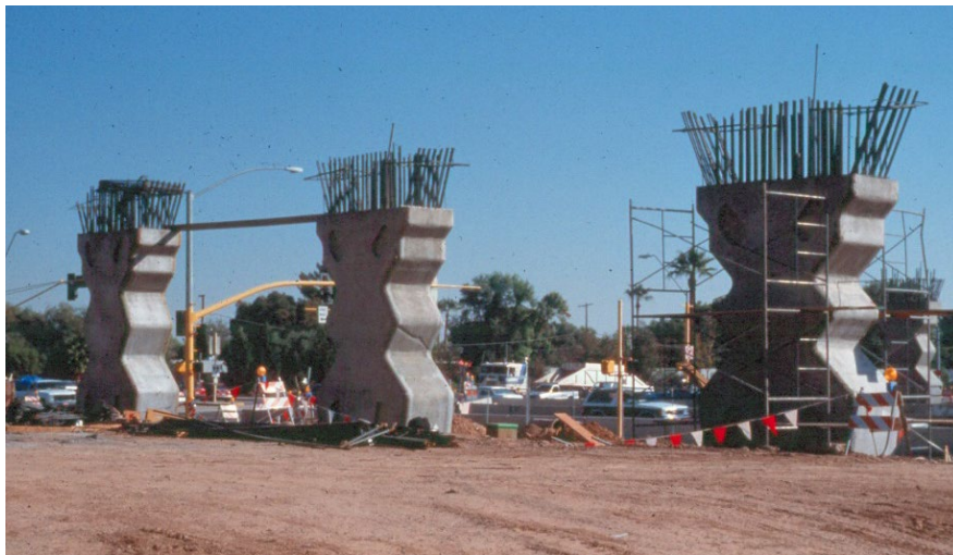
Figure 14.2.37 Reinforced Concrete Piers under Construction
