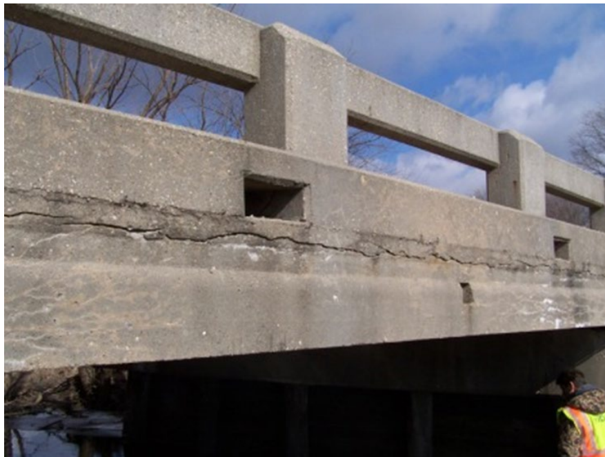
Figure 7.1.17 Longitudinal Cracks
