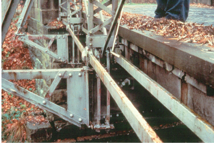
Figure 10.4.13 Bottom Chord with Eyebars
