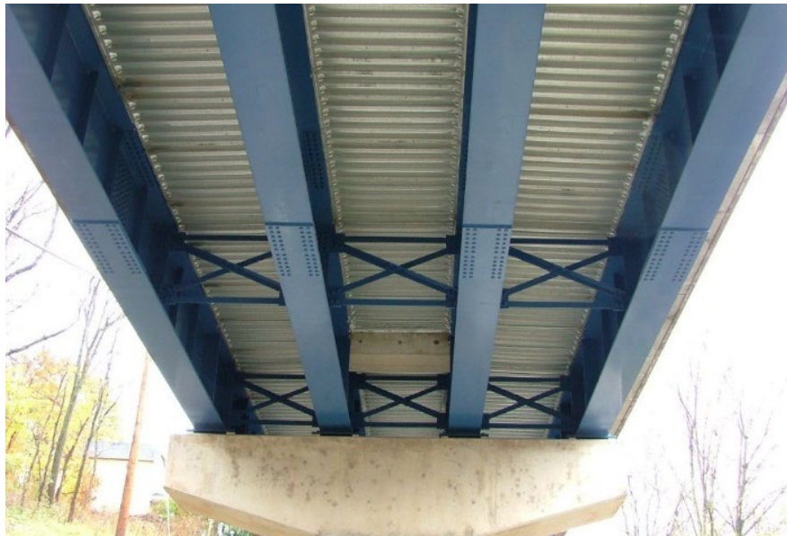
Figure 7.3.4 Load Path Redundant Girder Bridge
