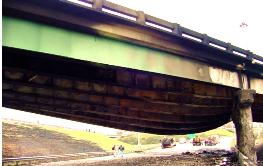
Figure 7.2.14 Heat Damage
