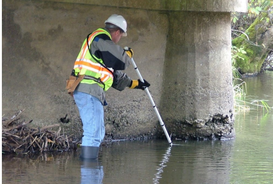
Figure 16.2.20 Inspector Wading and Probing during Inspection
