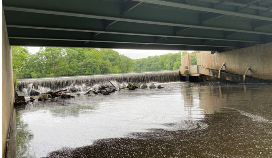
Figure 16.1.47 Upstream Dam Impacts Streamflow on Bridge
