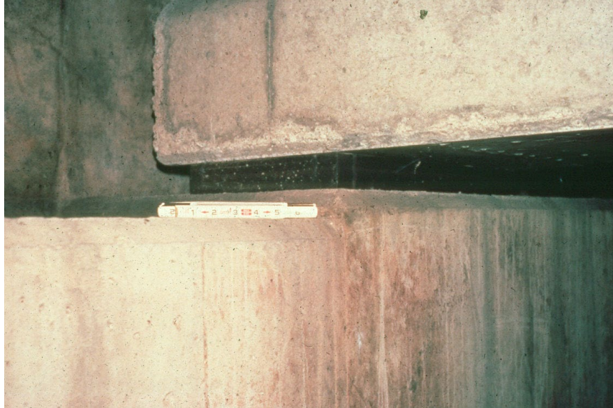
Figure 13.3.12 Plain Neoprene Bearing Pad
