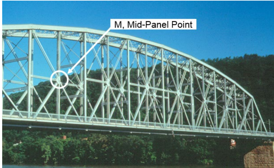
Figure 10.1.51 Pennsylvania Truss with Midpoint Panels
