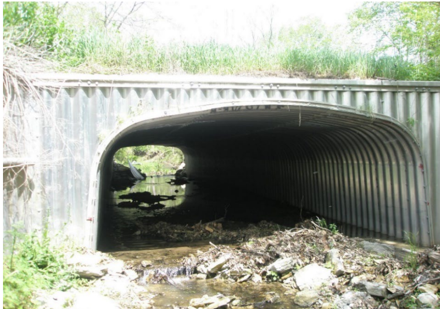
Figure 15.2.15 Flexible Box Culvert
