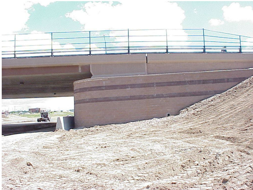
Figure 14.2.21 GRS Abutment
