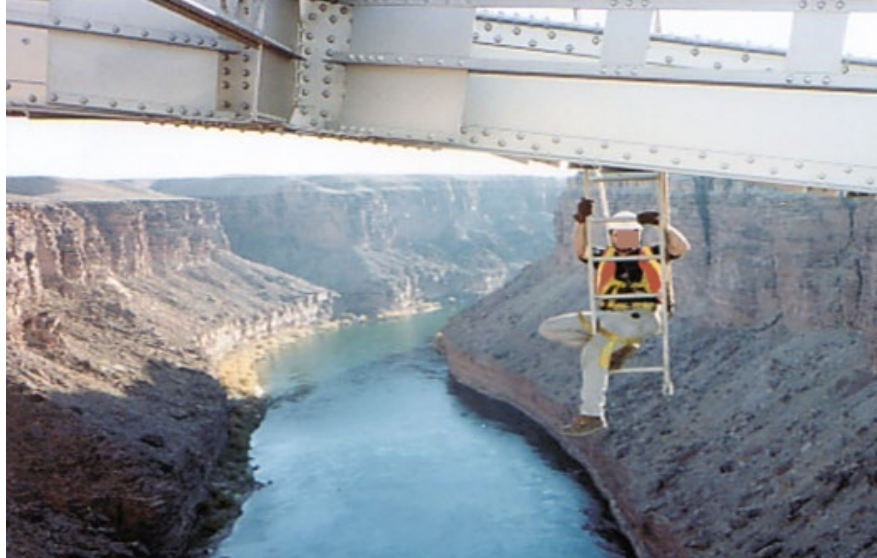
Figure 2.5.2 Inspector Using a Hook-ladder
