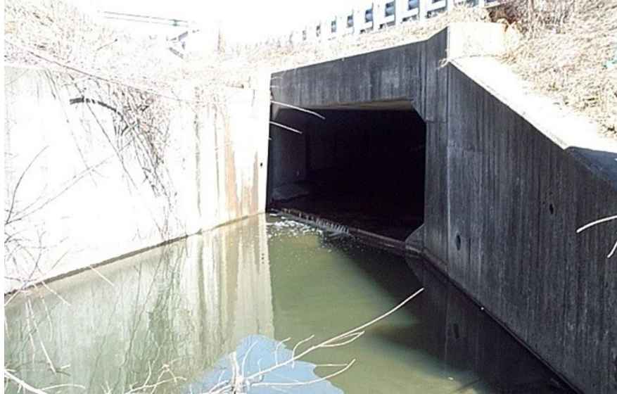
Figure 4.2.16 Culvert End
