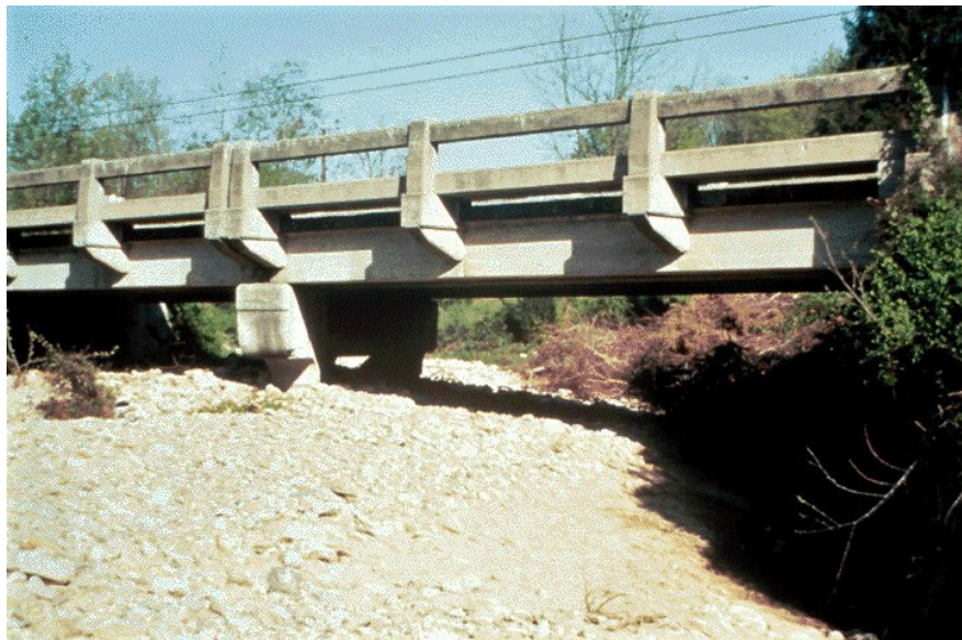
Figure 16.1.4 Streambed Aggradation
