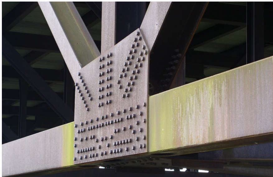
Figure 10.1.93 Gusset Plate Connecting Primary Truss Members
