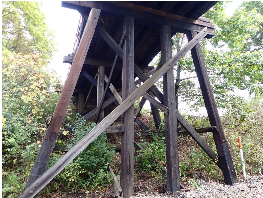
Figure 14.2.39 Pile Bent with Diagonal Bracing
