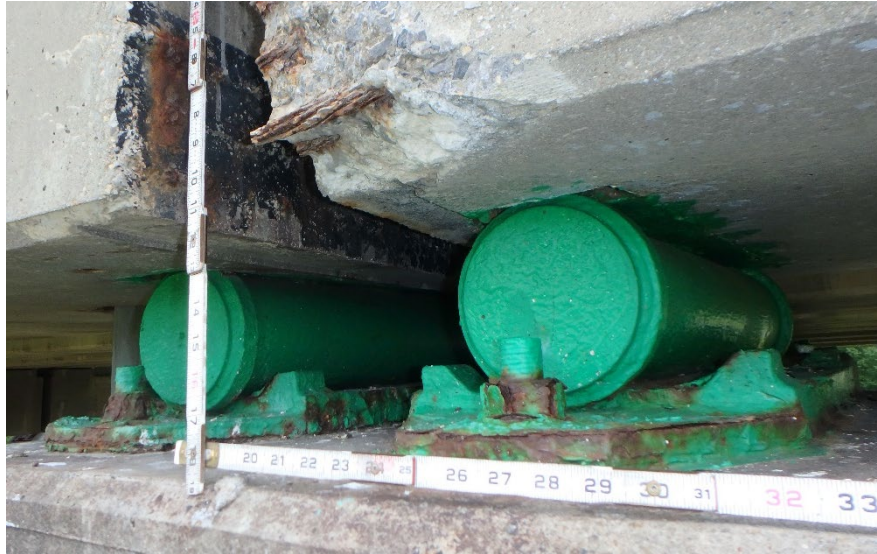
Figure 13.3.4 Single Roller Bearing
