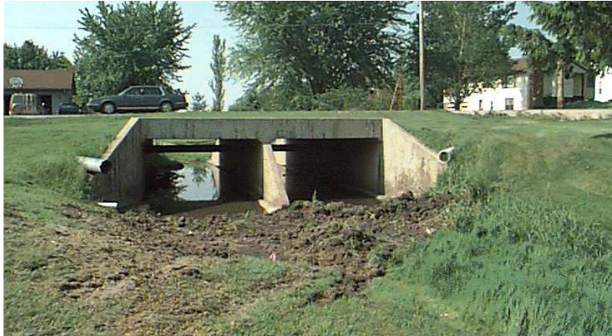
Figure 15.2.6 Concrete Frame Culvert
