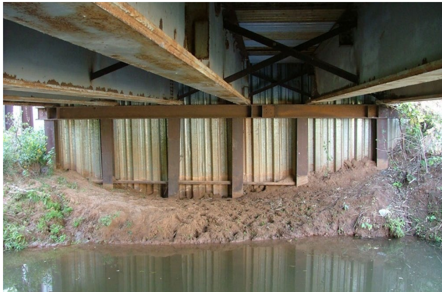
Figure 14.2.11 Steel Pile Bent Abutment
