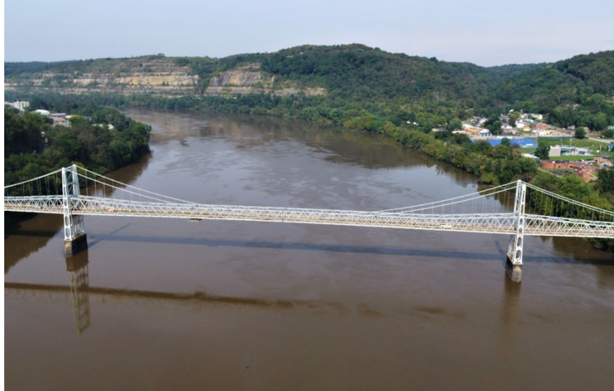
Figure 10.1.30 Suspension Bridge with Stiffening Truss
