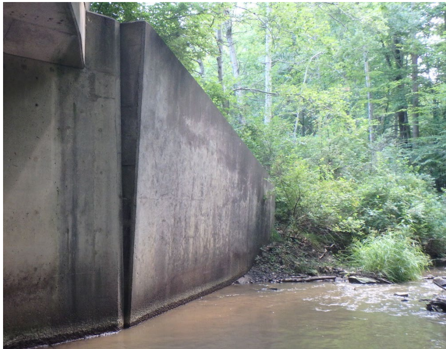
Figure 15.5.12 Tilted Wingwall
