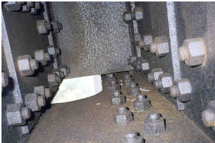
Figure 7.2.9 Black - Non-protective Oxide
