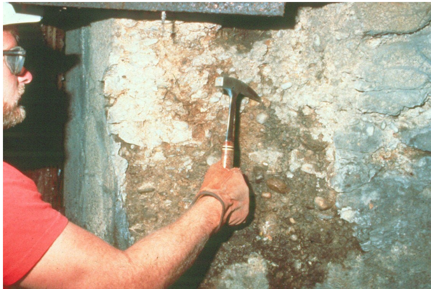
Figure 2.2.3 Inspector Wearing Safety Goggles and Gloves
