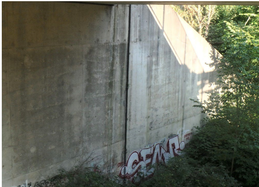
Figure 14.2.28 Typical Straight Wingwall
