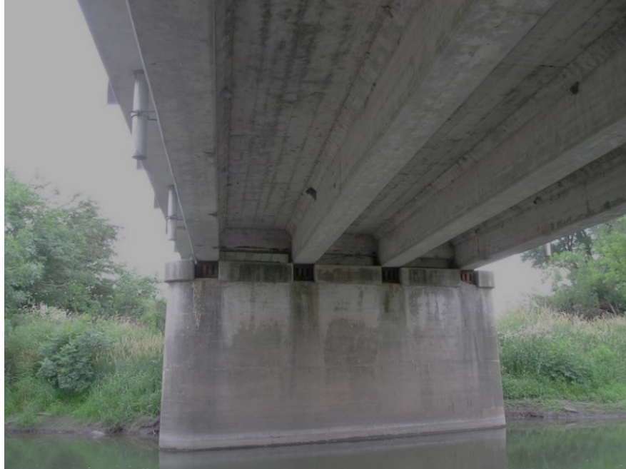
Figure 9.1.4 Simple Span Tee Beam Bridge
