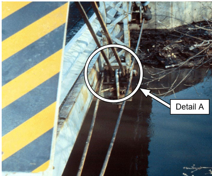
Figure 10.4.50 Eyebar Member with Unequal Load Distribution
