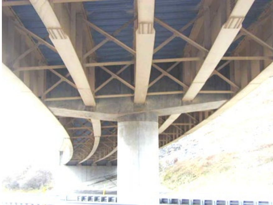
Figure 14.2.52 Concrete Column Pier with Integral Pier Cap
