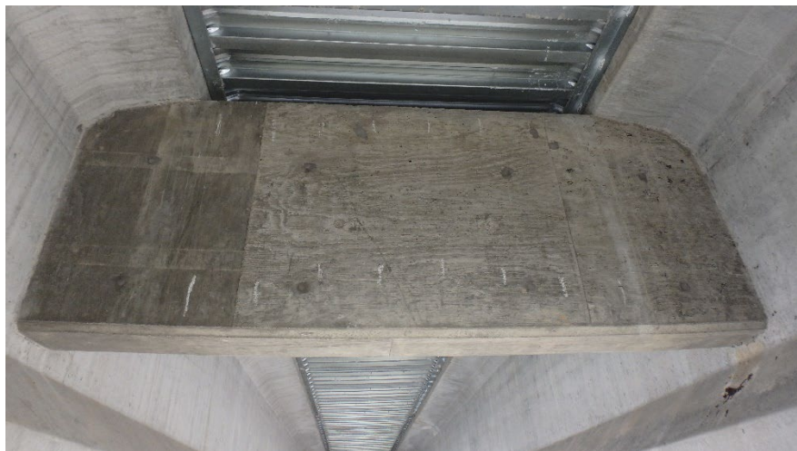
Figure 9.4.56 Intermediate Diaphragm (Secondary Member)
