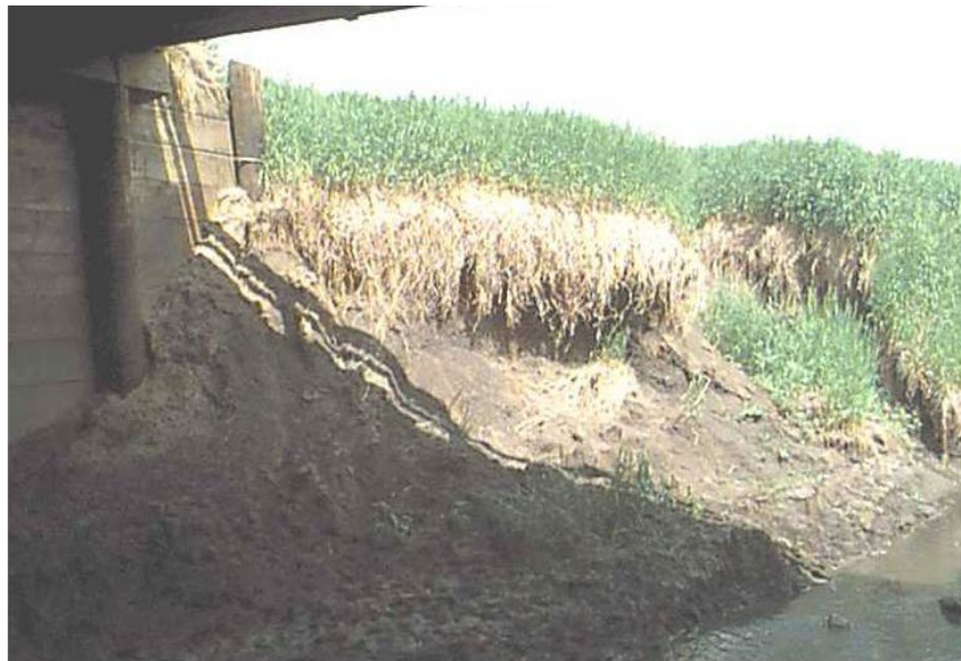
Figure 16.1.20 Undermined Streambank
