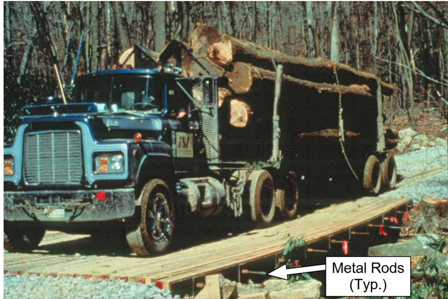
Figure 11.2.19 Stress-Laminated Timber Slab Bridge Carrying a Logging Truck
