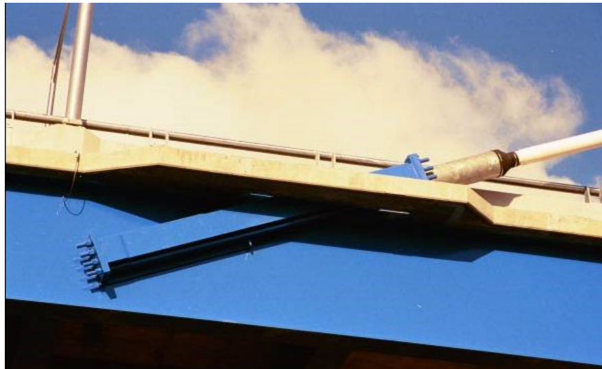
Figure 5.2.30 Cable Deck Anchorage
