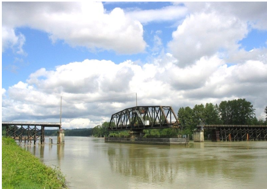
Figure 5.3.2 Center-Bearing Swing Bridge
