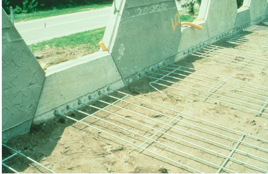
Figure 14.2.19 Mechanically Stabilized Earth Wall Under Construction
