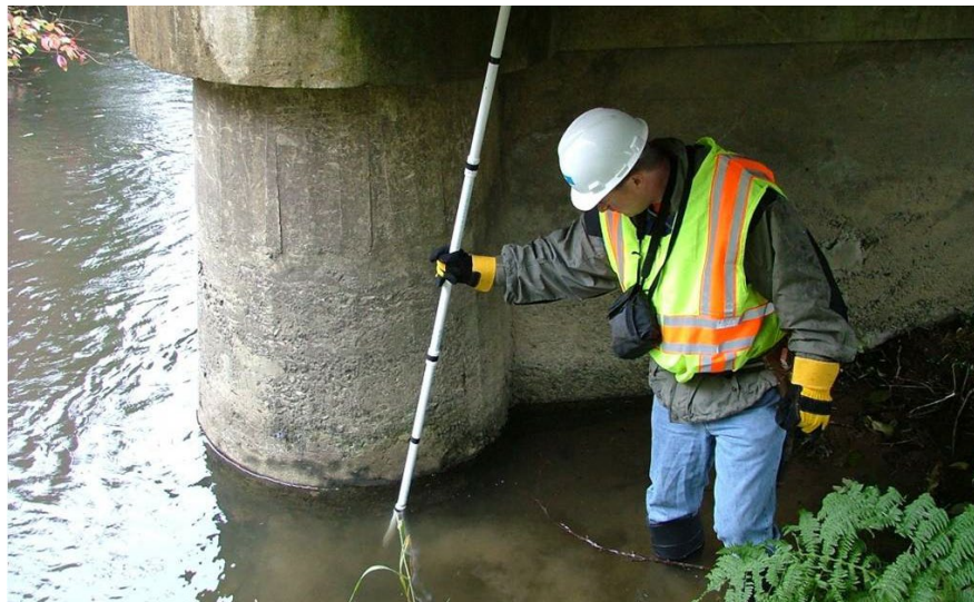
Figure 14.5.29 Inspector Checking for Scour
