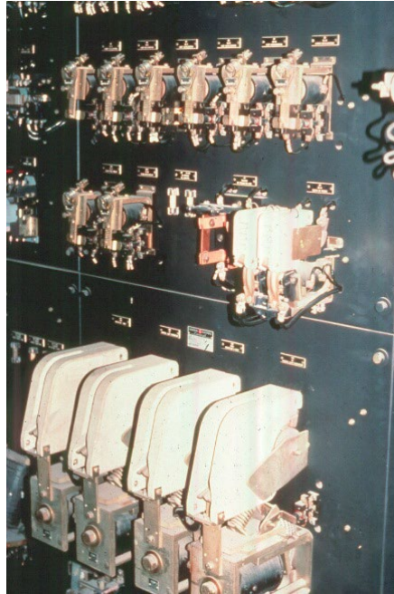
Figure 12.3.12 Open Switchboard
