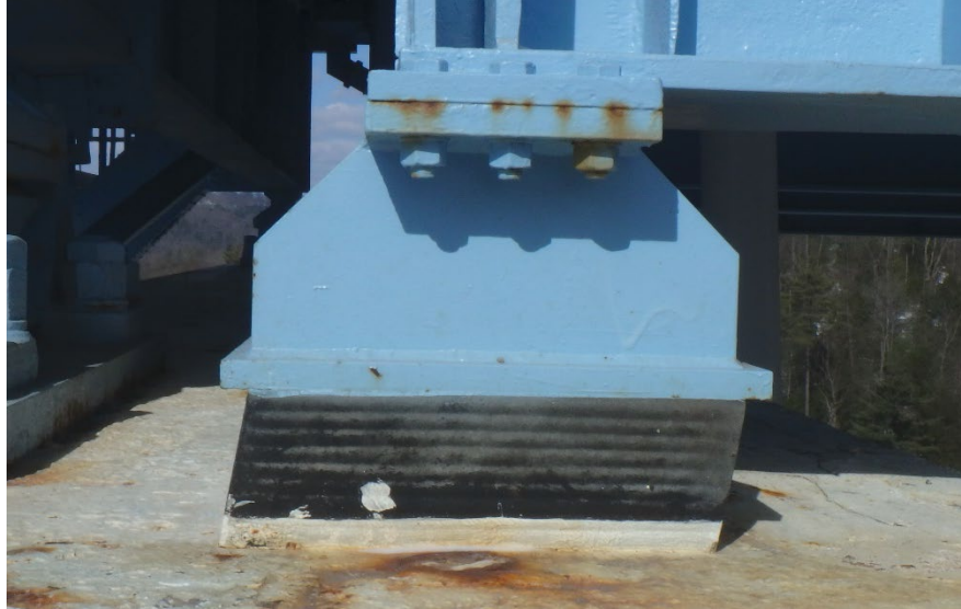
Figure 13.3.16 Laminated Neoprene Bearing Pad
