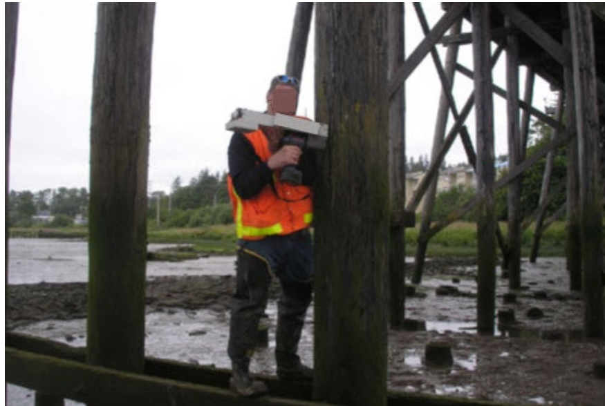
Figure 17.4.5 Inspector Using Decay Detection Device
