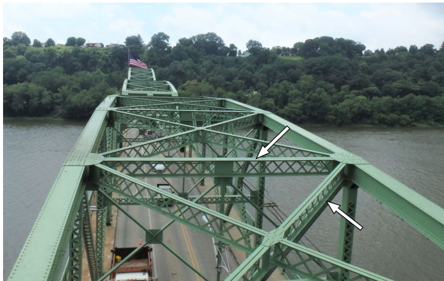
Figure 10.1.117 Upper Lateral Bracing on a Truss
