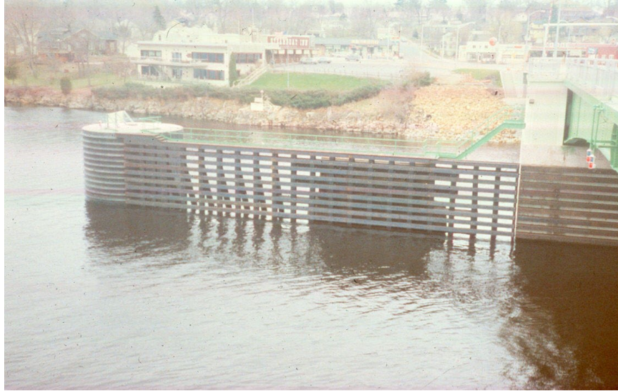
Figure 12.3.7 Pier Protection System (Fenders Shown)
