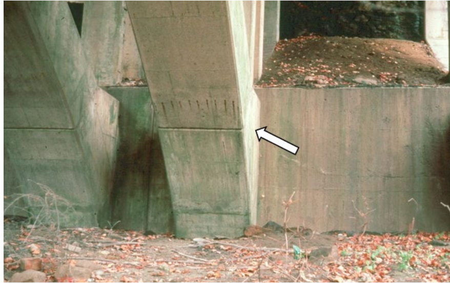
Figure 9.4.7 Bearing Area: Arch/Thrust Block Interface
