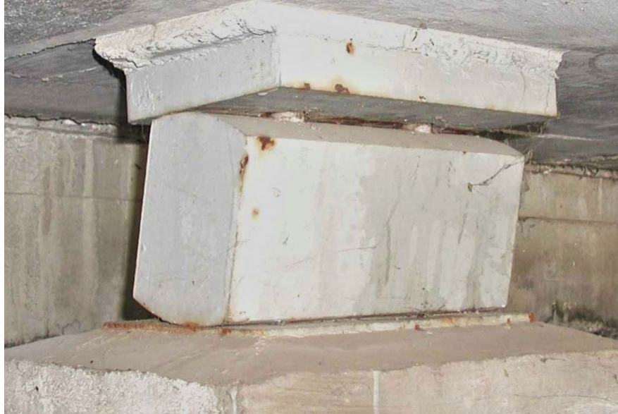
Figure 13.3.9 Segmental Rocker Bearing
