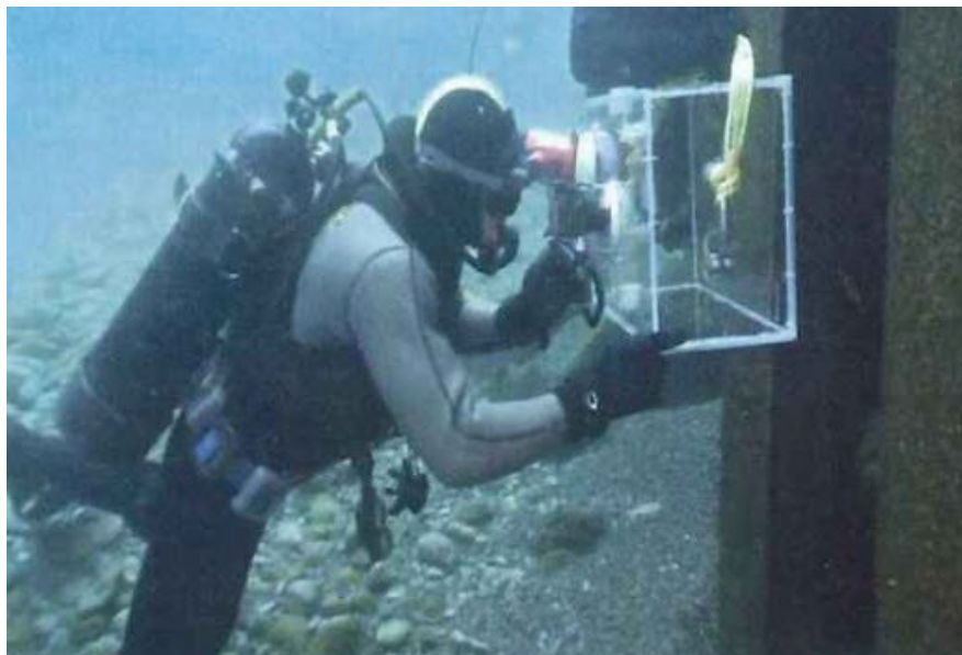
Figure 16.2.41 Diver Using a Clearwater Box
