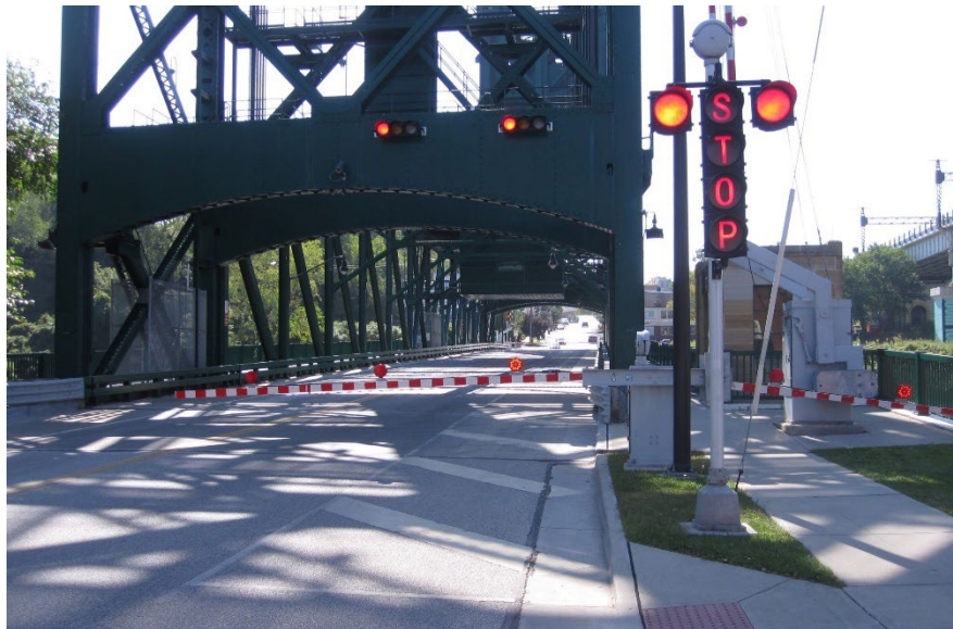
Figure 5.3.43 Traffic Barrier and Signal
