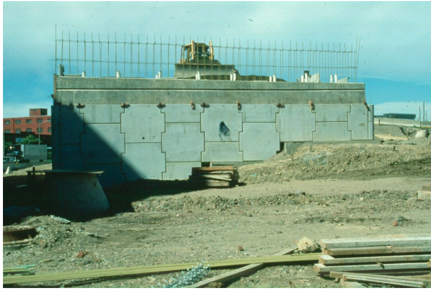
Figure 14.2.18 Mechanically Stabilized Earth Abutment
