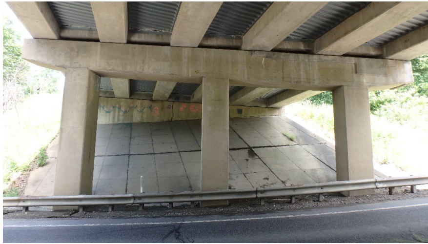
Figure 14.2.47 Column Bent or Open Bent
