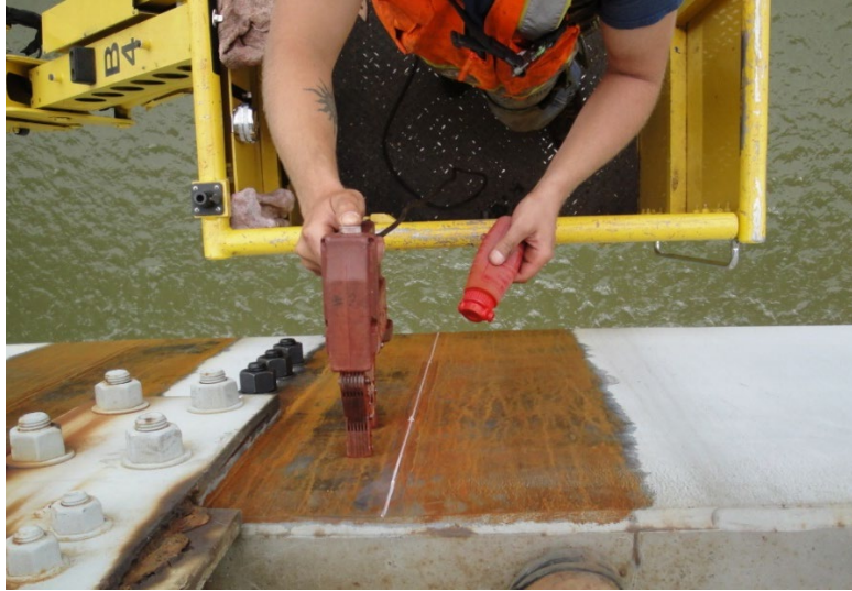
Figure 17.3.11 Magnetic Particle Testing (MT) on Member with Paint Removed
