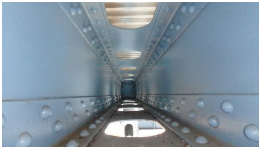
Figure 10.4.12 Inside of Box Chord Member
