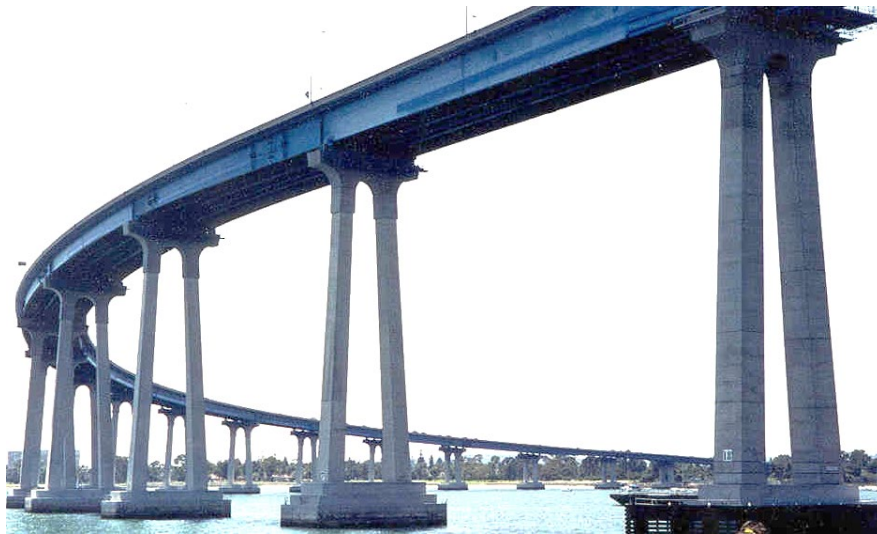
Figure 4.1.48 Steel Curved Girder Bridge
