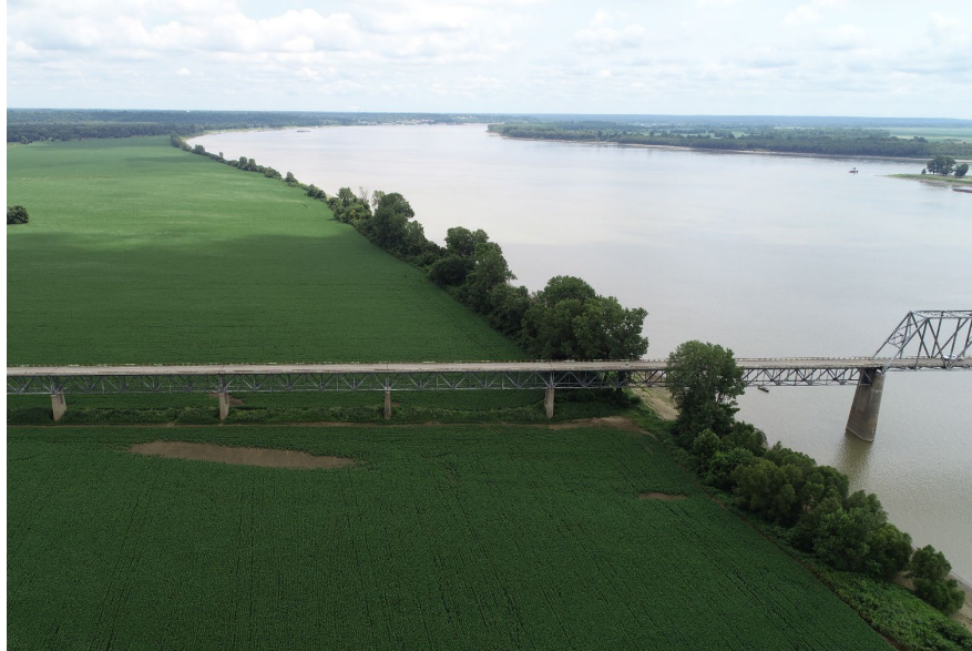
Figure 16.1.45 Approach Spans in the Floodplain
