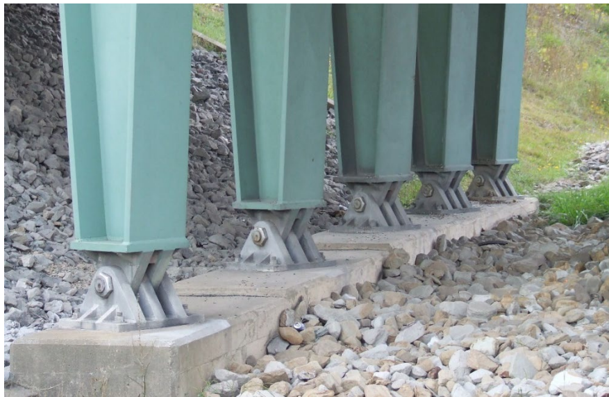
Figure 10.1.69 Rigid Frame Bearings
