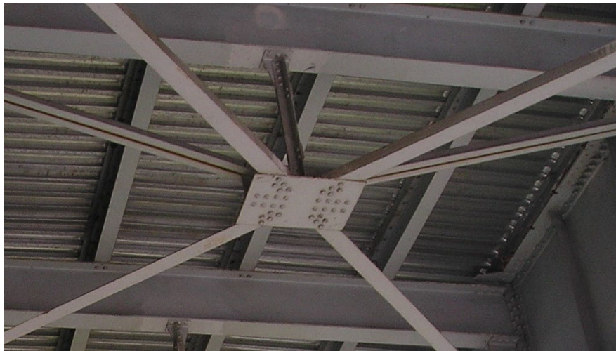
Figure 10.1.95 Gusset Plate Connecting Secondary (Bracing) Members
