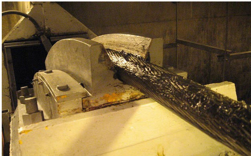
Figure 5.4.8 Anchor Cable Saddle
