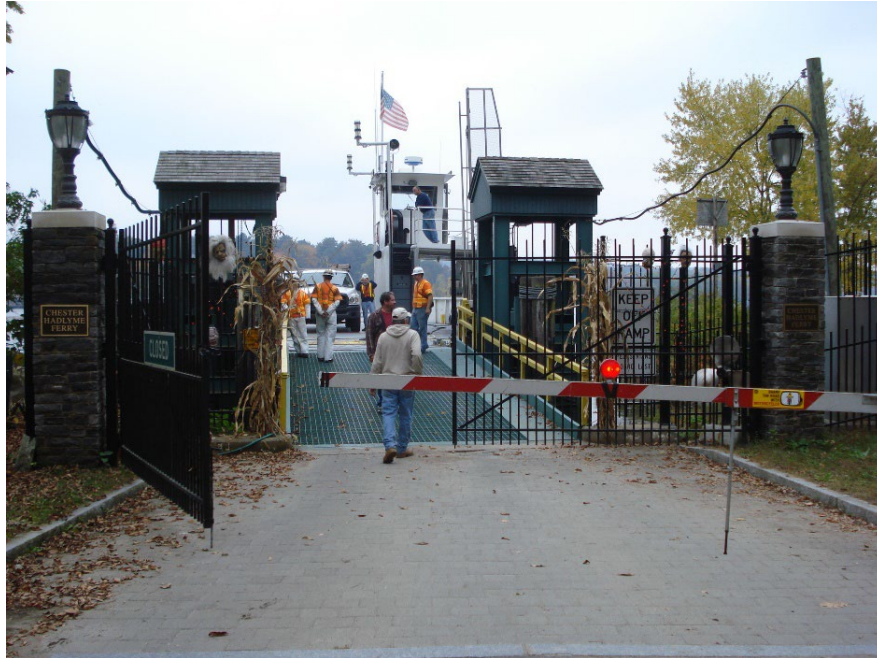
Figure 12.5.1 Ferry Transfer Bridge Traffic Control Gate
