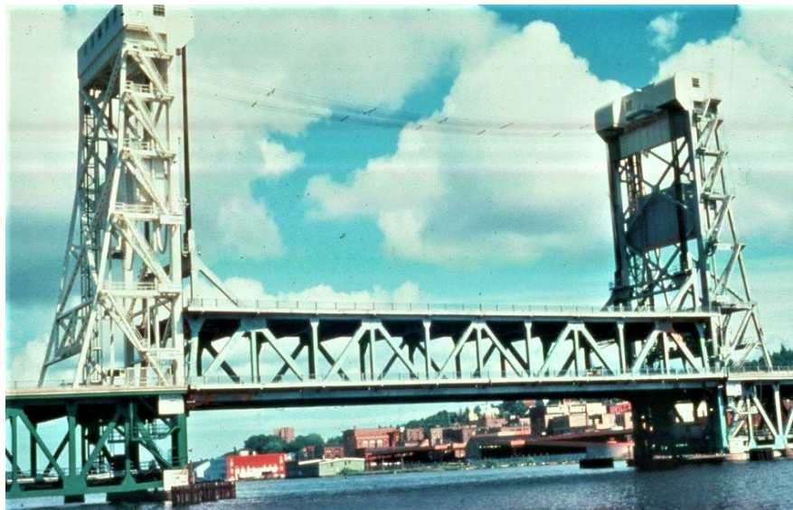
Figure 5.3.16 Tower-Drive Vertical Lift Bridge
