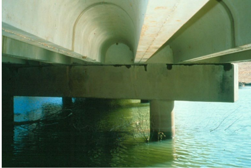
Figure 9.1.14 U-shaped Channel Beam Bridge
