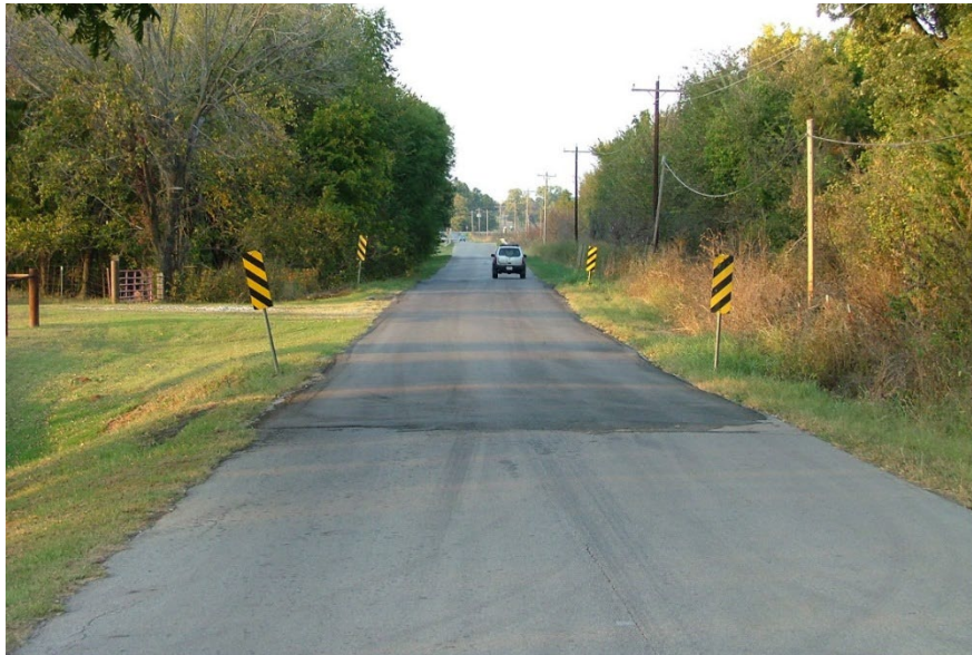
Figure 15.5.9 Repaired Roadway Over a Culvert
