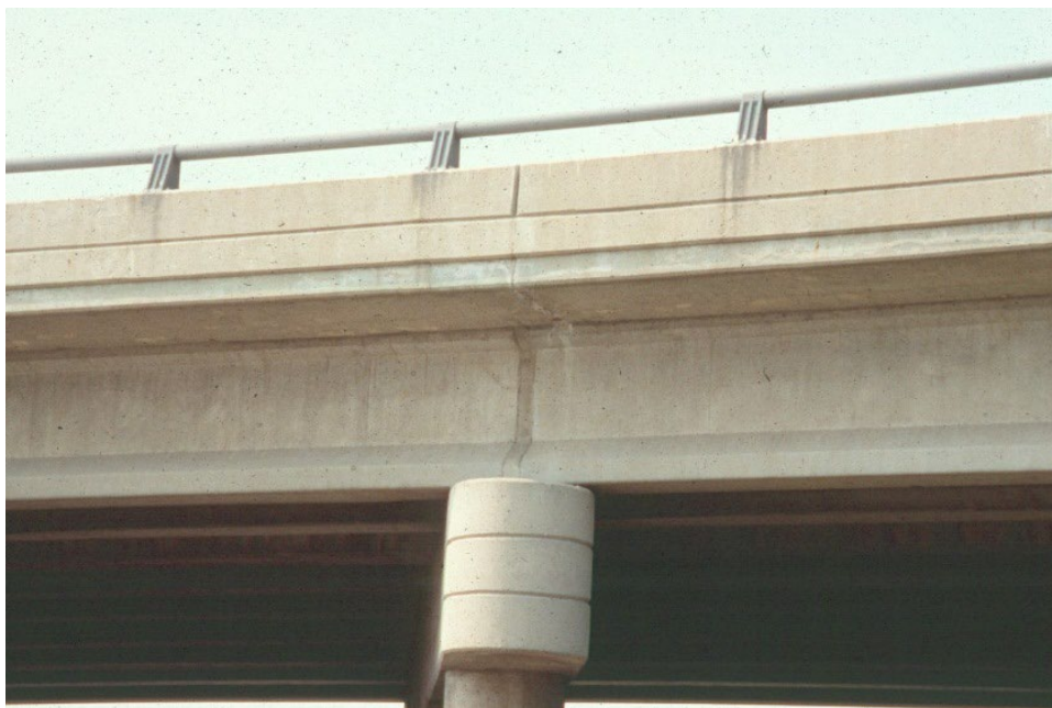
Figure 9.1.51 Continuous Prestressed I-beam Bridge
