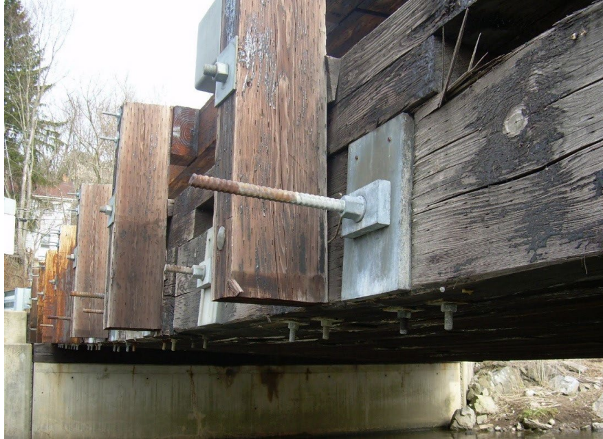
Figure 8.3.4 Stressed-laminated Deck
