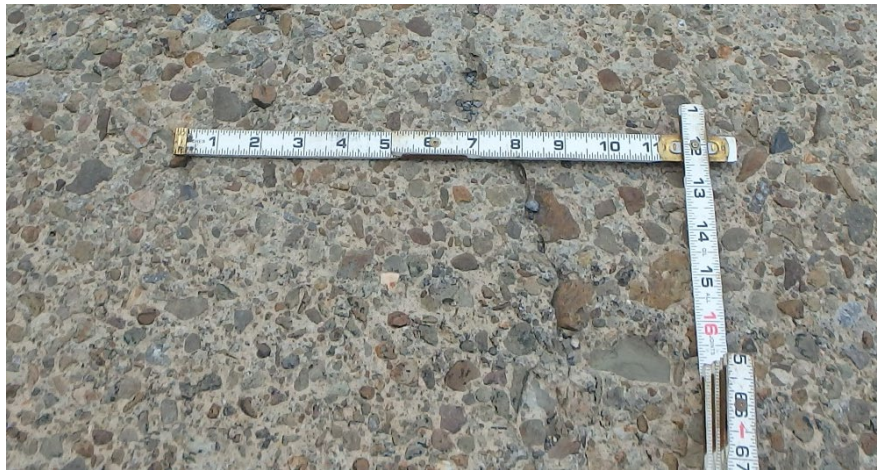
Figure 7.1.20 Medium or Moderate Scaling
