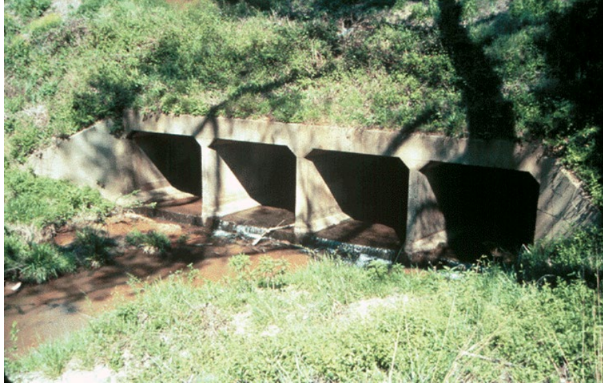
Figure 4.2.7 Multiple Cell Concrete Culvert
