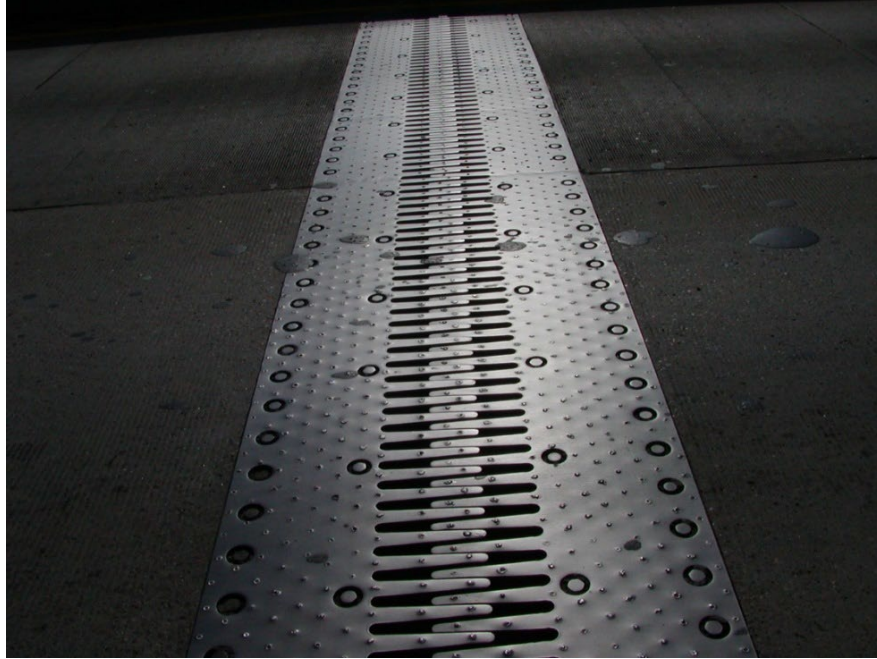
Figure 4.1.41 Top View of a Finger Plate Joint
