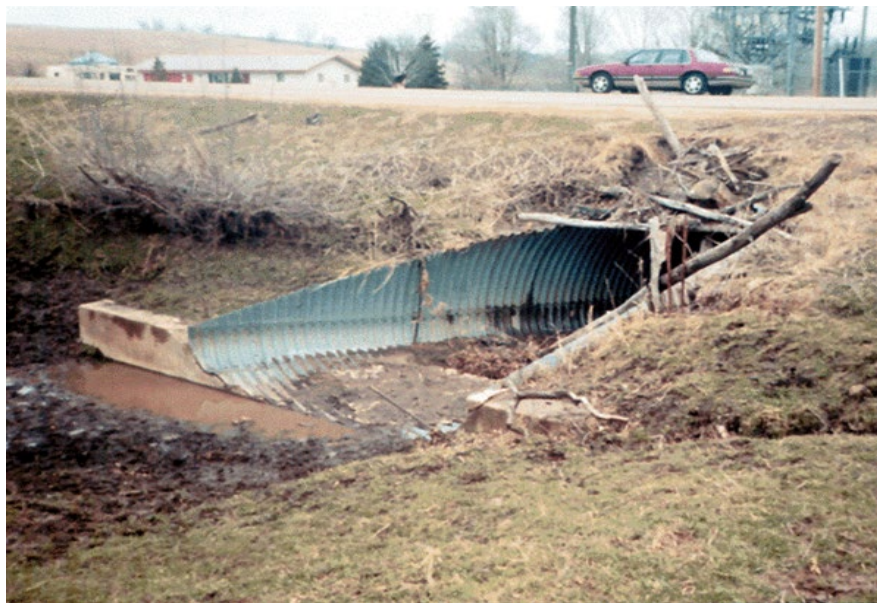
Figure 4.2.15 Culvert Mitered End
