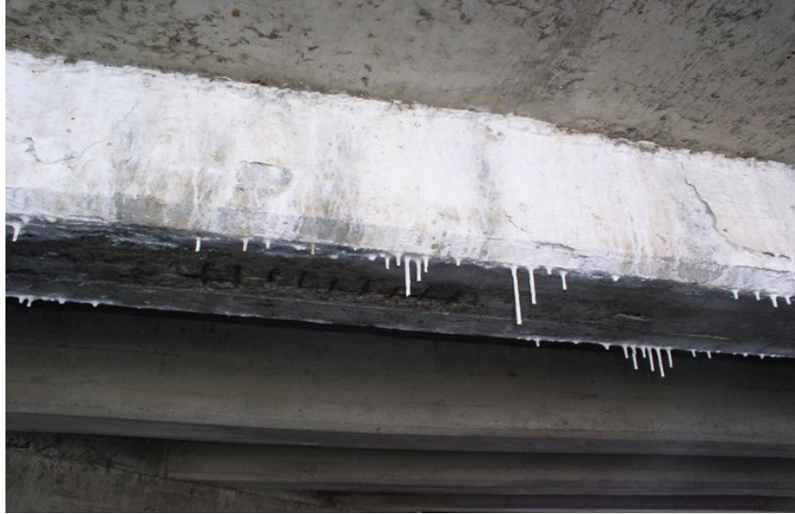
Figure 7.1.25 Efflorescence
