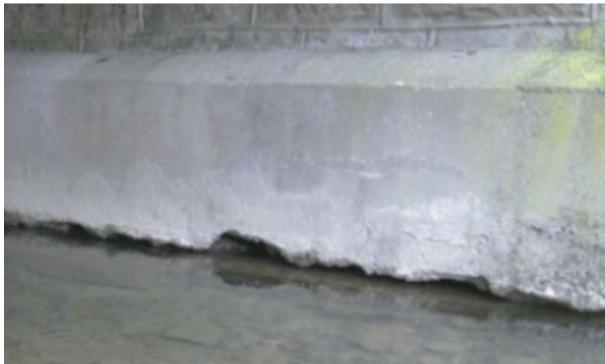
Figure 4.3.15 Concrete Footing Apron on a Masonry Abutment
