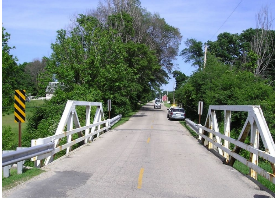
Figure 10.1.28 Pony Truss
