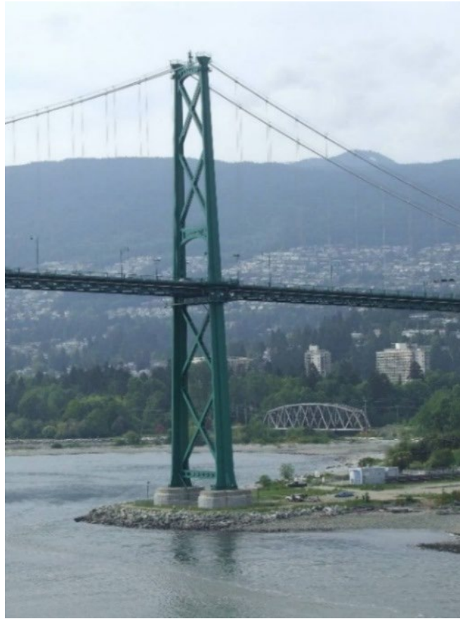
Figure 4.1.56 Suspension Bridge and Tower
