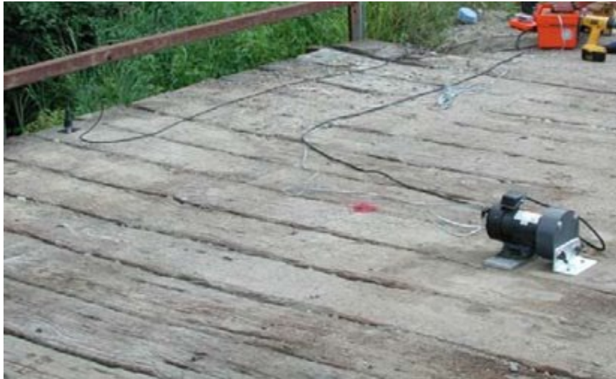
Figure 17.4.3 Vibration Testing on Timber Deck
