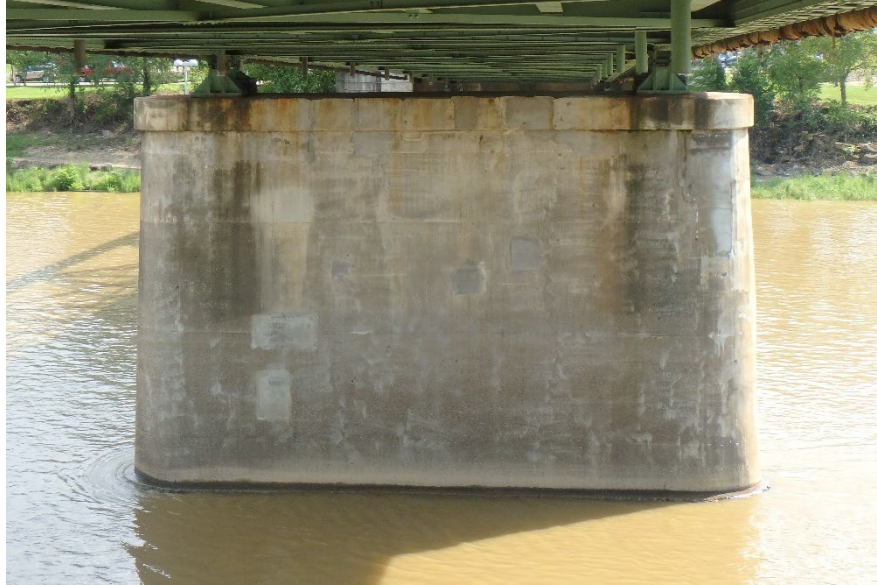
Figure 14.2.41 Solid Shaft or Wall Pier
