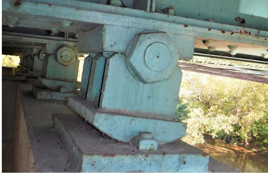
Figure 13.3.7 Rocker Bearing
