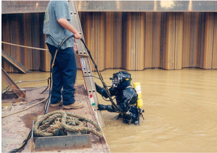
Figure 16.2.30 Access Barge and Exit Ladder
