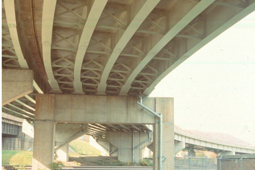
Figure 10.1.8 Curved Plate Girder Bridge
