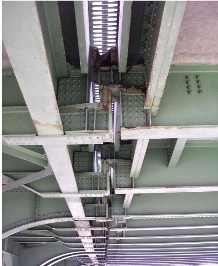
Figure 8.5.30 Support System under a Finger Plate Joint
