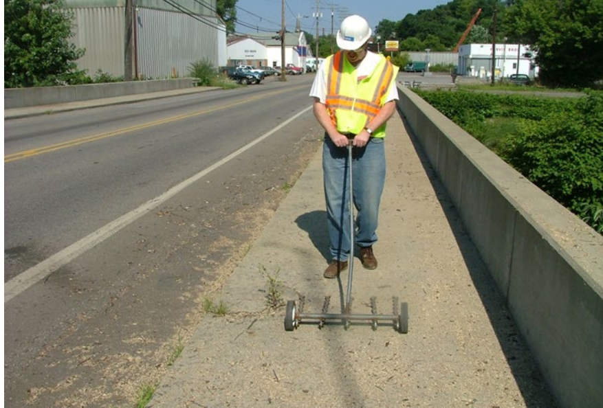
Figure 7.1.37 Inspector Using a Chain Drag looking for Delaminated Areas
