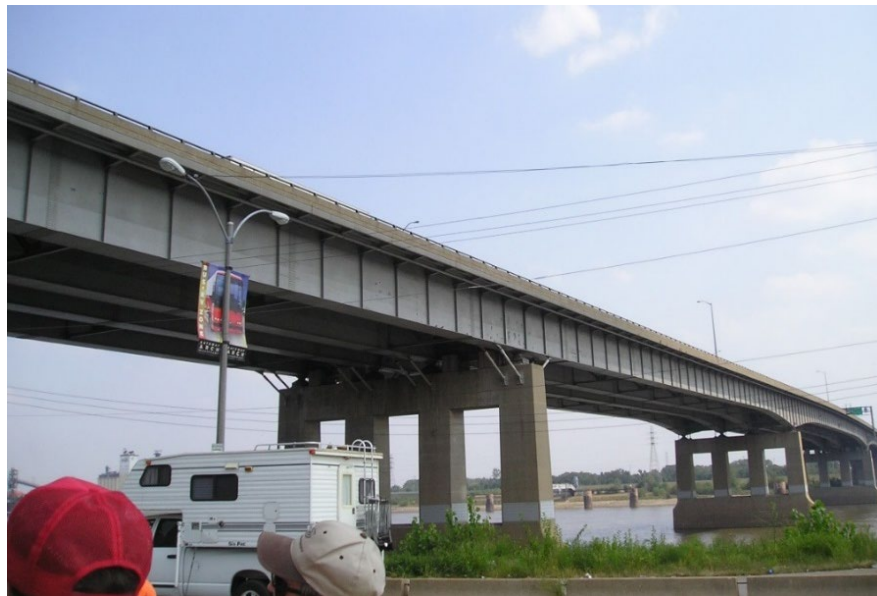
Figure 10.1.7 Continuous Span Plate Girder Bridge
