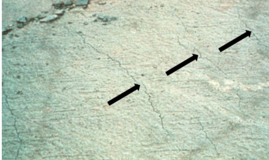
Figure 7.1.14 Temperature Cracks
