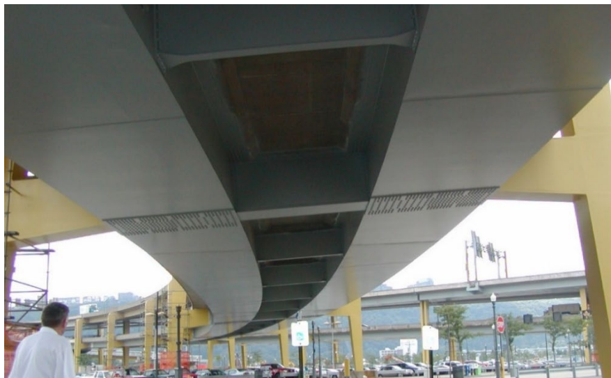
Figure 10.1.17 Spread Box Girders
