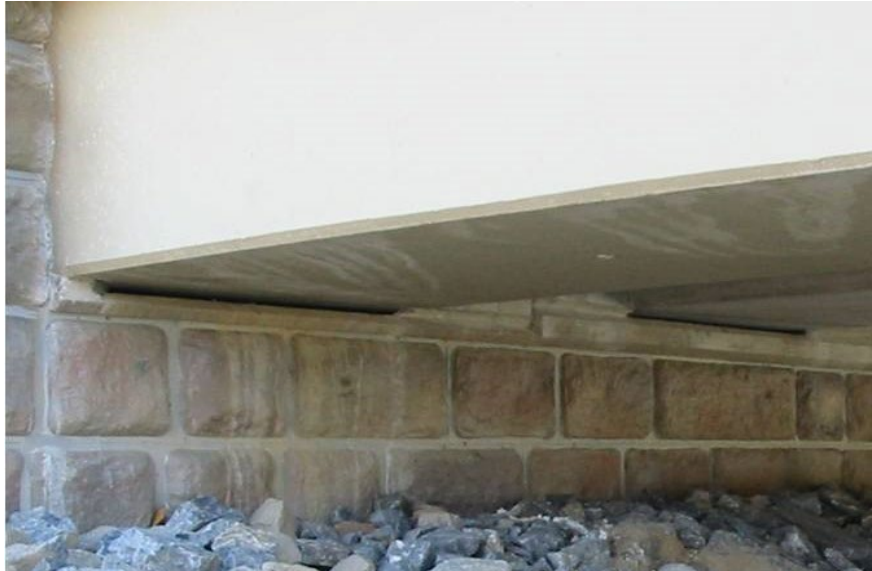
Figure 13.3.22 Enclosed or Concealed Bearing
