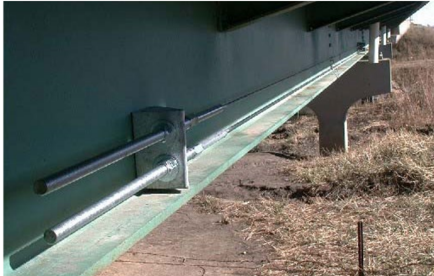
Figure 7.6.3 CFRP Post-tensioned Steel Girder
