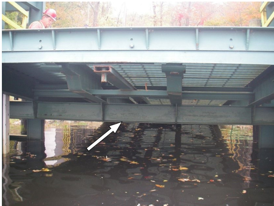
Figure 5.5.5 Lifting Girder
