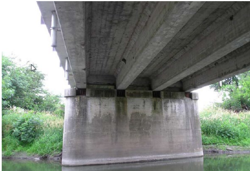
Figure 4.1.46 Concrete Tee Beam Bridge
