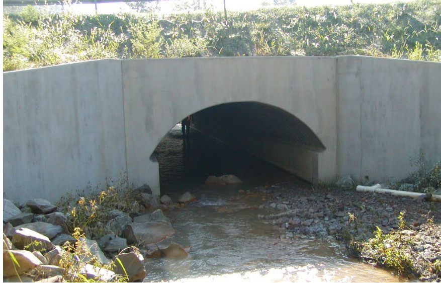
Figure 15.2.1 Rigid Culvert
