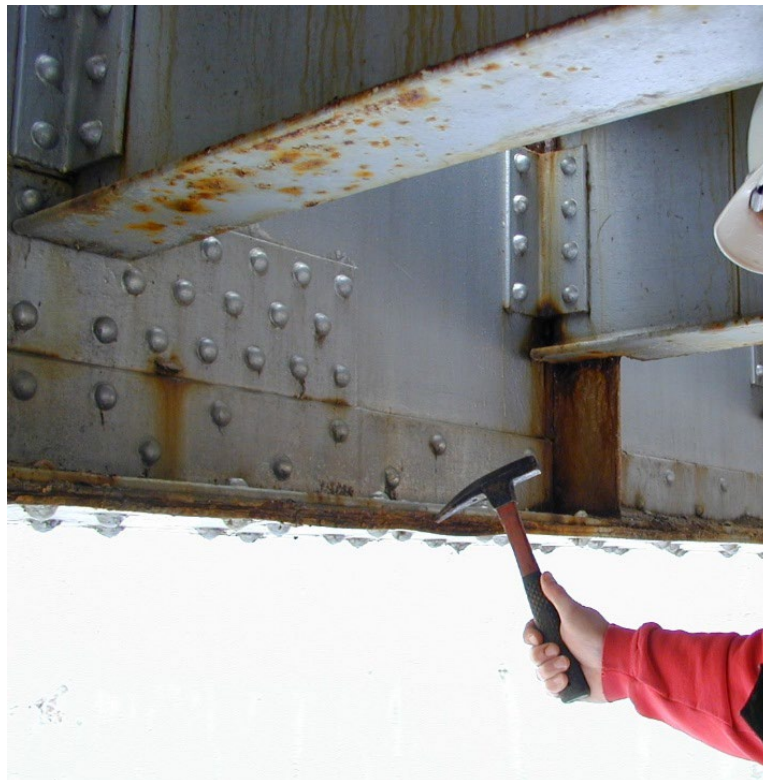
Figure 7.2.19 Inspector using a Hammer to Remove Loose or Scaling Rust
