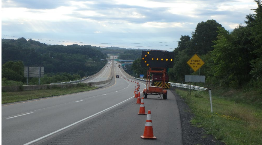
Figure 2.1.3 Temporary Traffic Control Operation
