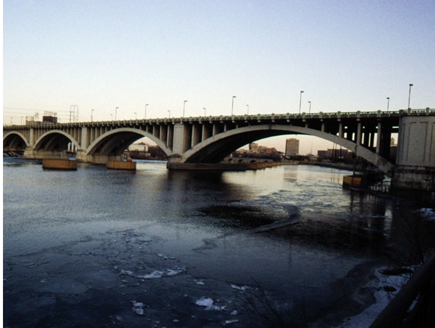
Figure 4.1.53 Deck Arch Bridge
