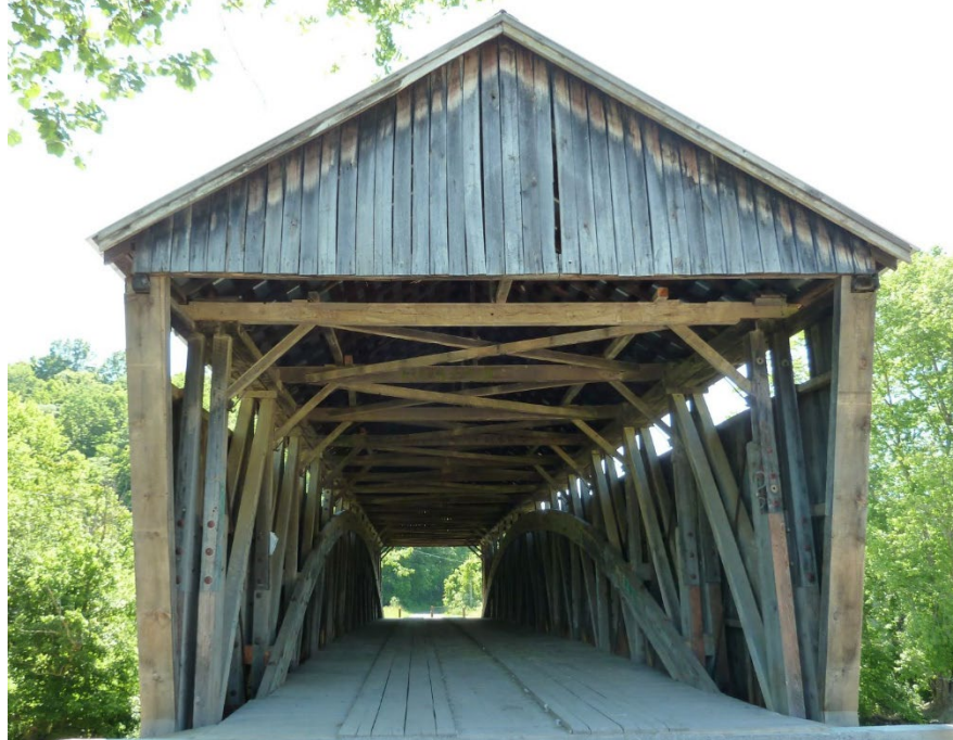
Figure 11.2.5 Truss Covered Bridge
