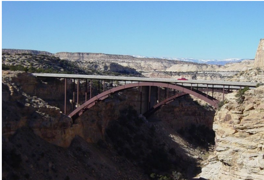
Figure 10.1.54 Solid Rib Deck Arch Bridge
