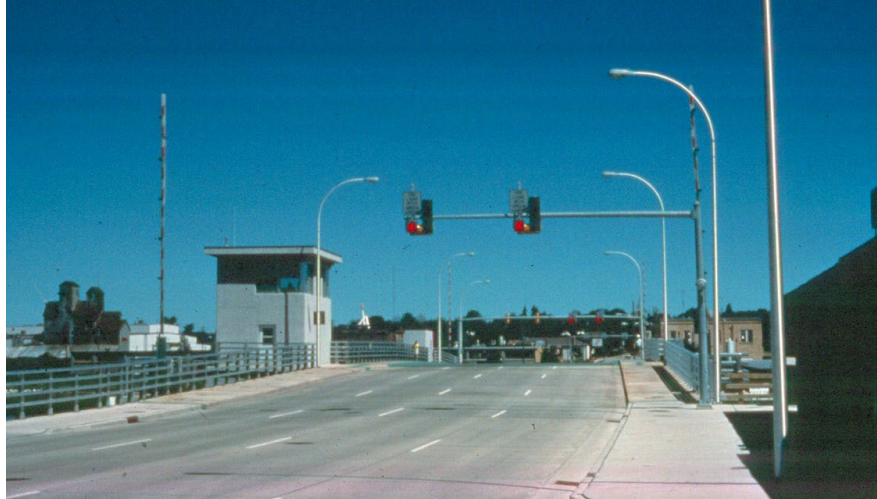
Figure 12.3.1 Operator's House with Clear View of Traffic Signals and Lane Gates
