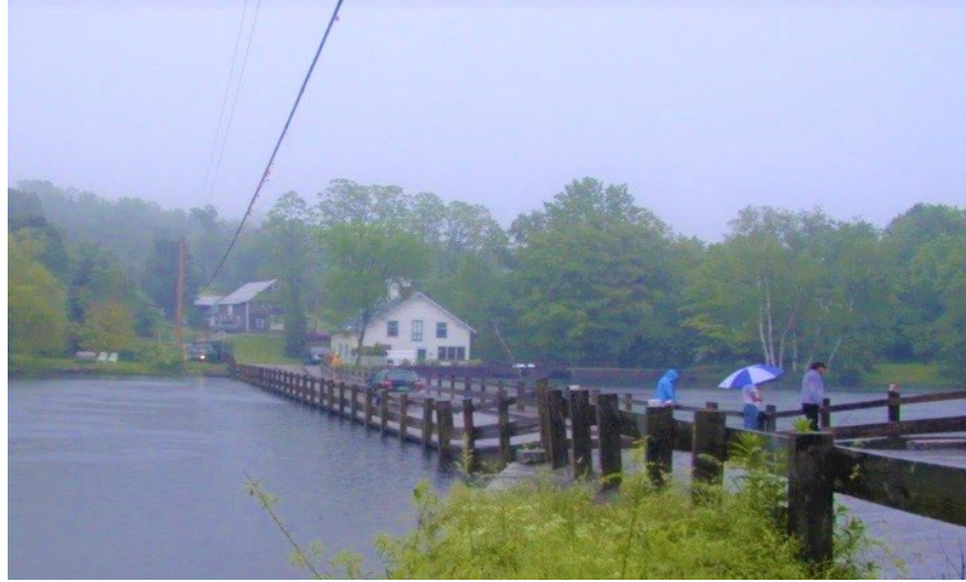
Figure 5.4.4 Floating Timber Bridge
