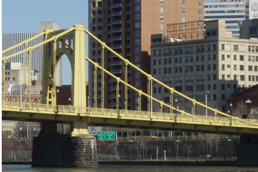
Figure 10.1.99 Eyebar Chain Suspension Bridge
