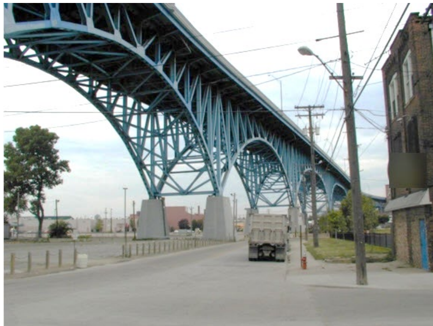
Figure 4.1.51 Deck Truss Bridge
