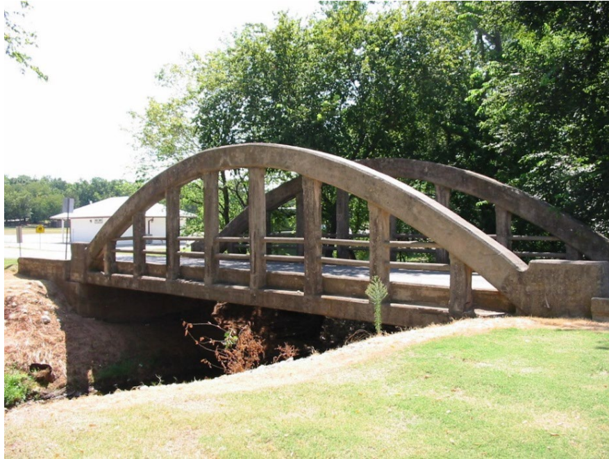
Figure 9.1.20 Concrete Through Arch Bridge
