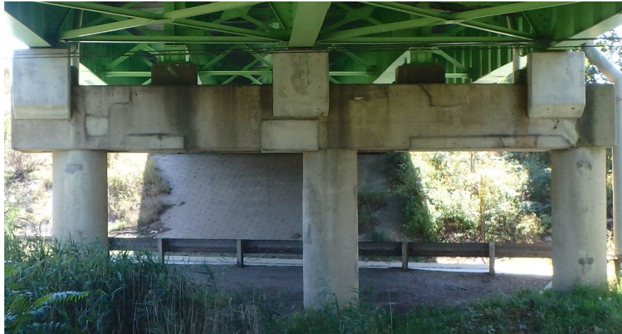
Figure 14.5.26 Repaired Concrete Pier Cap
