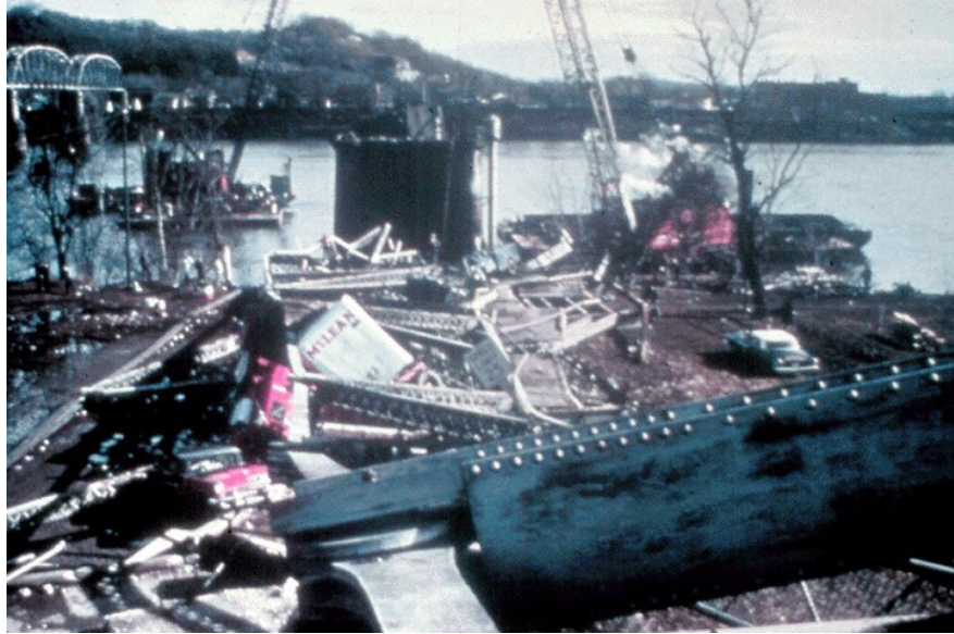
Figure 7.3.1 Silver Bridge Collapse
