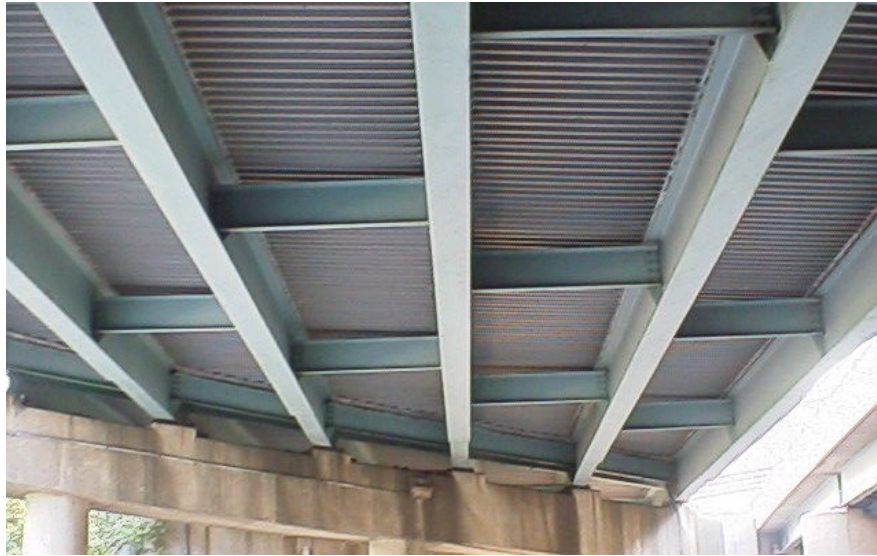
Figure 8.1.1 CIP Concrete Deck with Stay-in-Place Forms
