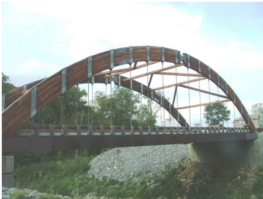
Figure 4.1.54 Through Arch Bridge
