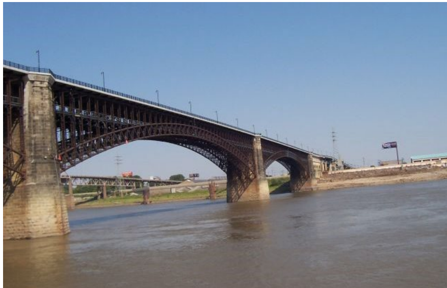
Figure 10.1.102 Eads Bridge using Steel Eyebars
