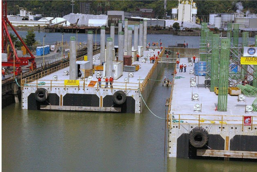
Figure 5.4.6 Concrete Pontoons being Transported to Site
