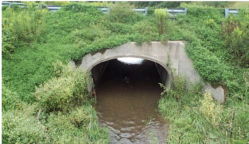
Figure 15.2.8 Concrete Arch Culvert
