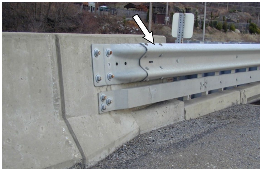
Figure 8.6.5 Proper Nesting of Guardrail at Transition
