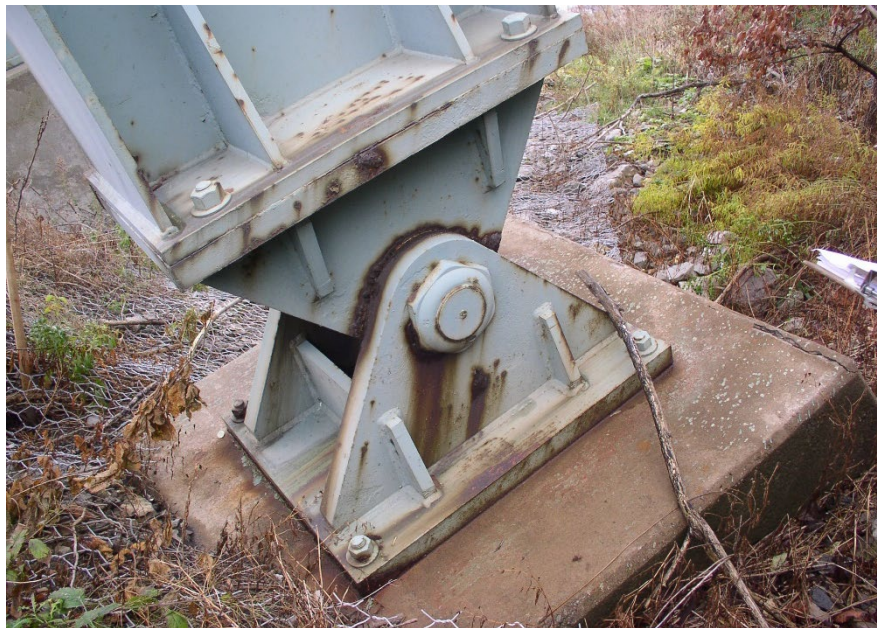
Figure 10.4.1 Bearing Area of a Rigid Frame Bridge
