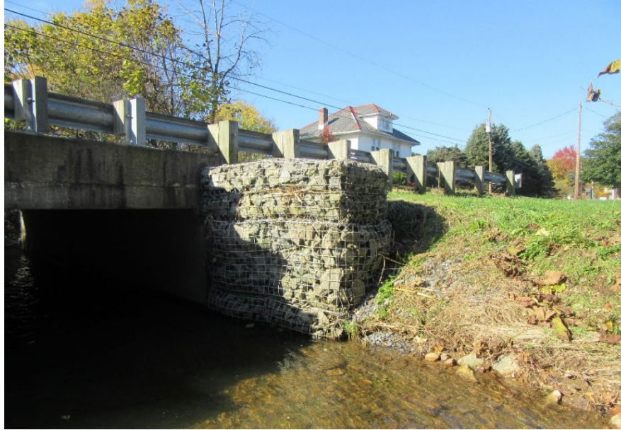
Figure 4.3.12 Gabion Basket Serving as Slope Protection
