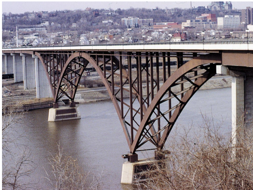
Figure 4.1.63 Deck Arch with Spandrel Columns
