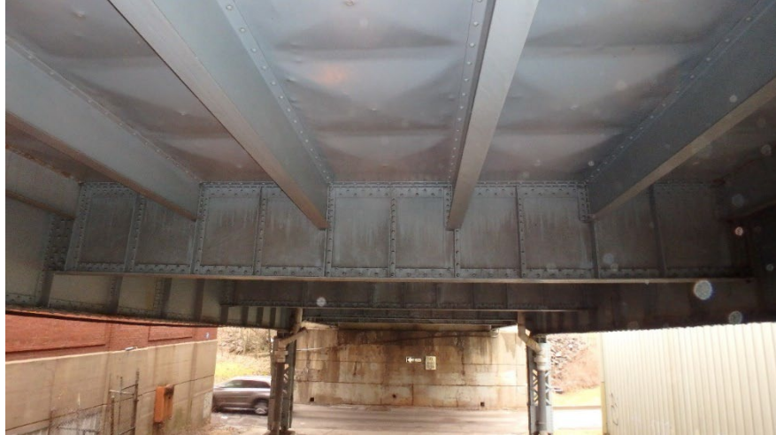
Figure 8.2.2 Underside View of Buckle Plate Deck
