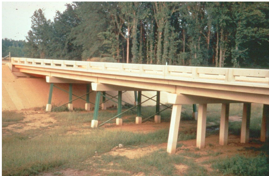
Figure 4.1.85 Steel and Concrete Pile Bents
