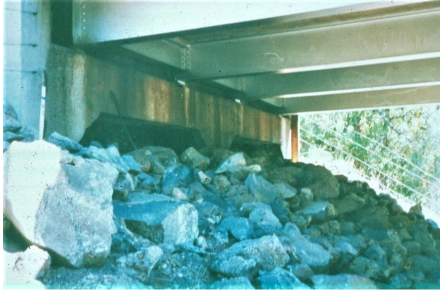
Figure 14.2.15 Spill Through/Open Abutment
