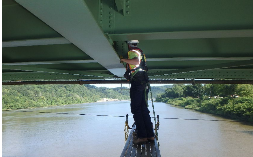
Figure 2.5.4 Rigging for Superstructure Inspection
