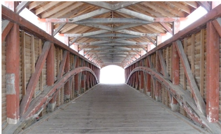
Figure 11.2.9 Inside View of Covered Bridge with Burr Arch-Truss Configuration
