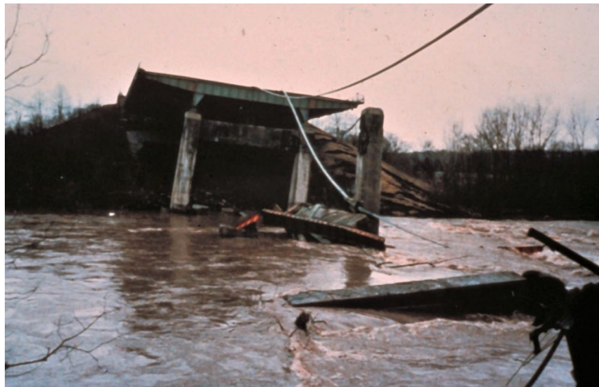
Figure 16.2.1 Schoharie Creek Bridge Failure
