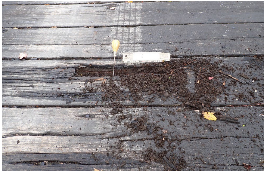
Figure 7.4.27 Results of a Pick Test
