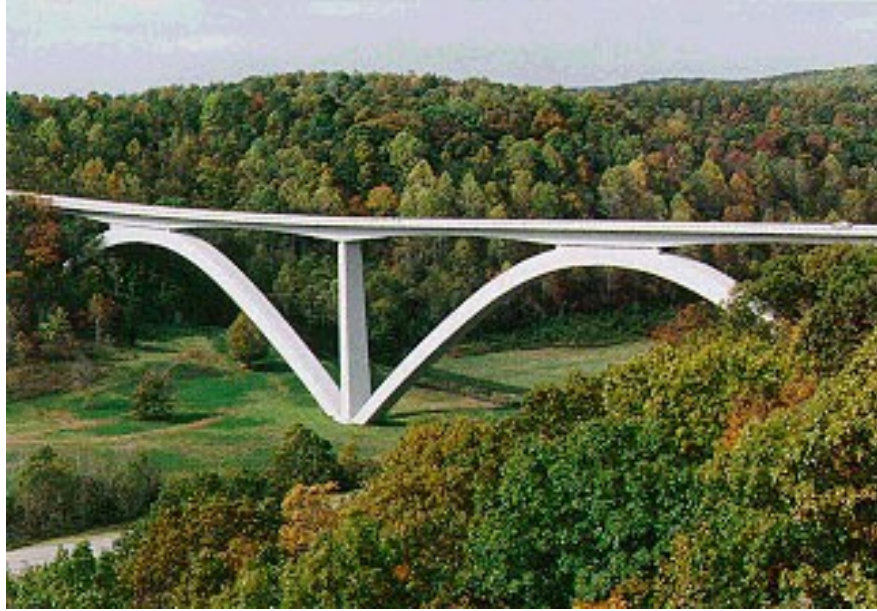
Figure 9.1.21 Precast Post-tensioned Concrete Arch without Spandrel Columns
