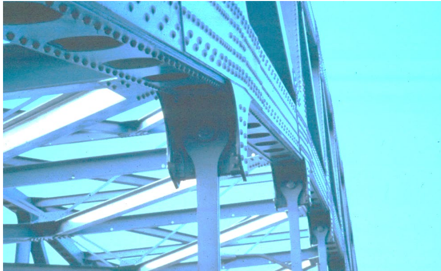
Figure 10.4.15 Hanger Connection on a Through Arch
