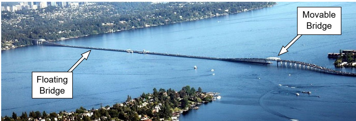
Figure 5.4.3 Floating Bridge and Movable Bridge Elevation
