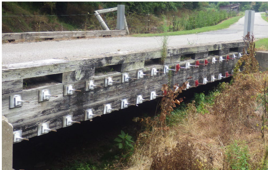
Figure 11.2.26 Stress-Laminated Timber Box Beam Bridge
