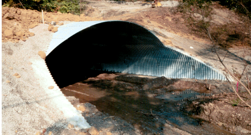
Figure 15.2.14 Pipe Arch Flexible Culvert
