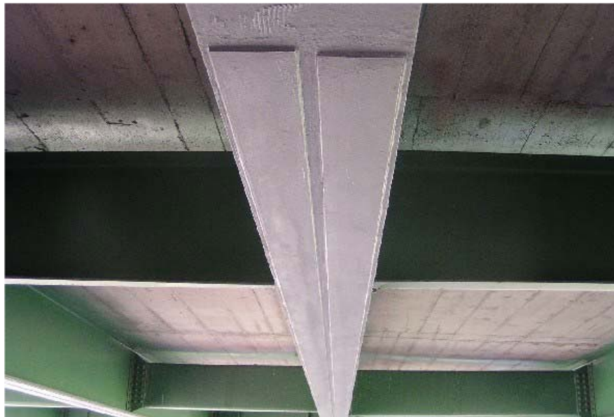
Figure 7.6.4 Externally Bonded CFRP Plates to Steel Girder Bottom Flange
