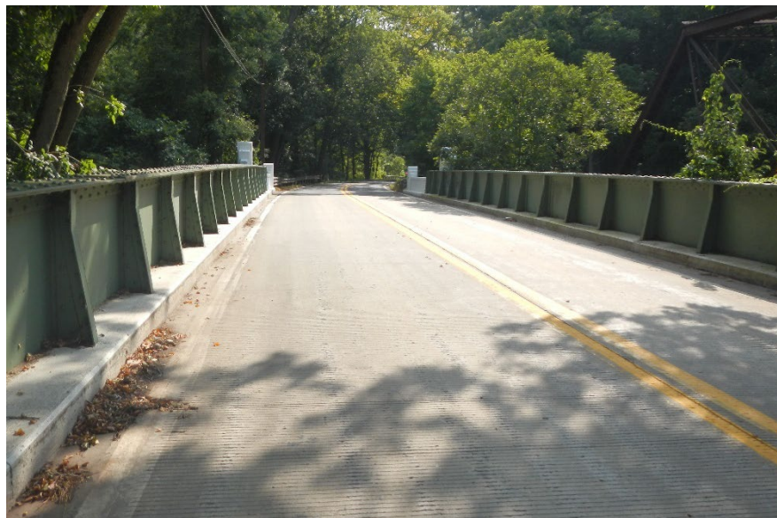
Figure 10.1.22 Through Girder Bridge
