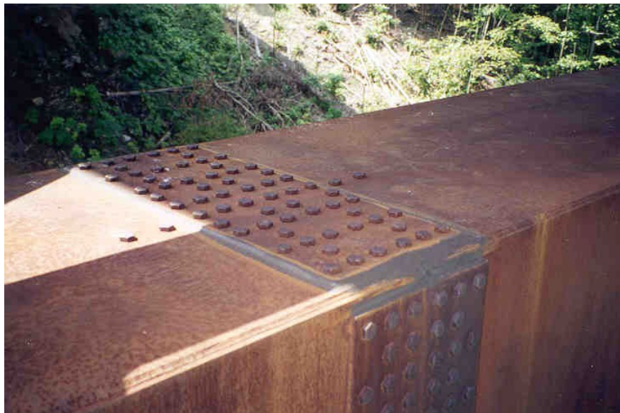
Figure 7.2.7 Light Brown - Early Development of the Oxide Film (Patina)
