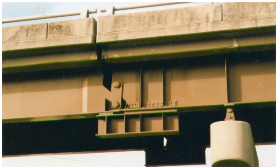
Figure 10.1.82 Underslung Catcher Retrofit
