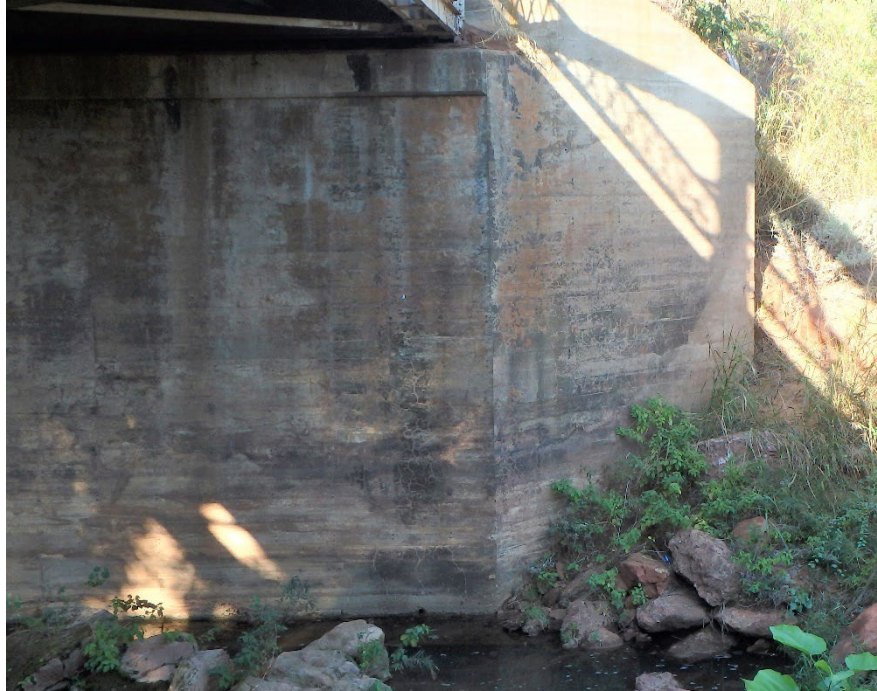
Figure 14.2.32 Integral Wingwall
