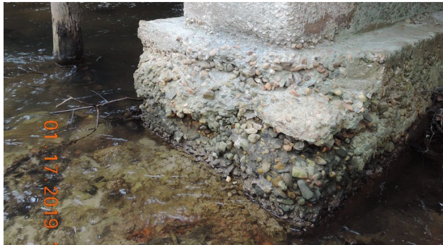
Figure 7.1.22 Severe Scaling
