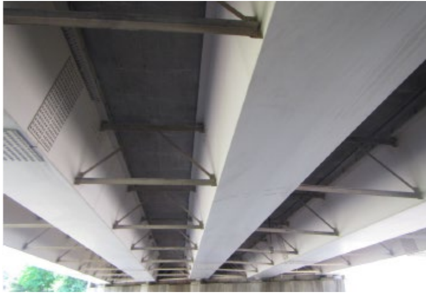
Figure 10.1.14 Simple Span Box Girder Bridge
