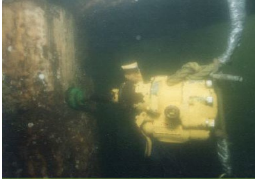
Figure 16.2.36 Concrete Coring Taking Place
