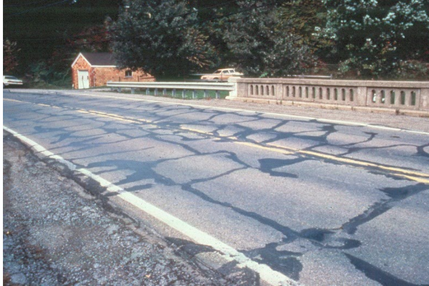
Figure 9.4.30 Asphalt Covered Tee Beam Flange
