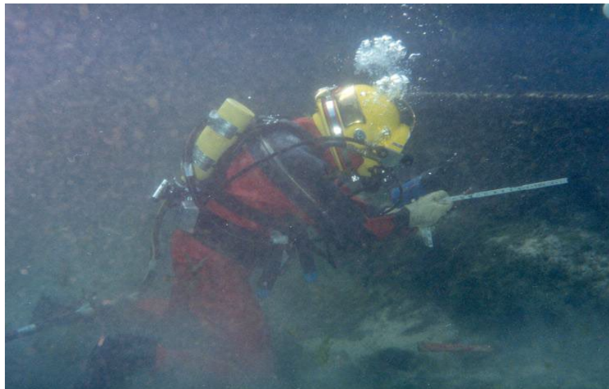
Figure 16.2.22 Surface-Supplied Diving Inspection
