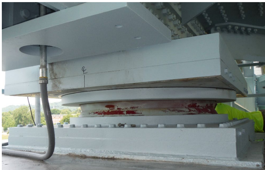
Figure 13.3.21 Disk Bearing
