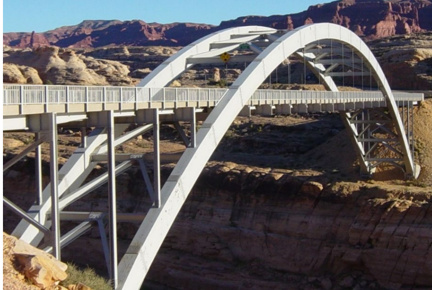
Figure 10.1.59 Modified Through Arch Bridge
