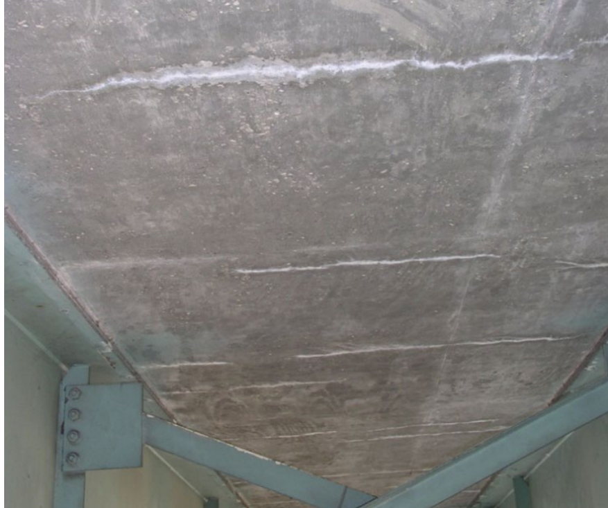
Figure 7.1.16 Transverse Cracks
