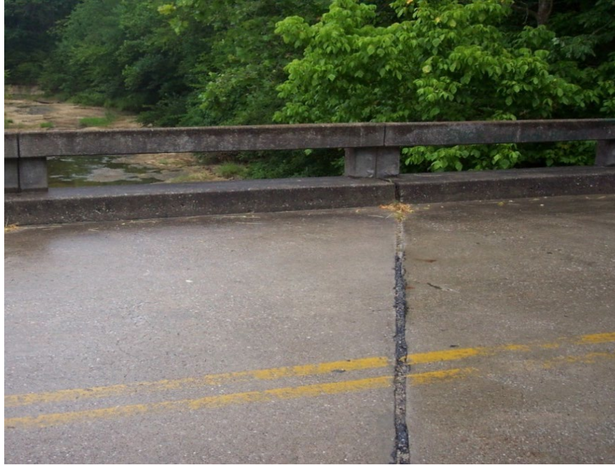
Figure 8.5.3 Pourable Joint Seal
