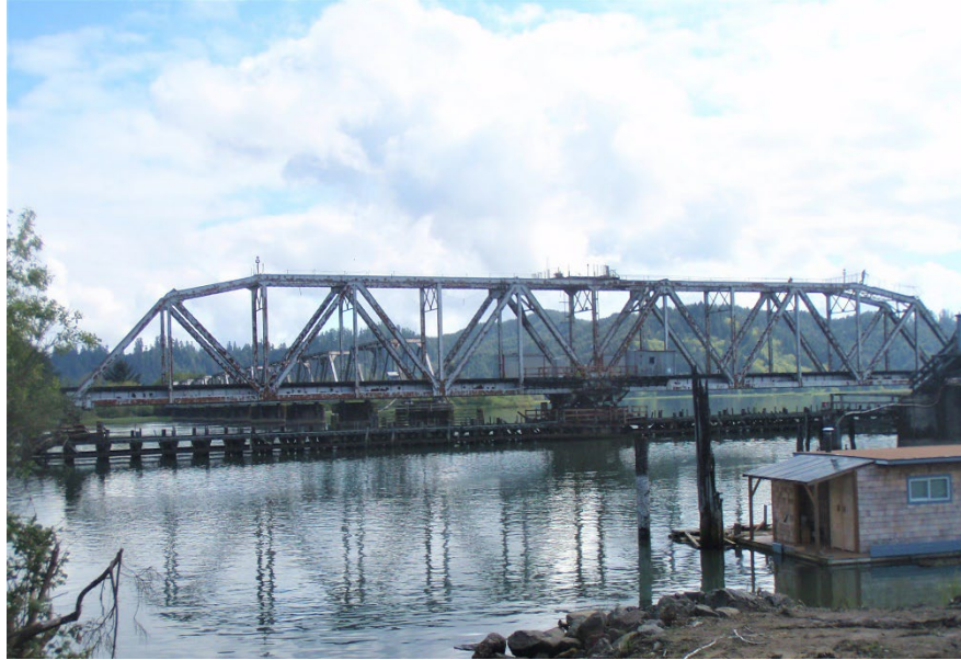
Figure 5.3.4 Rim-Bearing Swing Span in Open Position
