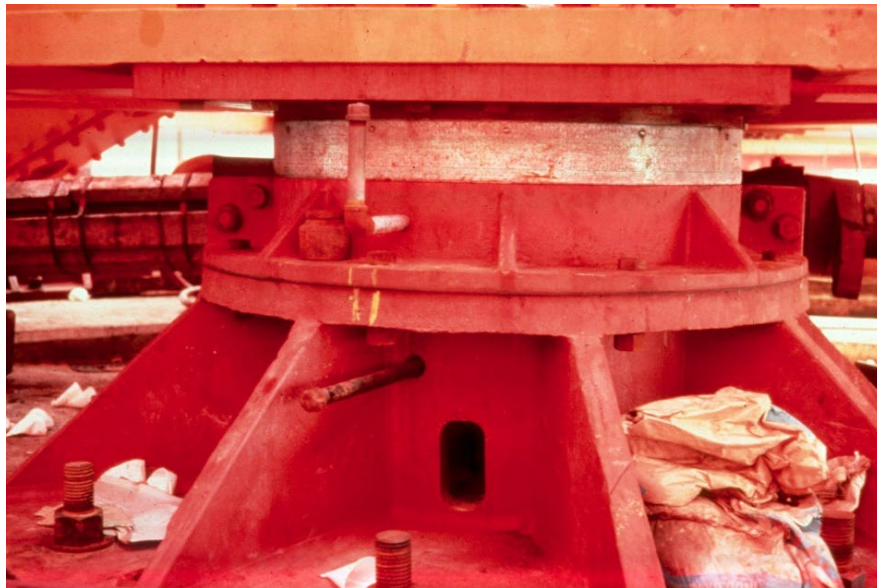
Figure 5.3.29 Center Pivot Bearing
