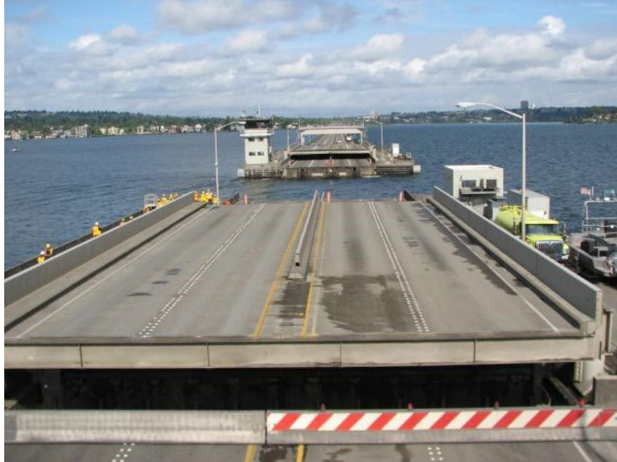
Figure 5.4.2 Movable Bridge Section
