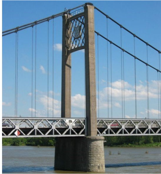
Figure 5.2.21 Concrete Portal Tower
