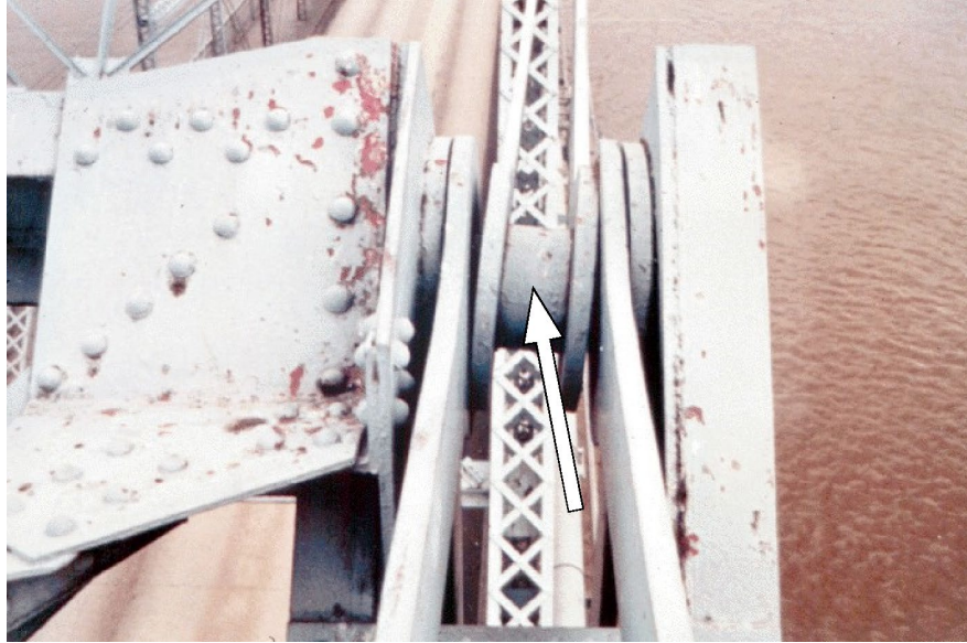
Figure 10.4.49 Spacer with Unsymmetrical Eyebars
