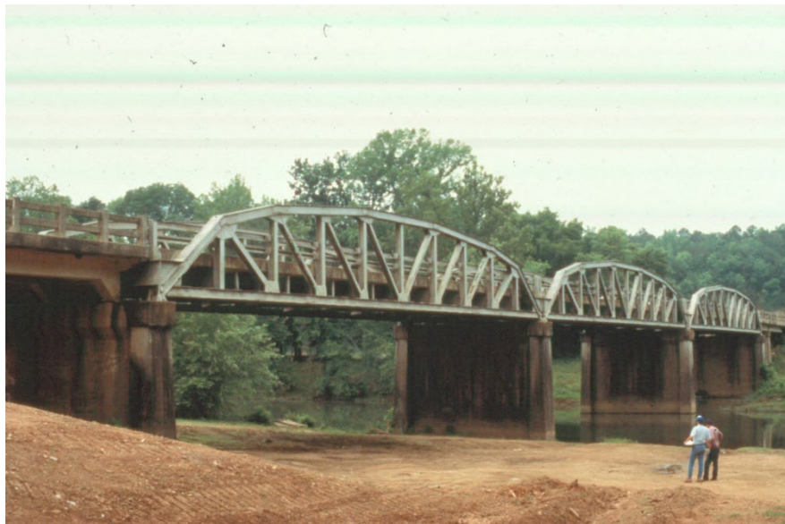
Figure 10.1.35 Multiple Simple Span Pony Truss
