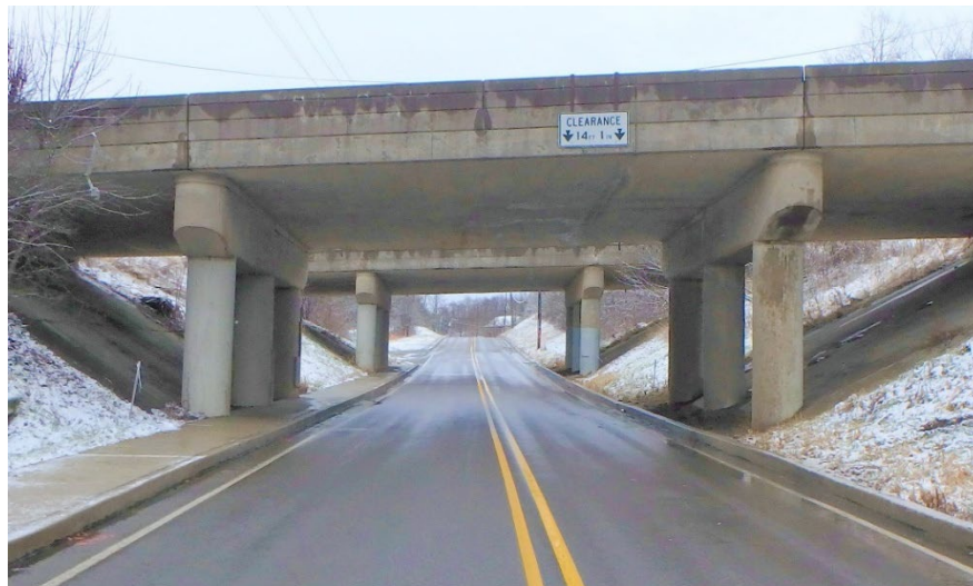
Figure 9.1.1 Typical Simple Span Cast-in-Place Slab Bridge
