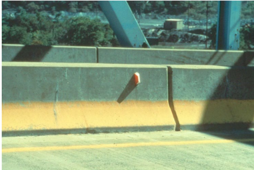
Figure 4.1.28 New Jersey Barrier
