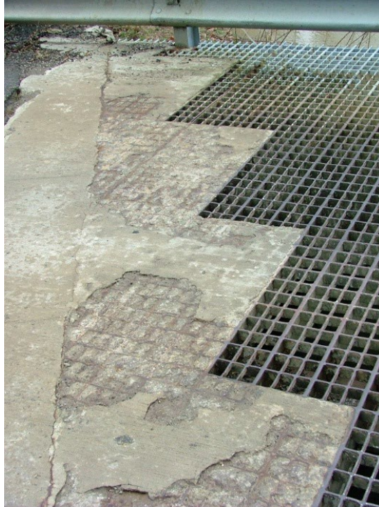
Figure 8.2.8 Filled and Un-filled Steel Grid Deck
