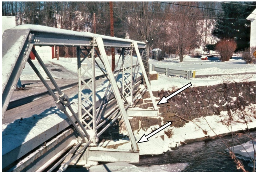
Figure 10.1.120 Pony Truss Sway Bracing
