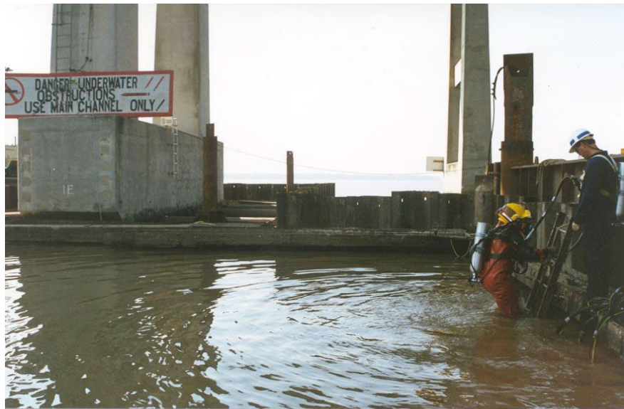
Figure 16.2.14 Diving Inside a Cofferdam
