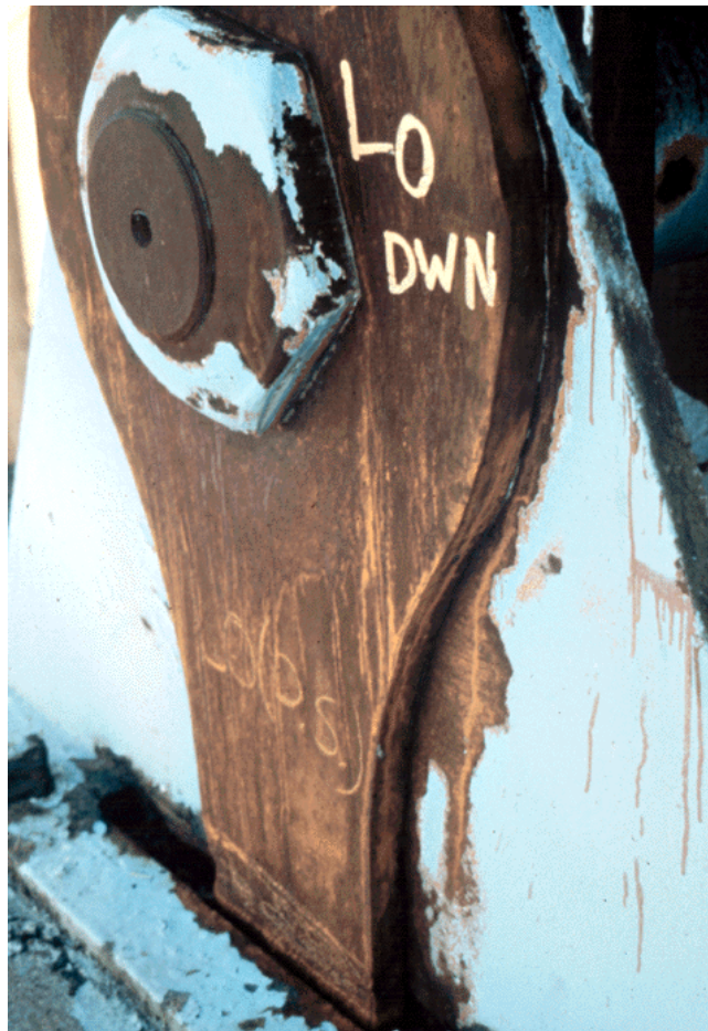
Figure 10.1.100 Anchorage Eyebar
