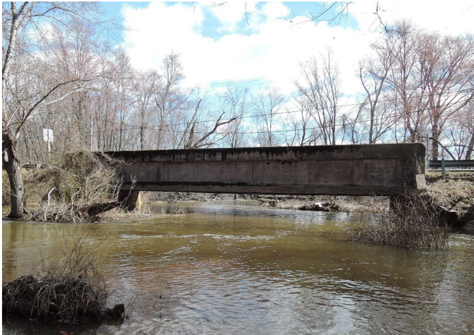
Figure 9.1.11 Concrete Through Girder Bridge
