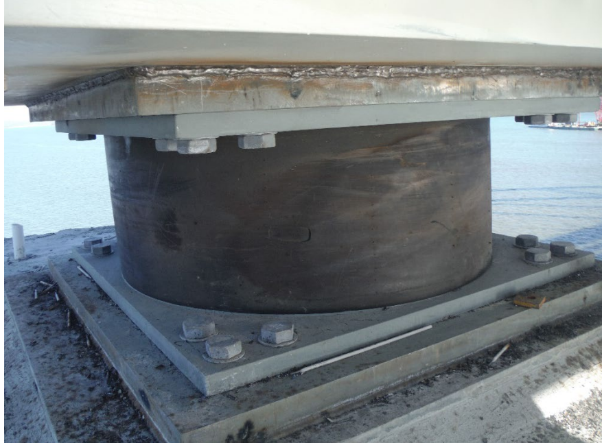
Figure 13.6.16 Lead Core Isolation Bearing
