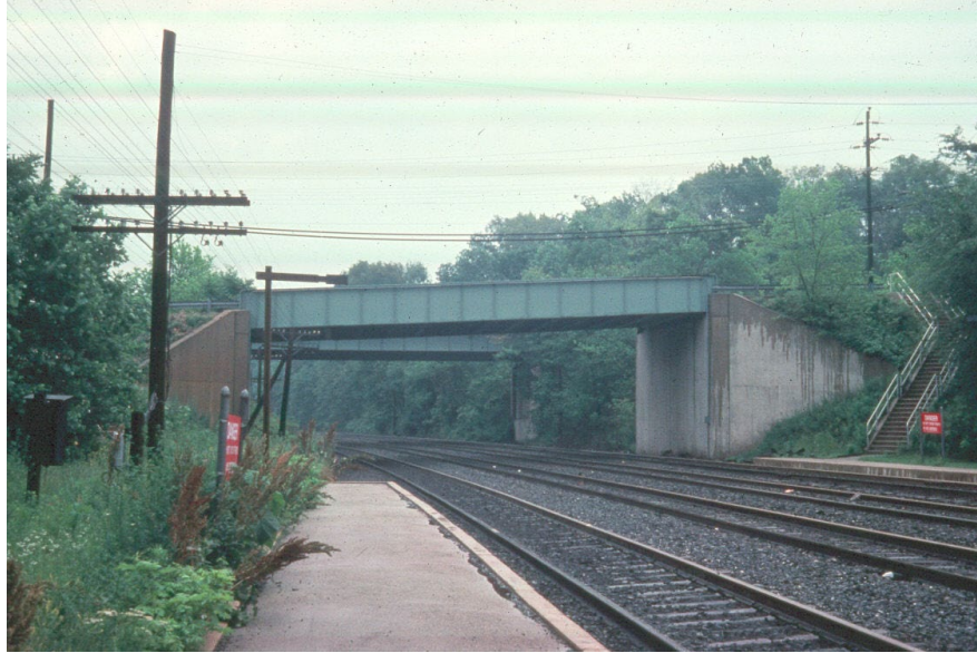
Figure 10.1.23 Through Girder Bridge with Limited Underclearance
