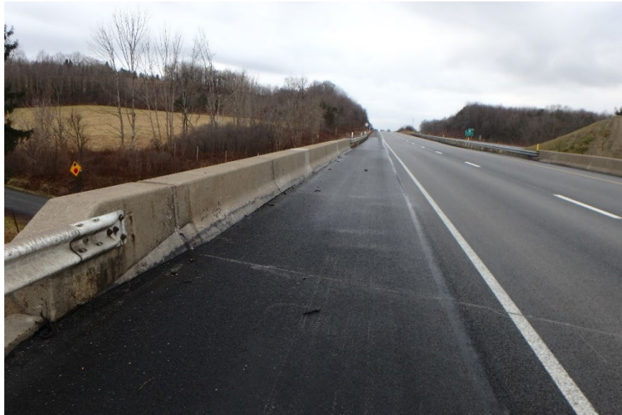
Figure 4.1.36 Asphalt Wearing Surface on a Concrete Deck
