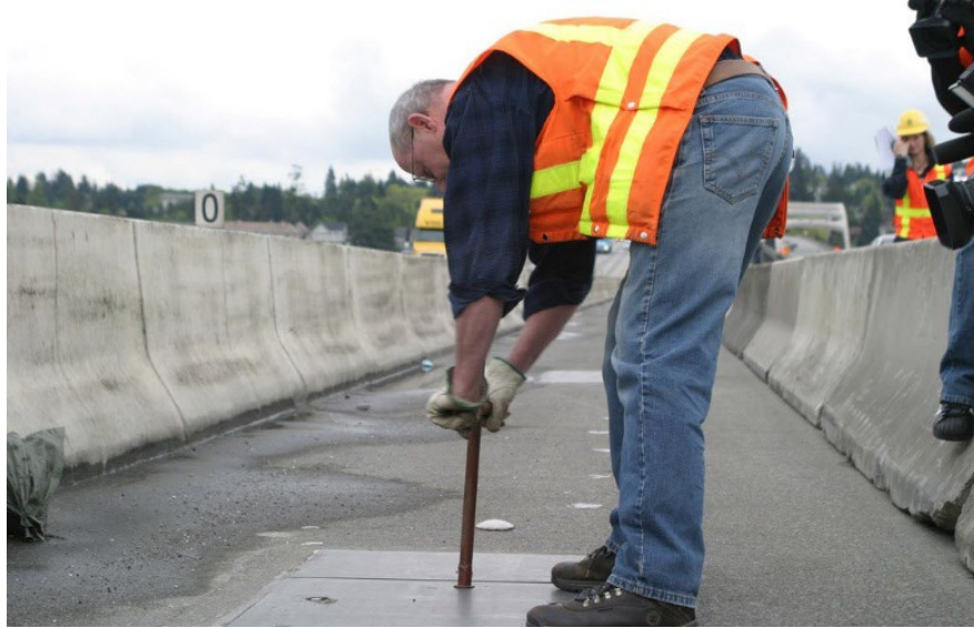
Figure 12.4.1 Inspector Opening Pontoon Access Hatch
