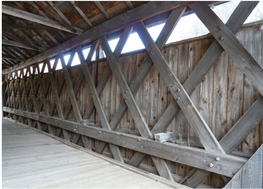
Figure 11.2.10 Town Truss Design
