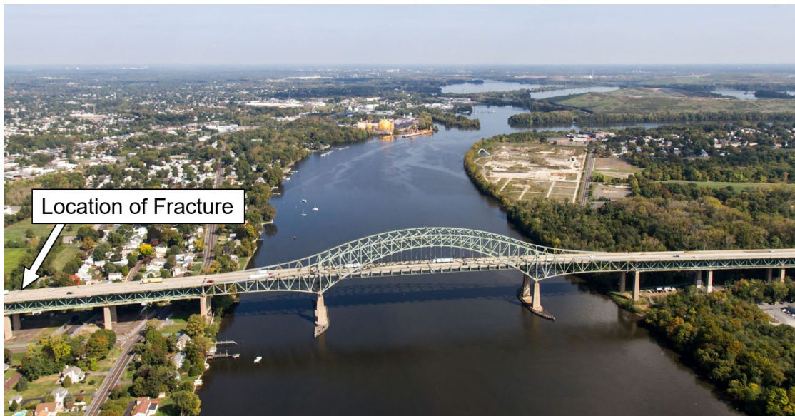
Figure 10.5.6 Delaware River-Turnpike Toll Bridge
