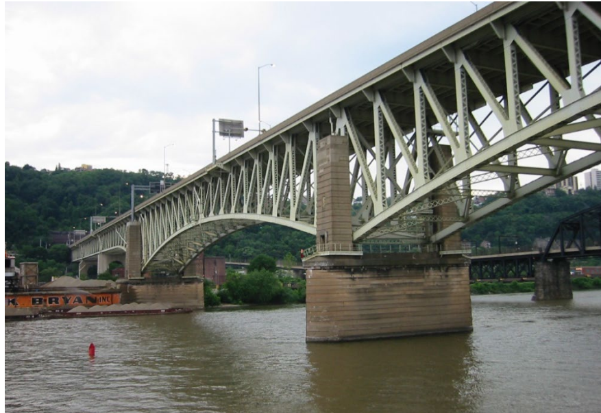
Figure 16.2.2 Liberty Bridge over Monongahela River
