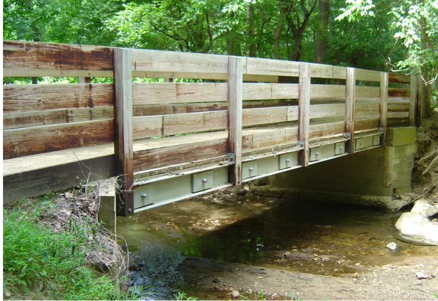
Figure 11.2.21 Stress-Laminated Timber Slab Bridge
