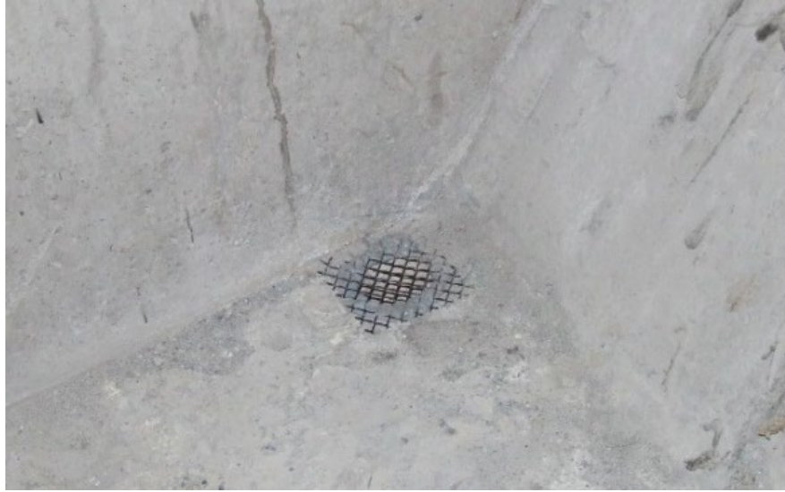
Figure 9.4.41 Concrete Box Girder Drain Hole with Screen
