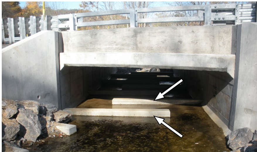
Figure 15.5.18 Energy Dissipater System
