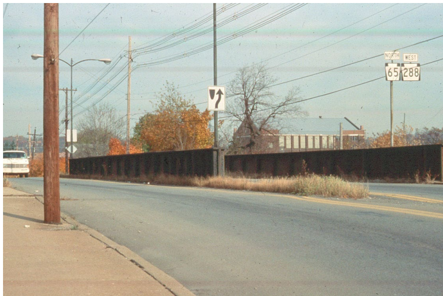
Figure 10.1.24 Through Girder Bridge with Three Girders
