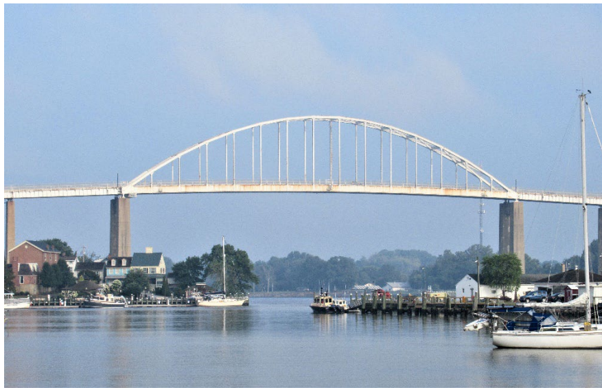
Figure 10.1.53 Through Arch Bridge
