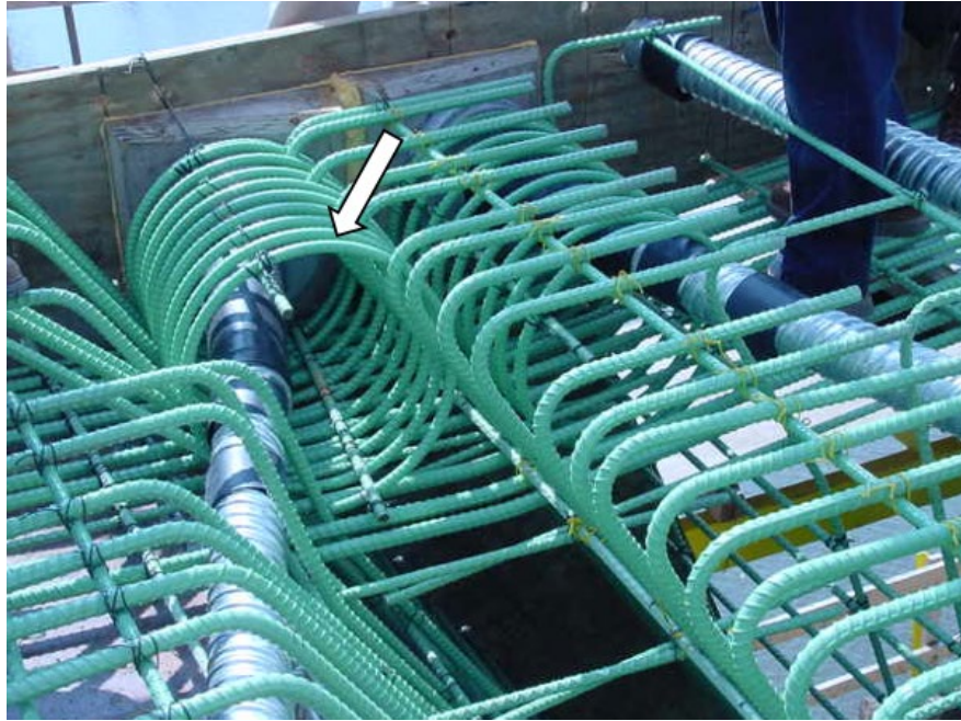
Figure 9.1.62 Post-tensioning Anchorage Reinforcement Before Concrete Placement
