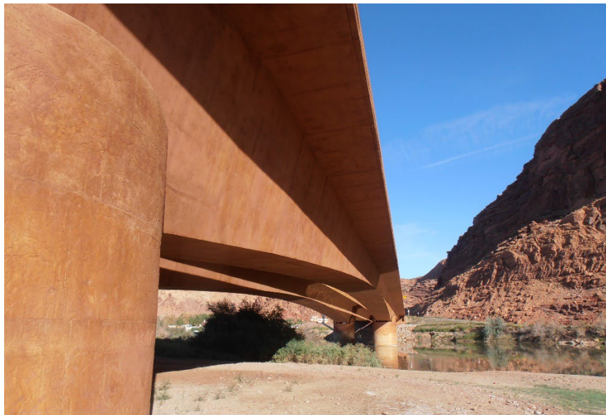
Figure 9.1.55 Cast-in-place Concrete Box Girder Bridge
