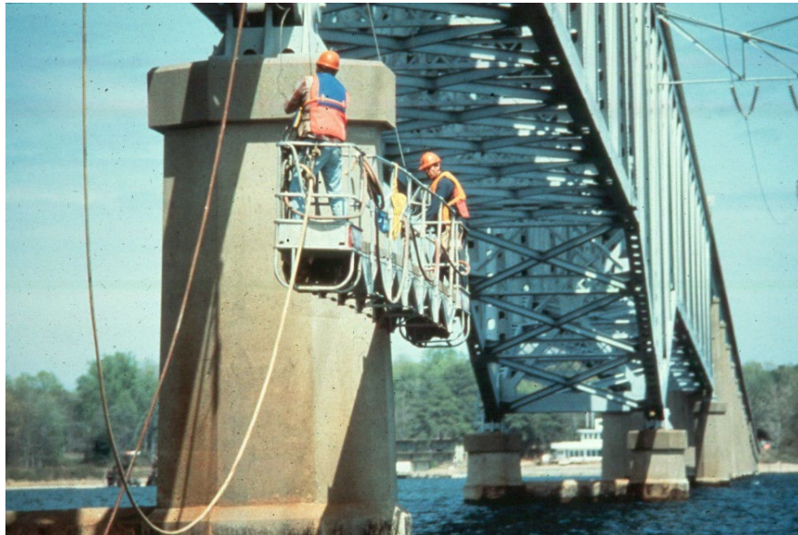
Figure 2.5.3 Rigging for Substructure Inspection
