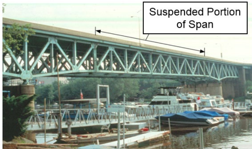
Figure 10.1.37 Cantilever Deck Truss
