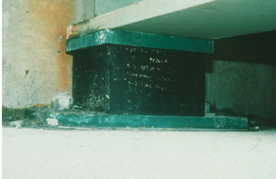
Figure 13.3.28 Lead Core Isolation Bearing
