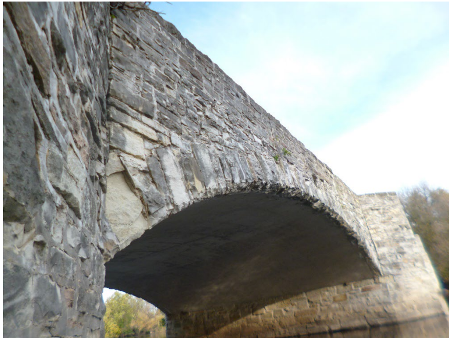
Figure 11.2.29 Masonry Closed Spandrel Arch Bridge
