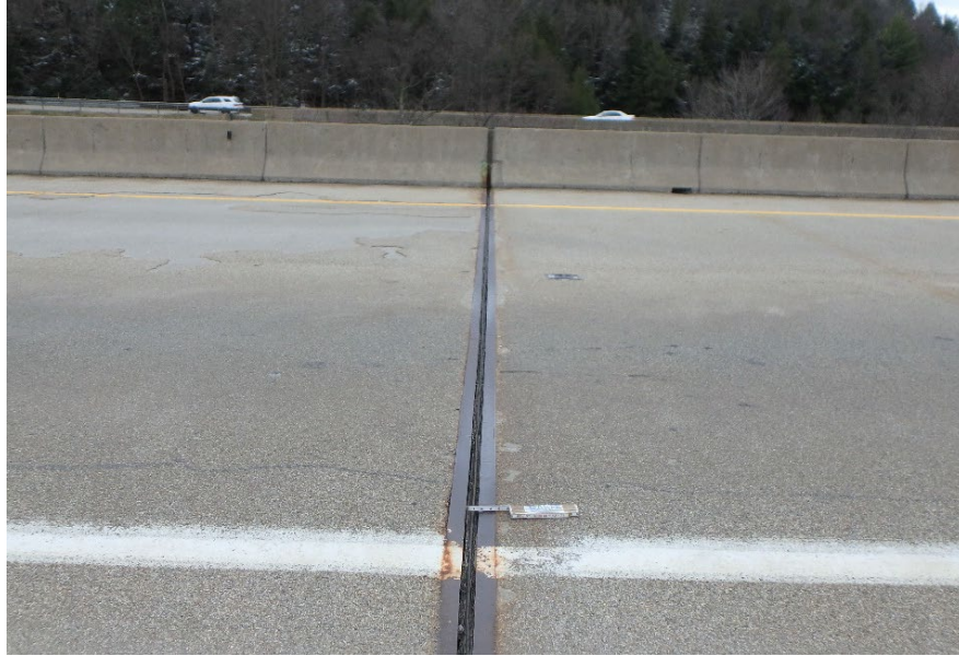
Figure 8.5.1 Strip Seal
