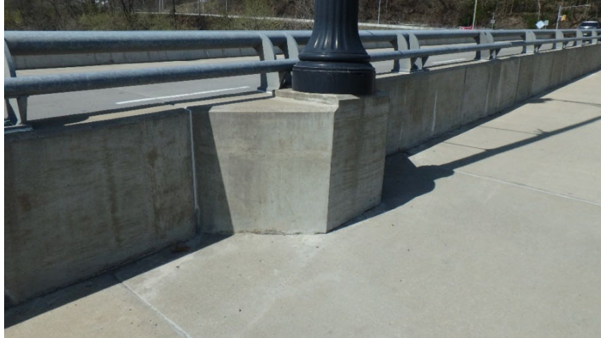
Figure 8.5.34 Light Pole Attached to a Bridge
