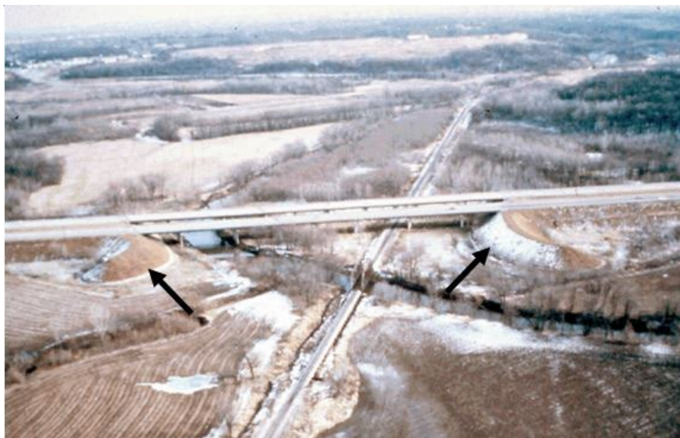
Figure 4.3.10 Guide Banks Constructed on Kickapoo Creek Near Peoria, Illinois
