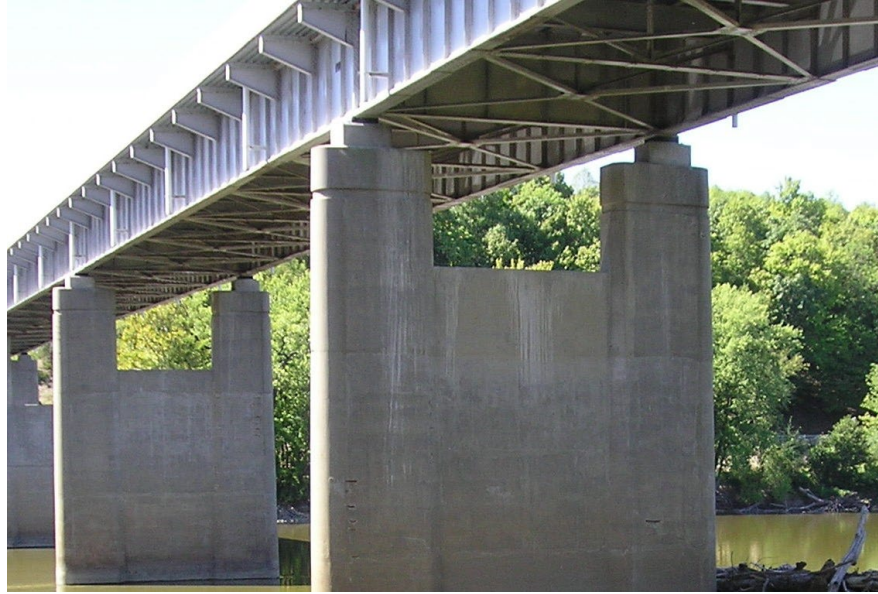
Figure 10.1.21 General View of a Deck Girder Bridge
