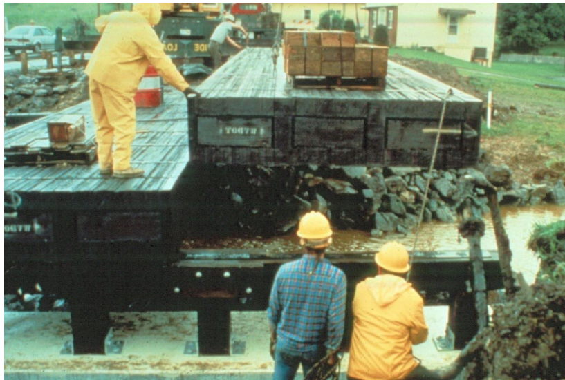
Figure 7.4.7 Coal Tar Creosote Treated Timber Beams
