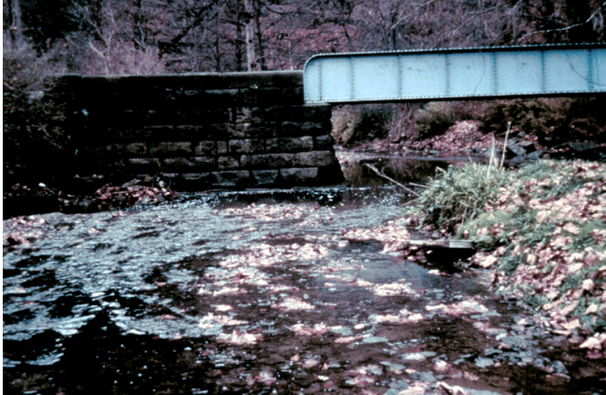
Figure 16.1.21 Stream Changes due to Lateral Migration
