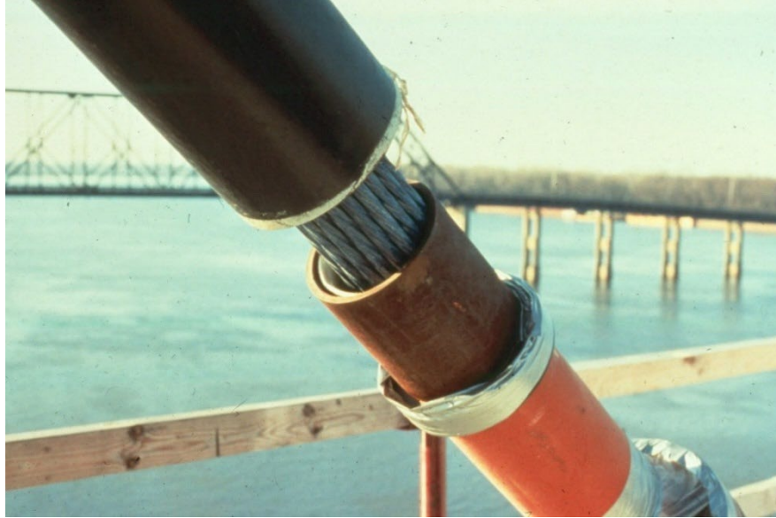
Figure 5.2.7 Parallel Strand Cable
