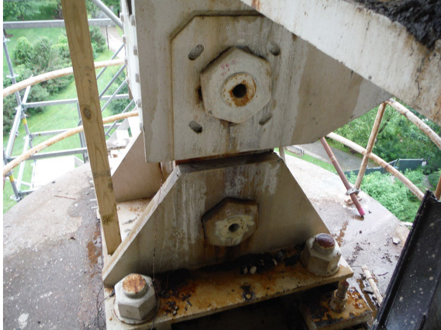
Figure 13.3.23 Fixed Bearing
