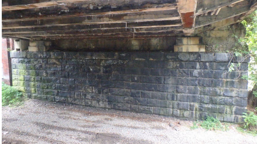
Figure 14.2.10 Stone Masonry Gravity Abutment
