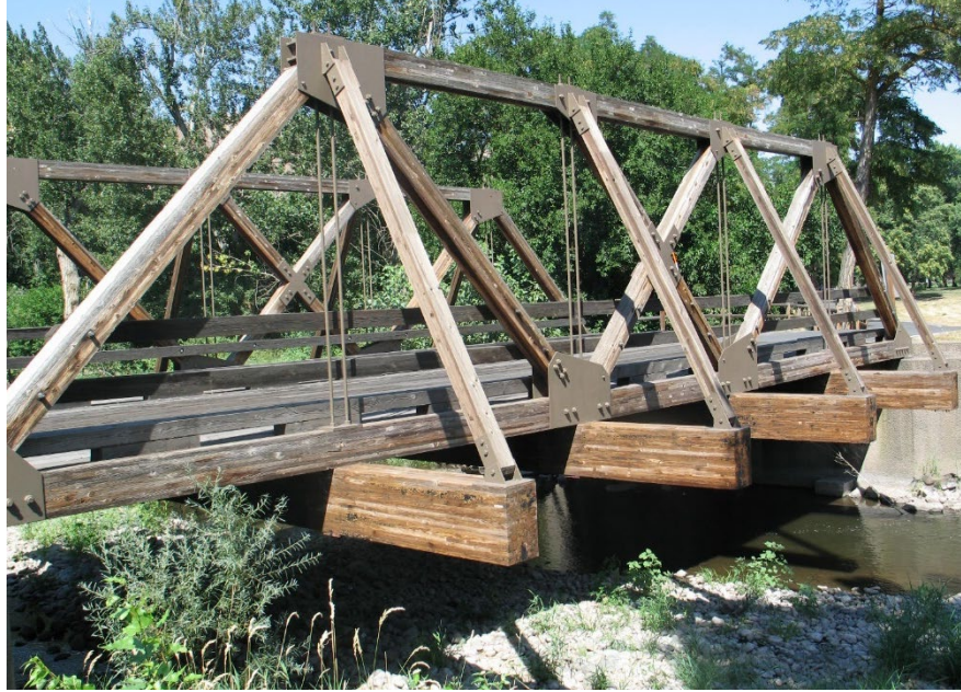
Figure 11.2.14 Timber Through Truss Bridge
