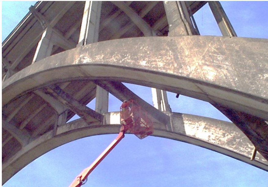
Figure 9.4.54 Inspection of Arch Strut (Secondary Member)
