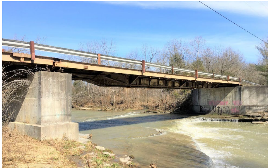
Figure 10.1.111 Elevation of a Converted Railroad Car Bridge
