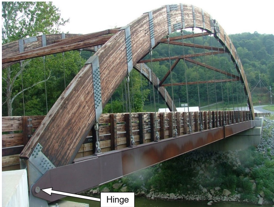
Figure 11.2.17 Glulam Arch Bridge with Steel Tie Girder
