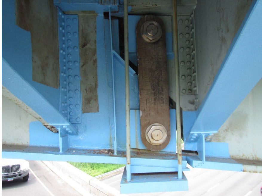
Figure 10.1.81 Rod and Saddle Retrofit
