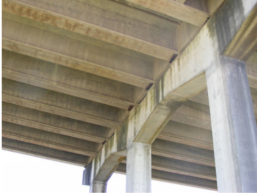
Figure 4.1.45 Multi-Beam Prestressed Concrete Bridge
