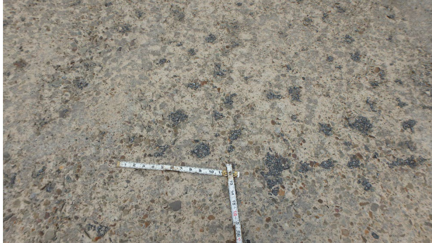
Figure 7.1.21 Heavy Scaling
