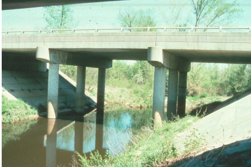
Figure 9.1.2 Typical Multi-Span Cast-in-Place Slab Bridge
