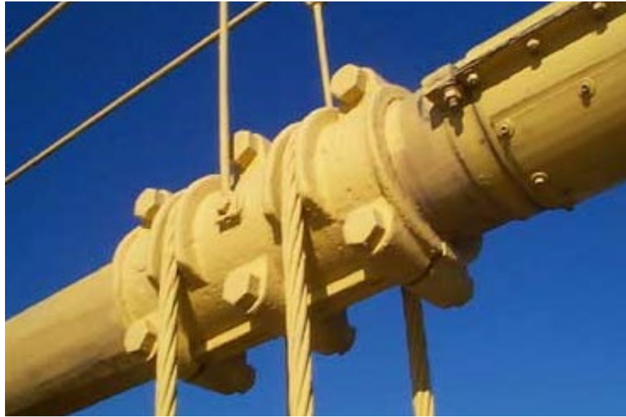
Figure 5.2.15 Grooved Cable Bands
