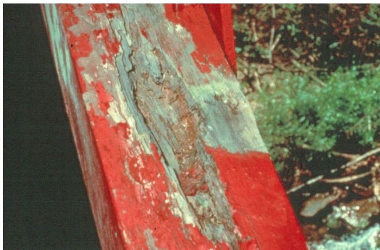
Figure 7.4.9 Decay of Wood by Fungi
