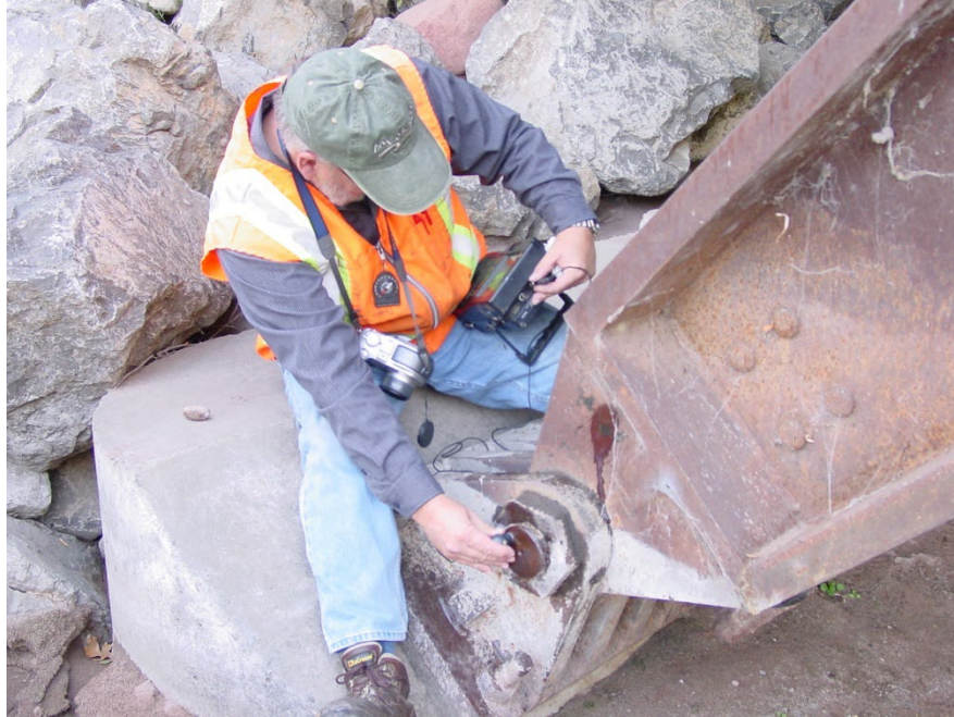
Figure 13.5.1 Ultrasonic Testing Inspection of a Pin in a Bearing
