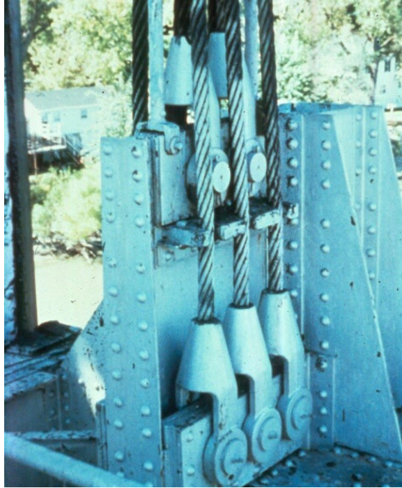
Figure 5.3.41 Wire Rope, Sockets, and Fittings
