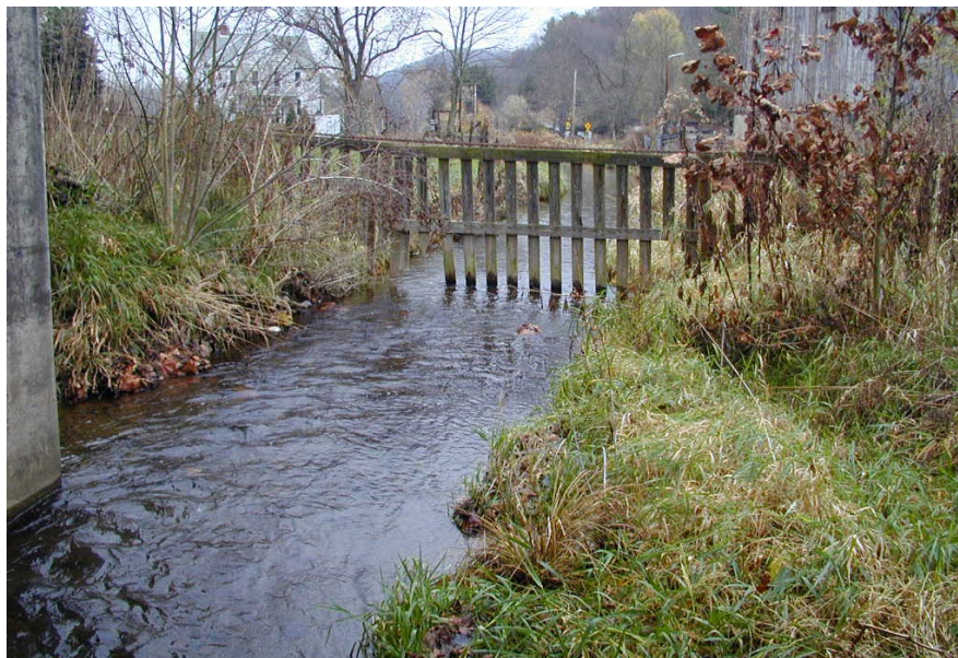
Figure 16.1.43 Fence in Stream at Bridge
