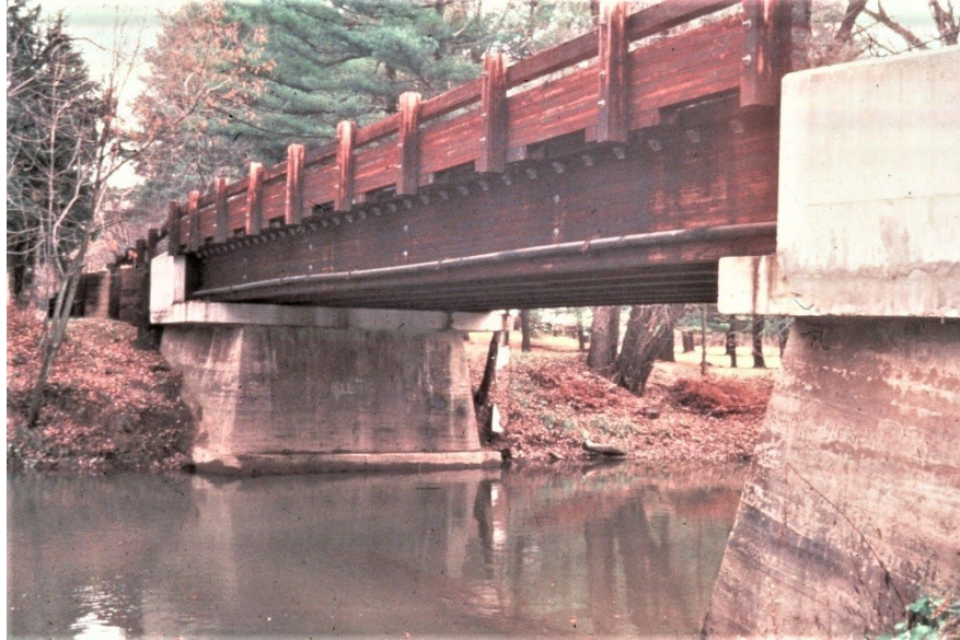
Figure 11.2.12 Elevation View of a Glulam Multi-Beam Bridge
