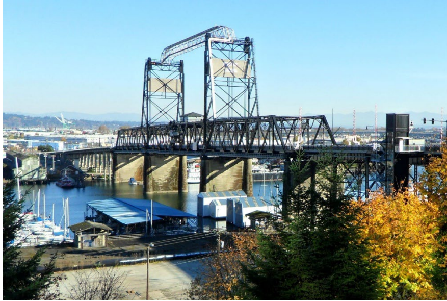
Figure 5.3.14 Connected-Tower Vertical Lift Bridge
