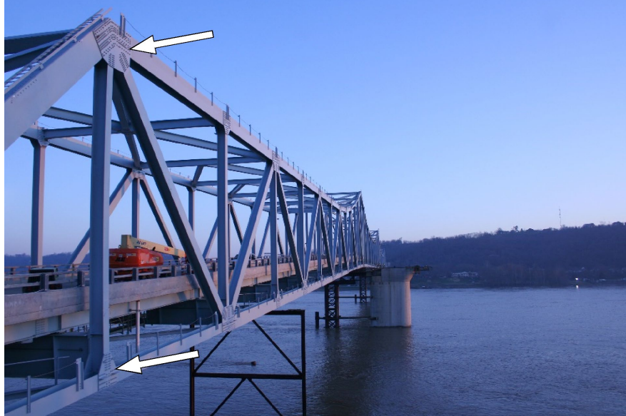
Figure 10.1.89 Steel Truss Superstructure with Gusset Plates
