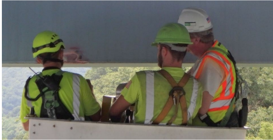
Figure 2.2.1 Inspectors Wearing Hard Hats
