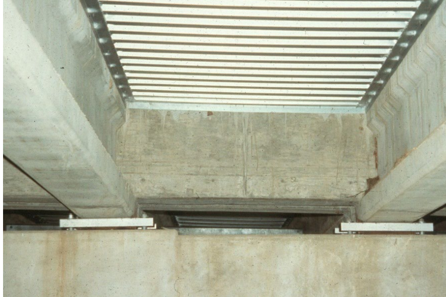
Figure 9.4.55 End Diaphragm (Secondary Member)
