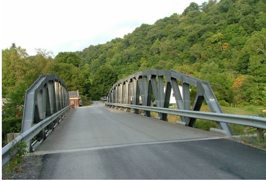
Figure 10.1.34 Single Span Camel Back Pratt Truss
