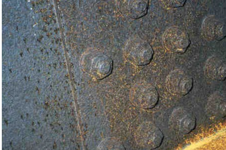
Figure 7.2.8 Chocolate Brown to Purple Brown - Fully Developed Oxide Film
