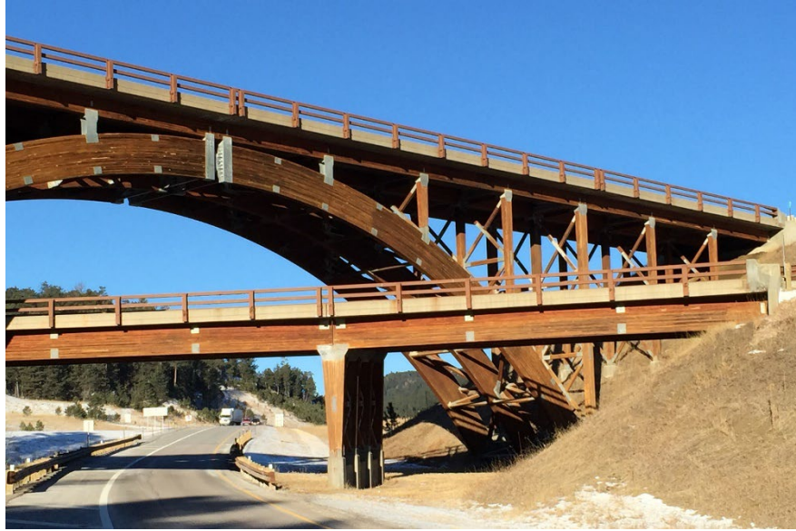
Figure 11.2.16 Glulam Arch Bridge over Glulam Multi-Beam Bridge
