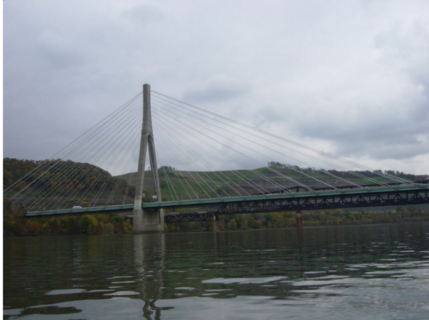
Figure 4.1.15 Cable-Supported Bridge: Cable-Stayed
