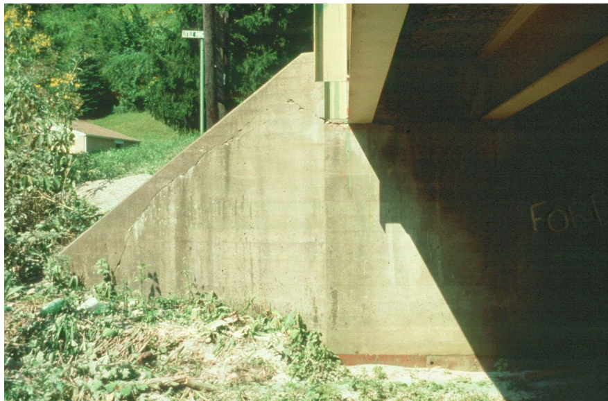
Figure 14.2.30 Flared Wingwall
