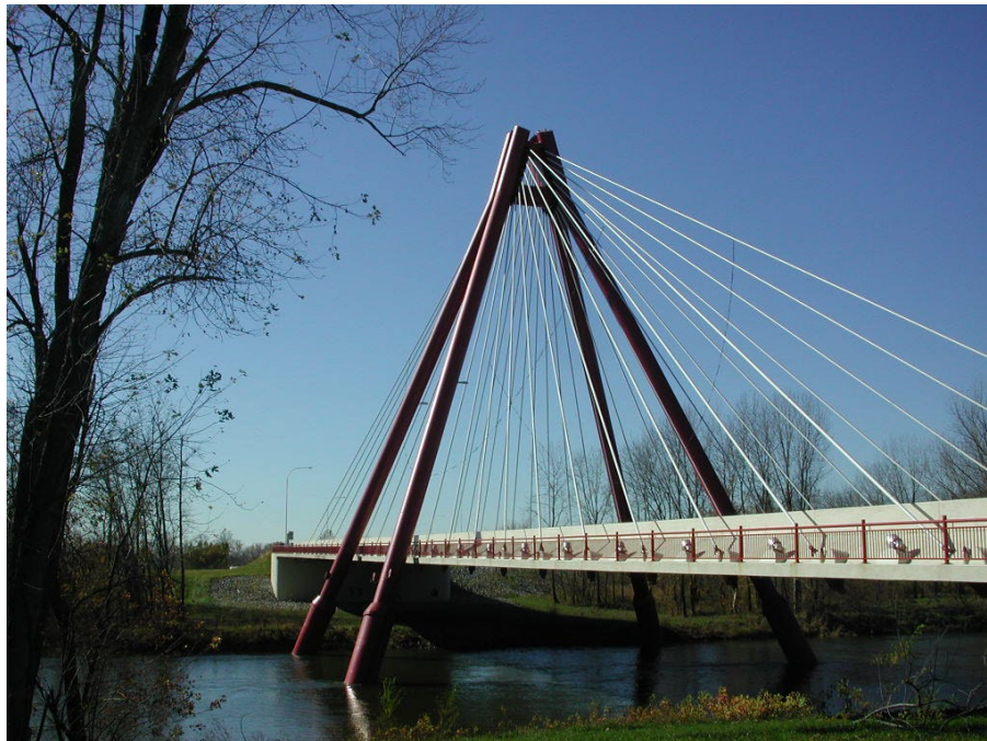
Figure 5.2.29 Oblique Double-Plane Cable System
