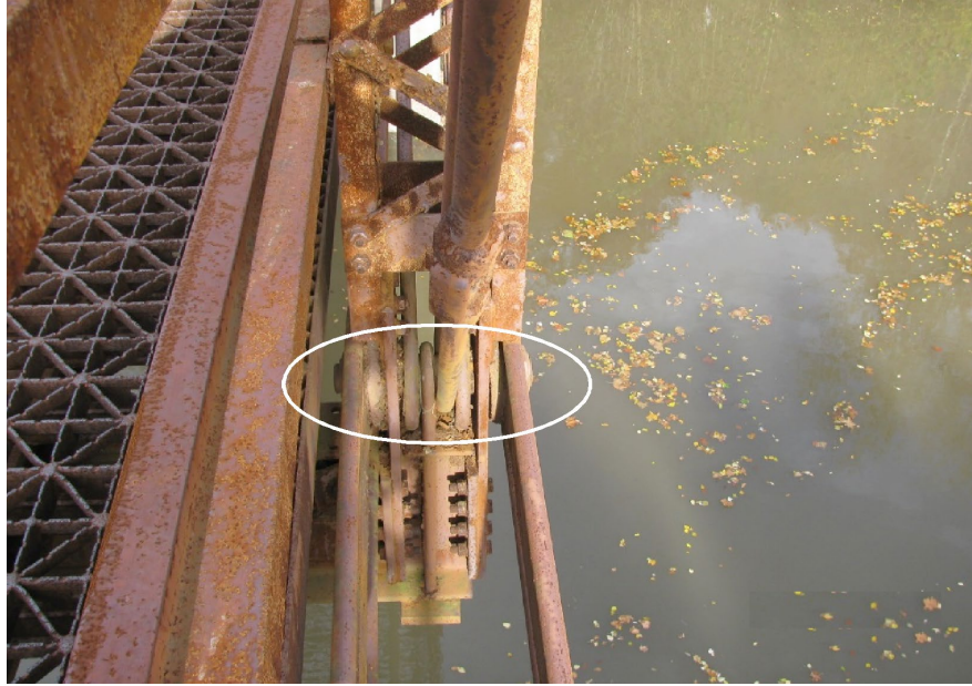
Figure 10.1.108 Loosely Packed Eyebar Connection
