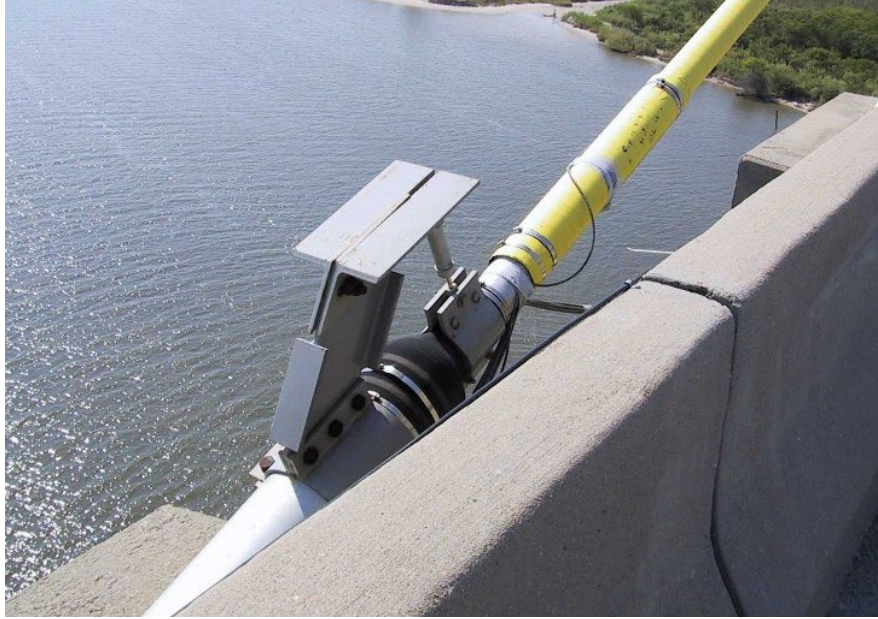
Figure 12.2.15 Small Shock Absorber Damper
