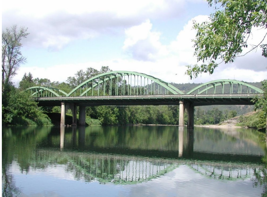
Figure 10.1.60 Three-Span Tied Arch Bridge
