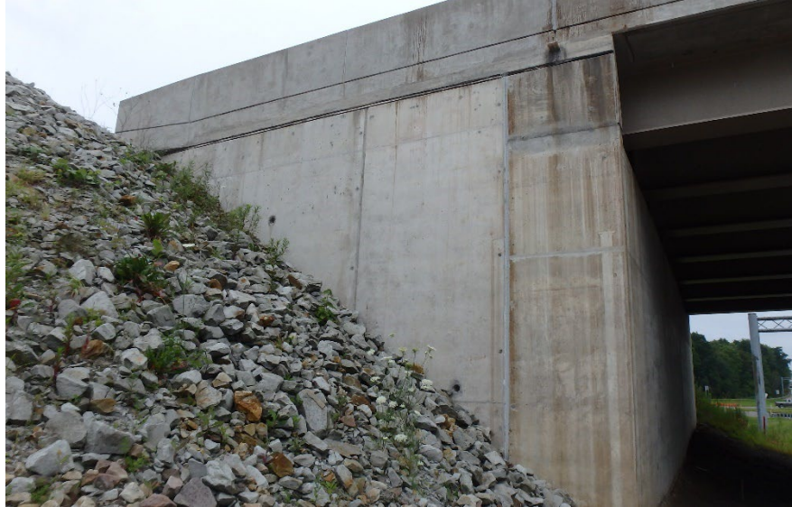
Figure 14.2.31 U-shaped Wingwall
