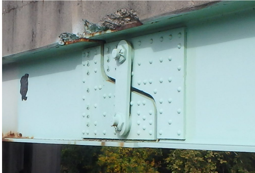
Figure 4.1.23 Pin and Hanger Assembly
