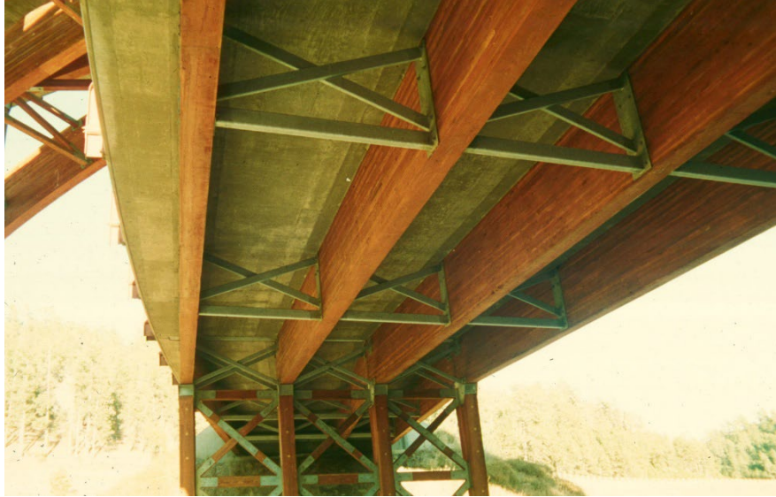
Figure 11.5.10 Steel Diaphragms Bolted to Glulam Beams
