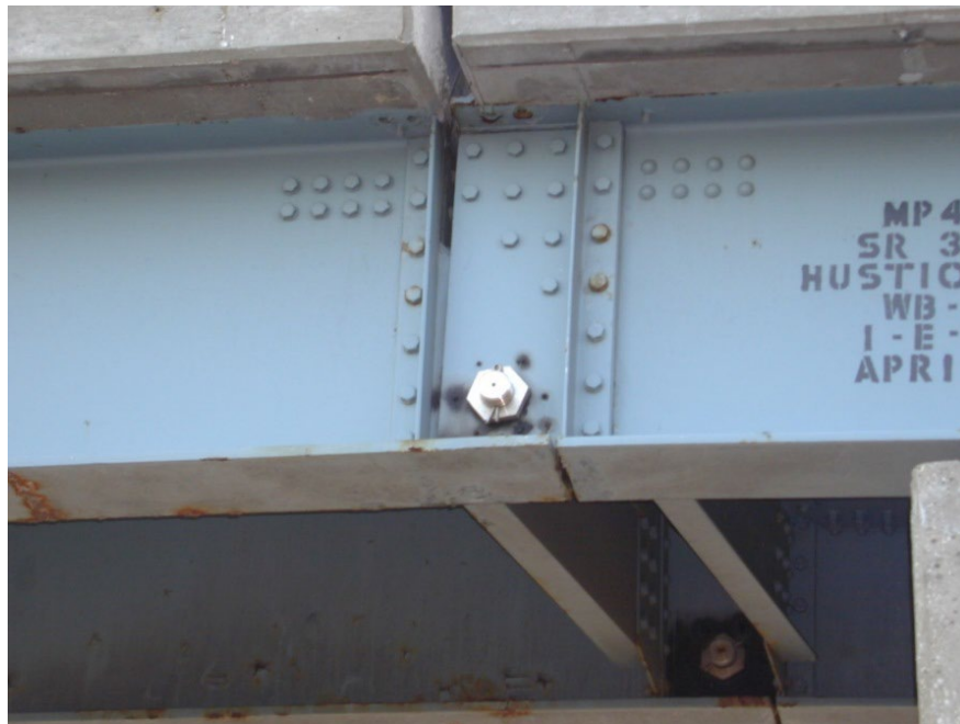
Figure 10.1.76 Single Pin Assembly
