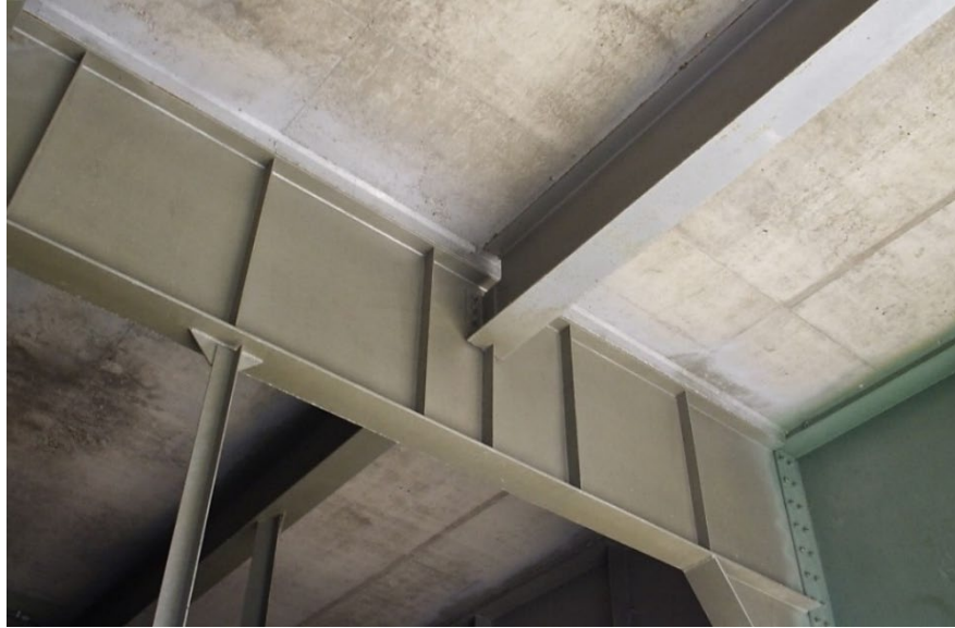
Figure 4.1.29 Underside View of a Bridge Deck
