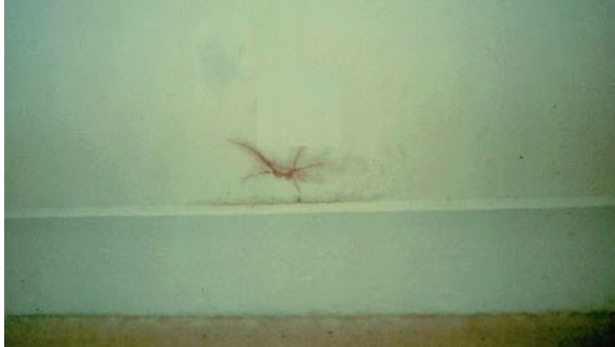
Figure 7.3.37 Through Crack in the Web
