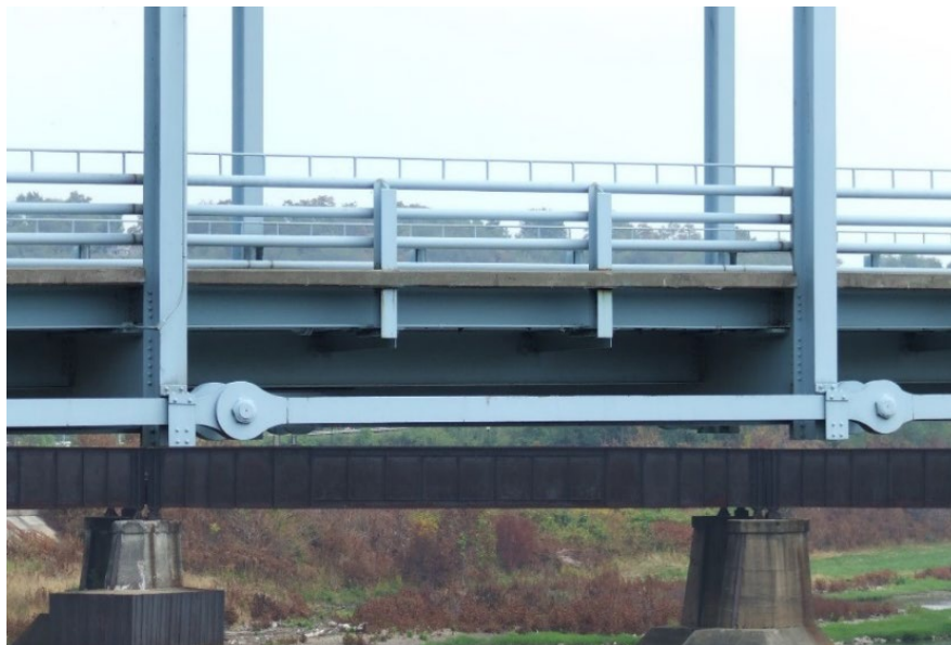
Figure 4.1.19 Pin-Connected Eyebars
