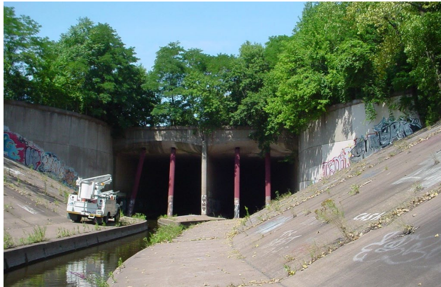
Figure 4.3.13 Formed Concrete Channel Lining
