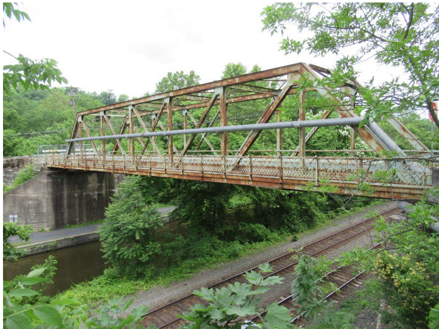
Figure 10.1.25 Simple Span Truss
