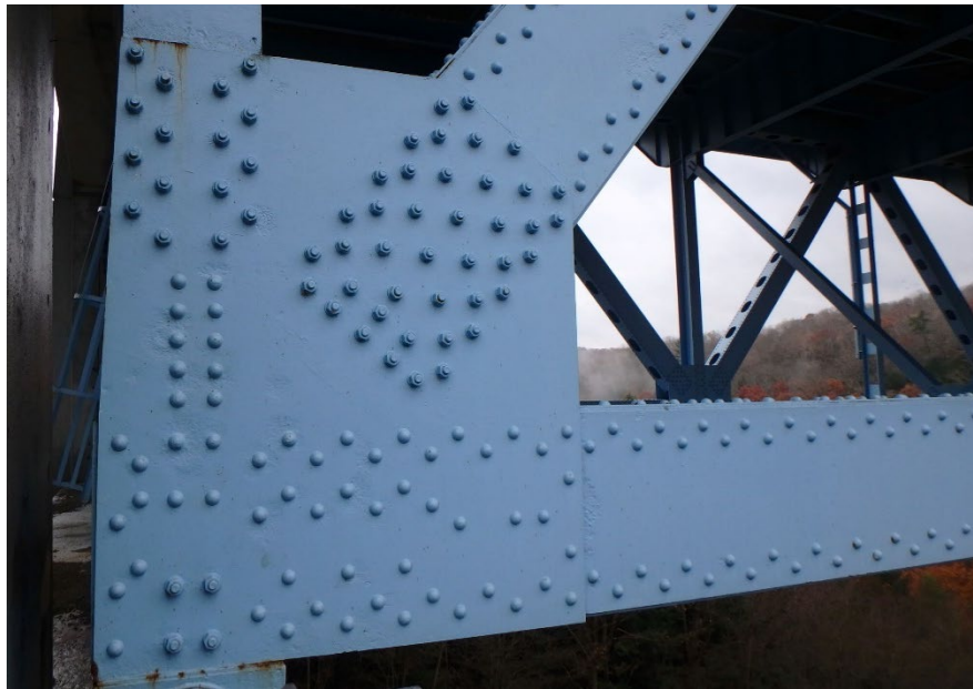
Figure 10.1.47 Truss Panel Point using Rivets and Bolts
