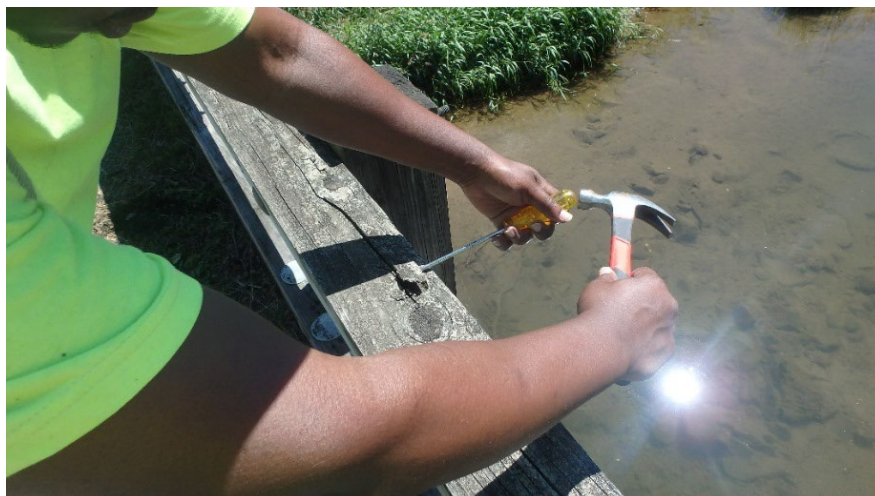
Figure 8.3.7 Inspector Probing Timber with a Pick
