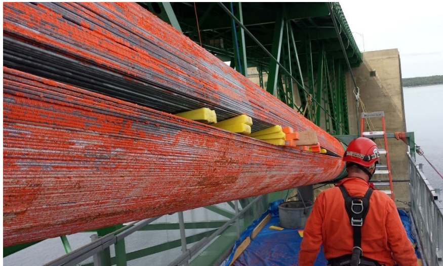
Figure 12.2.1 Inspection of Cable with Wedges
