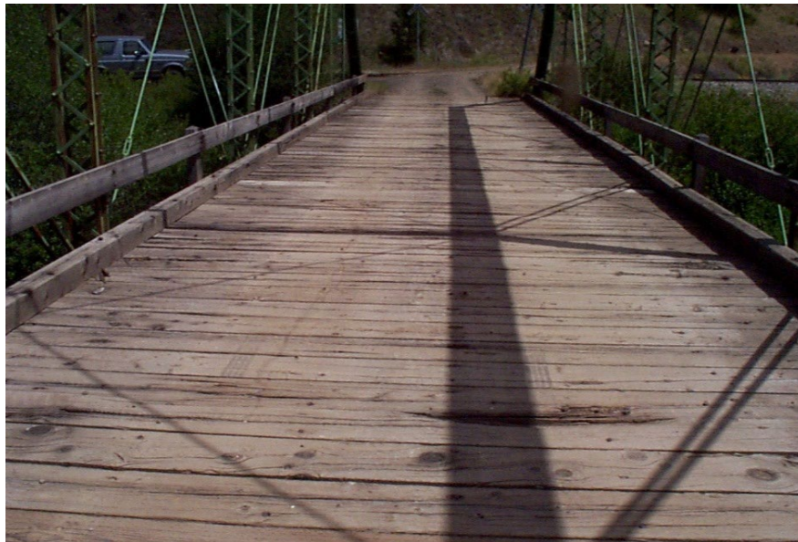
Figure 4.1.34 Plank Deck
