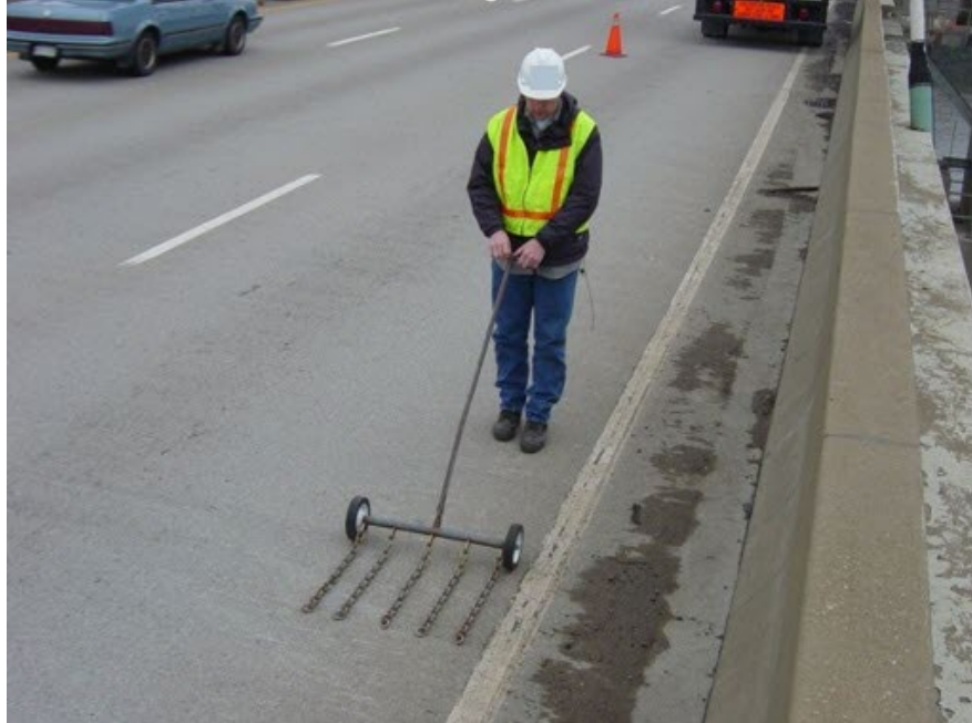
Figure 8.1.7 Sounding for Delaminated Areas of Concrete
