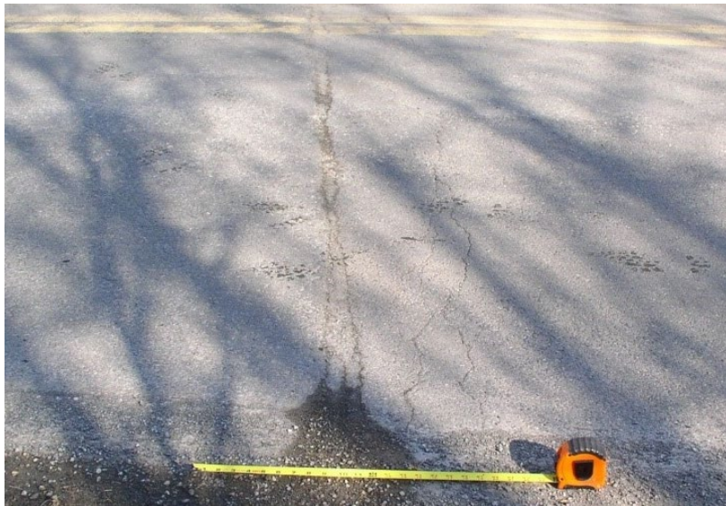
Figure 8.5.29 Asphalt Wearing Surface over an Expansion Joint
