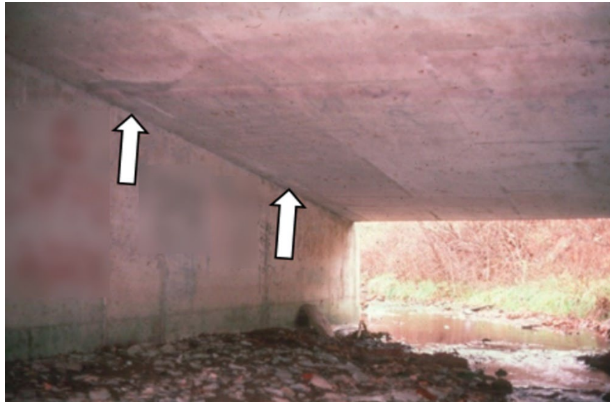
Figure 9.4.1 Bearing Area: Cast-in-Place Slab
