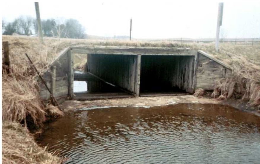
Figure 15.2.5 Timber Box Culvert
