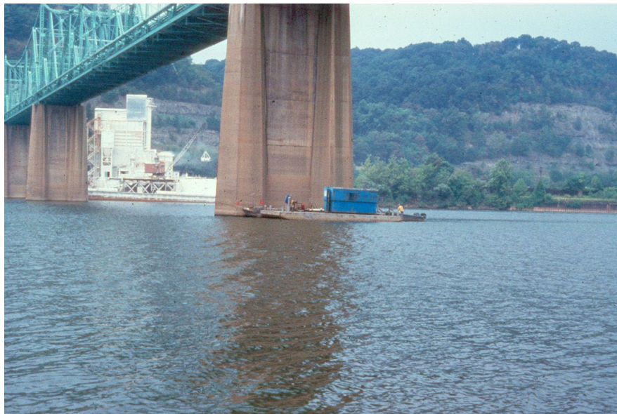
Figure 2.5.13 Inspection Operations from a Barge
