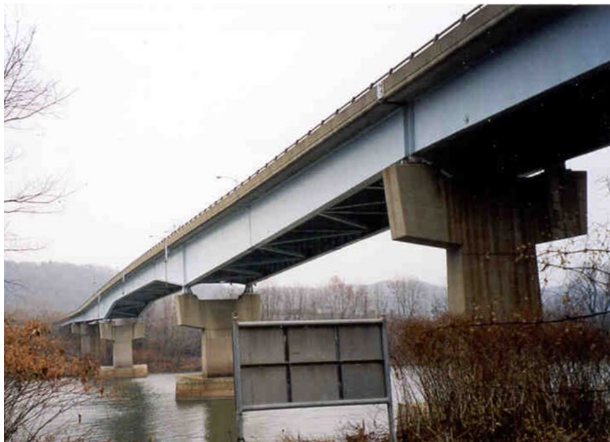
Figure 7.2.5 Built-up Girders
