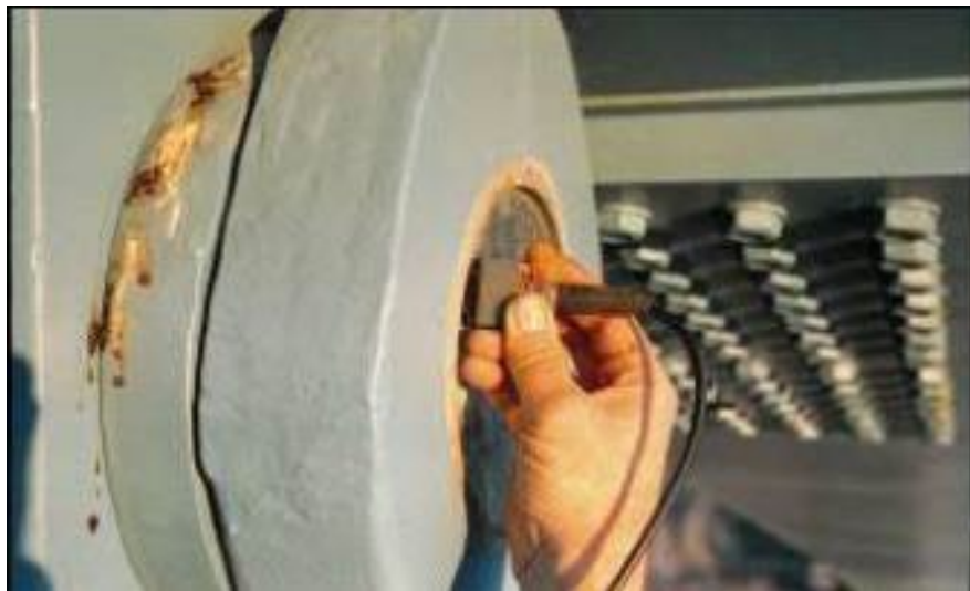
Figure 10.4.56 Ultrasonic Inspection of an Eyebar Pin
