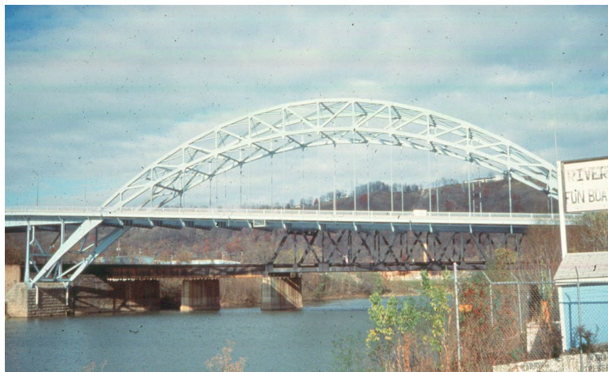
Figure 10.1.58 Braced Rib Through Arch Bridge
