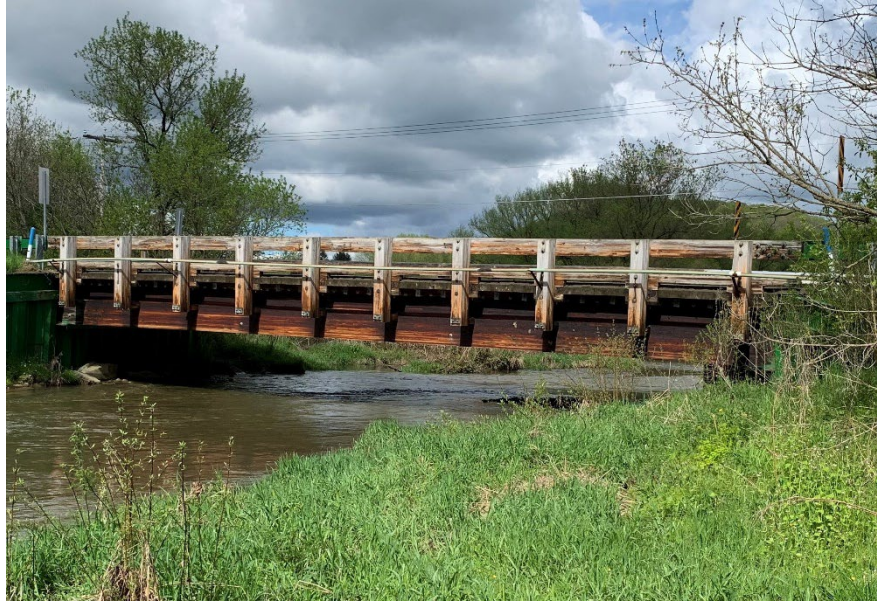
Figure 7.4.1 Glued-Laminated Modern Timber Bridge
