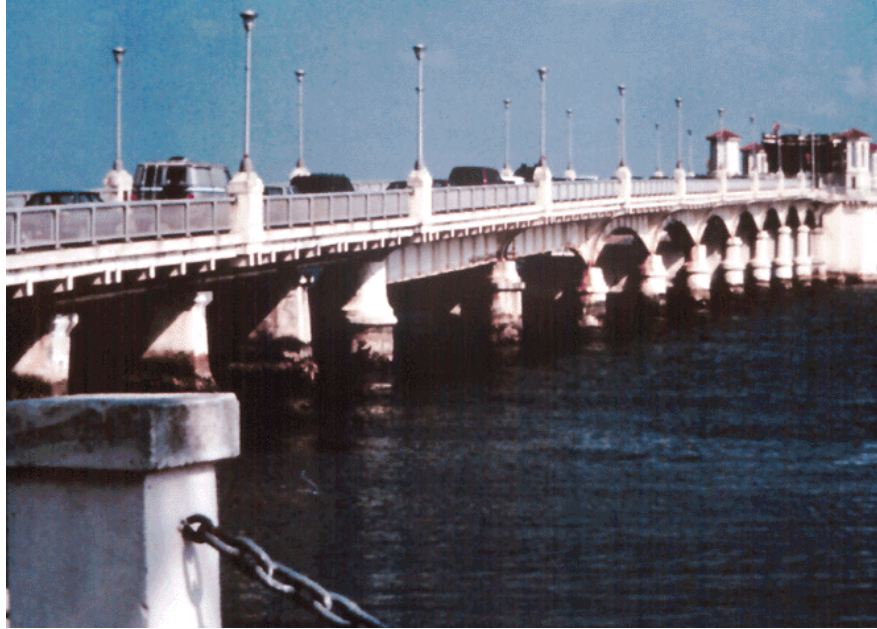
Figure 16.1.9 Large Number of Piers Reducing the Hydraulic Opening
