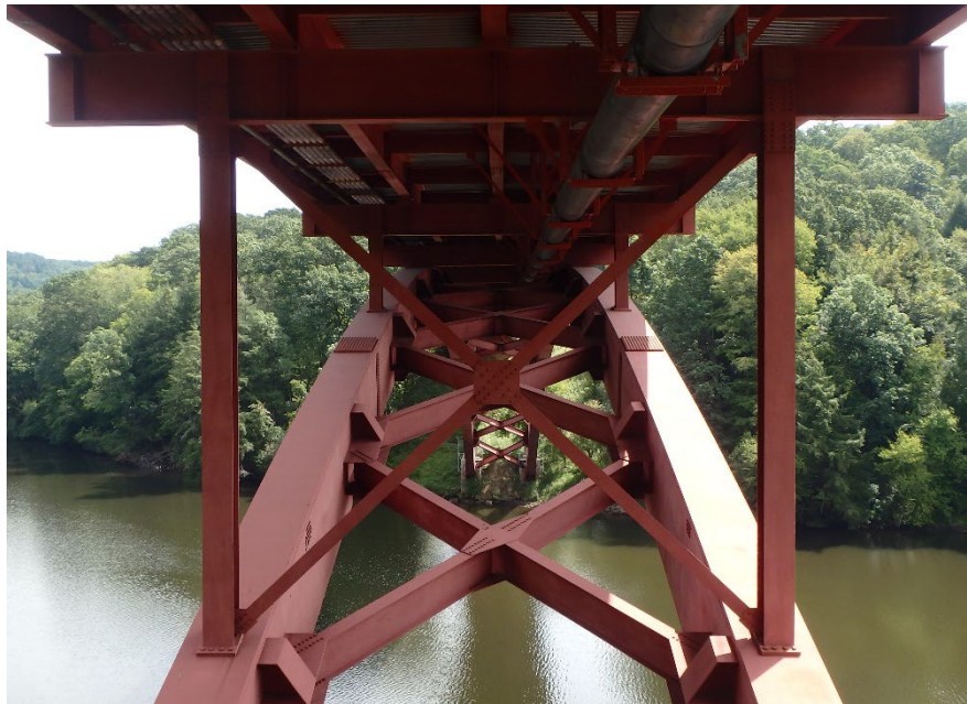
Figure 10.4.9 Braced Rib Deck Arch Showing Spandrel Columns
