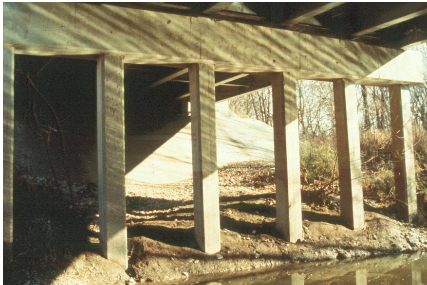
Figure 14.2.48 Concrete Pile Bent
