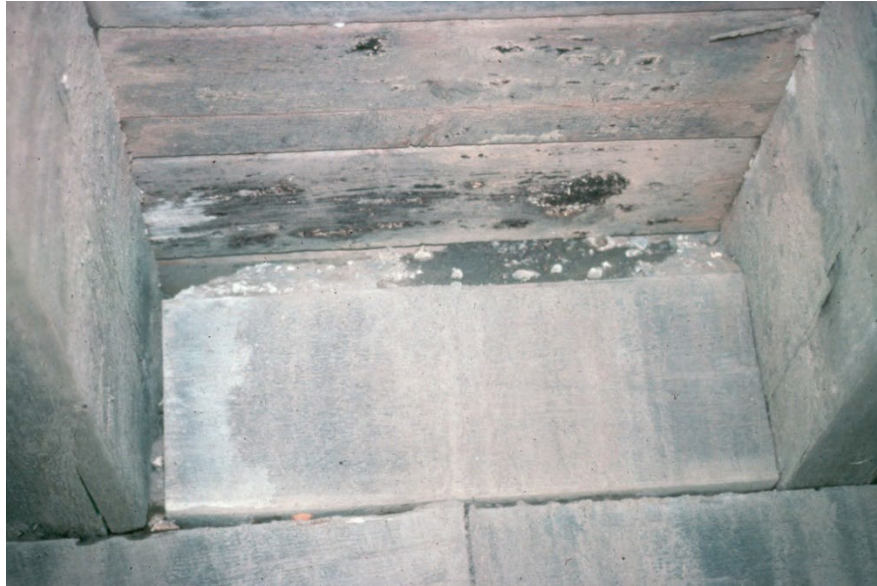
Figure 11.5.7 Typical Timber End Diaphragm
