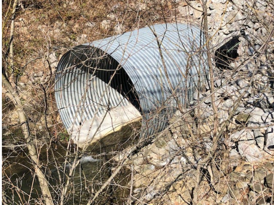
Figure 4.2.14 Culvert End Projection
