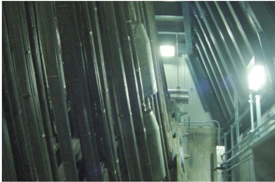
Figure 12.2.11 Chain Gallery (Anchor Vault) Interior
