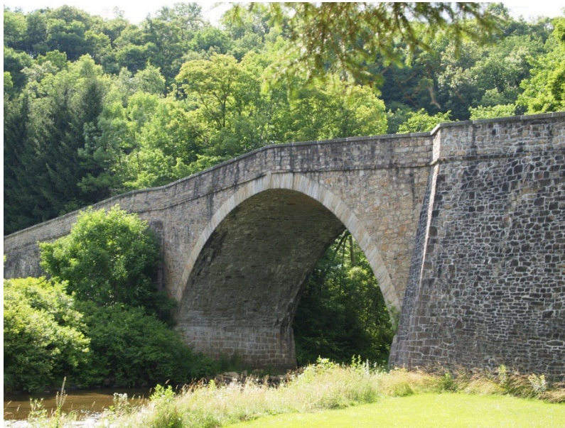
Figure 7.5.1 Stone Masonry Arch
