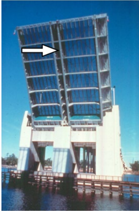
Figure 5.3.40 Engaged Transverse Locks
