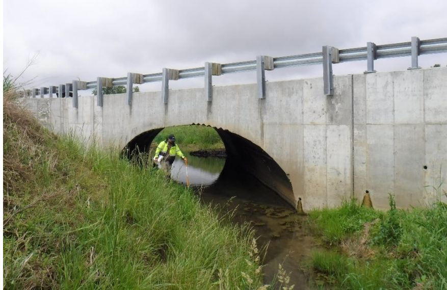
Figure 15.5.21 Flexible Culvert with Concrete Headwall
