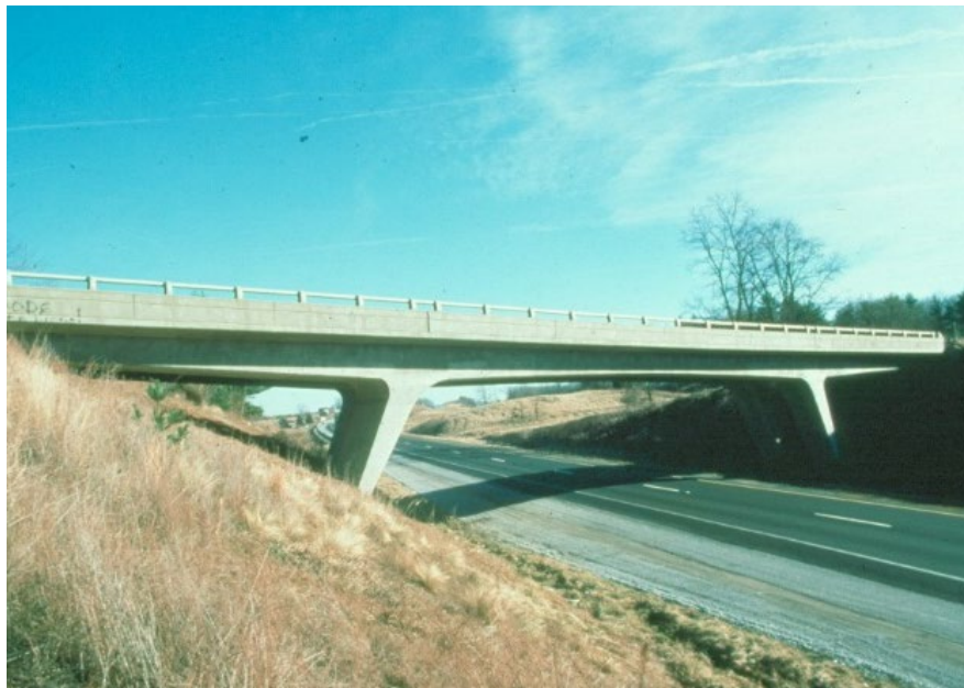
Figure 9.1.24 Three Span Concrete K-frame Bridge
