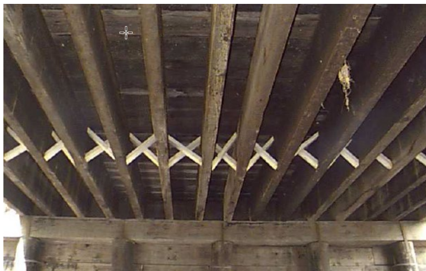
Figure 4.1.44 Multi-Beam Timber Bridge
