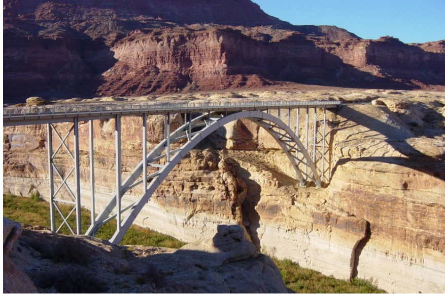
Figure 10.1.52 Deck Arch Bridge
