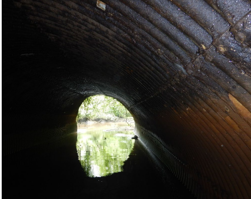
Figure 15.5.1 Sighting Along Culvert to Check Alignment
