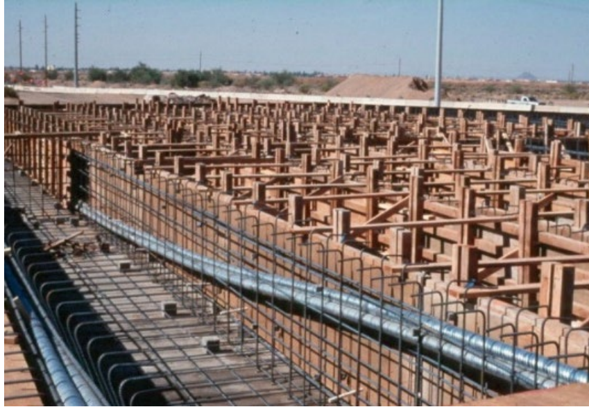
Figure 9.4.48 Post-tensioning Tendon Duct
