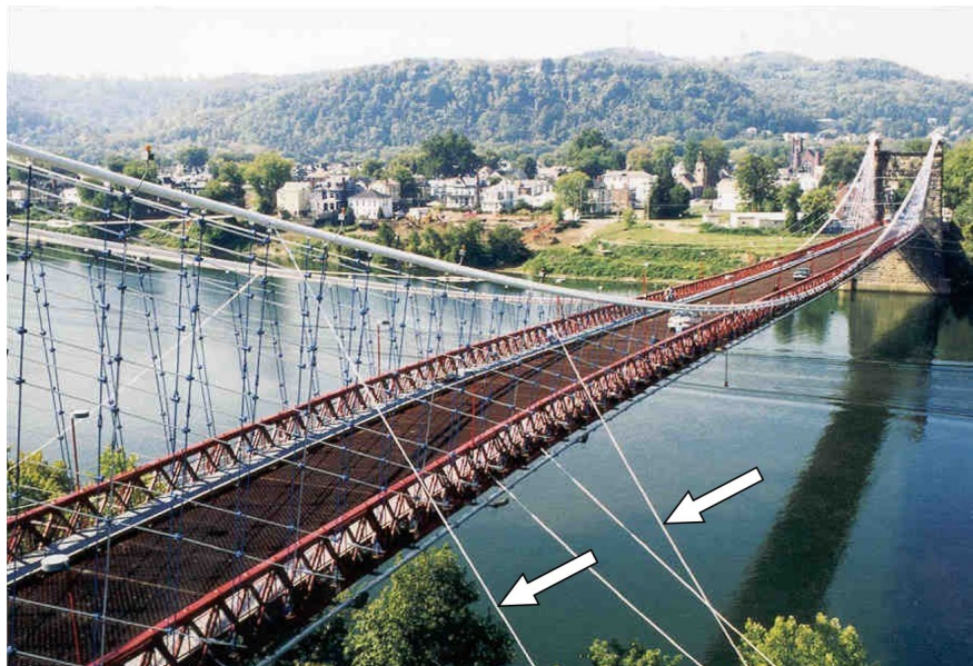
Figure 5.2.19 Cable Damping System for Suspension Bridge
