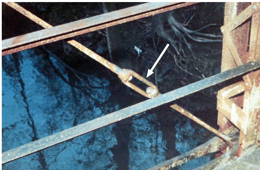
Figure 10.4.54 Turnbuckle on a Truss Diagonal
