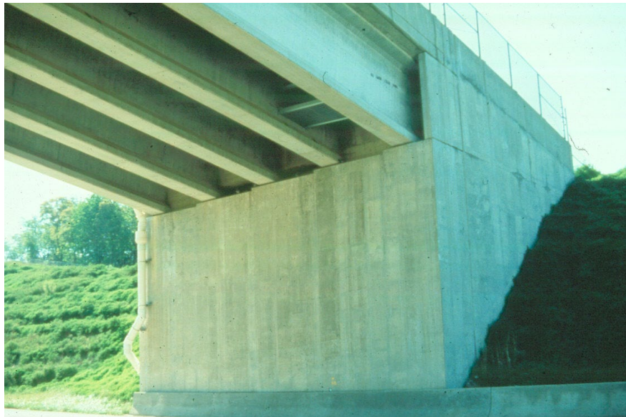
Figure 14.2.13 Full Height Abutment
