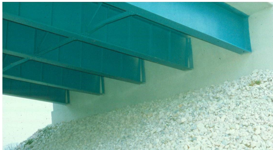
Figure 4.1.78 Integral Abutment
