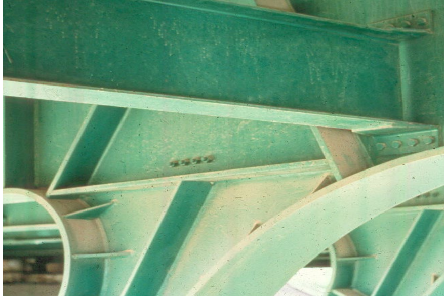
Figure 10.1.66 Connection Between Legs and Girder Portion
