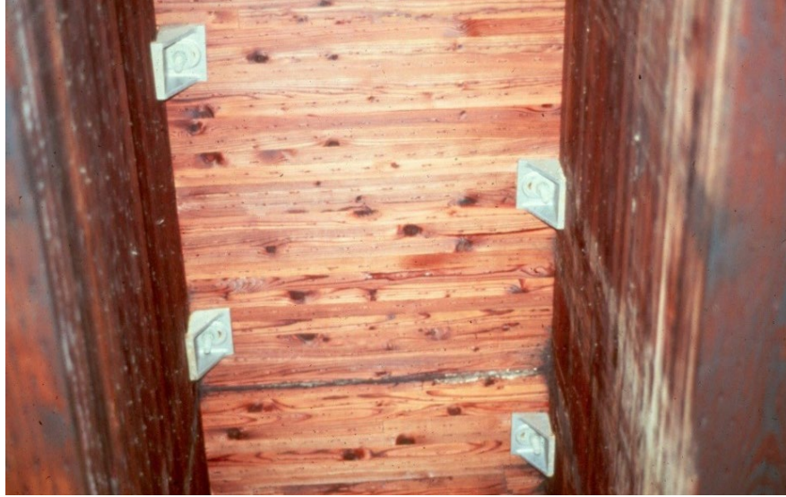
Figure 8.3.3 Glued-laminated Deck Panels Attached to Superstructure
