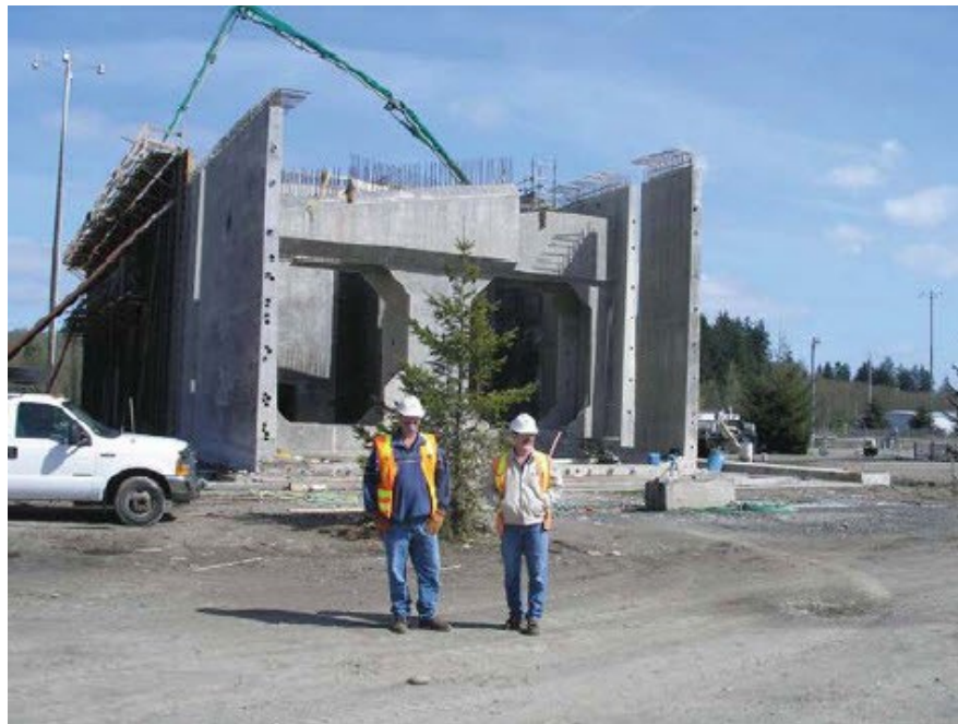
Figure 5.4.5 Concrete Pontoons Under Construction
