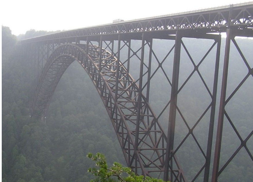
Figure 10.1.55 Braced Rib Deck Arch Bridge
