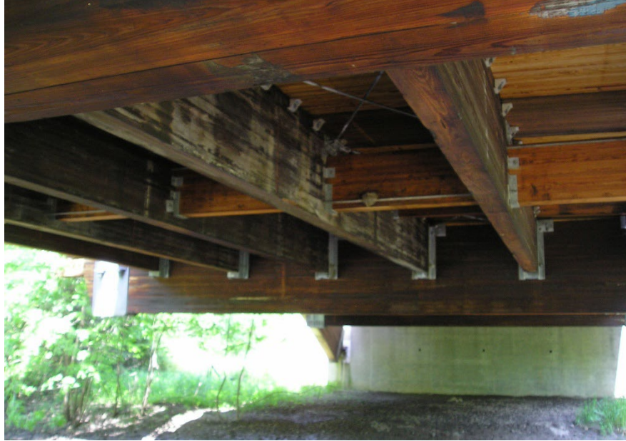
Figure 11.2.11 Underside View of a Glulam Timber Bridge
