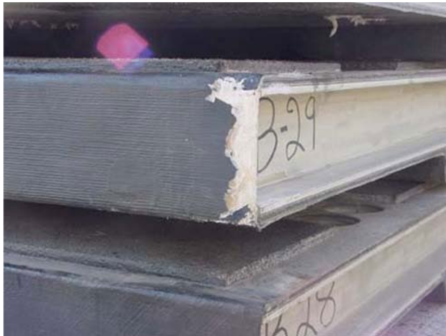
Figure 7.6.15 Fiber Exposure from Improper Handling and Erection Methods
