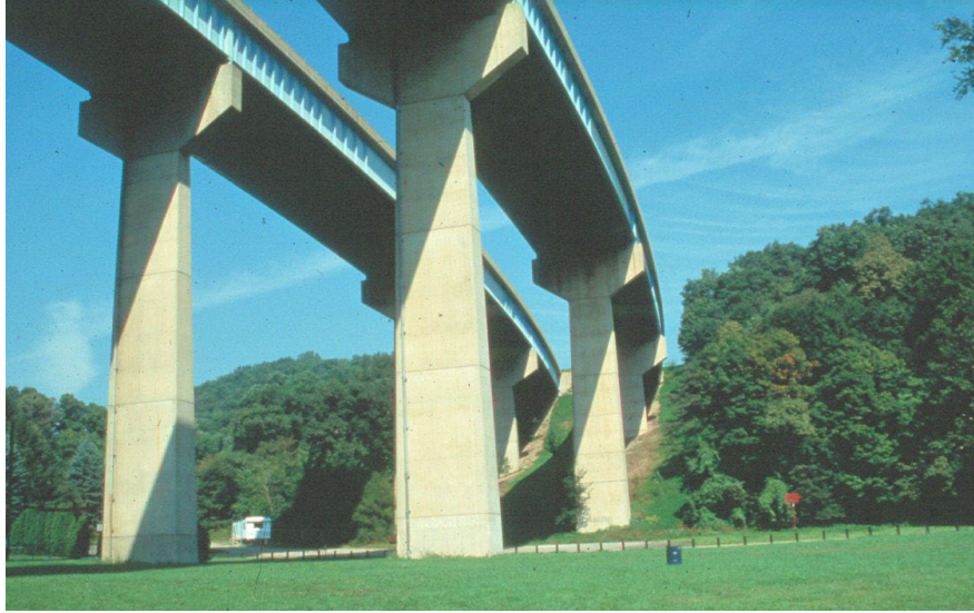
Figure 14.2.36 Typical Concrete Piers
