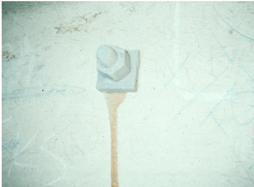
Figure 9.4.35 Transverse Tie Bolt with Epoxy
