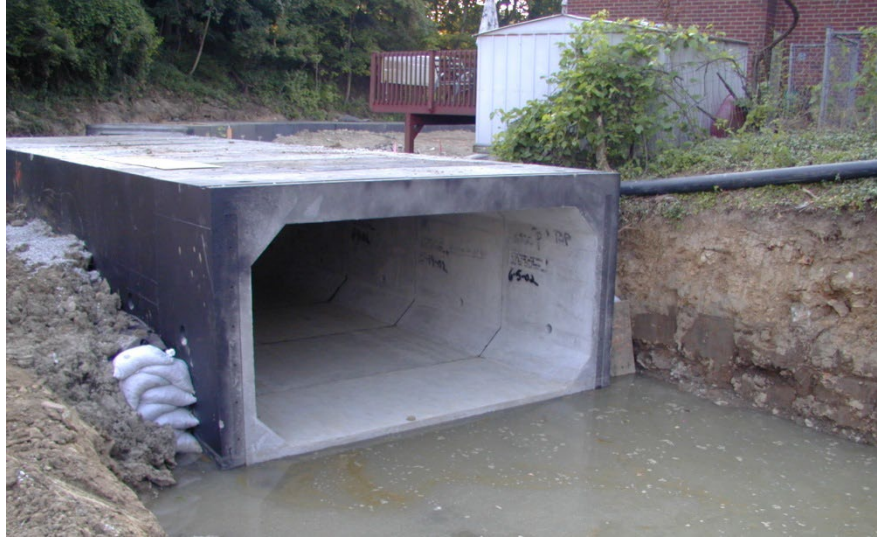
Figure 15.2.4 Precast Concrete Box Culvert under Construction
