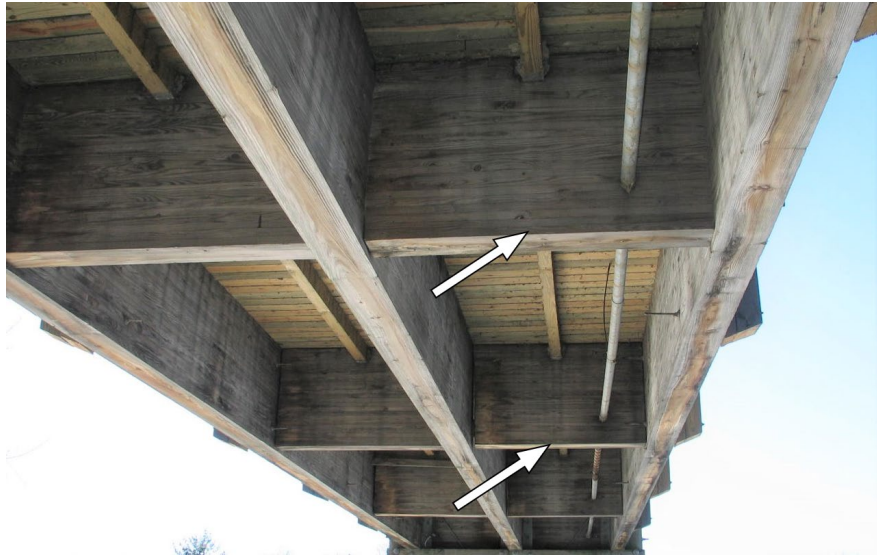
Figure 11.2.18 Glulam Diaphragms
