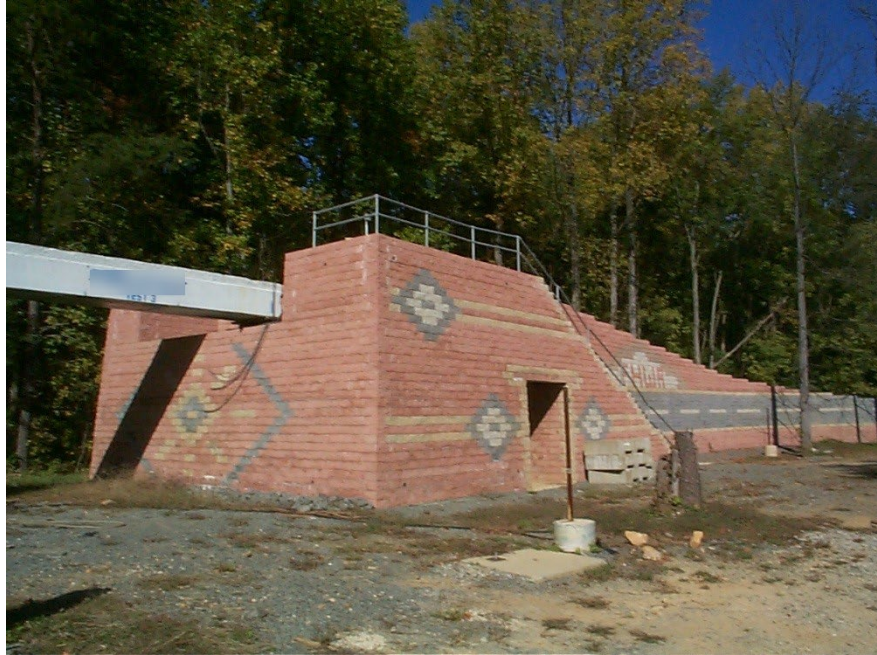
Figure 14.2.20 GRS Bridge Abutment at the FHWA Highway Research Center
