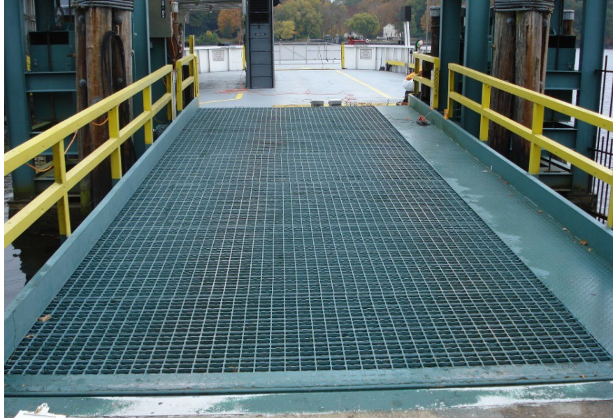
Figure 5.5.2 Ferry Transfer Bridge Steel Grid Deck
