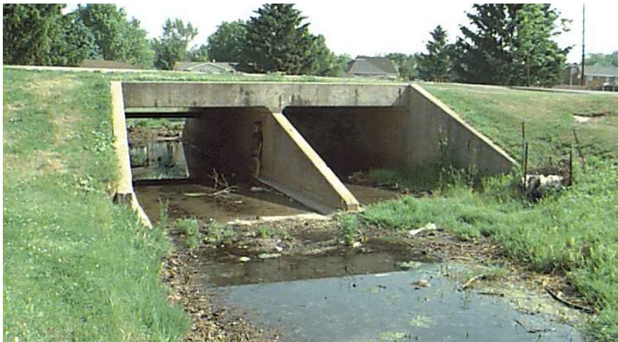
Figure 15.2.3 Multi-Cell Concrete Box Culvert
