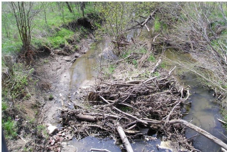
Figure 16.1.46 Debris and Sediment in the Channel
