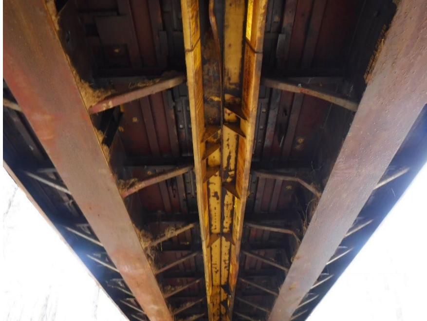
Figure 10.1.113 Underside of a Double Converted Railroad Car Bridge
