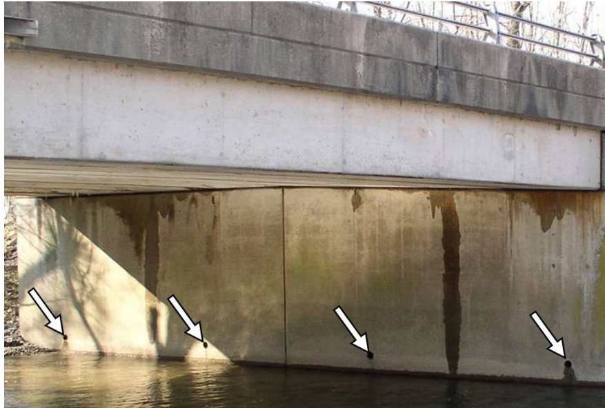
Figure 8.5.24 Weep Holes
