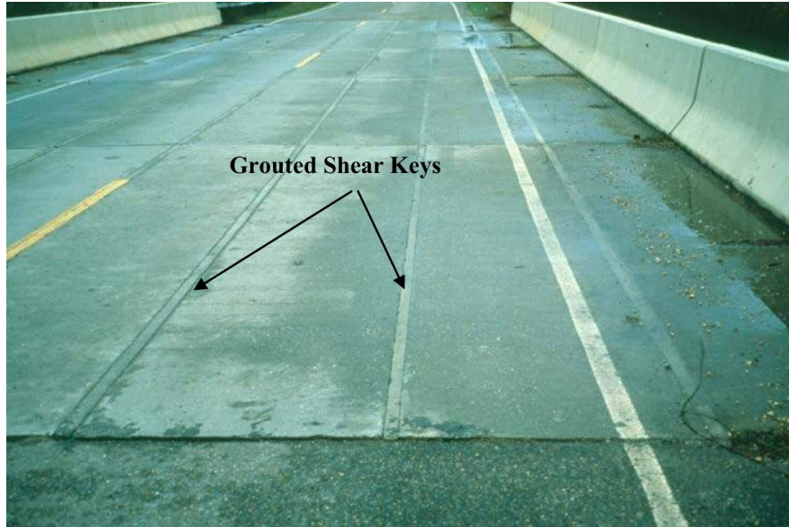
Figure 9.4.34 Top Surface of Deck of Precast Channel Beam Bridge
