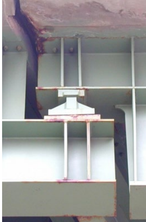
Figure 4.1.24 Cantilevered/Suspended Beam Seat
