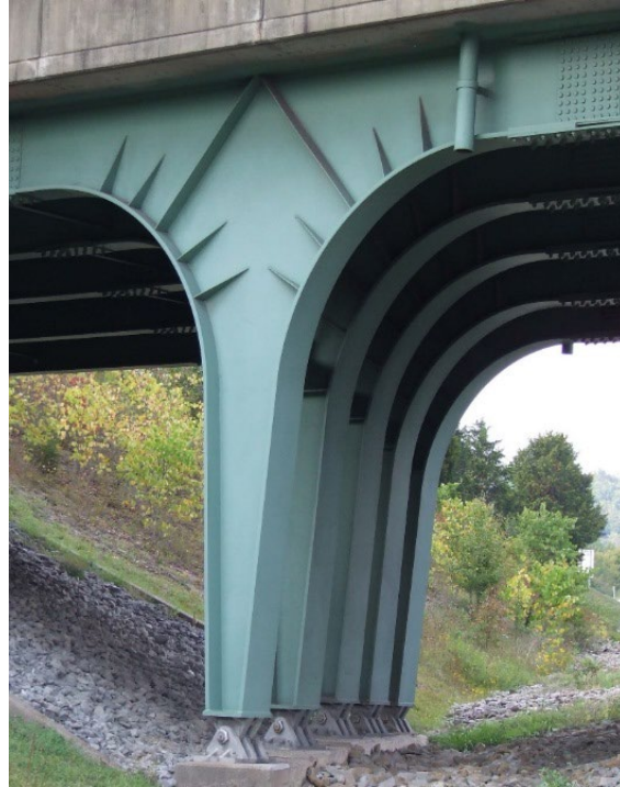
Figure 10.1.65 Rigid Frame Bridge Constructed of Multiple Frames
