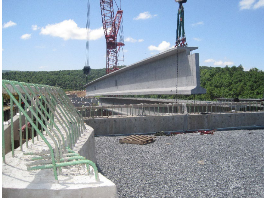
Figure 9.1.48 Placement of an AASHTO-PCI Bulb Tee Beam
