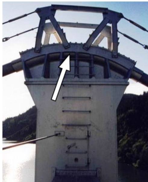
Figure 5.2.14 Cable Saddle
