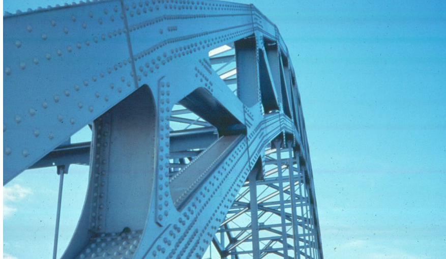
Figure 10.4.18 Through Truss Arch Compressive Members
