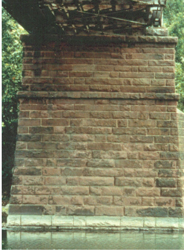
Figure 14.2.38 Stone Masonry Pier
