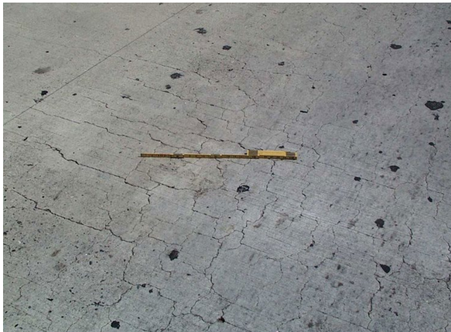
Figure 7.1.15 Shrinkage Cracks
