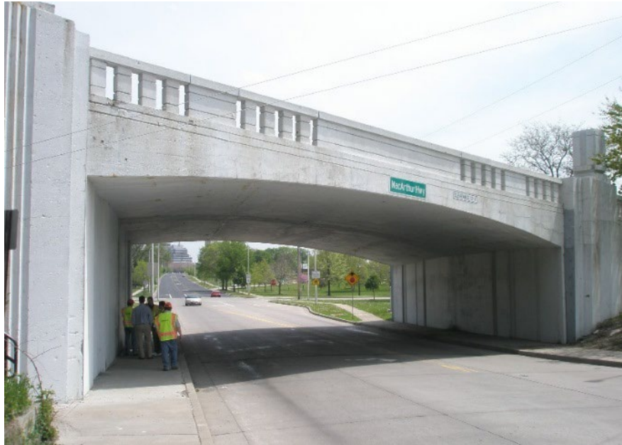
Figure 9.1.23 Single-span Rectangular Concrete Rigid Frame Bridge
