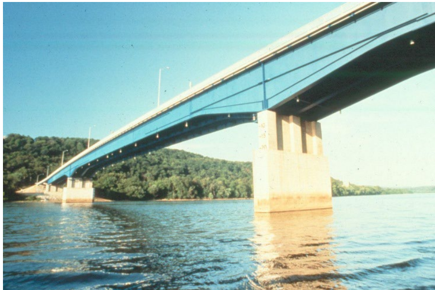
Figure 10.1.11 Fabricated Variable Depth Girder Bridge
