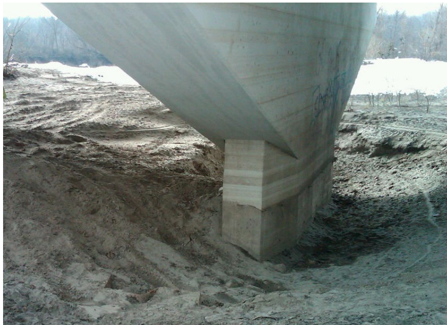
Figure 16.1.14 Local Scour at a Pier
