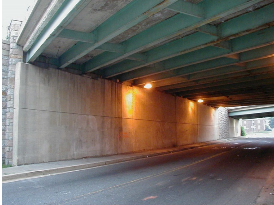
Figure 4.1.75 Cantilever Abutment (or Full Height Abutment)
