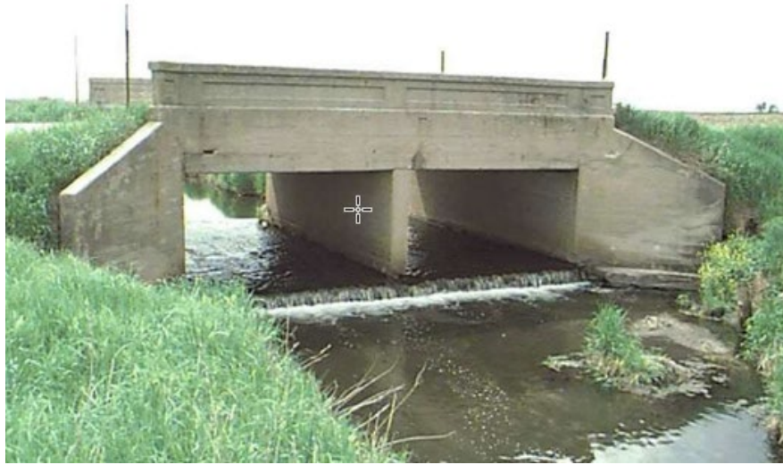
Figure 4.2.2 Box Culvert with Shallow Cover
