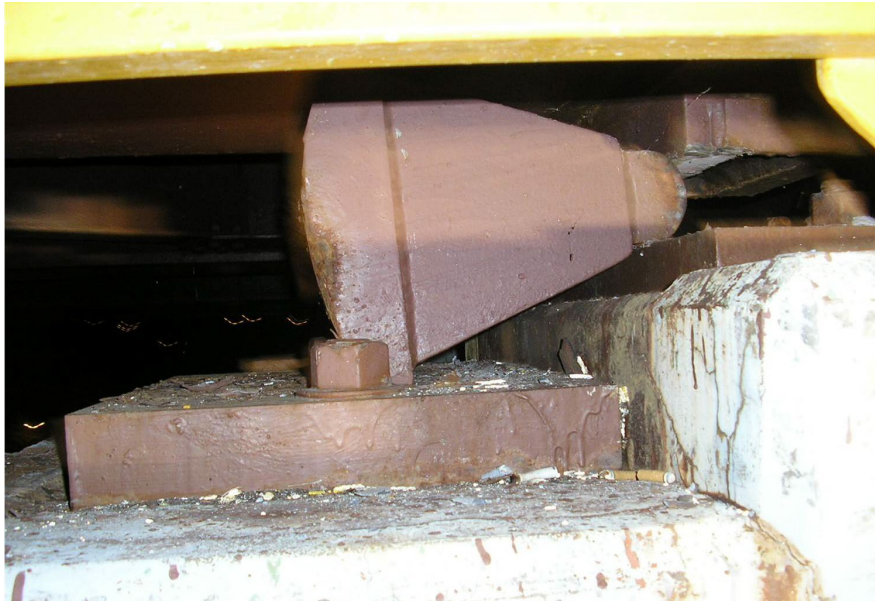
Figure 13.6.9 Overturned Rocker Bearing
