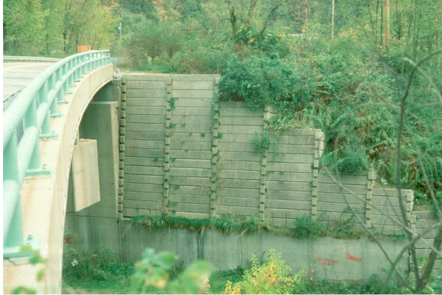
Figure 14.2.29 Straight Cribbed Wingwall
