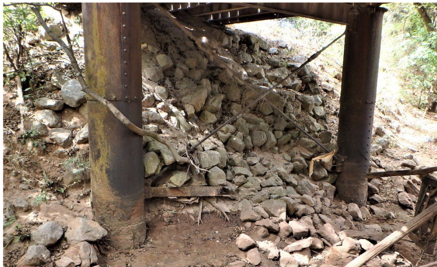
Figure 14.2.59 Caissons with Permanent Steel Casing
