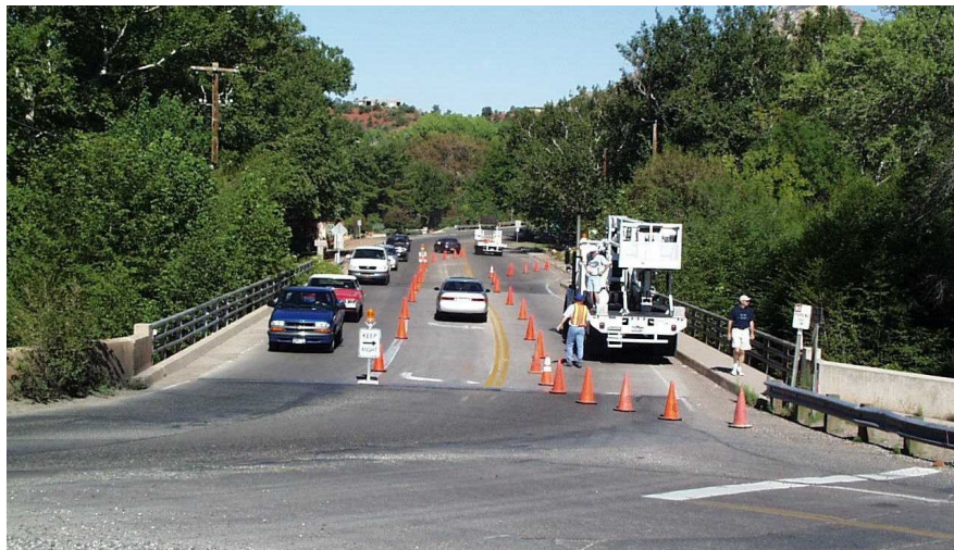
Figure 2.3.1 Temporary Traffic Control Operation
