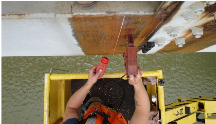
Figure 10.5.10 Magnetic Particle Testing on Sherman Minton Bridge
