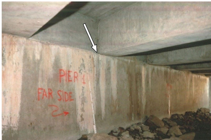
Figure 9.4.2 Bearing Area: Cast-in-Place Concrete Tee Beam Bridge
