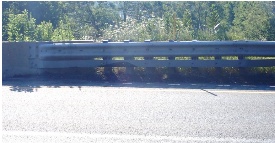
Figure 8.6.3 Bridge Railing Transition
