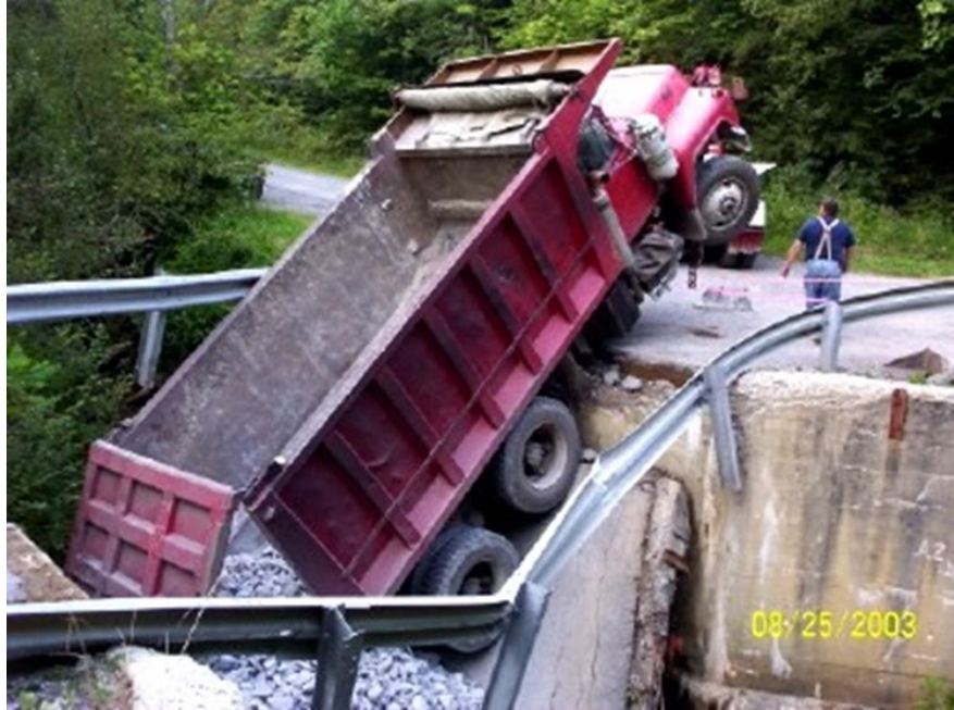
Figure 7.1.33 Overload Damage
