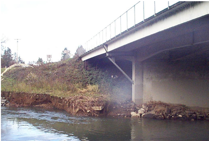
Figure 16.1.22 Channel Degradation due to Lateral Migration
