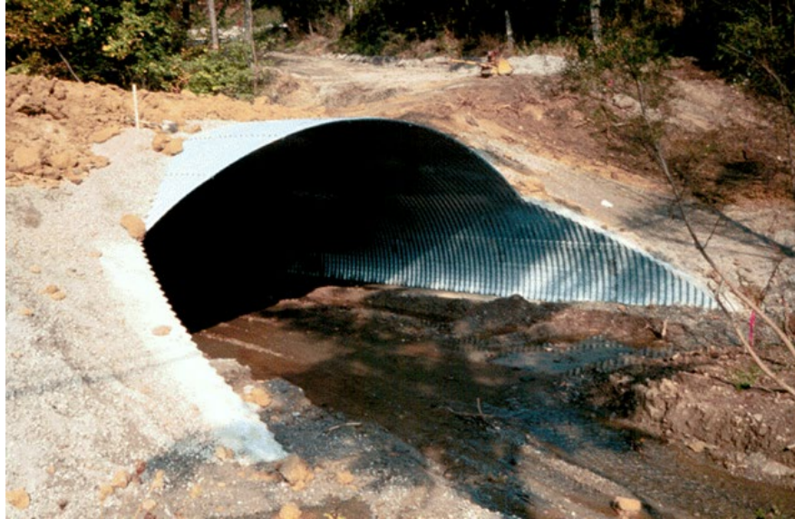
Figure 4.2.5 Pipe Arch Culvert
