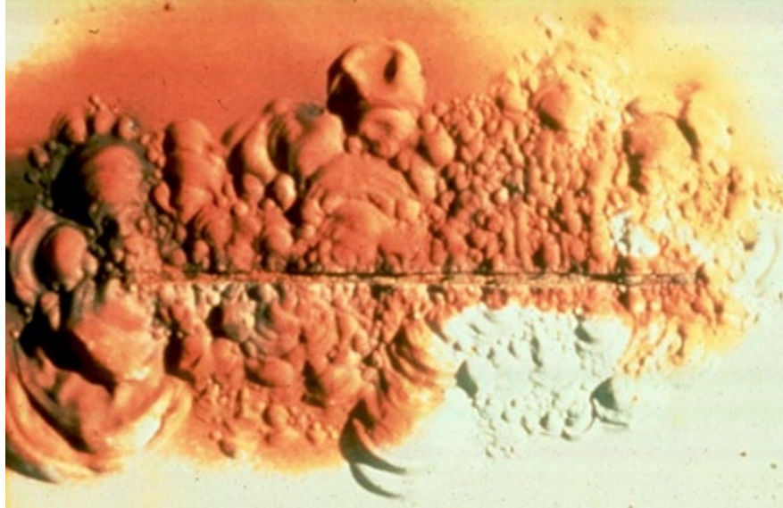
Figure 7.2.16 Rust Undercutting at Scratched Area
