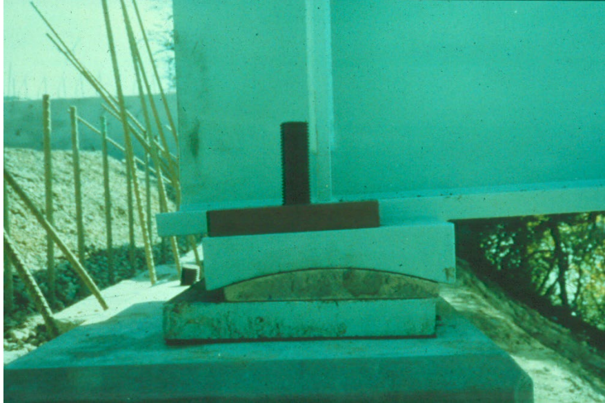
Figure 13.3.2 Bronze Sliding Plate Bearing
