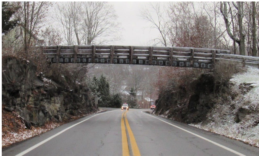
Figure 11.2.22 Glulam Stress-Laminated Timber Slab Bridge
