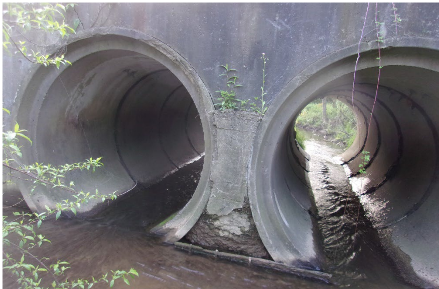
Figure 15.2.7 Twin Concrete Pipe Culvert
