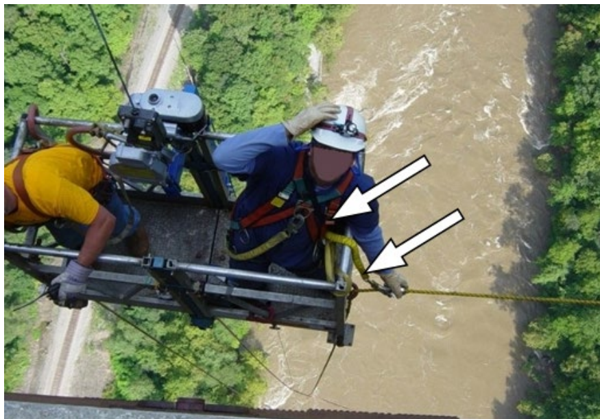
Figure 2.2.7 Inspector with Safety Harness with a Lanyard
