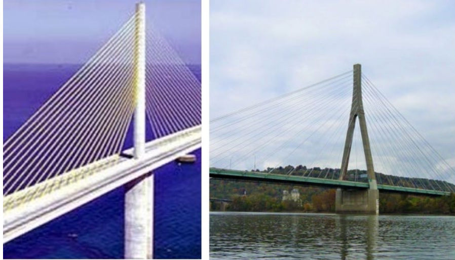
Figure 5.2.37 Single Column Tower and A-Frame Tower
