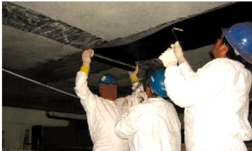
Figure 7.6.1 Concrete Beam Repaired Using FRP
