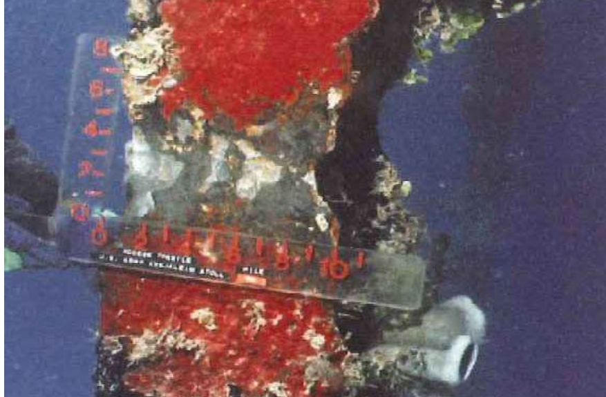
Figure 16.2.3 Level II Cleaning of a Steel Pile
