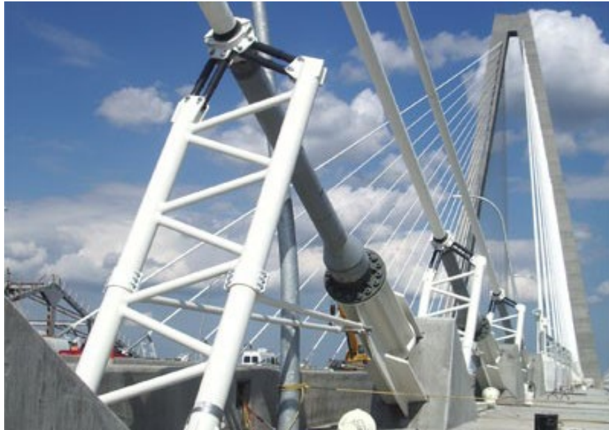
Figure 12.2.14 Shock Absorber Damper System
