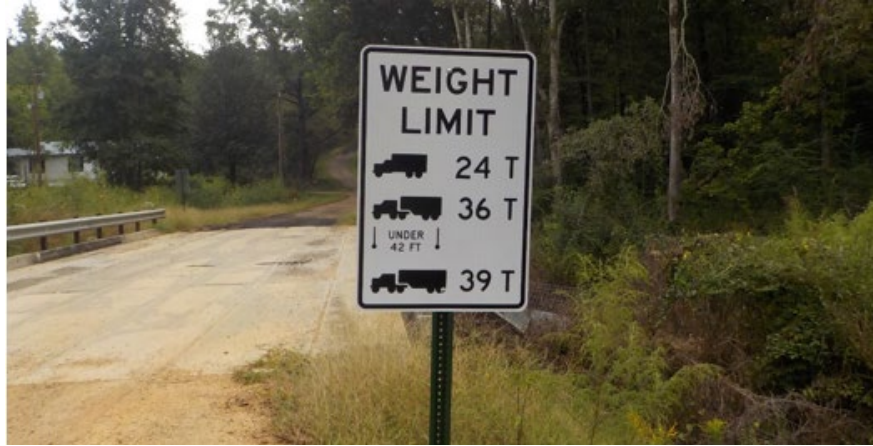
Figure 6.2.22 Bridge Weight Limit Posting
