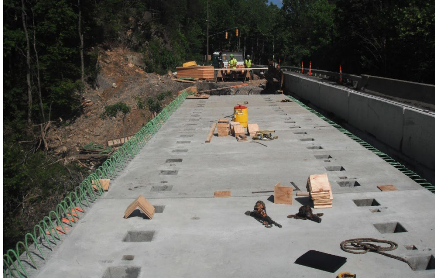
Figure 8.1.2 Block-Out Holes in Precast Panels
