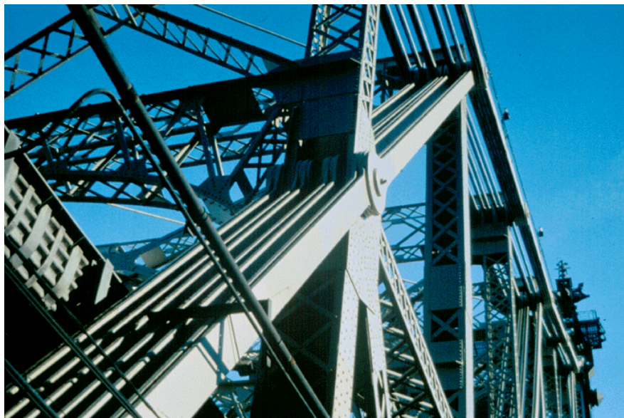
Figure 10.1.98 Eyebar Cantilevered Truss Bridge
