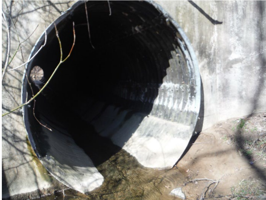
Figure 4.2.4 Circular Culvert Structure
