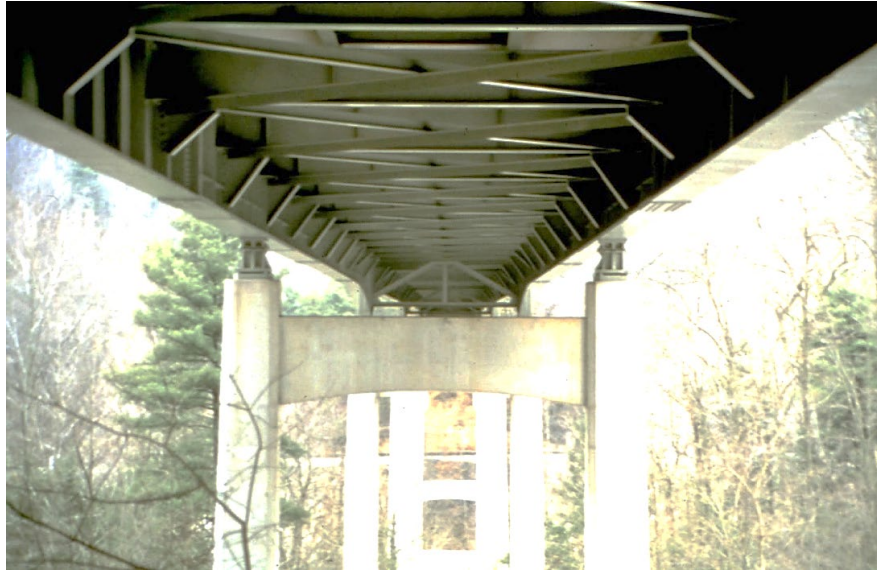
Figure 7.3.8 Nonredundant Two Girder Bridge
