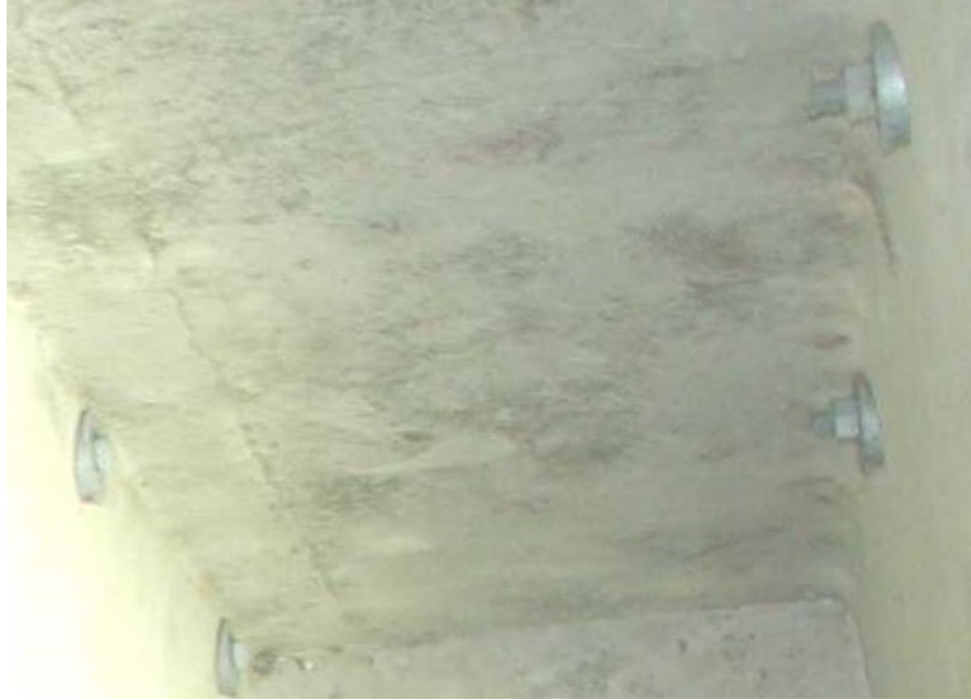
Figure 9.4.36 Stem Tie Bolts
