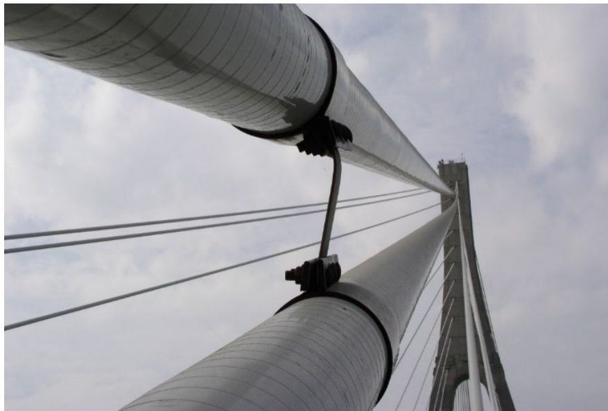
Figure 12.2.16 Cable Tie Type Damper System
