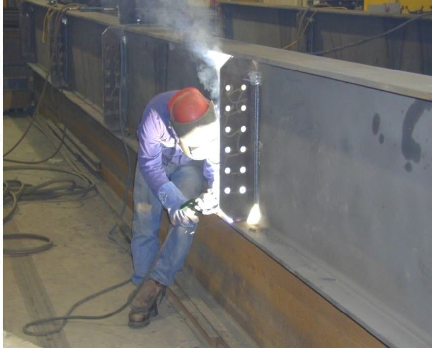
Figure 7.2.2 Steel Plate Welded to Girder
