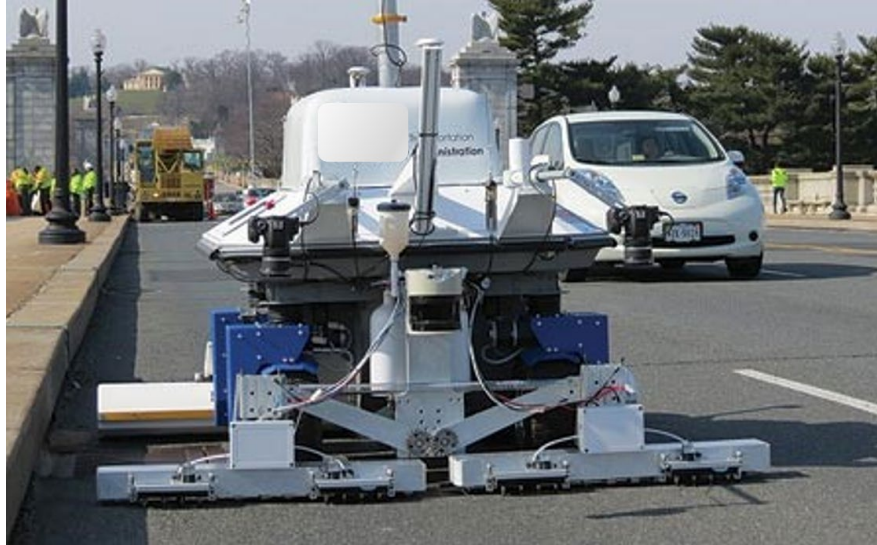
Figure 17.6.2 Robotics Assisted Bridge Inspection Tool (RABIT™)
