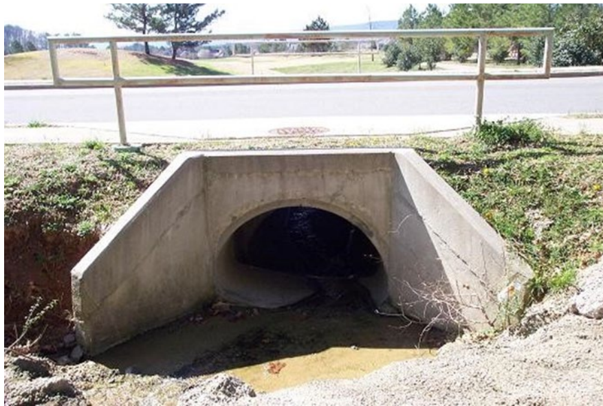
Figure 4.2.17 Culvert Head Wall and Wingwalls
