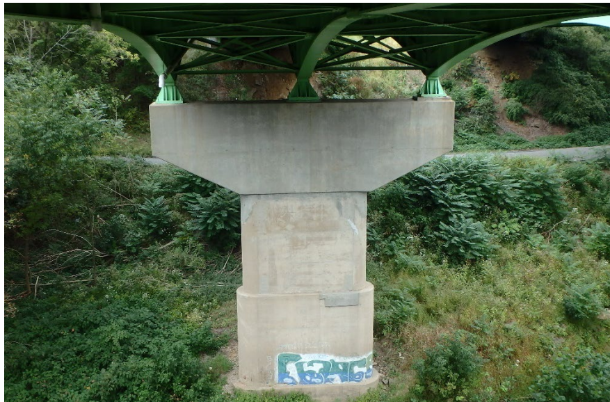
Figure 14.2.46 Hammerhead Pier
