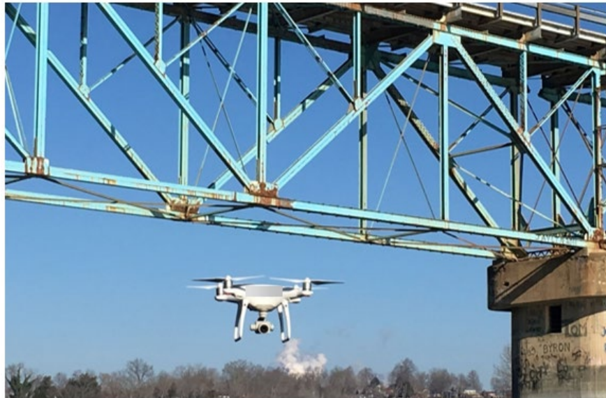
Figure 17.6.4 Drone Used for Bridge Inspection
