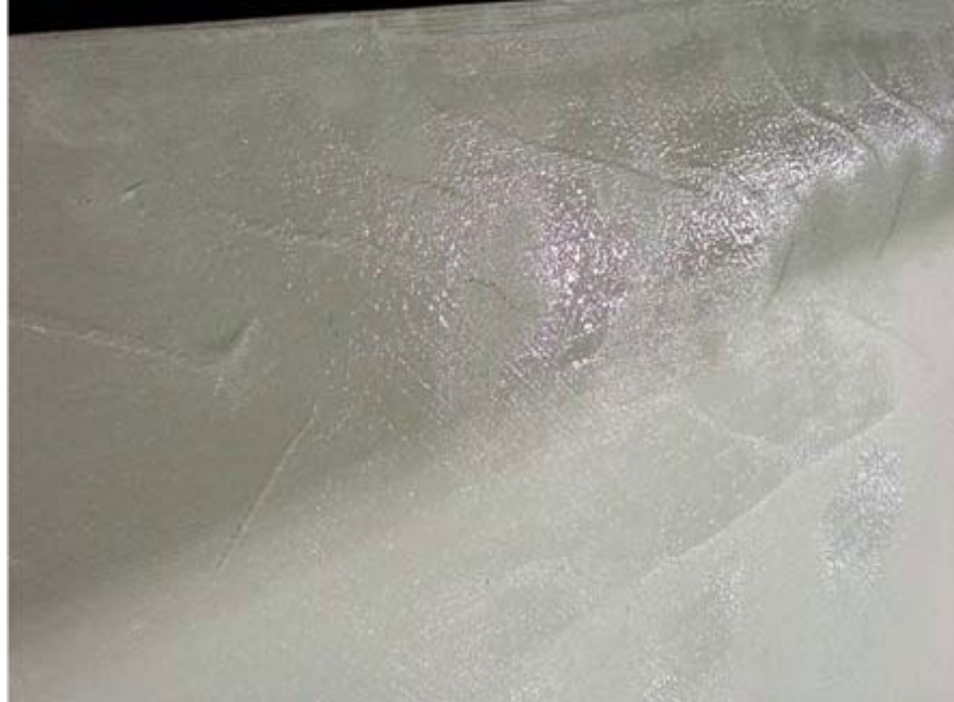
Figure 7.6.14 Wrinkling of FRP Fabric
