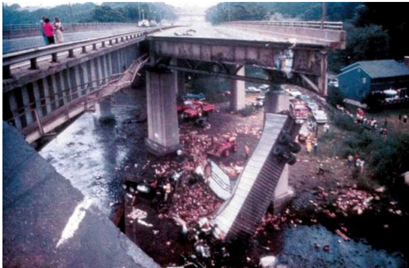
Figure 1.1.2 Mianus Bridge Failure
