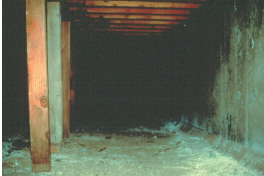
Figure 9.4.52 Interior Formwork Left in Place
