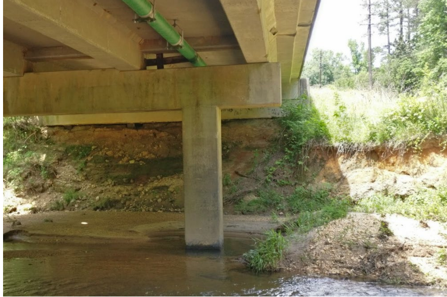
Figure 16.1.19 Sloughing Streambank
