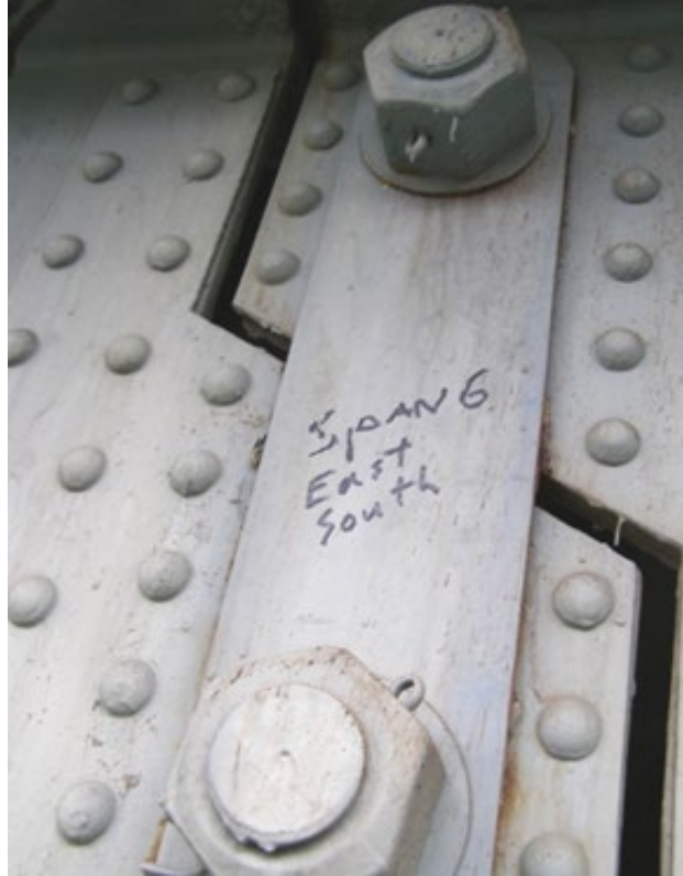
Figure 10.1.75 Pin-and-Hanger Assembly
