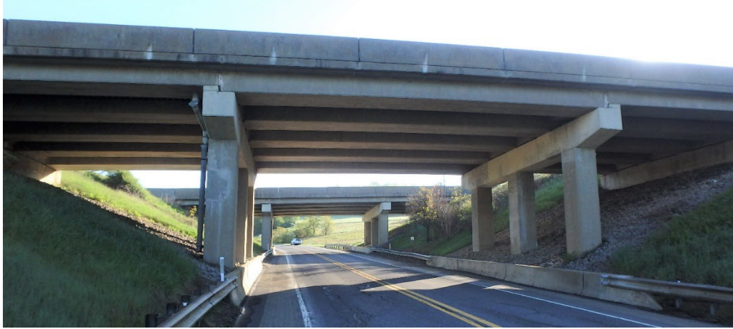
Figure 9.1.34 Typical Box Beam Bridge
