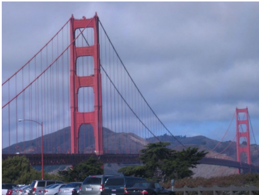
Figure 4.1.14 Cable-Supported Bridge: Suspension Cables and Hangers
