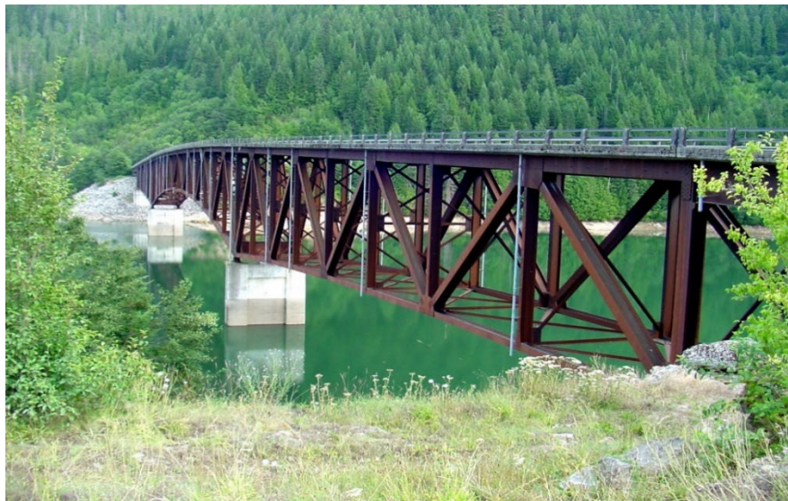
Figure 10.1.29 Deck Truss
