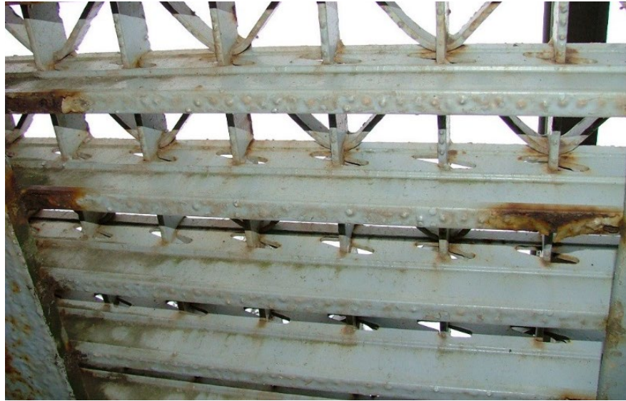
Figure 8.2.6 Steel Grid Deck with Slotted Holes to Eliminate Welding and Riveting
