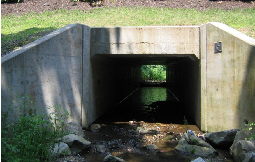
Figure 15.2.2 Concrete Box Culvert
