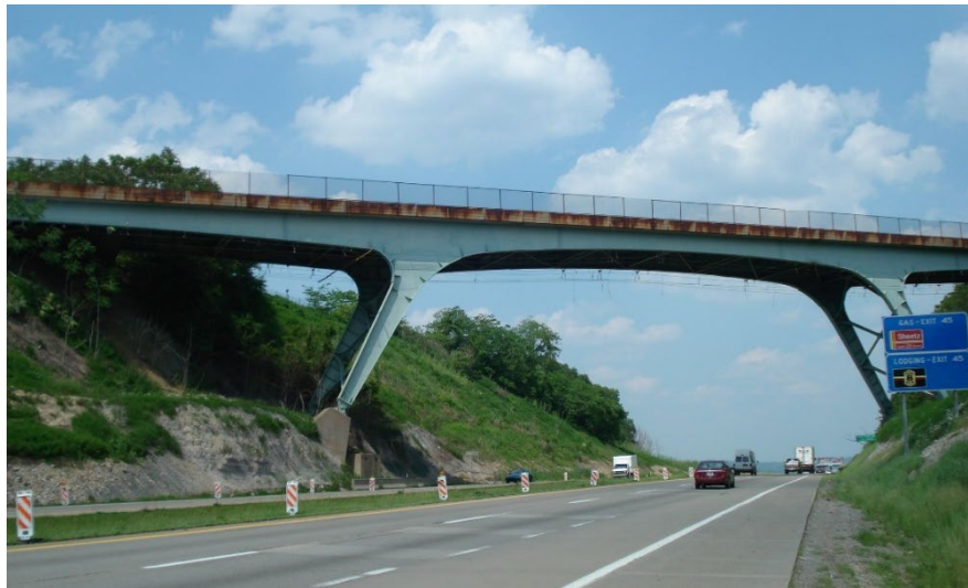
Figure 10.1.64 Rigid K-frame Bridge Constructed of Two Frames
