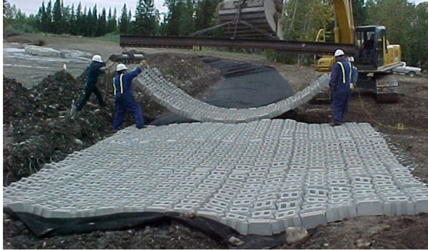
Figure 4.3.14 Concrete Revetment Mat
