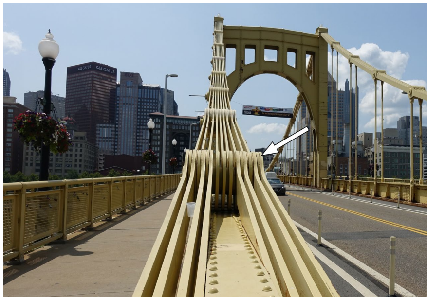
Figure 10.1.109 Tightly Packed Eyebar Connection
