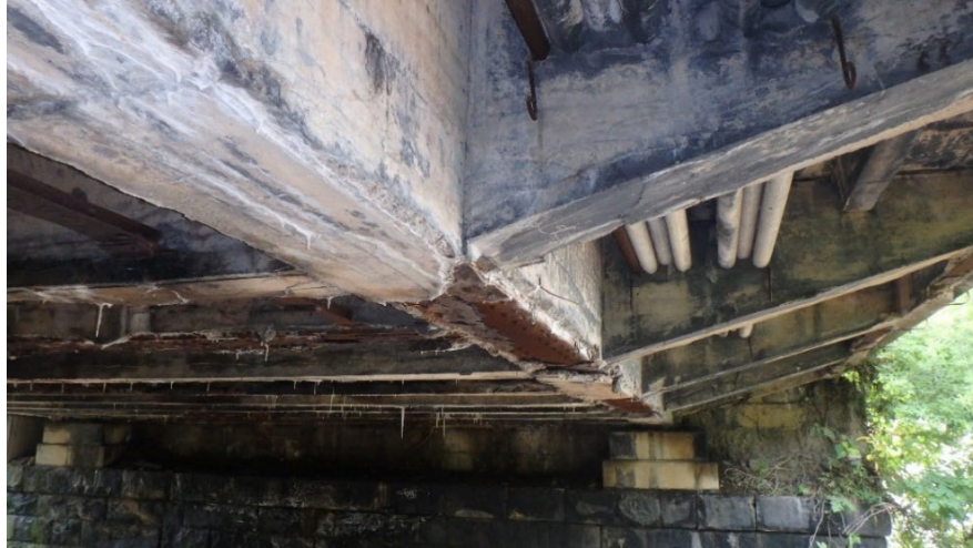
Figure 9.1.8 Concrete Encased Steel I-beam
