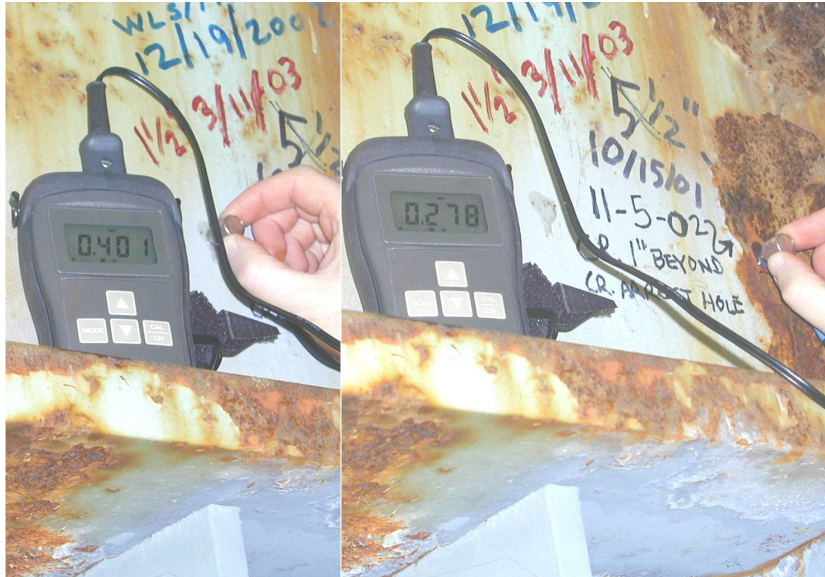
Figure 17.3.14 Ultrasonic Thickness Depth Meter (D-meter)
