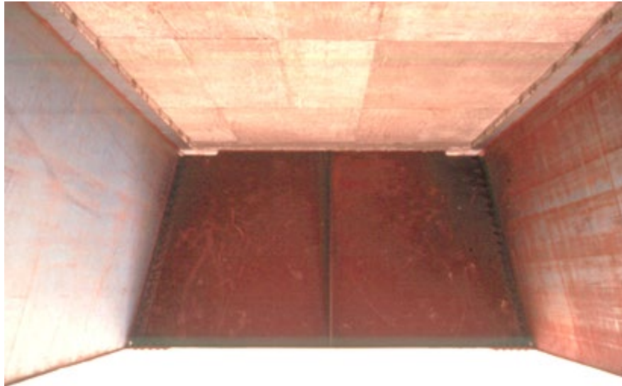
Figure 10.1.18 External Diaphragm between Spread Steel Box Girders
