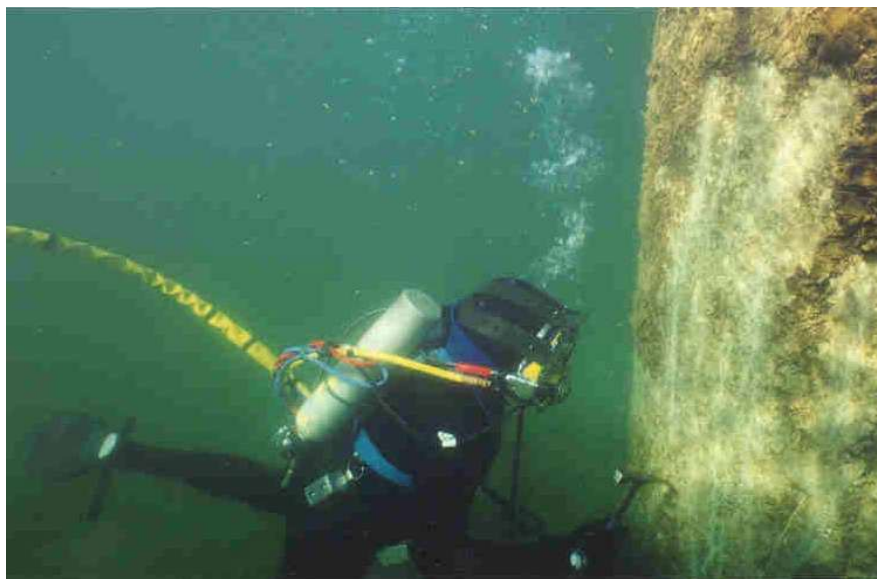
Figure 16.2.4 Diver Cleaning Pier Face for Inspection
