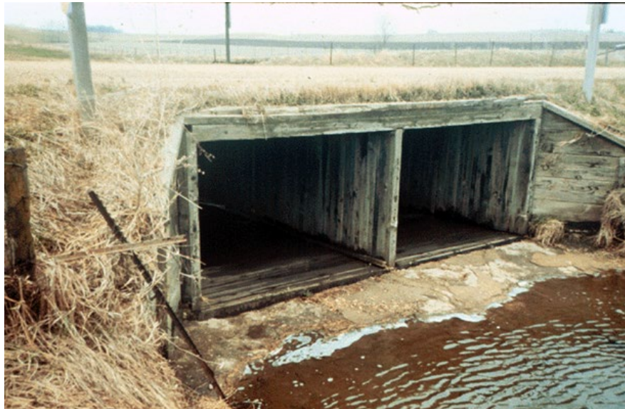
Figure 4.2.12 Timber Box Culvert
