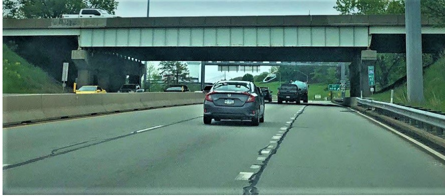
Figure 10.1.10 Combination Rolled Beams and Plate Girders
