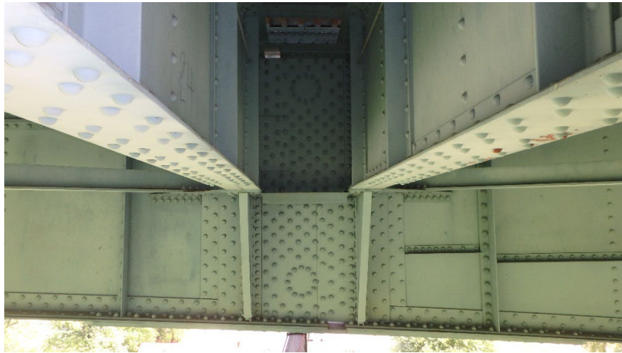
Figure 10.1.83 Pin and Hanger Replaced with Bolted Retrofit
