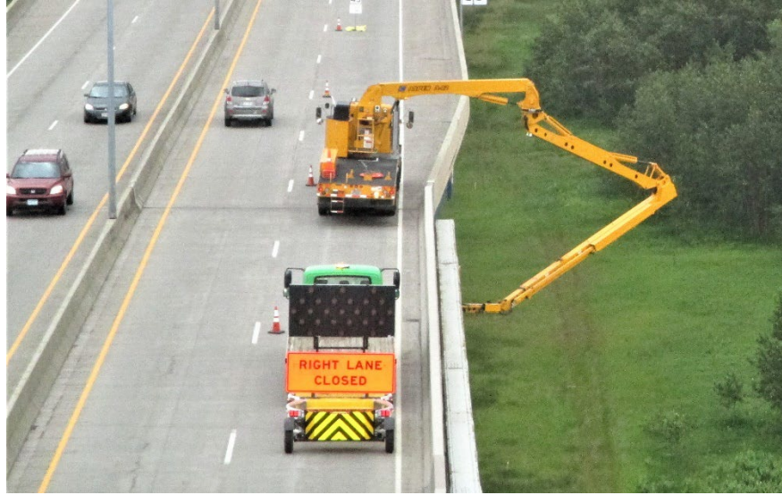
Figure 2.3.3 Inspection Vehicle with Traffic Control
