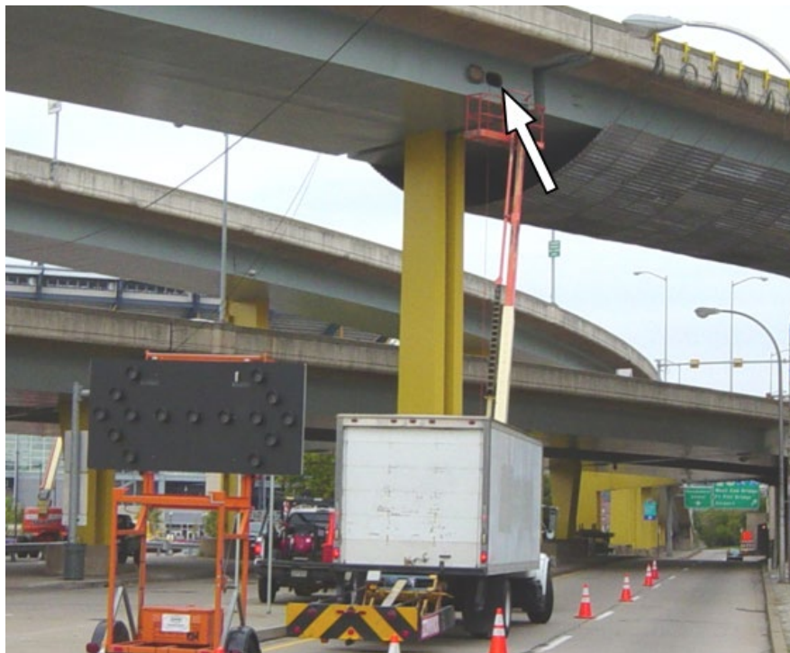
Figure 10.1.19 Inspection Access Door in a Box Girder
