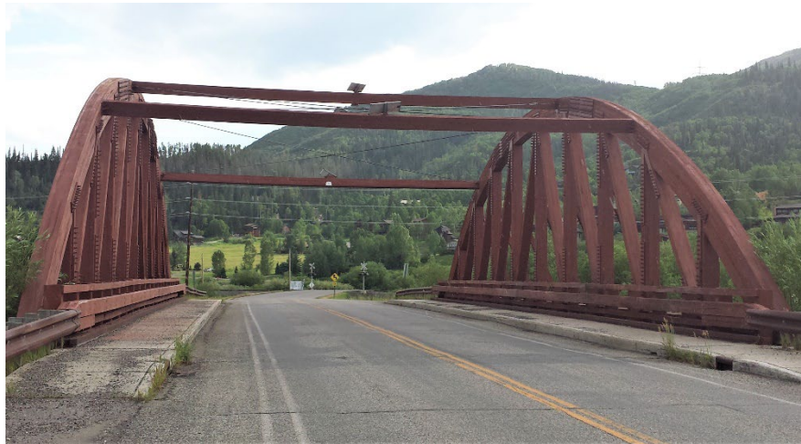
Figure 11.2.15 Long Span Timber Through Truss
