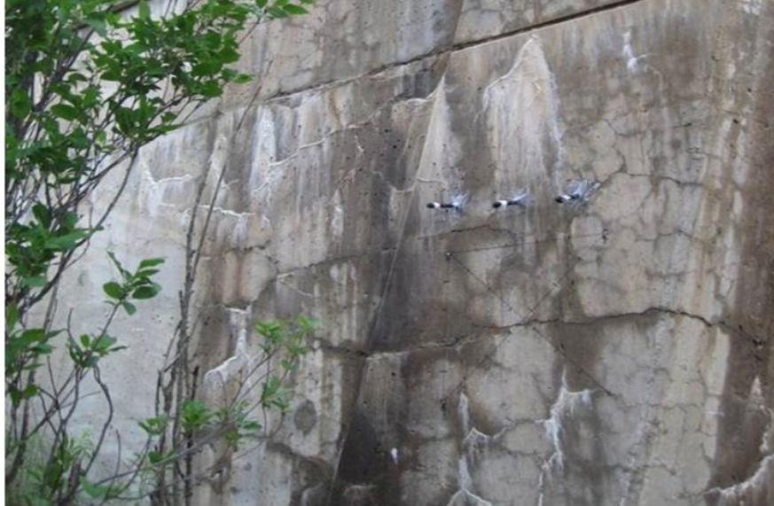
Figure 7.1.28 Alkali-Silica Reaction (ASR)
