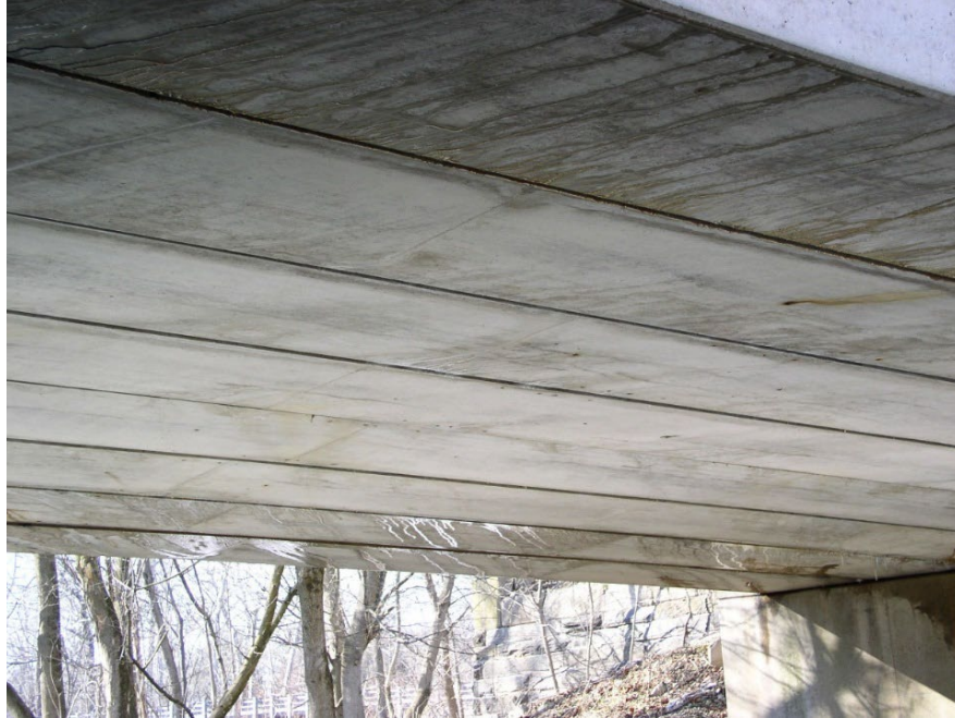
Figure 4.1.47 Adjacent Box Beam Bridge
