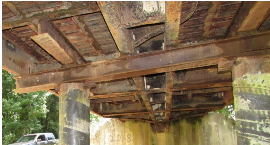
Figure 10.4.60 Flat Car Bearing Directly on Bent Cap
