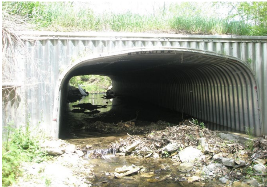
Figure 4.2.10 Large Structural Plate Box Frame Culvert
