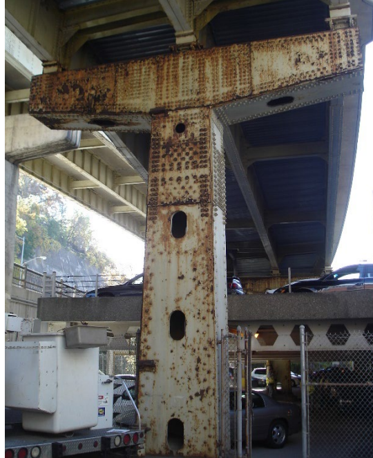
Figure 14.2.50 Hollow Steel Hammerhead Pier
