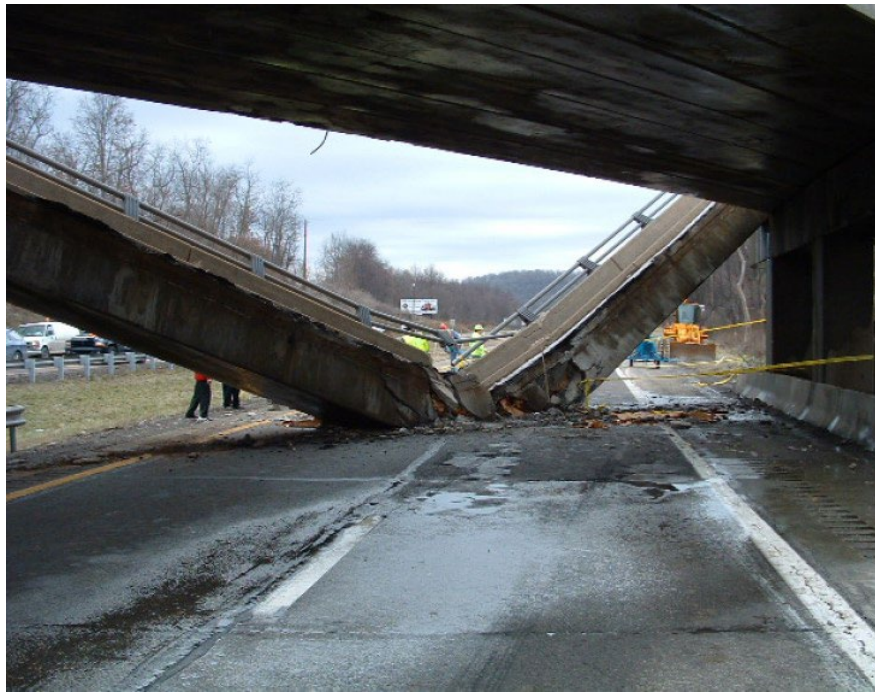
Figure 9.5.1 View Northeast of I-70 EB from Beneath Span 3
