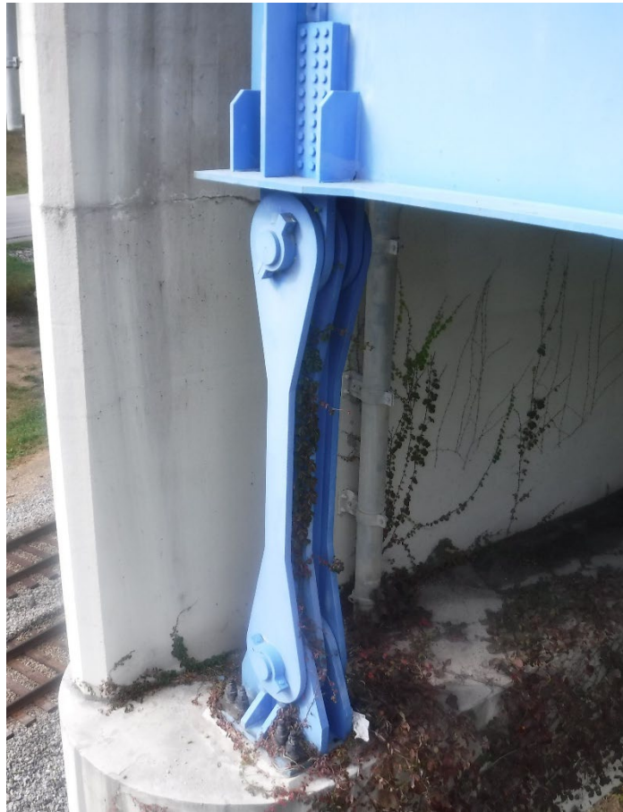
Figure 13.3.25 Pin and Link Bearing
