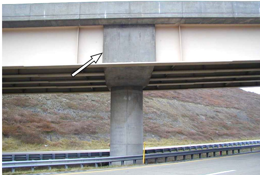
Figure 14.2.51 Integral Concrete Pier Cap
