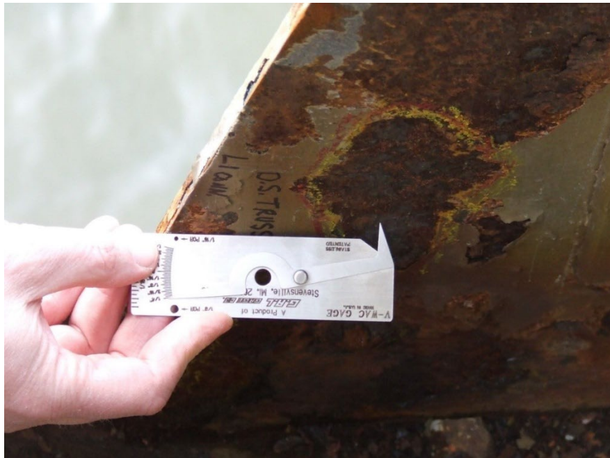
Figure 10.4.40 Using V-WAC in the Field to Measure Gusset Plate Section Loss
