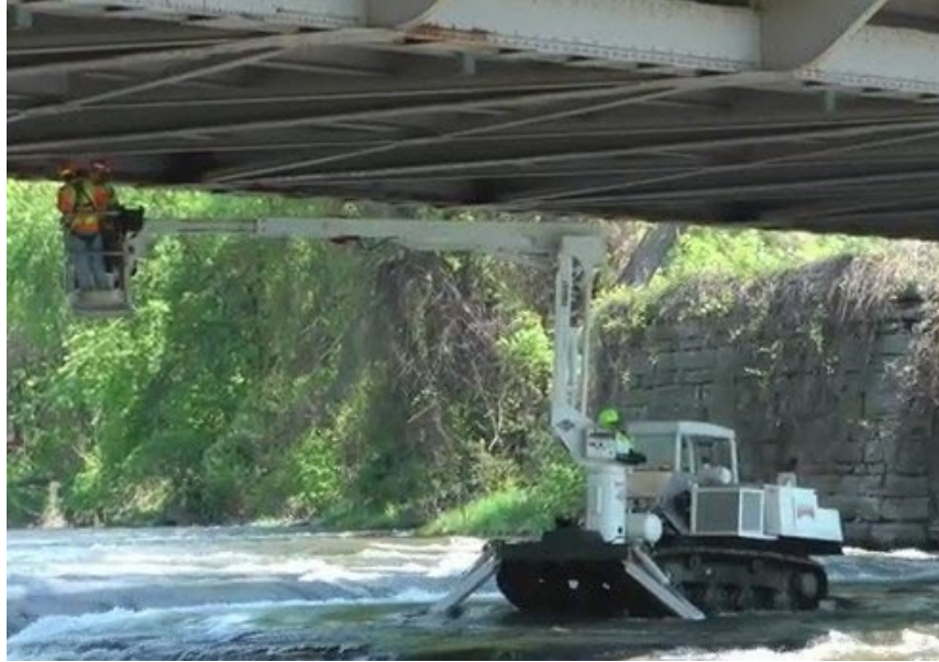
Figure 2.5.7 Track-mounted Lift in a Stream
