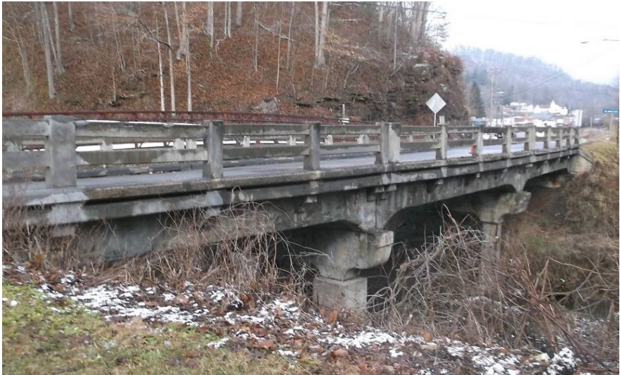
Figure 6.2.30 Integral Bridge
