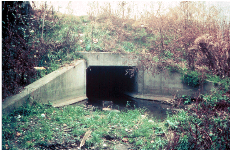
Figure 15.5.14 Culvert Wingwalls with Exposed Footings
