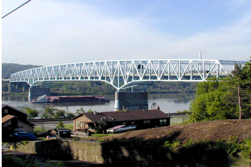
Figure 10.1.36 Continuous Through Truss
