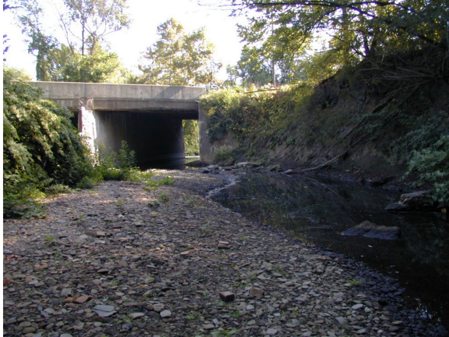
Figure 16.1.51 Misaligned Waterway
