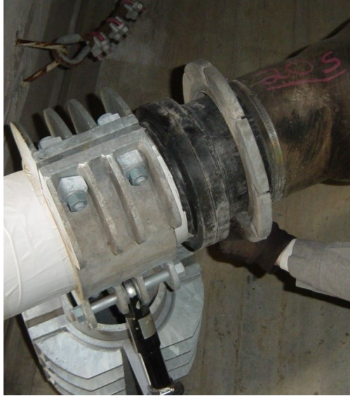
Figure 5.2.35 Damper for Cable-Stayed Bridge
