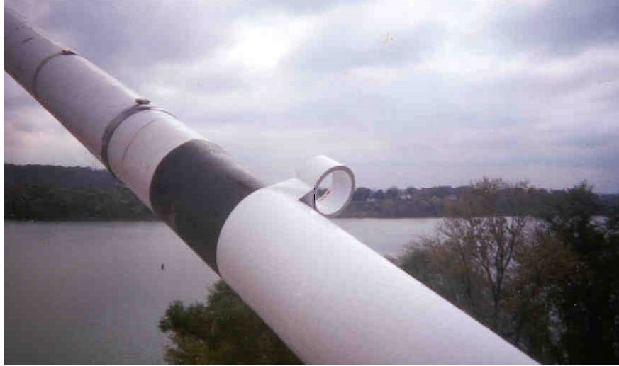
Figure 12.2.4 Cable-Wrapping Placement
