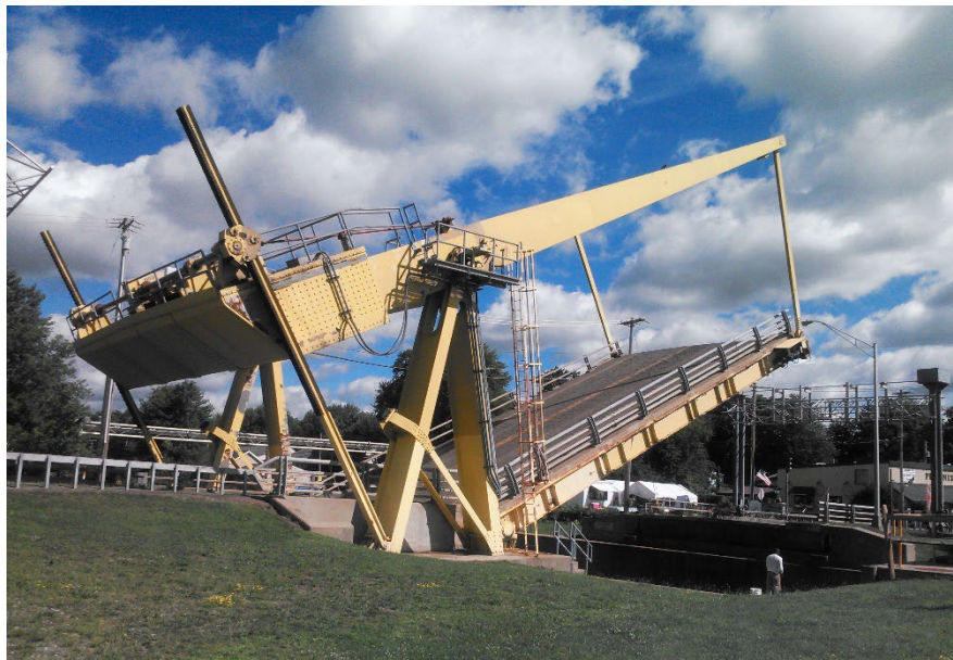
Figure 5.3.7 Single-Leaf Bascule Bridge in the Open Position
