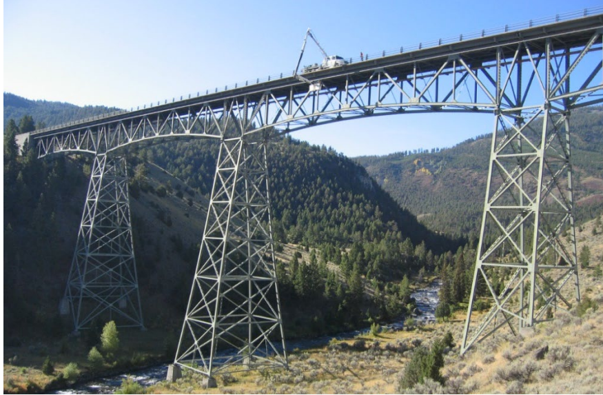
Figure 14.2.49 Steel Trestle or Tower
