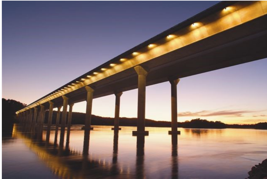
Figure 9.1.54 Precast Segmental Concrete Box Girder Bridge
