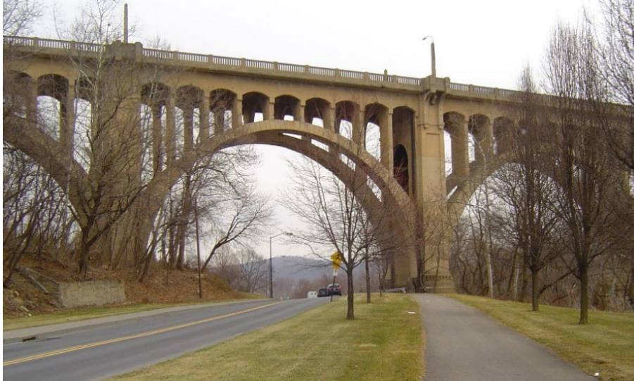
Figure 9.1.18 Open Spandrel Arch Bridge
