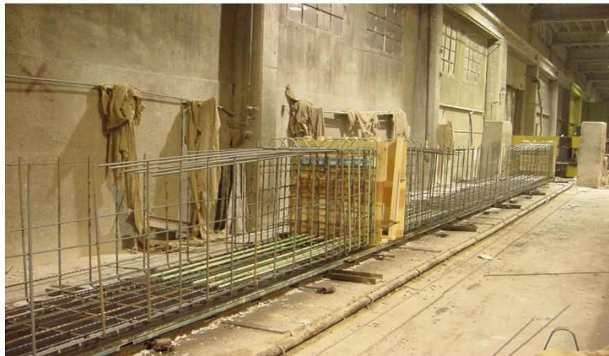
Figure 7.1.5 Fabrication of a Prestressed Concrete Beam
