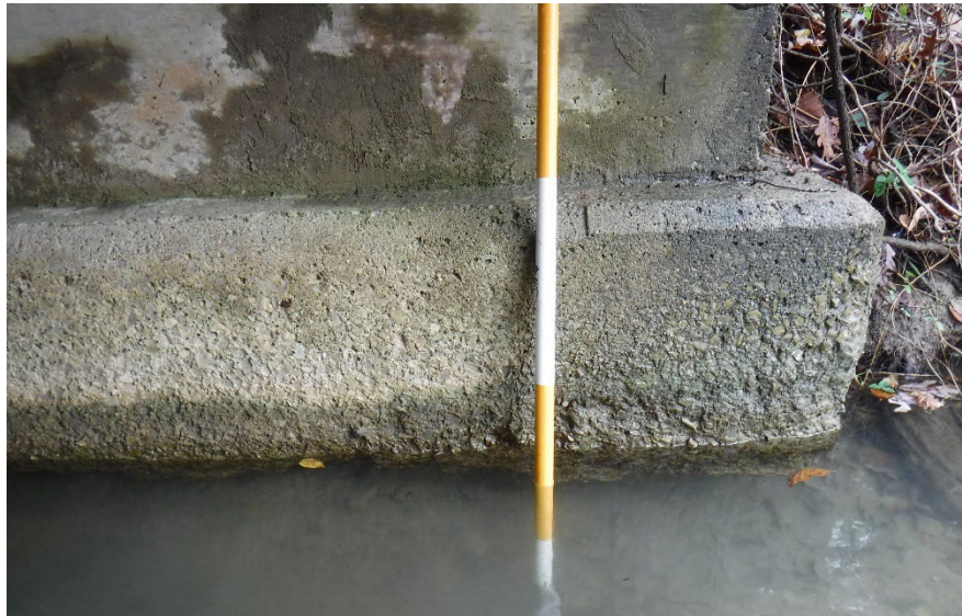
Figure 7.1.32 Substructure Abrasion
