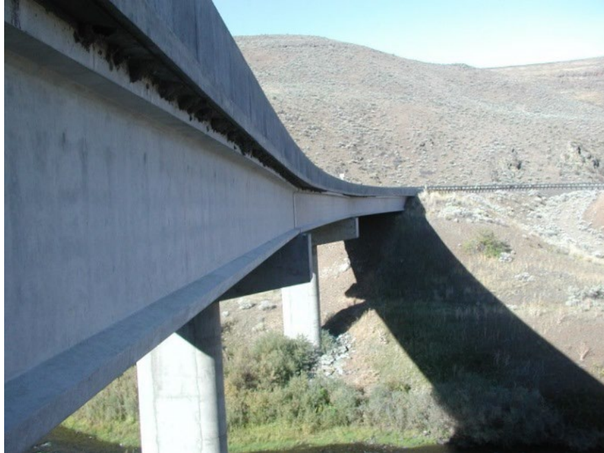
Figure 9.1.45 Prestressed I-beam Bridge
