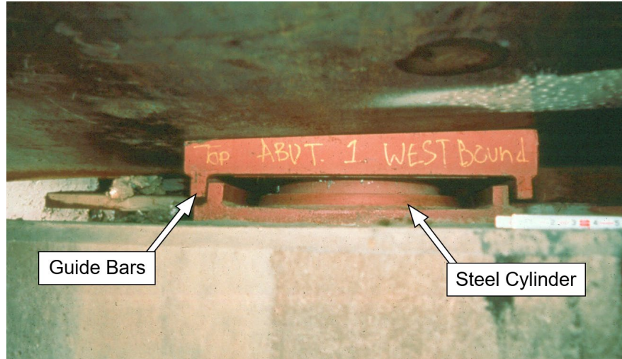
Figure 13.3.18 Neoprene Pot Bearing with Guide Bars
