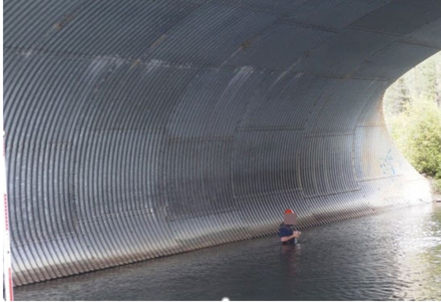
Figure 4.2.9 Large Structural Plate Pipe Arch Culvert
