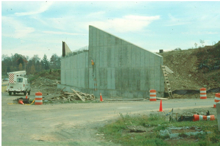
Figure 14.2.9 Reinforced Concrete Cantilever Abutment
