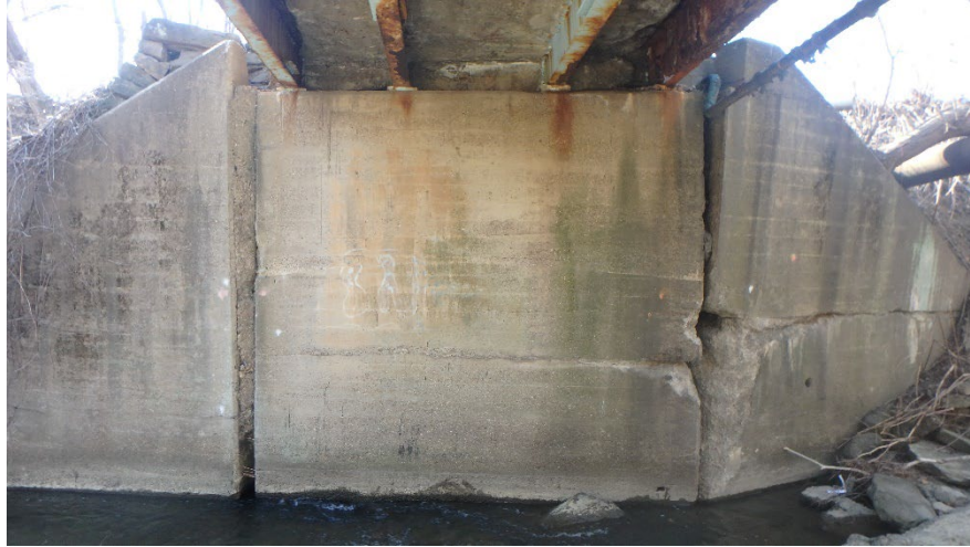
Figure 14.2.8 Plain Unreinforced Concrete Gravity Abutment
