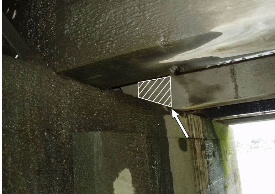
Figure 11.5.1 Bearing Area of Typical Solid Sawn Beam
