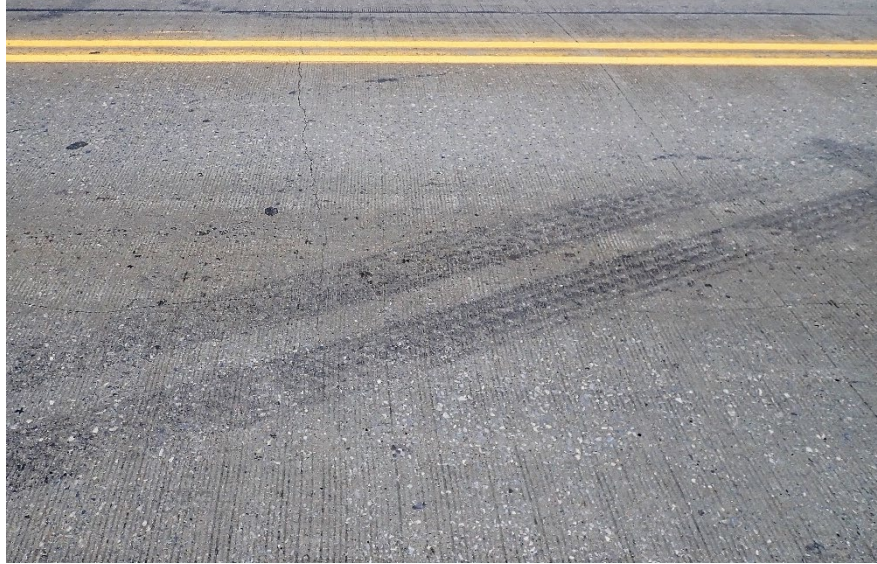
Figure 7.1.30 Wear in Wheel Paths
