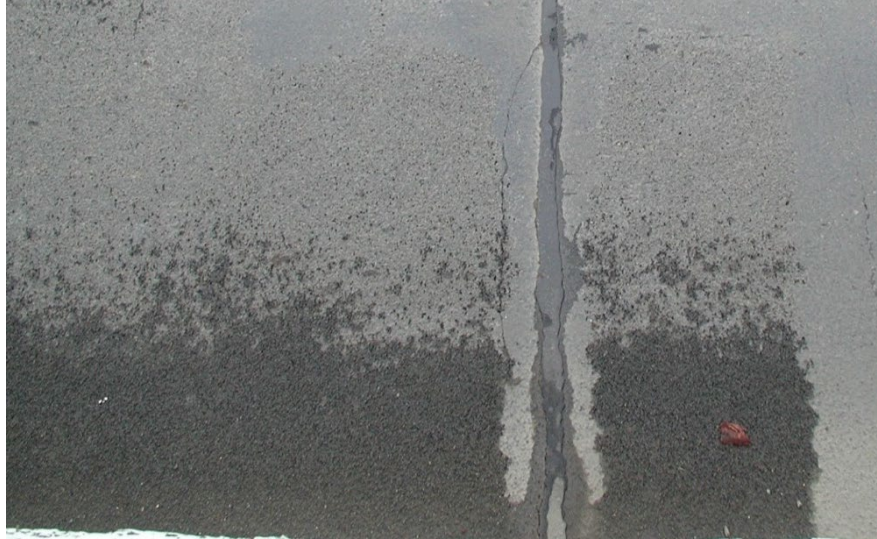
Figure 8.4.7 FRP Panel Splice
