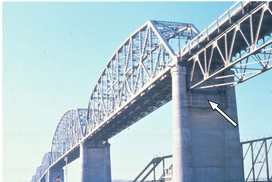
Figure 14.2.44 Column Pier with Web Wall
