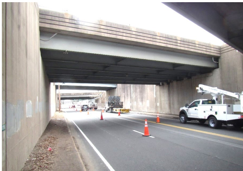
Figure 10.1.1 Simple Span Rolled Beam Bridge
