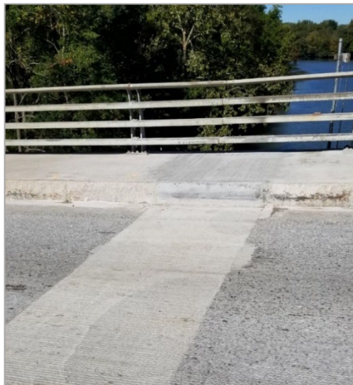
Figure 7. Photo. Link Slab, Rte. 51 over Erie Canal, CSX, Rte. 5 Ilion, NY.
