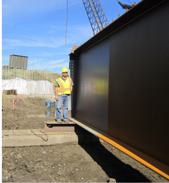
Figure 20. Iowa DOT photo of a weathering steel girder zone painted under the deck joint.
