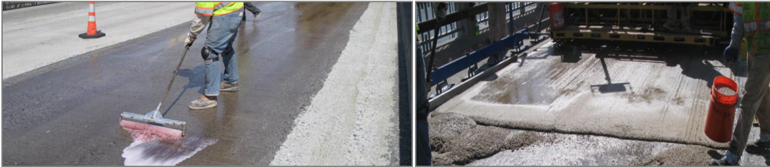
Figure 7. Photo of a milled deck receiving a high molecular weight methacrylate primer (left photo) and a PPC overlay being placed and finished (right photo).
