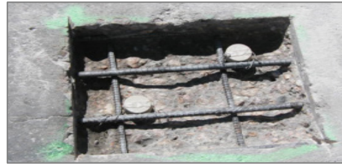
Source: Ohio DOT
