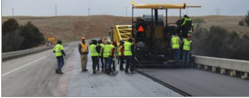
Figure 6. Photo of a concrete bridge deck showing membrane in place (middle lane) and overlay being placed on top (right lane).
