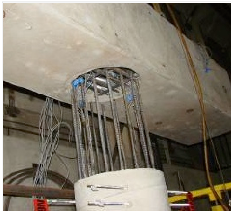
Figure 5.2.3.3-2. CMP Pipe Void Connection Installation (Source: NCHRP Project 12-74).
