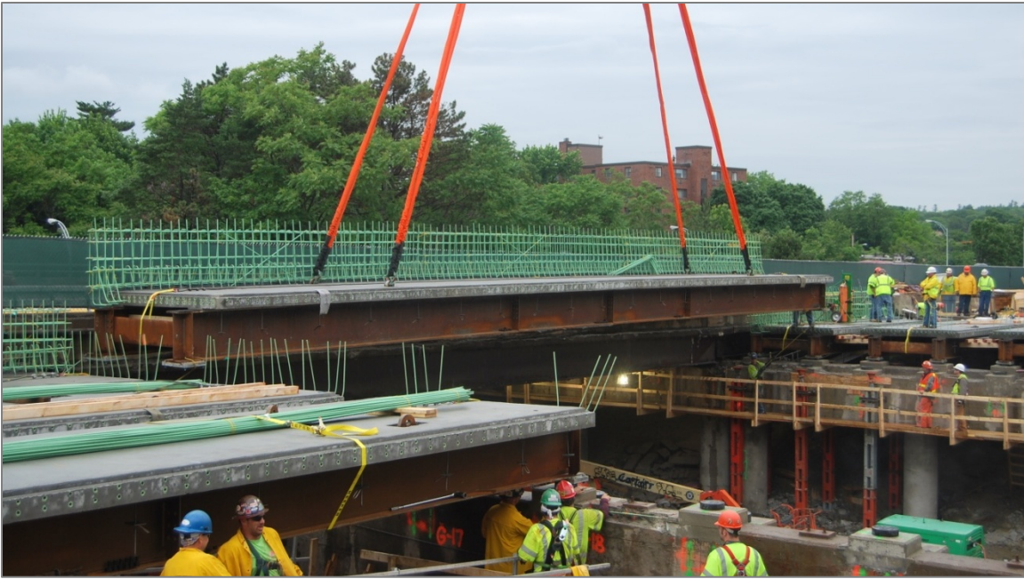
Figure 4.3-1. Massachusetts DOT 93 Fast 14 Construction using Modular Elements.
