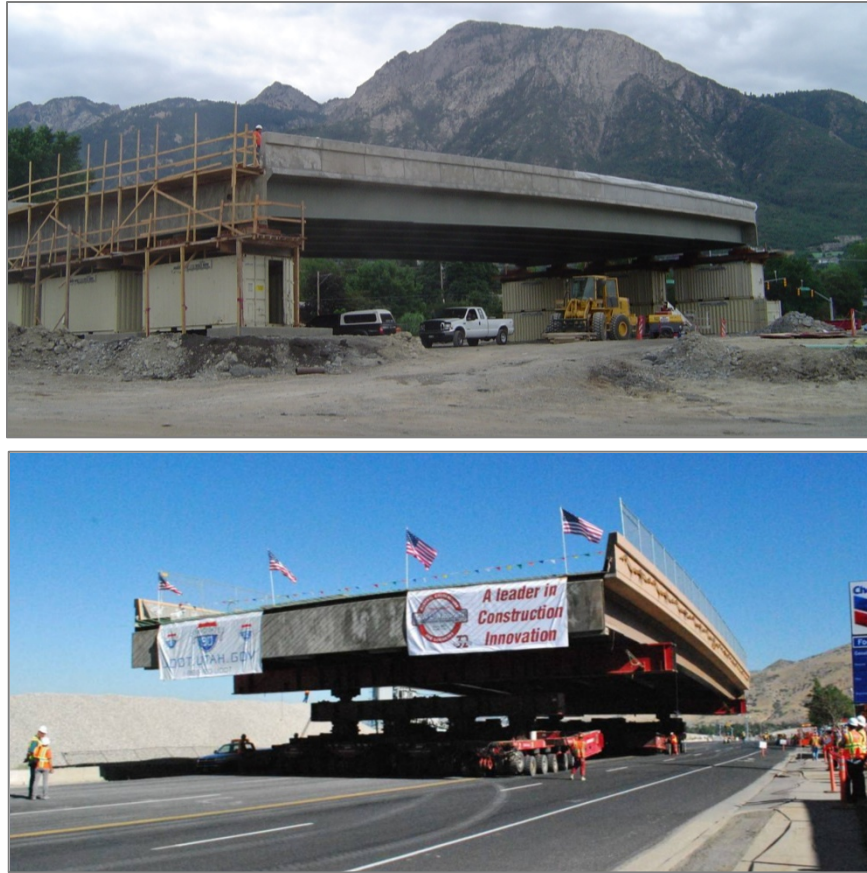
Figure 11.4.4-1. Construction and Installation of a Bridge System
