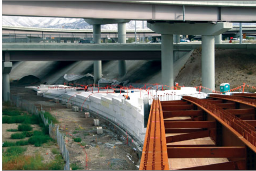
Figure 5.1.8.3-2. EPS Geofoam Embankment (Source: ACH Foam Technologies).
