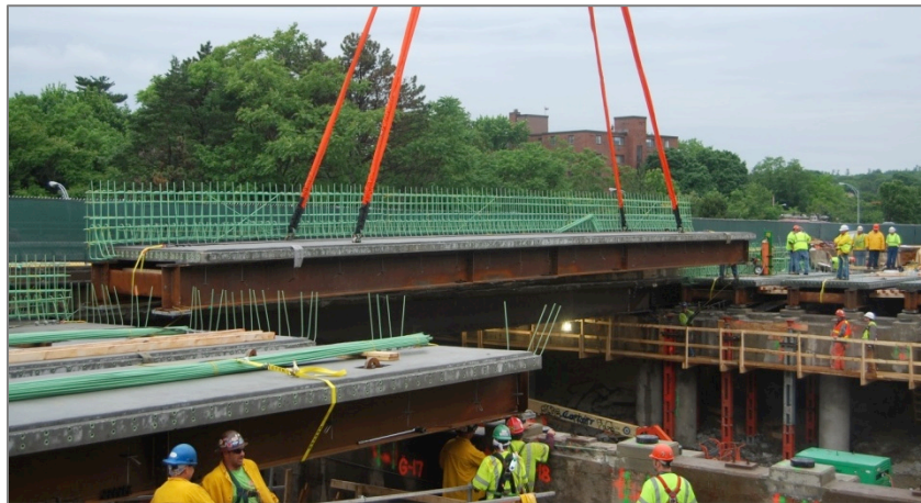
Figure 2.2.1-1. Modular Steel Deck/Beam Element Construction.
