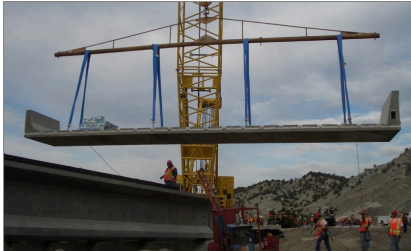
Figure 8.1.4.2-1. Integral Barrier on Full Depth Deck Panel (Source: Utah DOT).
