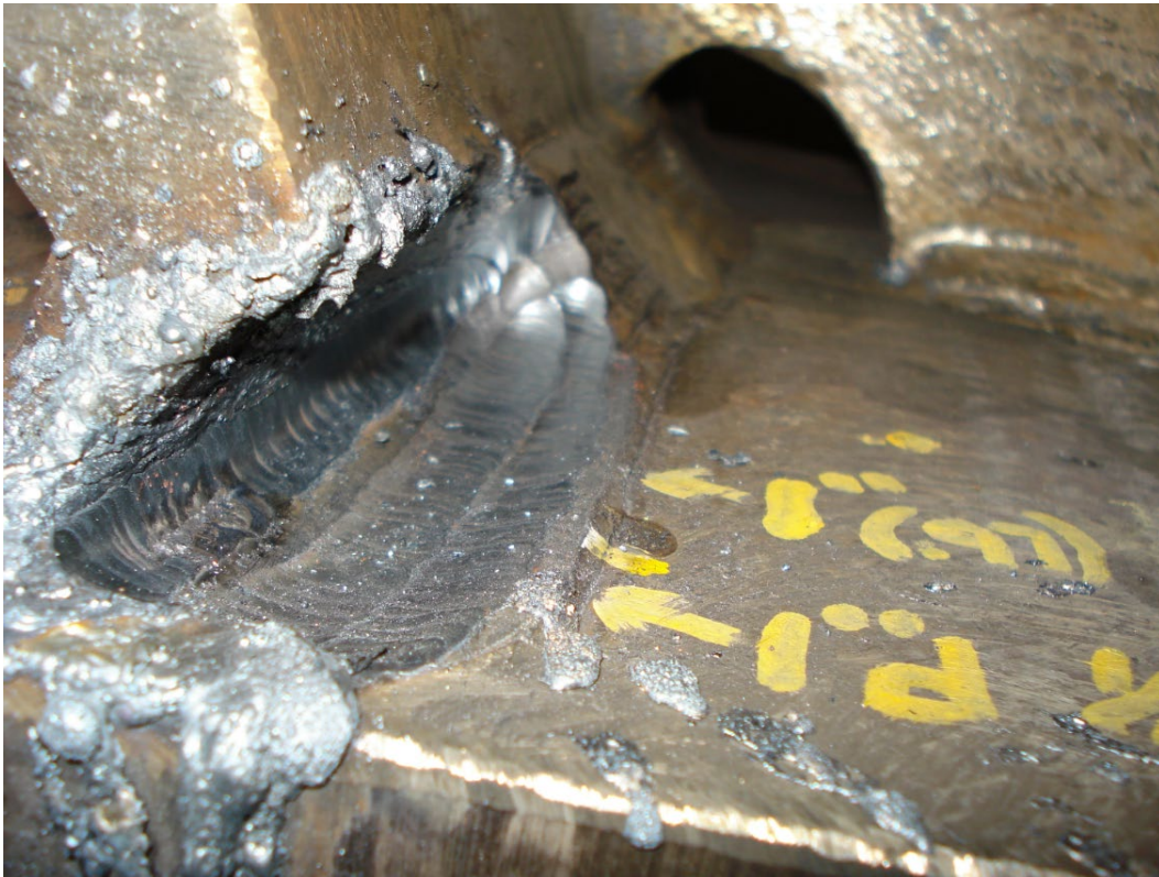
Figure 46. Photo. Example of partially gouged joint.
