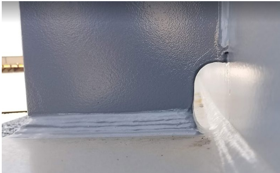
Figure 139. Photo. Beads in a CJP weld T-joint terminated in access hole.
