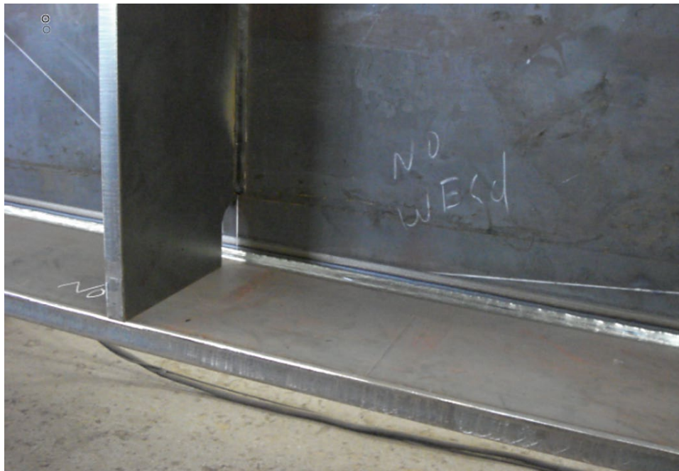
Figure 176. Photo. Stiffener not welded, full depth.
