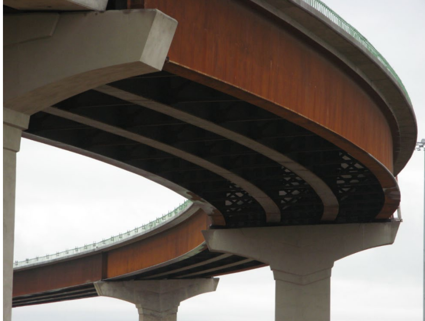
Figure 196. Photo. Use of field welding provides a pleasing uniform finish free of bolted splices (courtesy of John Holt).
