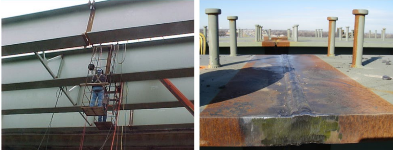
Figure 194. Photos. Bridge girder welded field splices in progress. Girder elevation (left, courtesy of Lewis Gamboa, LJA Engineering) and flange splice (right, courtesy of John Holt).
