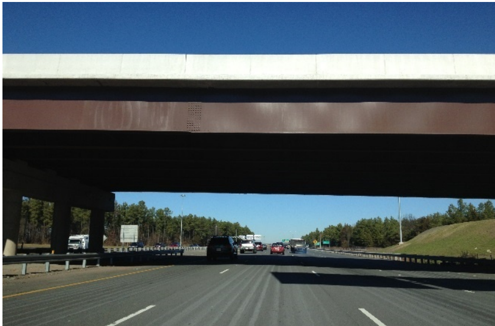
Figure 85. Photo. Warped (out-of-flat) girder webs.
