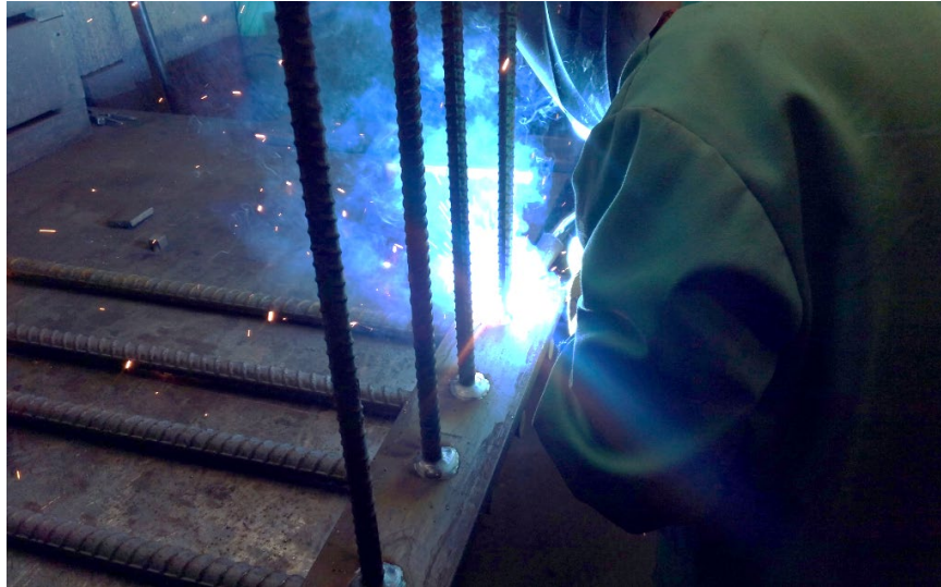
Figure 190. Photo. Welding reinforcing steel to structural plate.
