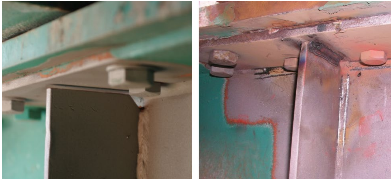
Figure 201. Photos. I-80 bridge field weld retrofit, before and after welding (courtesy Illinois Department of Transportation).
