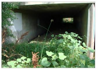
*Figure 3-15: Large culvert following major storm event* Large culverts tend to collect sediment on the upstream end, limiting the ability to convey flows during major storm events.
