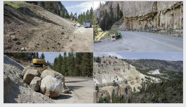
**Top left**: Topsoil is pushed to the top of slope for placement following construction. **Top right**: Vertical walls make construction challenging through this area. **Bottom left**: Large boulders are excavated and placed elsewhere in the project area. **Bottom right**: View from the corridor to the valley below
