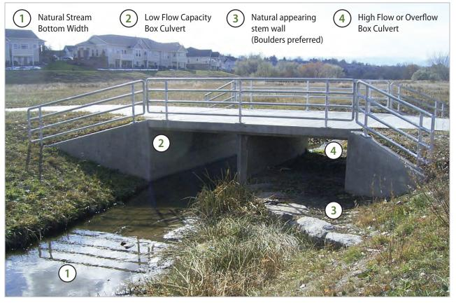
Figure 3-21: Multi-cell box culvert
