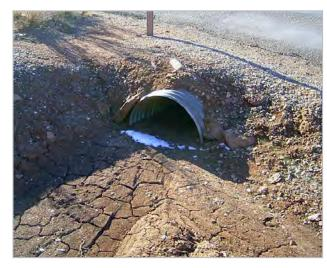
*Figure 4-2: Example of a culvert clogged by sediment* (Source: Parsons Brinckerhoff, Capitol Reef Route 10, Utah)
