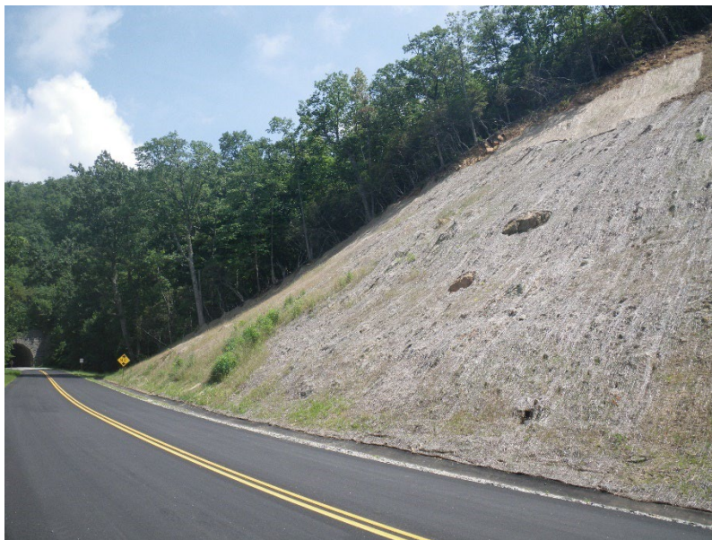
Figure 8-1: Example of slope stabilization mitigation measures. Anchors and slope face stabilization fabric with topsoil and seeds. Blue Ridge Parkway, Henderson County, NC.
