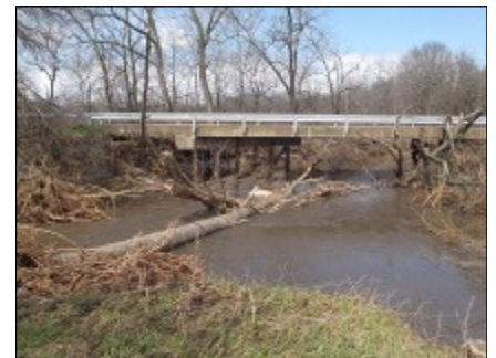
Upstream View of Bridge
