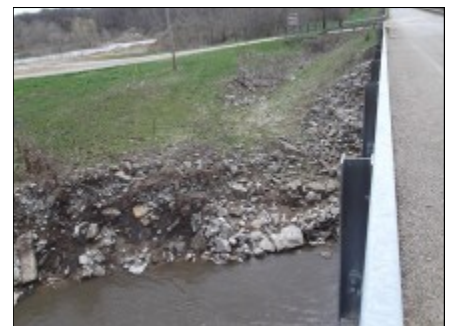
View of Upstream Face Outside Bend
