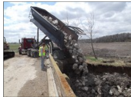
View of Riprap Being Dumped
