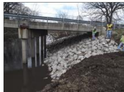
View of Riprap Armor at Abutment
