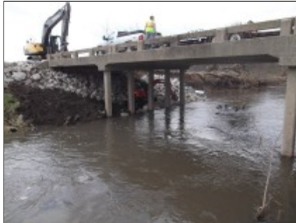
View of Riprap Placement on Abutment
