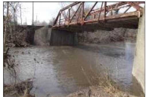
View of Township Road 82 Bridge looking at South
