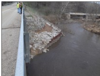
View of Upstream Abutment Cone
