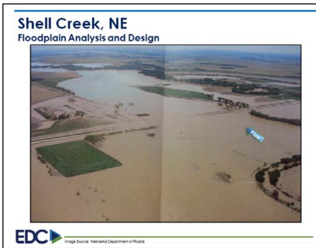
Figure 7: Roadway overtopped during a flood smaller than a 100-yr flood.
