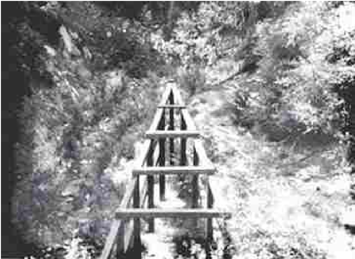
Figure 5.8. Timber pile debris deflector for boulders and large floating debris.
