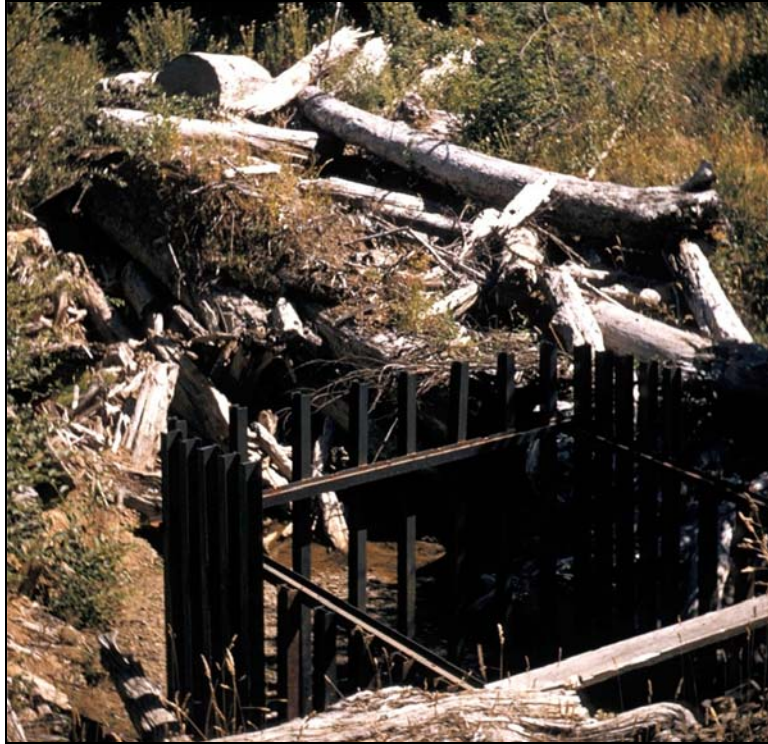
Figure 5.19. Steel rail debris rack. Note amount of debris accumulation in upstream channel.
