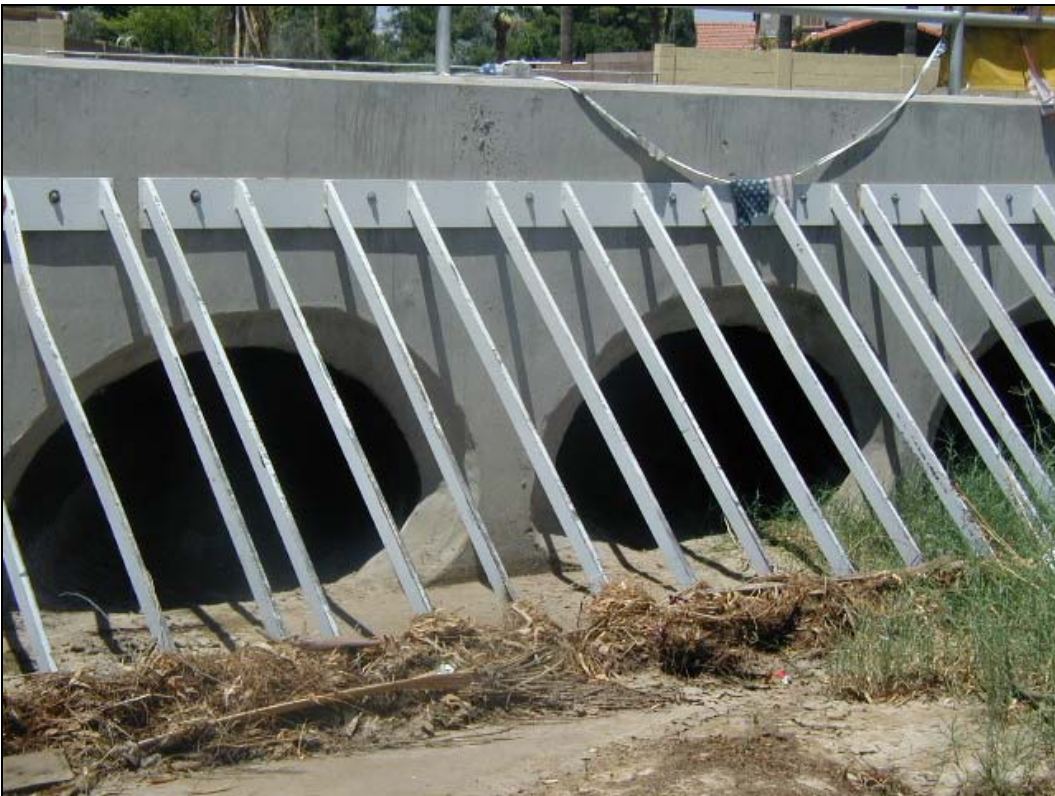
Figure 5.15. Steel debris rack in urban area.
