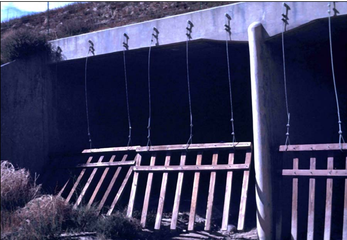
Figure 5.13. Timber debris rack (note how suspended by cables).
