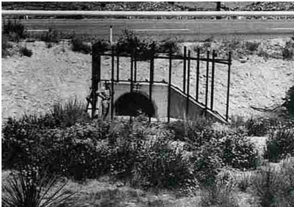
Figure 5.18. Installation in Figure 5.17 after several years of fine silt deposition at entrance.
