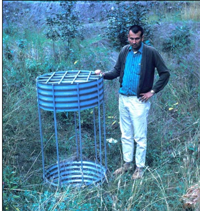
Figure 5.23. Metal pipe debris riser in basin (note anti-vortex device on top).
