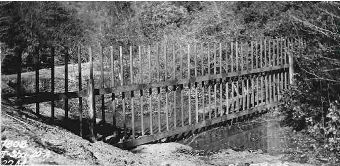
Figure 5.11. Post and rail debris rack, in place for 35 years, for light to medium floating debris installed 100 ft upstream of culvert.
