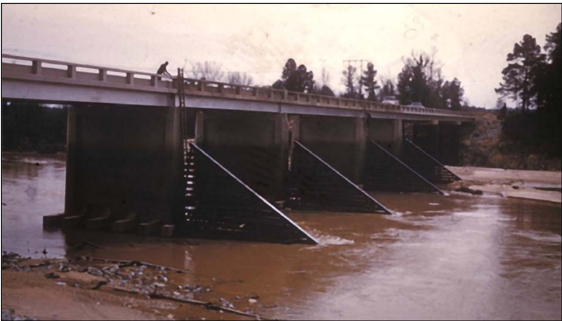
Figure 5.35. Timber debris fins with sloping leading edge.
