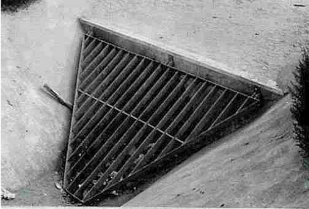
Figure 5.14. Hinged steel debris rack in urban area. Due to nature of debris and possible entry by children, bar spacing is close.
