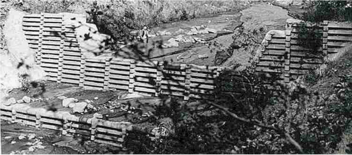
Figure 5.38. Debris dam of precast concrete sections fabricated to enable placement in interlocking fashion.
