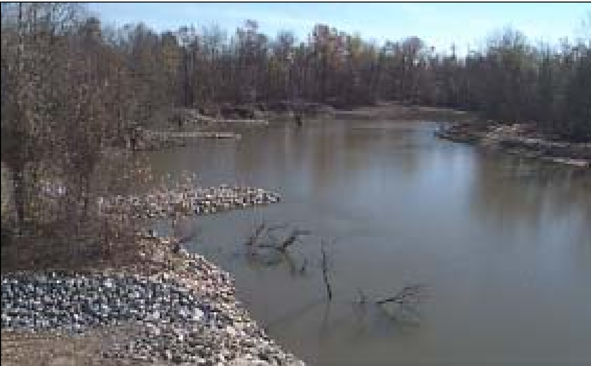
Figure 5.41. Bendway weirs on outer bank of Hatchie River looking upstream (TDOT).
