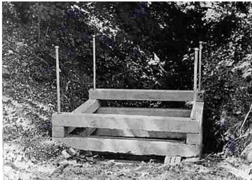
Figure 5.26. Debris crib of precast concrete sections and metal dowels. Height increased by extending dowels and adding more sections.
