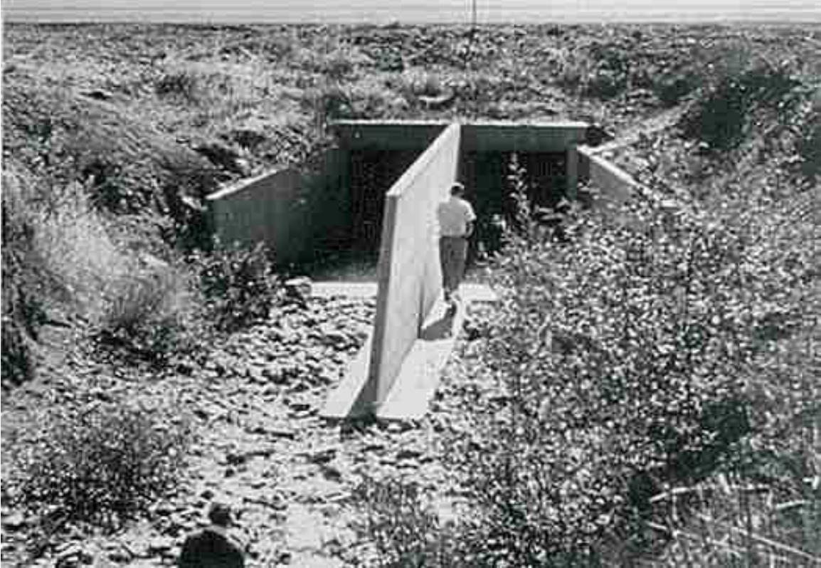
Figure 5.31. Concrete debris fin with rounded vertical leading edge as extension of culvert center wall.
