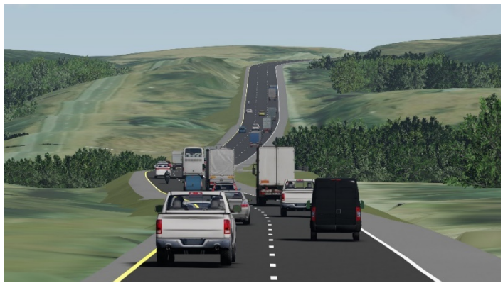
Figure 1: Rendering of the new Mineola Hill segment of I-70 featuring the new truck climbing lane. Image courtesy of Emery Sapp & Sons.
