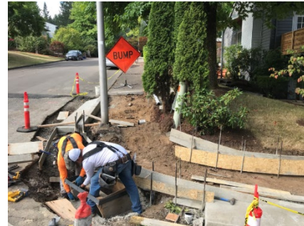
Figure 6: The City of Lake Oswego uses street maintenance fees to maintain its transportation infrastructure, including repairs to a curb ramp as shown above. Source: Lake Oswego Department of Public Works.
