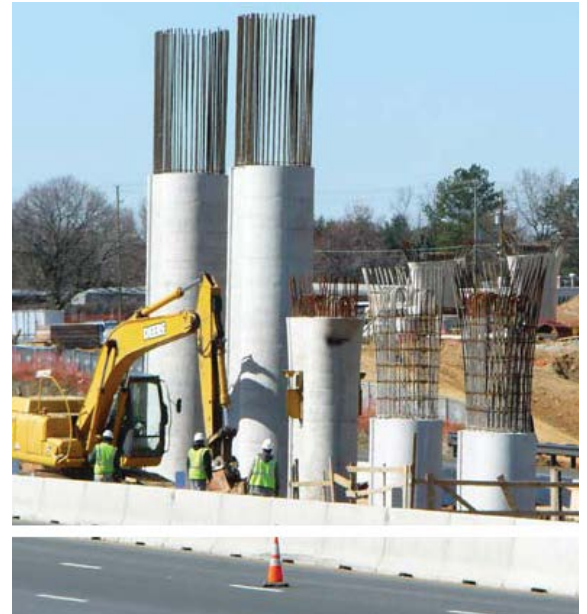
Maryland's Intercounty Connector uses GARVEE bonds.
