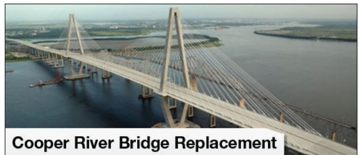
Cooper River Bridge Replacement The Cooper River Bridge replacement was financed by a loan from the South Carolina SIB.
