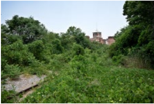
Before Atlanta BeltLine Construction
