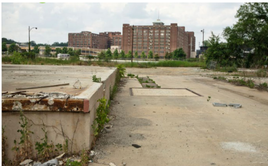
Before Atlanta BeltLine Construction
