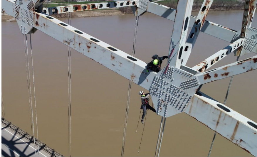
Figure 2.2.8 Inspection Involving Extensive Climbing
