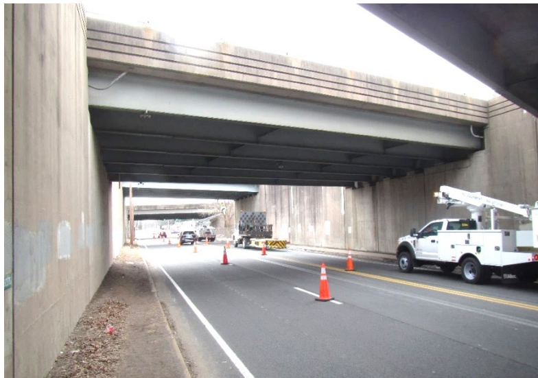
Figure 10.1.1 Simple Span Rolled Beam Bridge
