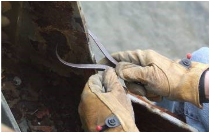
Figure 10.4.38 Using Calipers to Measure Gusset Plate Thickness
