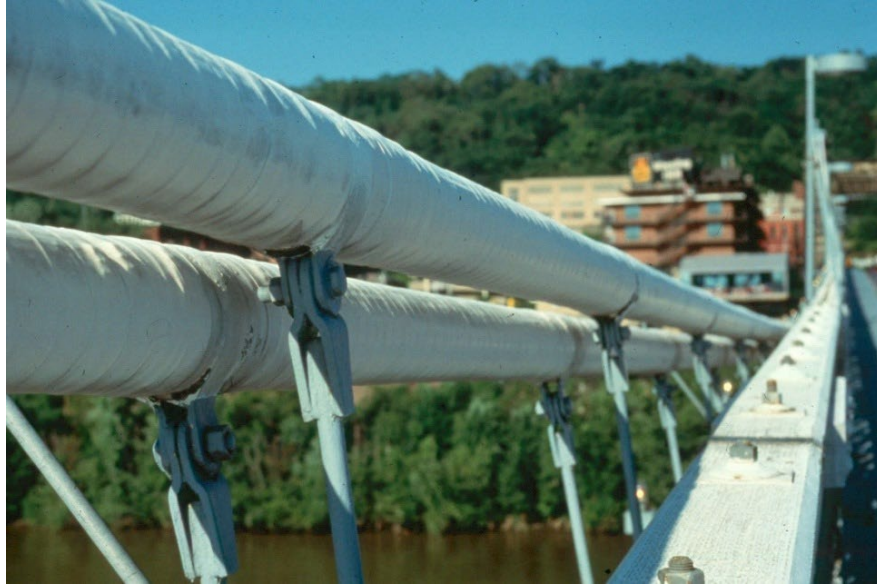
Figure 5.2.9 Cable Wrapping on Older Suspension Bridge
