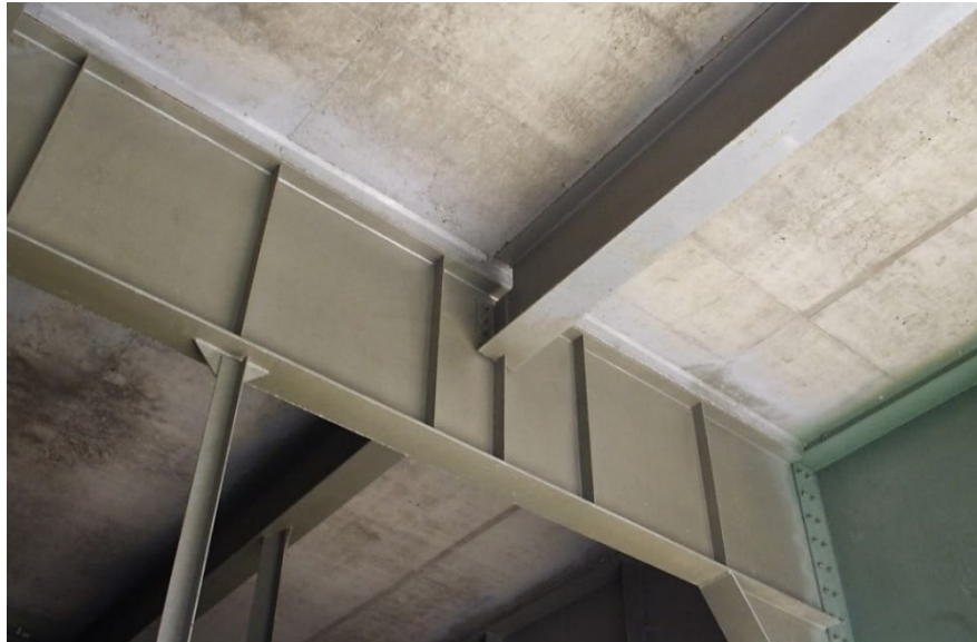
Figure 4.1.26 Underside View of a Bridge Deck
