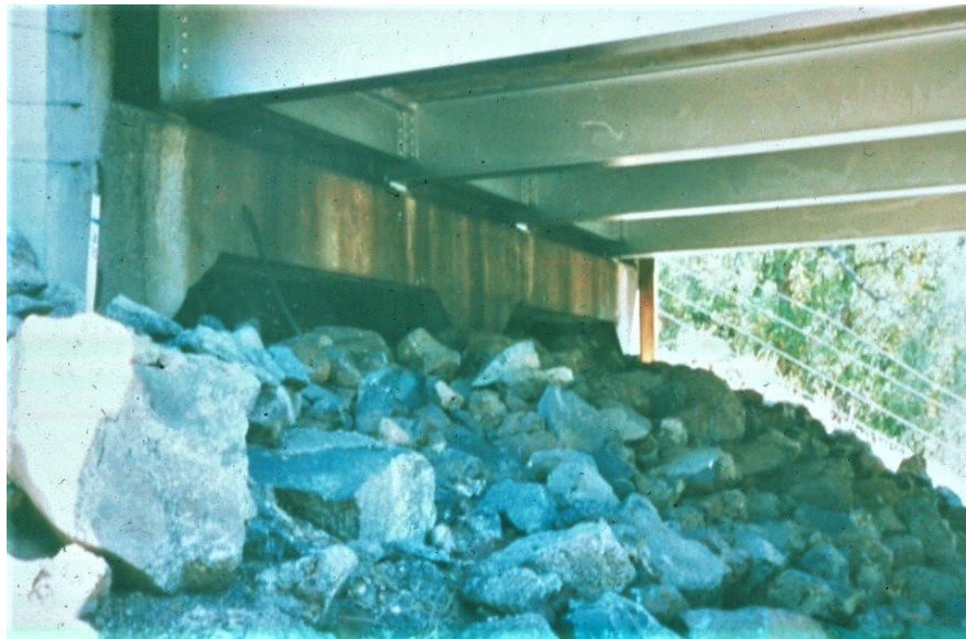
Figure 14.2.15 Spill Through/Open Abutment
