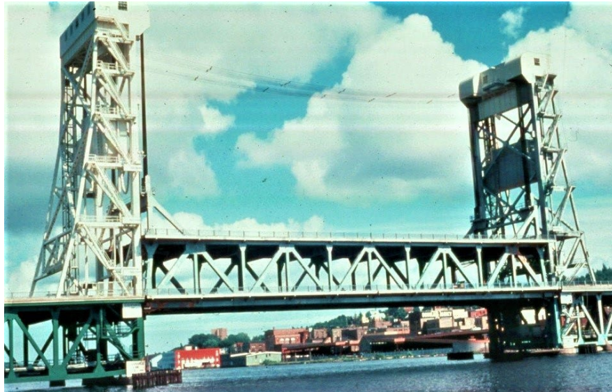
Figure 5.3.16 Tower-Drive Vertical Lift Bridge
