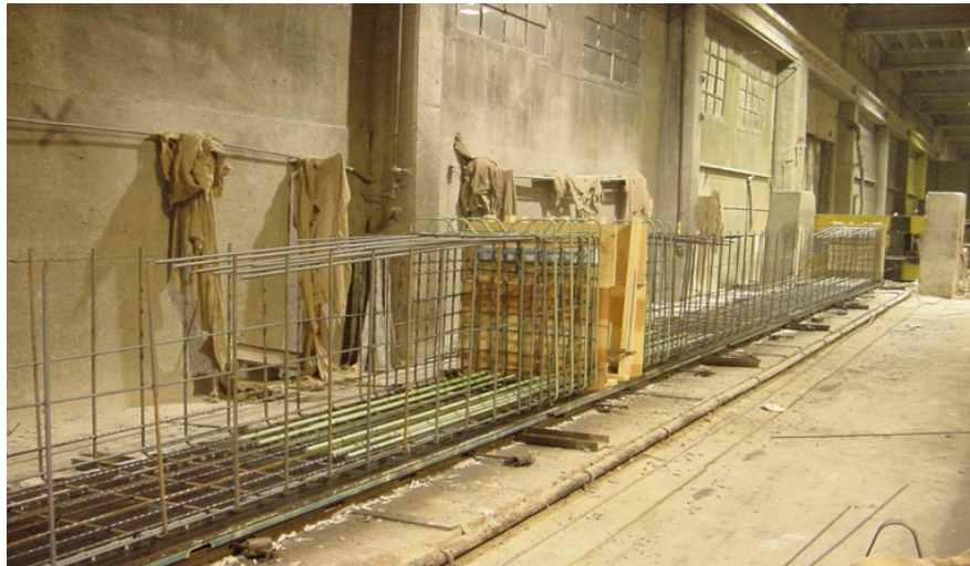
Figure 7.1.5 Fabrication of a Prestressed Concrete Beam
