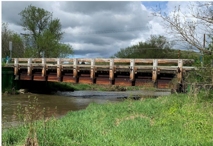
Figure 7.4.1 Glued-Laminated Modern Timber Bridge
