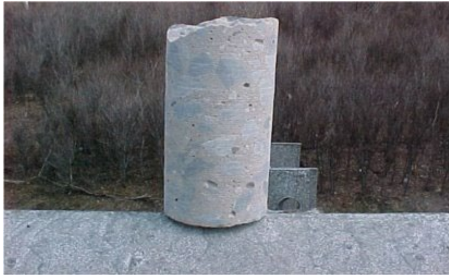
Figure 17.2.16 Concrete Core Sample
