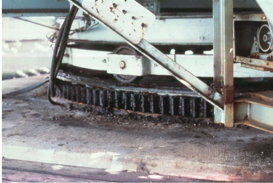
Figure 5.3.30 Balance Wheel in Place Over Circular Rack
