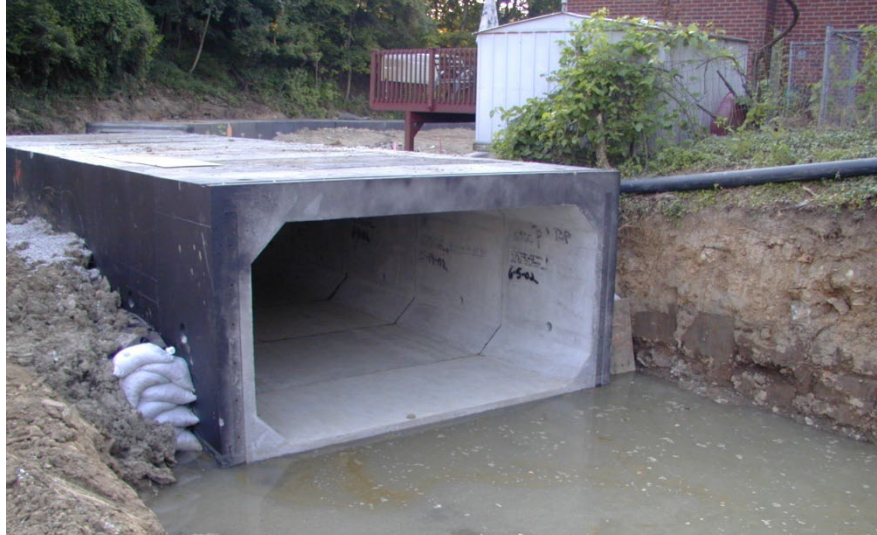
Figure 15.2.4 Precast Concrete Box Culvert under Construction
