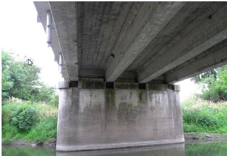
Figure 4.1.44 Concrete Tee Beam Bridge
