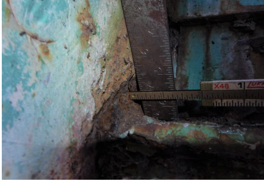
Figure 10.4.39 Using a Straightedge to Measure Gusset Plate Section Loss
