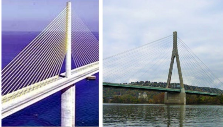
Figure 5.2.37 Single Column Tower and A-Frame Tower
