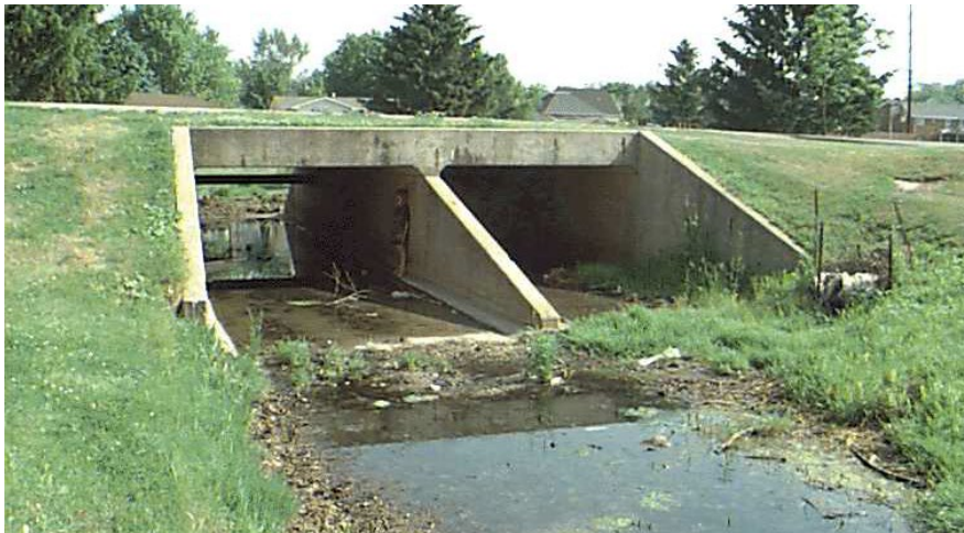
Figure 15.2.3 Multi-Cell Concrete Box Culvert
