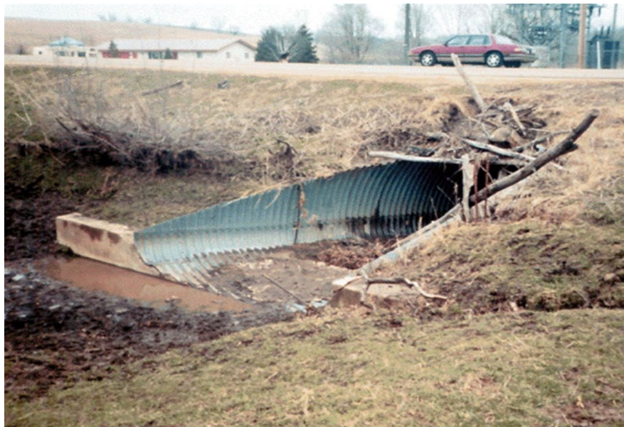
Figure 4.2.15 Culvert Mitered End
