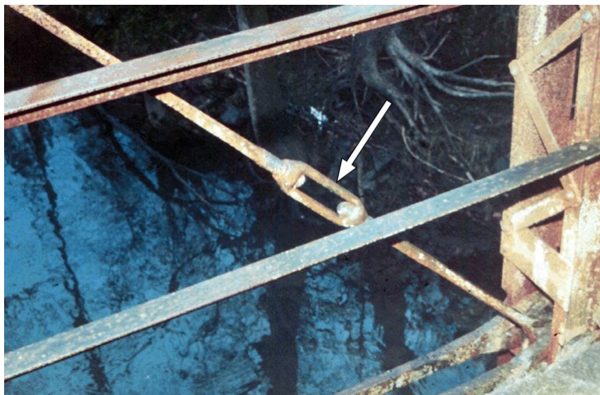
Figure 10.4.54 Turnbuckle on a Truss Diagonal
