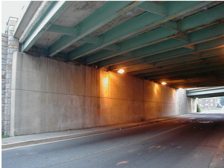
Figure 4.1.73 Cantilever Abutment (or Full Height Abutment)
