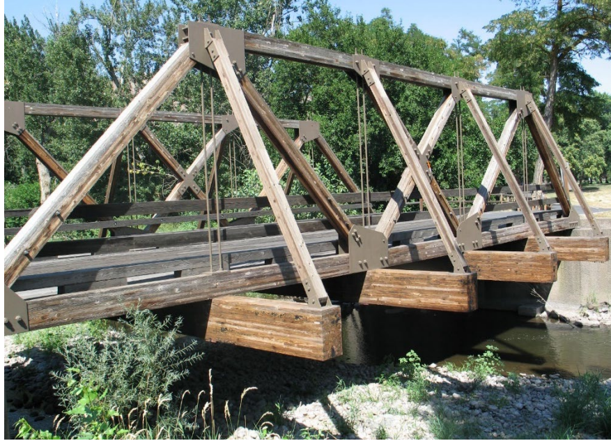
Figure 11.2.14 Timber Through Truss Bridge
