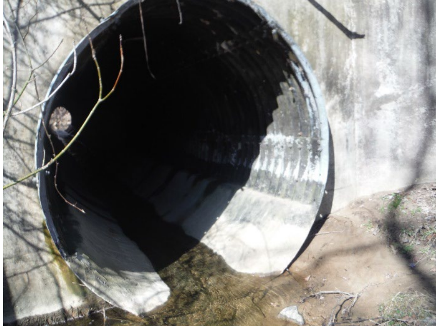
Figure 4.2.4 Circular Culvert Structure
