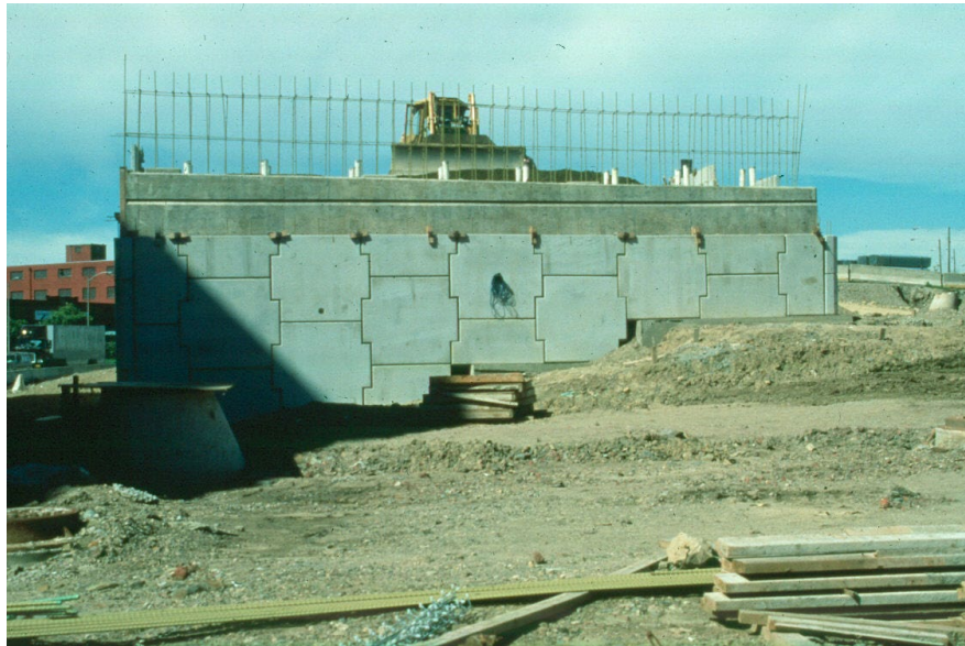
Figure 14.2.18 Mechanically Stabilized Earth Abutment
