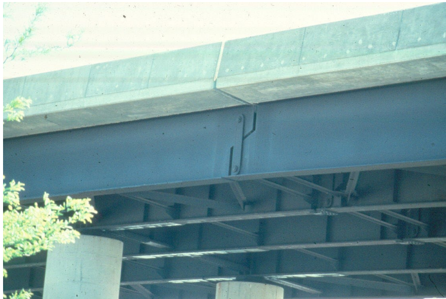
Figure 10.1.9 Plate Girder Bridge with Pin & Hanger Connection
