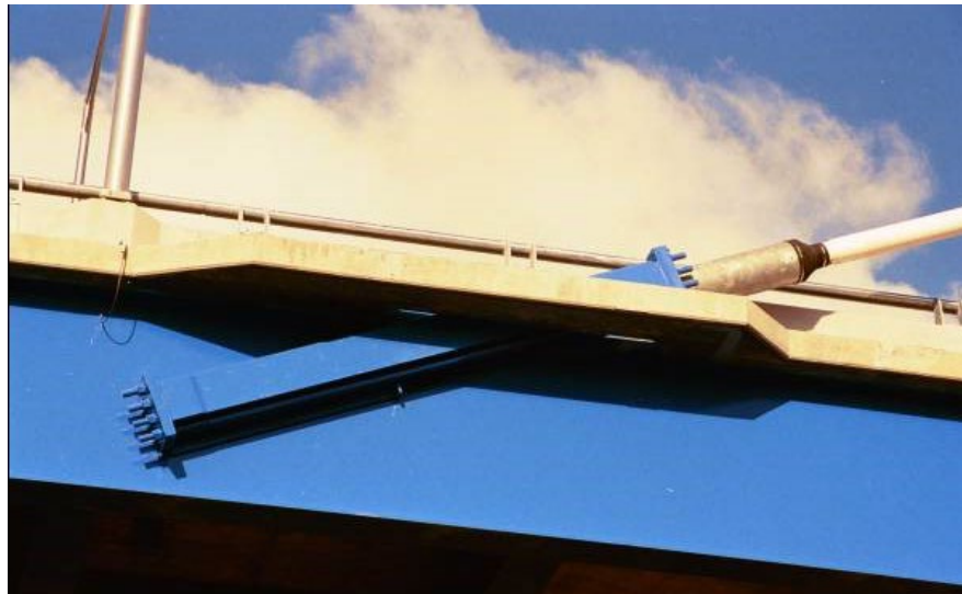
Figure 5.2.30 Cable Deck Anchorage
