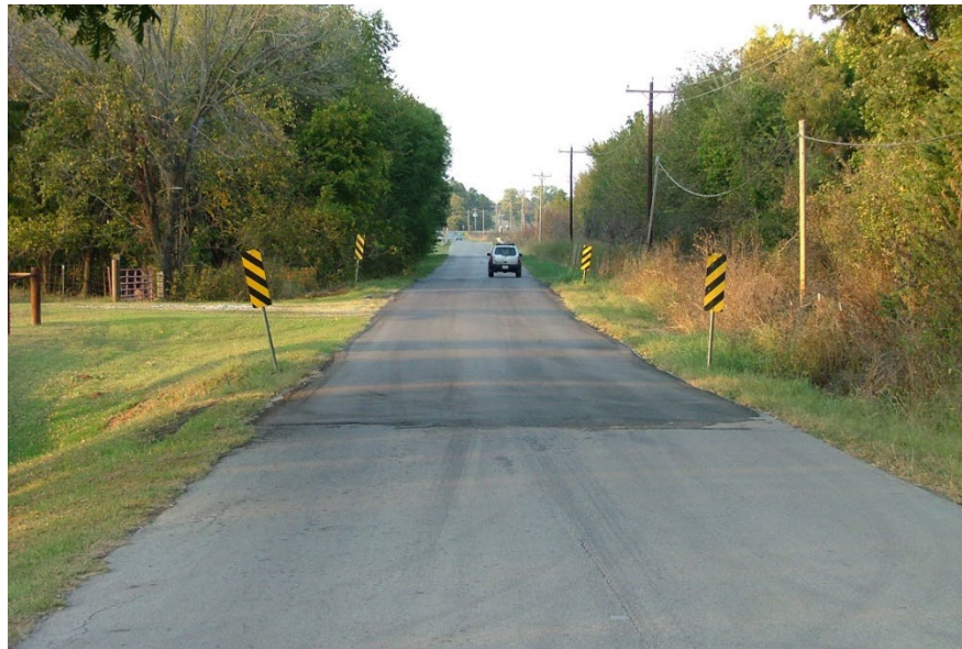
Figure 15.5.9 Repaired Roadway Over a Culvert
