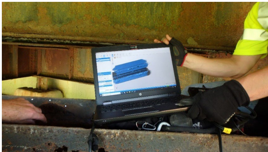
Figure 17.6.6 Laser Scan of Deteriorated Bridge Member
