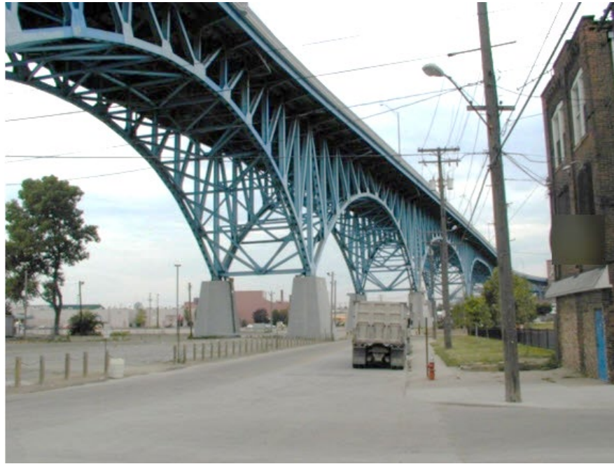
Figure 4.1.49 Deck Truss Bridge
