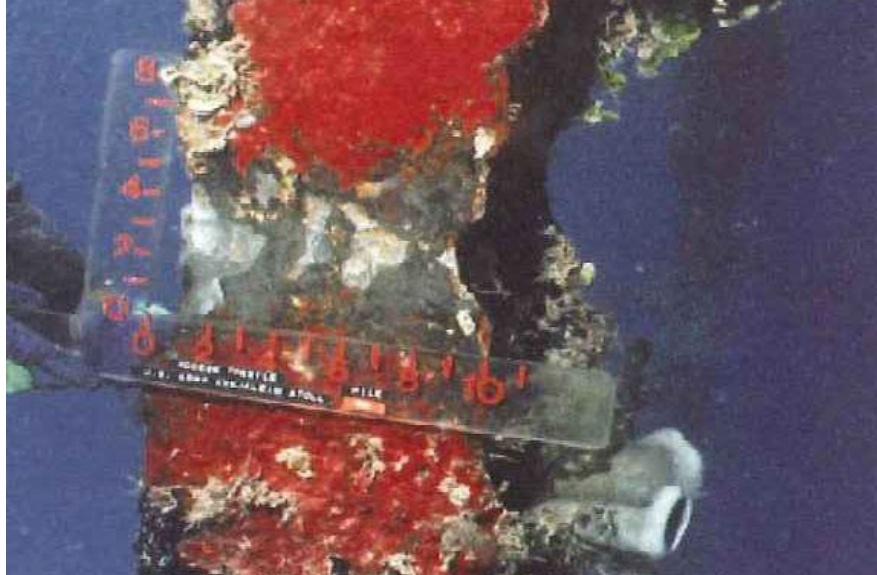
Figure 16.2.3 Level II Cleaning of a Steel Pile
