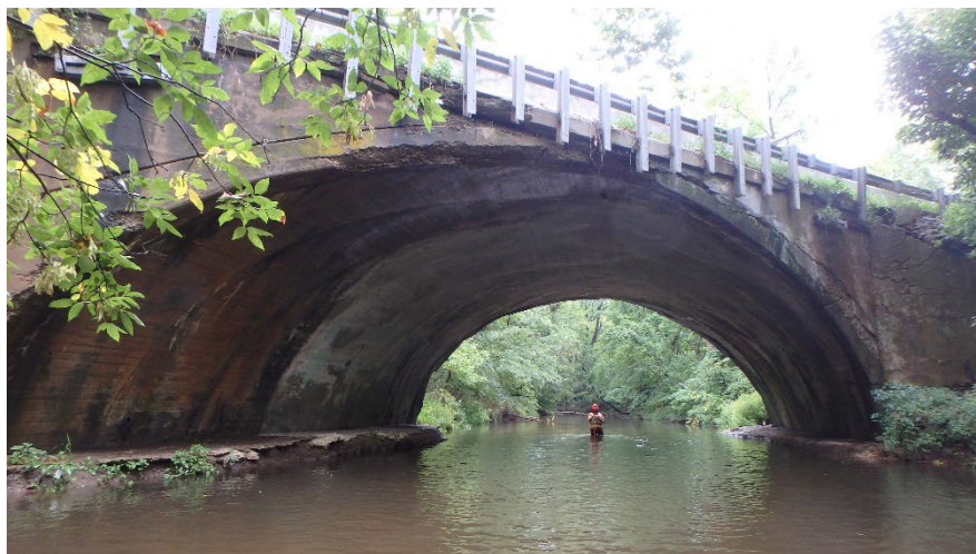
Figure 9.1.19 Closed Spandrel Arch Bridge
