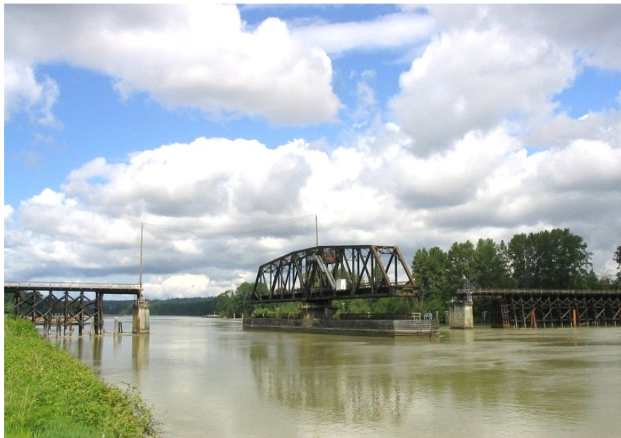
Figure 5.3.2 Center-Bearing Swing Bridge
