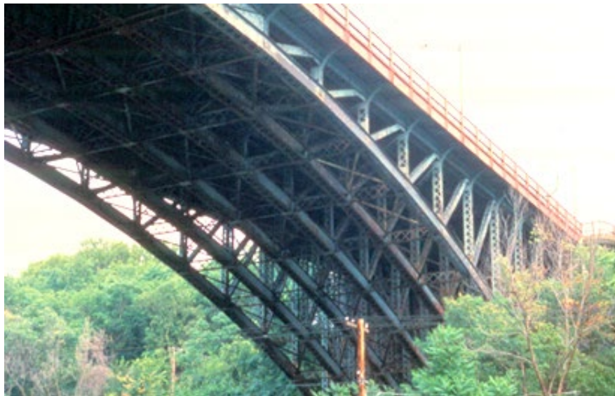
Figure 10.1.56 Spandrel Braced Deck Arch Bridge with Six Arch Ribs
