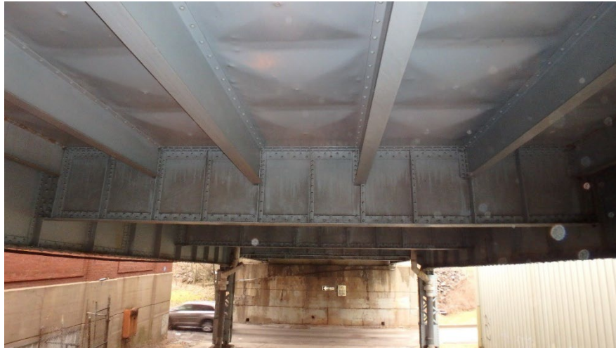
Figure 8.2.2 Underside View of Buckle Plate Deck
