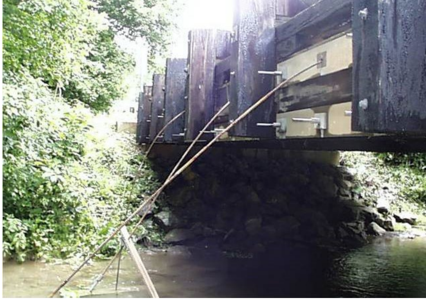
Figure 8.3.11 Failed Post-Tensioning Tendons
