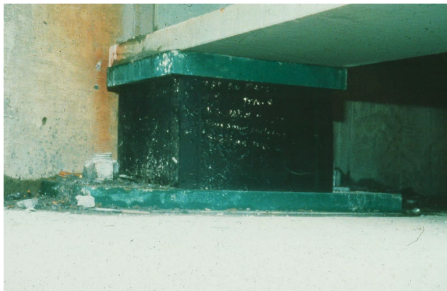
Figure 13.3.28 Lead Core Isolation Bearing
