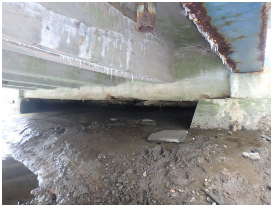
Figure 4.1.75 Spill Through or Open Abutment
