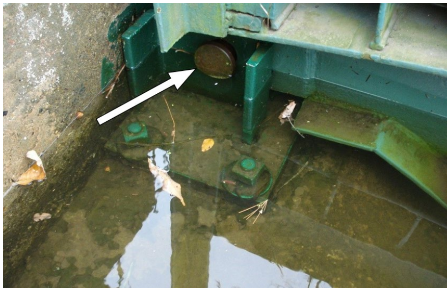
Figure 5.5.3 Fixed Pin Bearing
