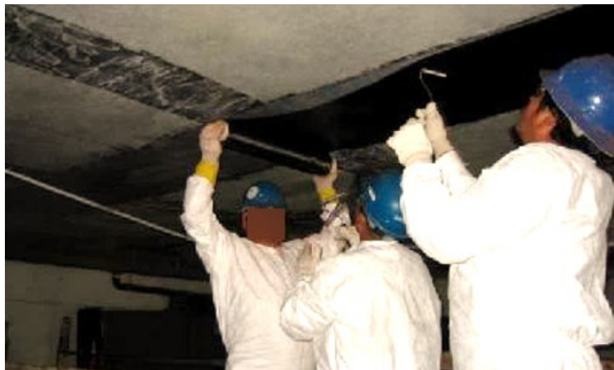
Figure 7.6.1 Concrete Beam Repaired Using FRP
