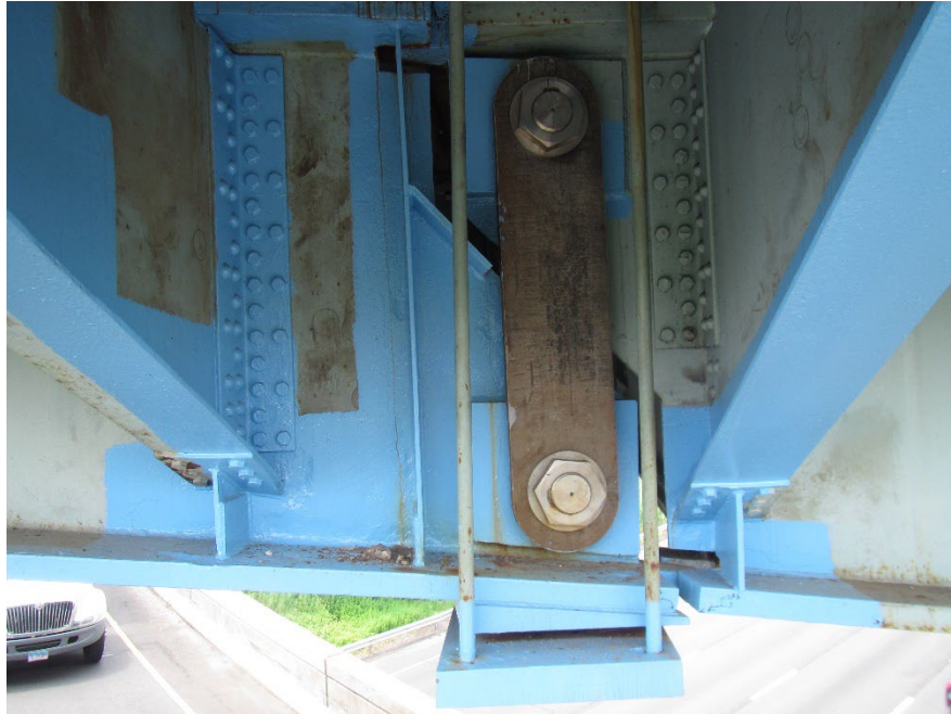
Figure 10.1.81 Rod and Saddle Retrofit
