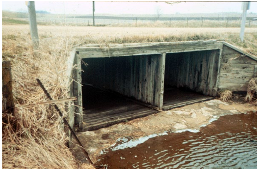
Figure 4.2.12 Timber Box Culvert
