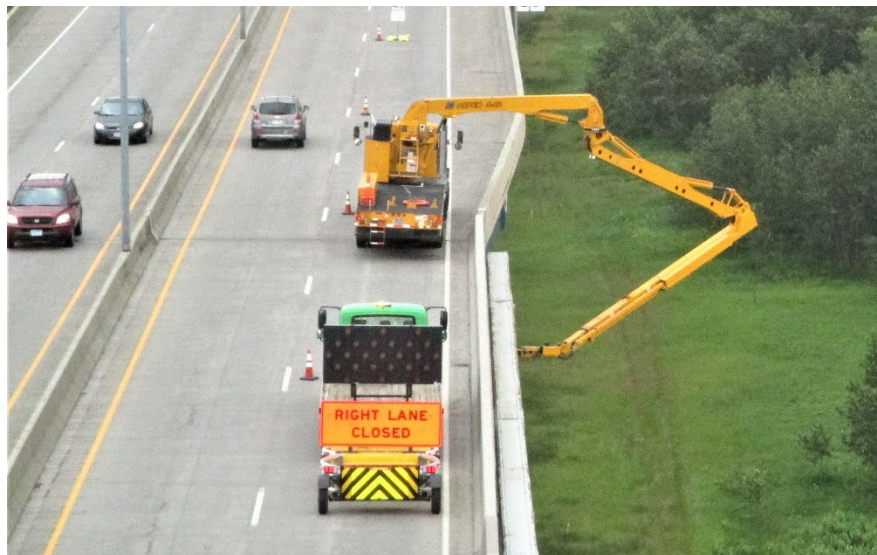
Figure 2.3.3 Inspection Vehicle with Traffic Control
