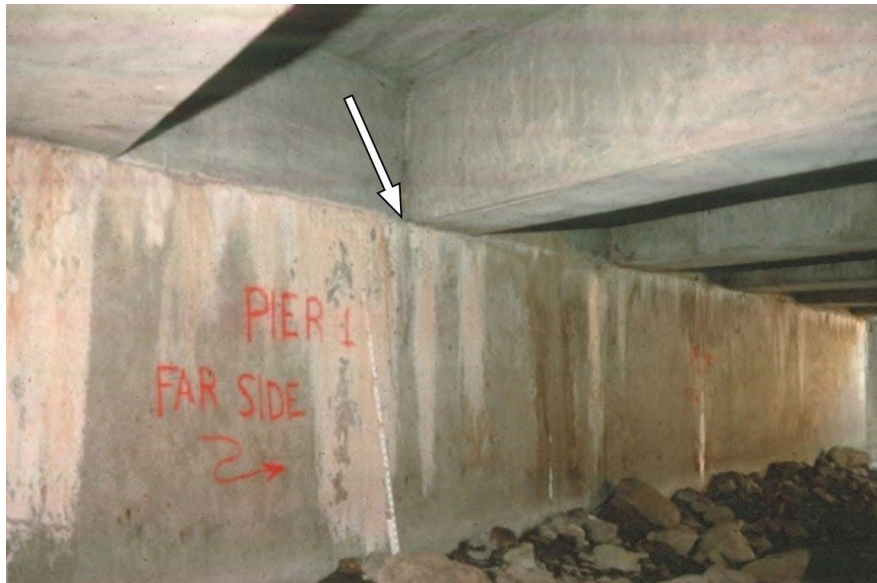
Figure 9.4.2 Bearing Area: Cast-in-Place Concrete Tee Beam Bridge
