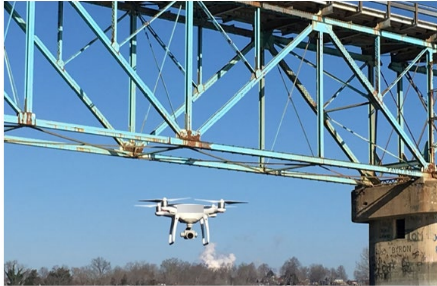
Figure 17.6.4 Drone Used for Bridge Inspection
