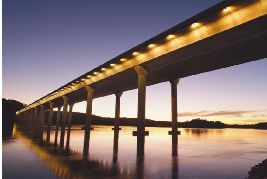
Figure 9.1.54 Precast Segmental Concrete Box Girder Bridge
