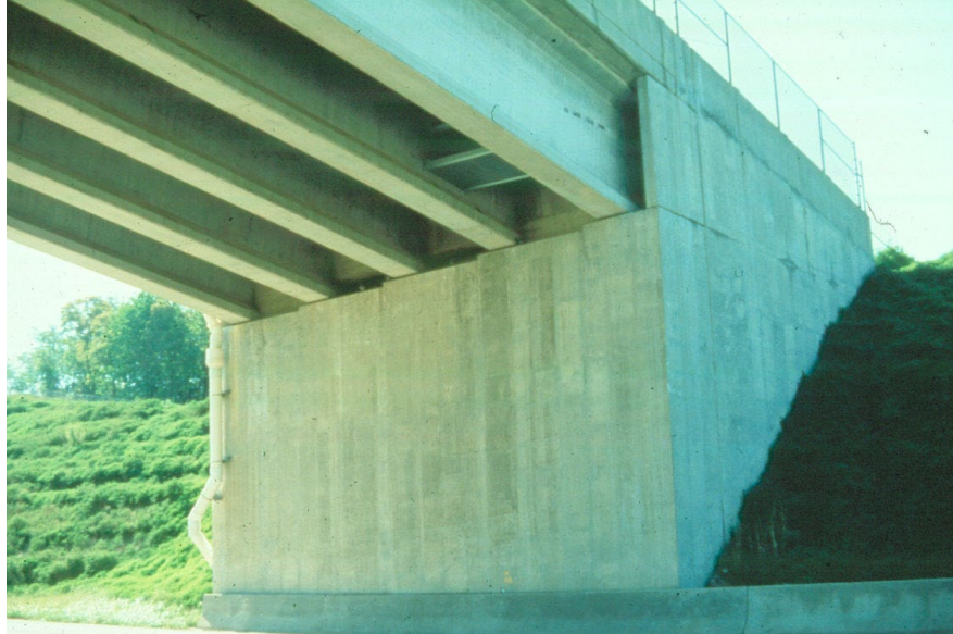
Figure 14.2.13 Full Height Abutment
