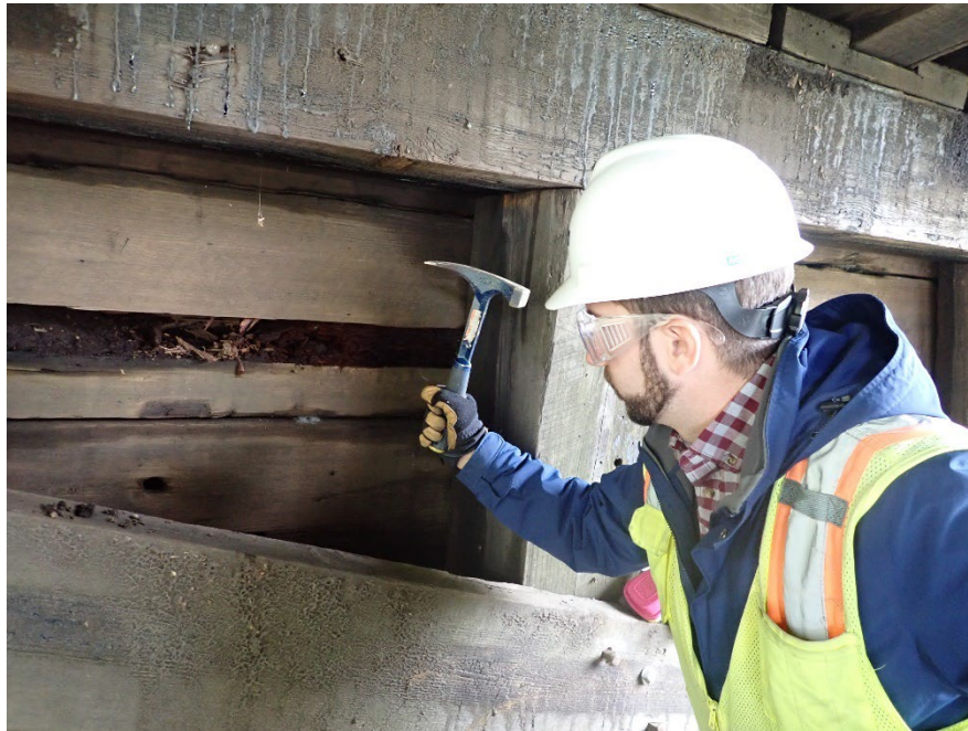
Figure 11.4.1 Inspector using Pick Hammer to Inspect Timber Substructure
