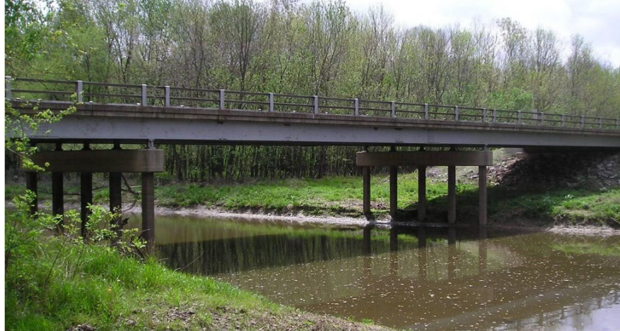
Figure 7.3.5 Structurally Redundant Continuous Span Bridges
