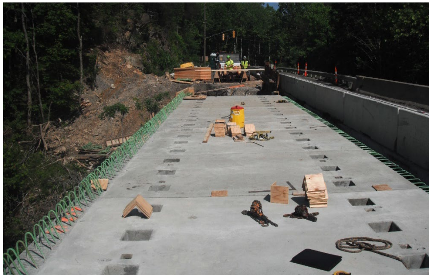
Figure 8.1.2 Block-Out Holes in Precast Panels
