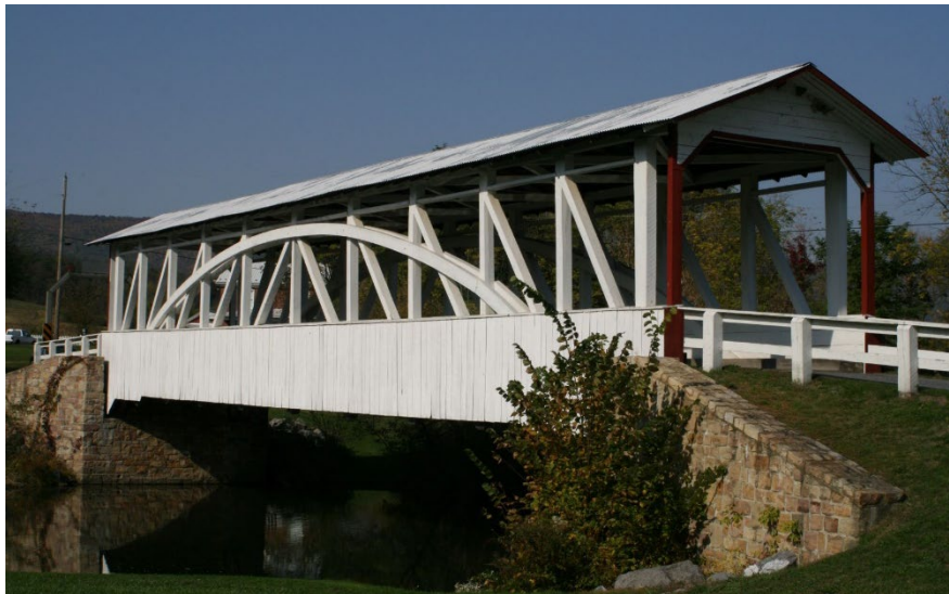
Figure 11.2.8 Burr Arch-truss Covered Bridge
