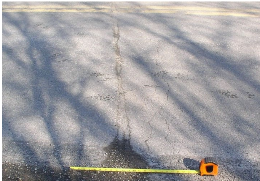
Figure 8.5.29 Asphalt Wearing Surface over an Expansion Joint
