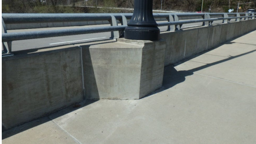
Figure 8.5.34 Light Pole Attached to a Bridge
