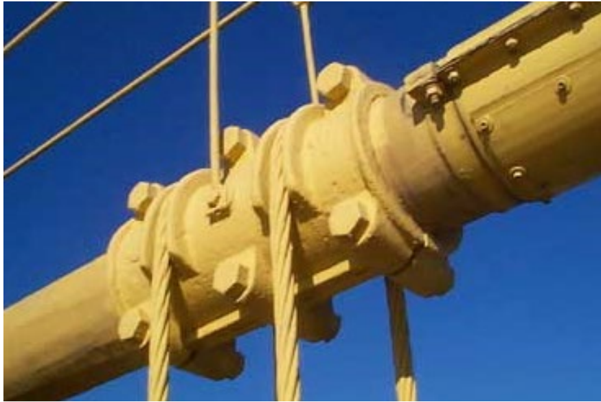
Figure 5.2.15 Grooved Cable Bands
