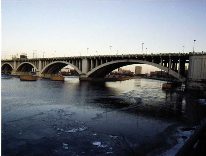
Figure 4.1.51 Deck Arch Bridge
