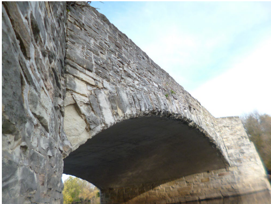
Figure 11.2.29 Masonry Closed Spandrel Arch Bridge
