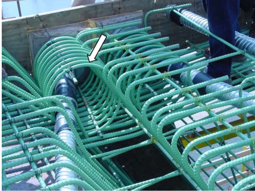
Figure 9.1.62 Post-tensioning Anchorage Reinforcement Before Concrete Placement
