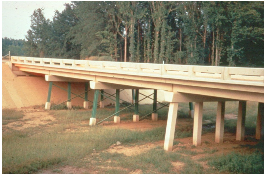
Figure 4.1.83 Steel and Concrete Pile Bents
