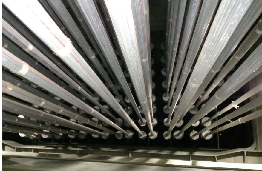
Figure 5.2.4 Parallel Wire Cables
