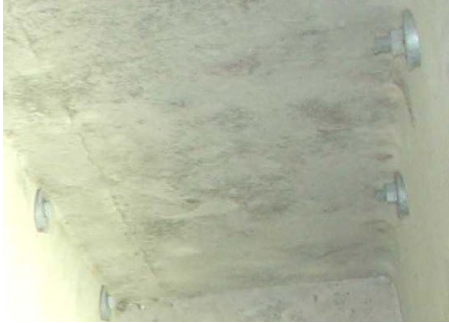
Figure 9.4.36 Stem Tie Bolts
