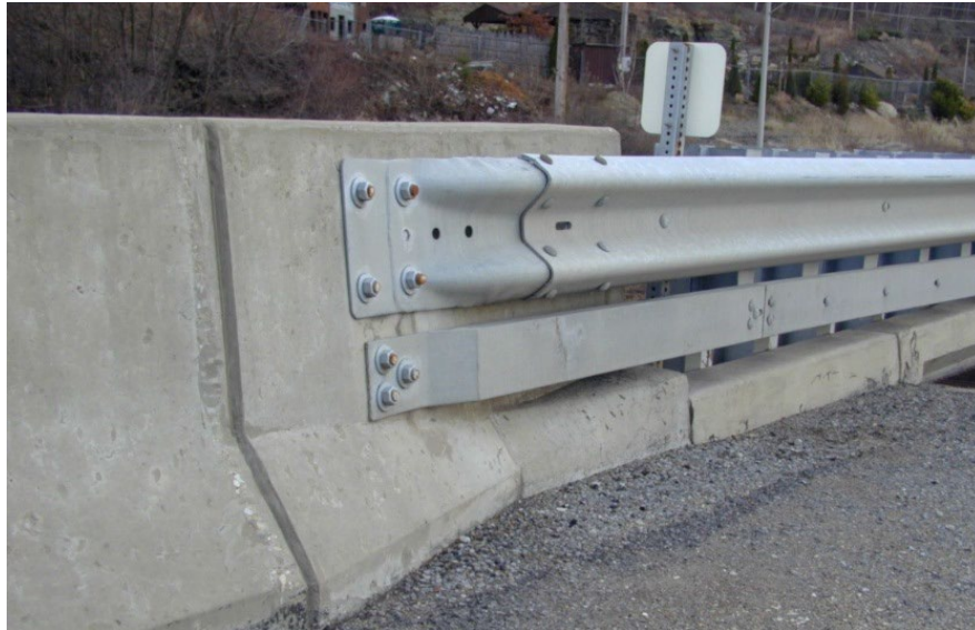
Figure 8.6.7 Proper Nesting of Guardrail at Transition
