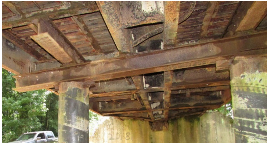
Figure 10.4.60 Flat Car Bearing Directly on Bent Cap
