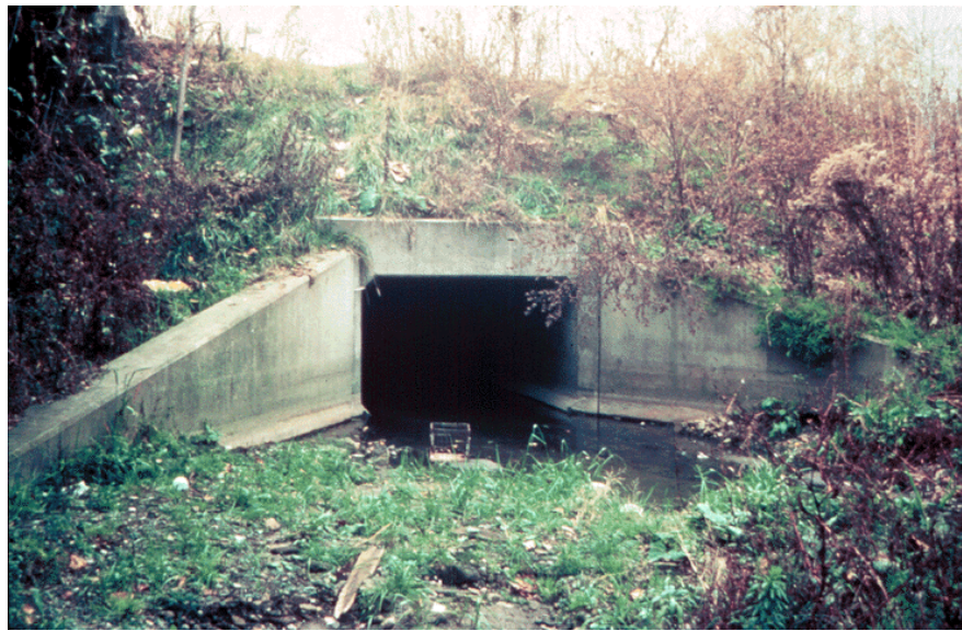
Figure 15.5.14 Culvert Wingwalls with Exposed Footings
