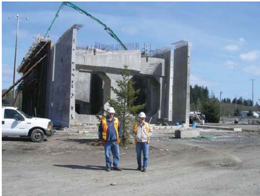
Figure 5.4.5 Concrete Pontoons Under Construction
