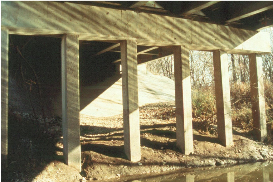
Figure 14.2.48 Concrete Pile Bent
