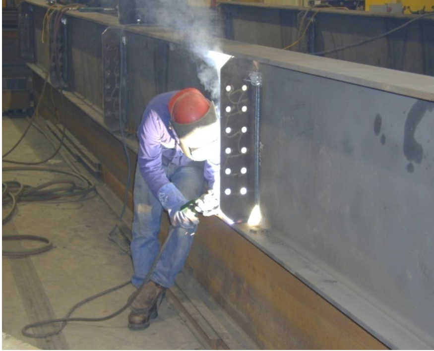
Figure 7.2.2 Steel Plate Welded to Girder
