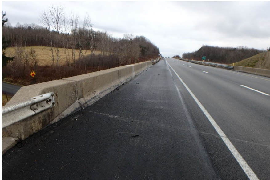
Figure 4.1.33 Asphalt Wearing Surface on a Concrete Deck
