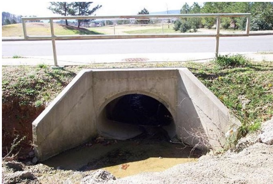
Figure 4.2.17 Culvert Head Wall and Wingwalls
