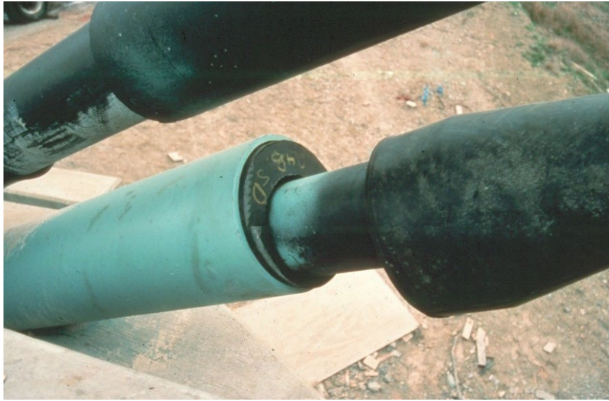
Figure 12.2.12 Neoprene Boot at Steel Anchor Pipe Near Anchor
