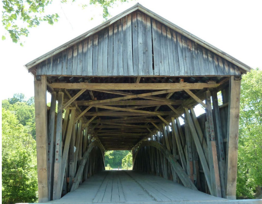
Figure 11.2.5 Truss Covered Bridge
