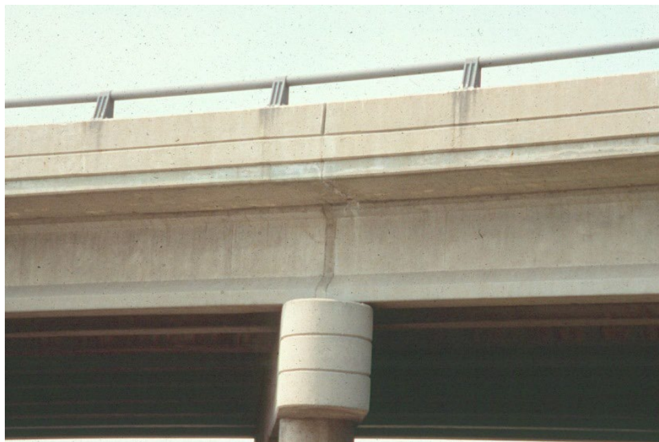
Figure 9.1.51 Continuous Prestressed I-beam Bridge
