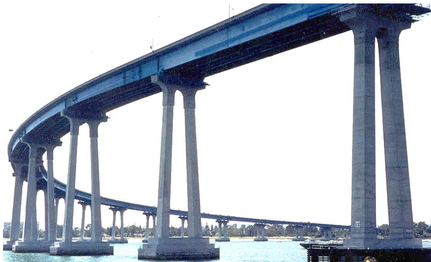
Figure 4.1.46 Steel Curved Girder Bridge
