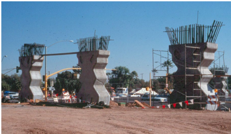
Figure 14.2.37 Reinforced Concrete Piers under Construction
