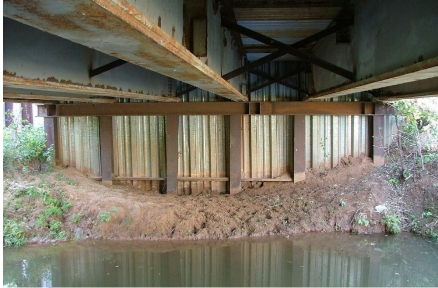
Figure 14.2.11 Steel Pile Bent Abutment
