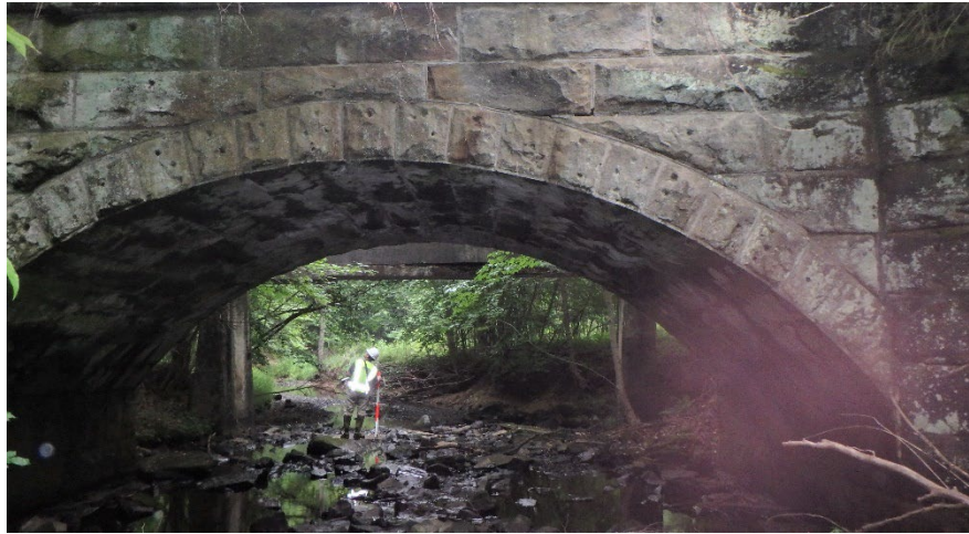
Figure 15.2.9 Stone Masonry Arch Culvert
