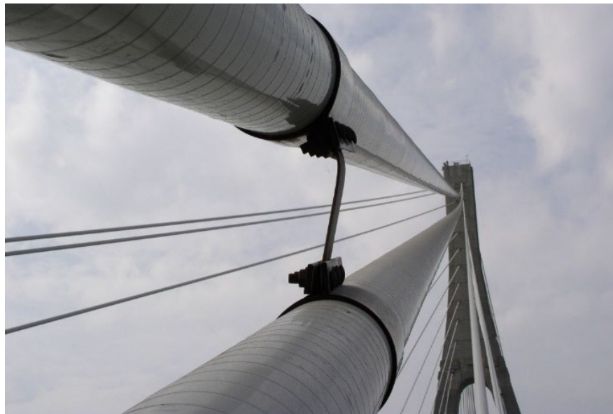
Figure 12.2.16 Cable Tie Type Damper System
