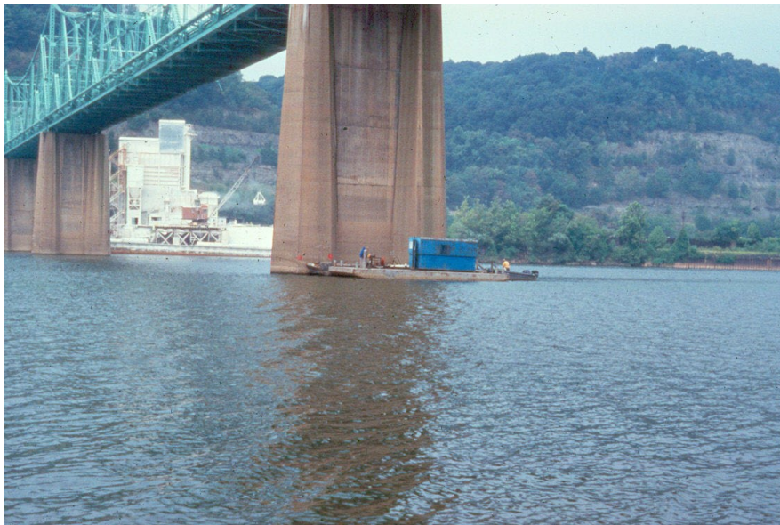
Figure 2.5.13 Inspection Operations from a Barge
