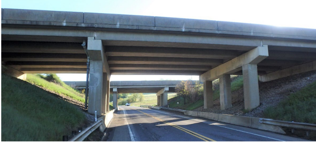
Figure 9.1.34 Typical Box Beam Bridge
