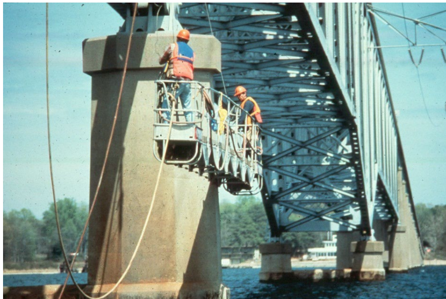
Figure 2.5.3 Rigging for Substructure Inspection
