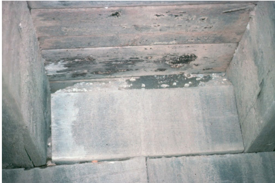
Figure 11.5.7 Typical Timber End Diaphragm
