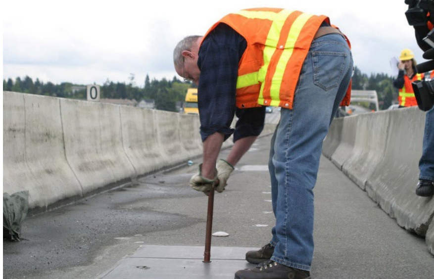
Figure 12.4.1 Inspector Opening Pontoon Access Hatch
