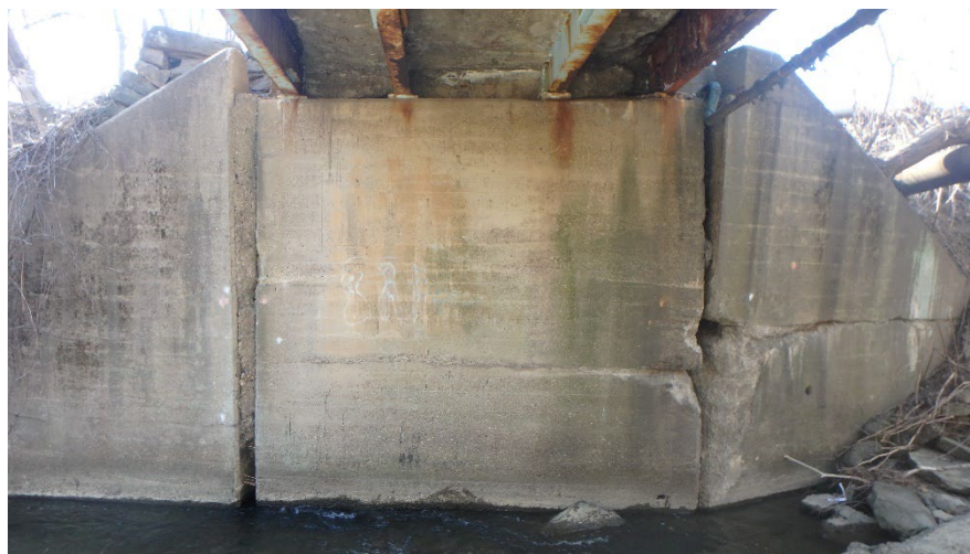
Figure 14.2.8 Plain Unreinforced Concrete Gravity Abutment
