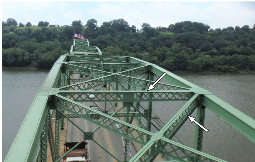
Figure 10.1.117 Upper Lateral Bracing on a Truss
