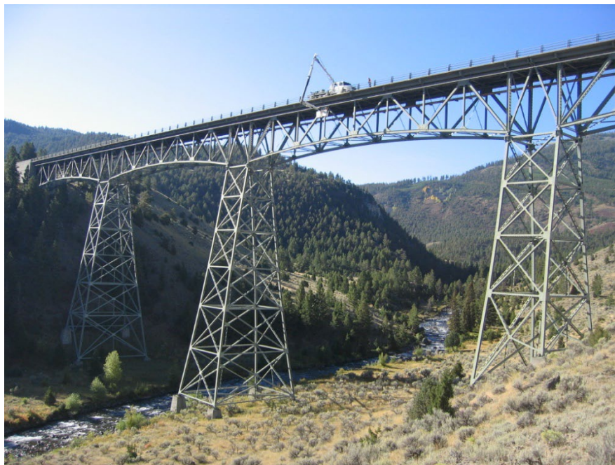
Figure 4.1.79 Tower (Trestle) Pier
