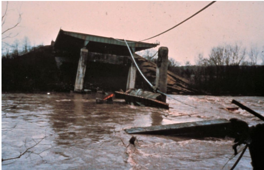
Figure 16.2.1 Schoharie Creek Bridge Failure
