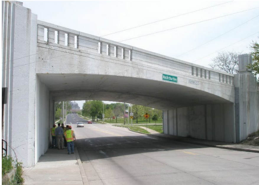
Figure 9.1.23 Single-span Rectangular Concrete Rigid Frame Bridge
