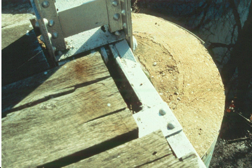
Figure 8.3.9 Bearing Area on a Timber Deck
