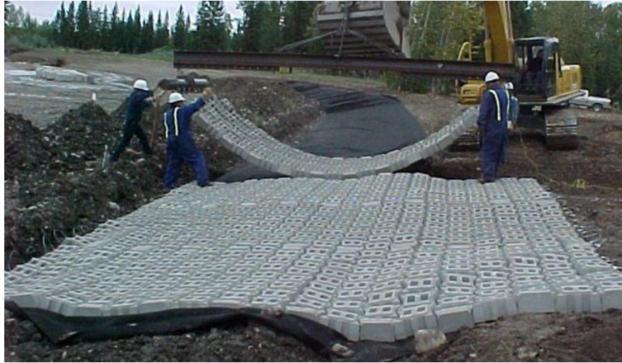
Figure 4.3.14 Concrete Revetment Mat
