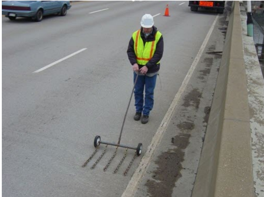
Figure 8.1.7 Sounding for Delaminated Areas of Concrete
