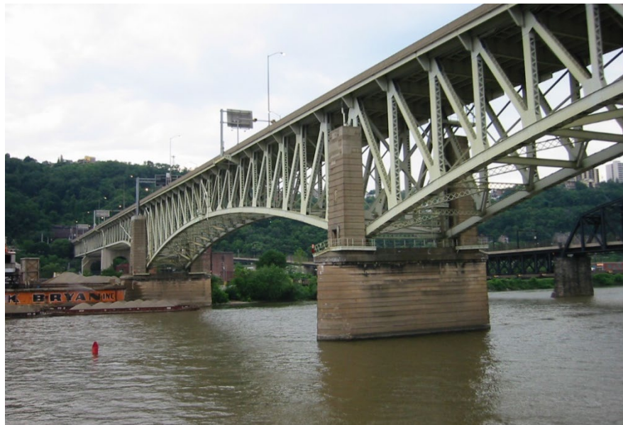
Figure 16.2.2 Liberty Bridge over Monongahela River
