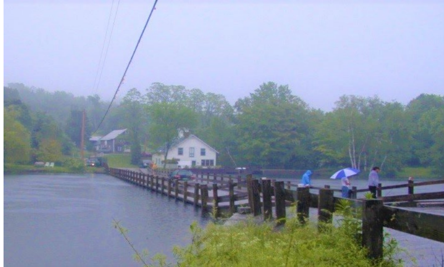
Figure 5.4.4 Floating Timber Bridge
