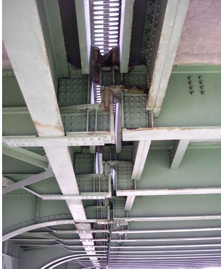
Figure 8.5.30 Support System under a Finger Plate Joint
