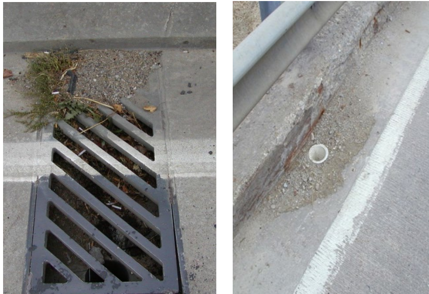
Figure 8.5.20 Bridge Deck Scupper (left) and Deck Drain (right)
