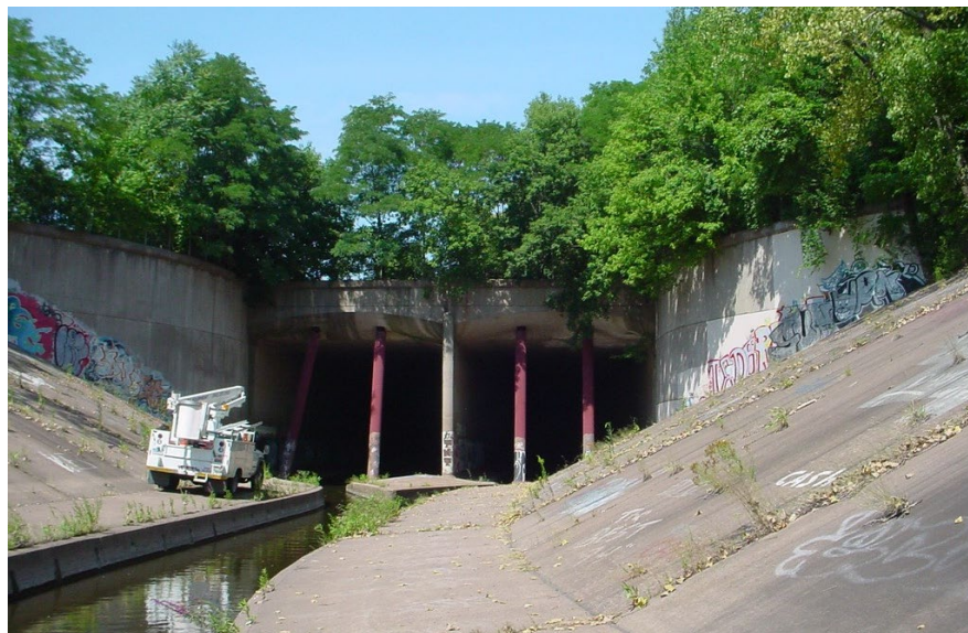
Figure 4.3.13 Formed Concrete Channel Lining
