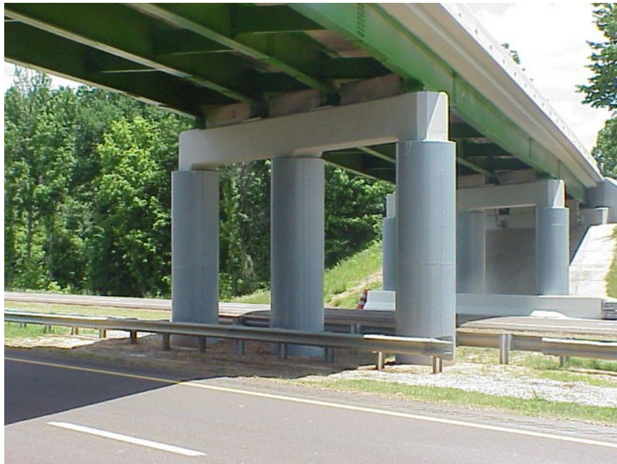
Figure 7.6.2 Seismic Retrofit of Concrete Columns Using FRP Composites
