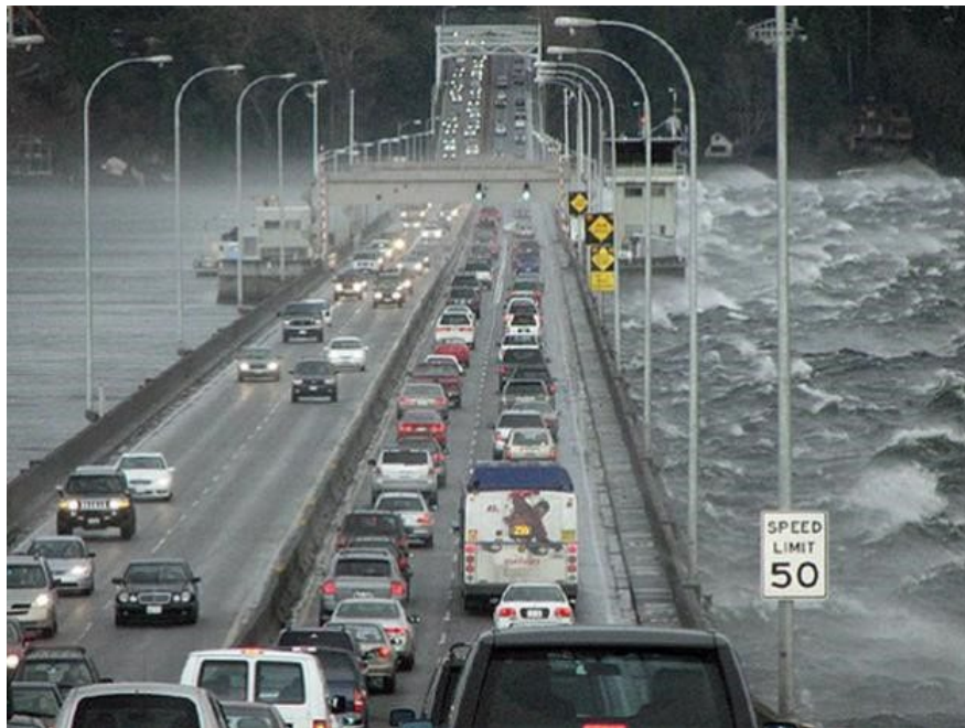
Figure 5.4.1 Floating Bridge During Stormy Weather
