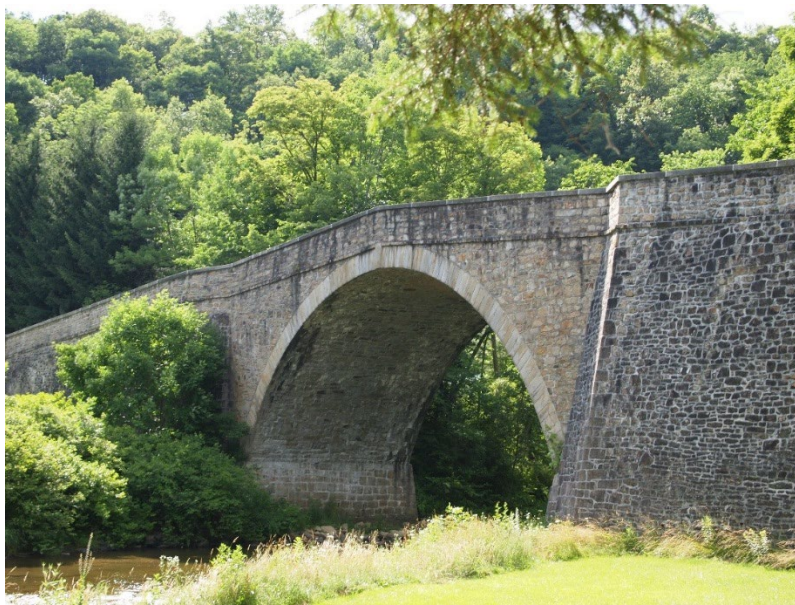
Figure 7.5.1 Stone Masonry Arch
