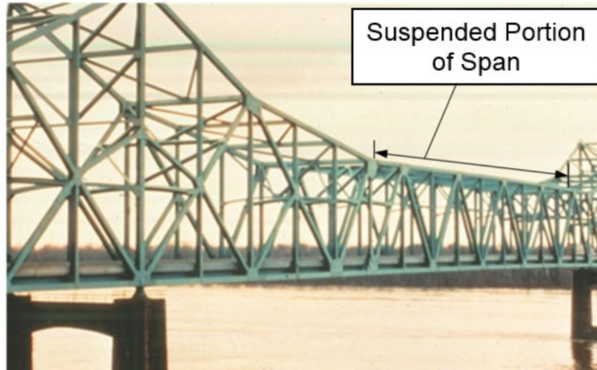
Figure 10.1.38 Cantilever Through Truss
