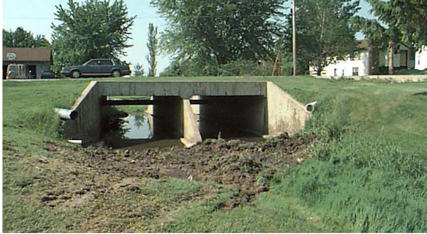
Figure 15.2.6 Concrete Frame Culvert
