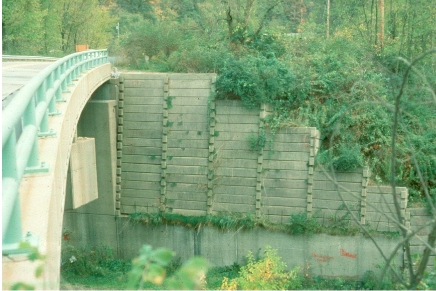
Figure 14.2.29 Straight Cribbed Wingwall
