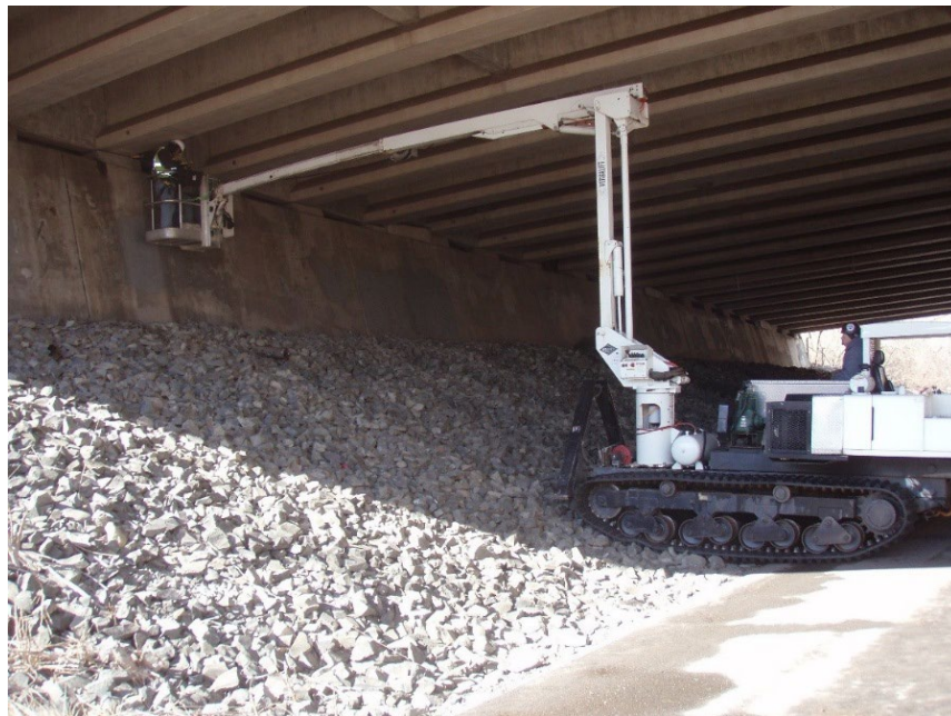
Figure 2.5.8 Track-mounted Manlift on a Slope
