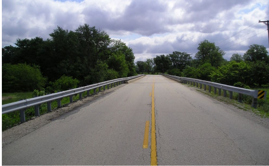
Figure 8.6.3 Bridge Railing, Transition, Approach Guardrail and Approach Guardrail End
