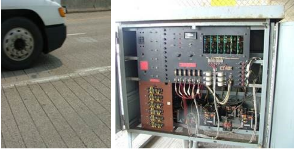
Figure 7.1.36 Cathodic Protection: Deck Wires Connected to Direct Current
