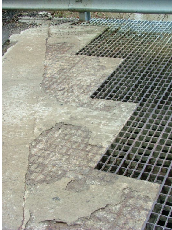
Figure 8.2.8 Filled and Un-filled Steel Grid Deck
