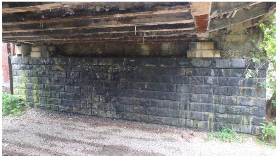
Figure 14.2.10 Stone Masonry Gravity Abutment
