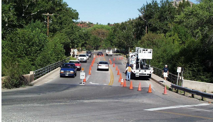
Figure 2.3.1 Temporary Traffic Control Operation
