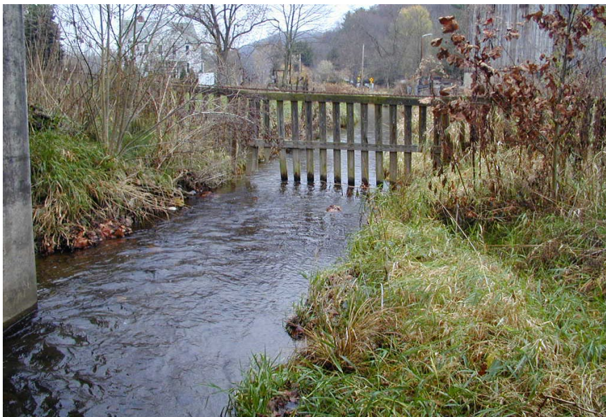
Figure 16.1.43 Fence in Stream at Bridge
