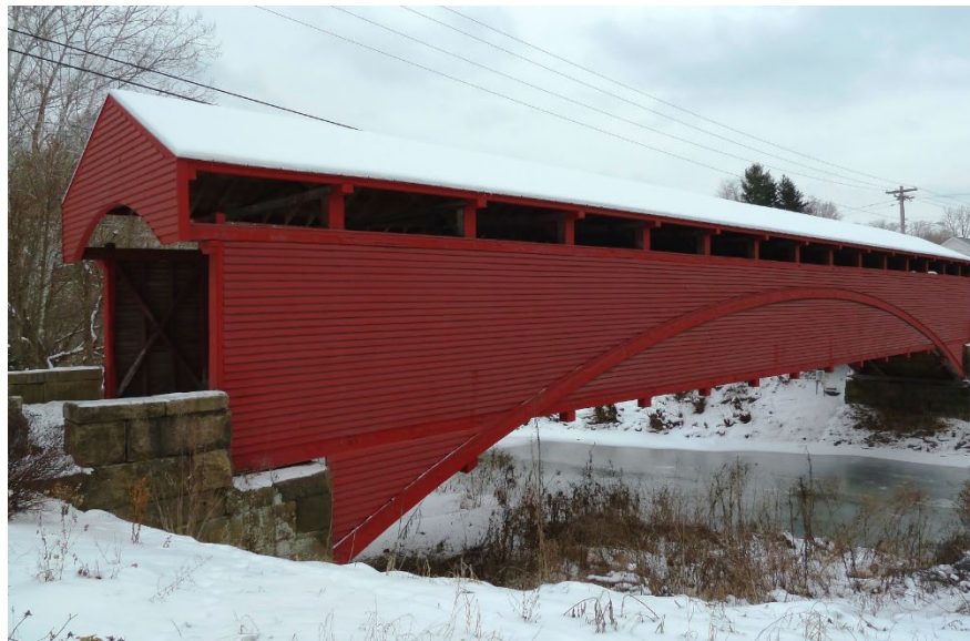
Figure 11.2.3 Elevation View of Covered Bridge
