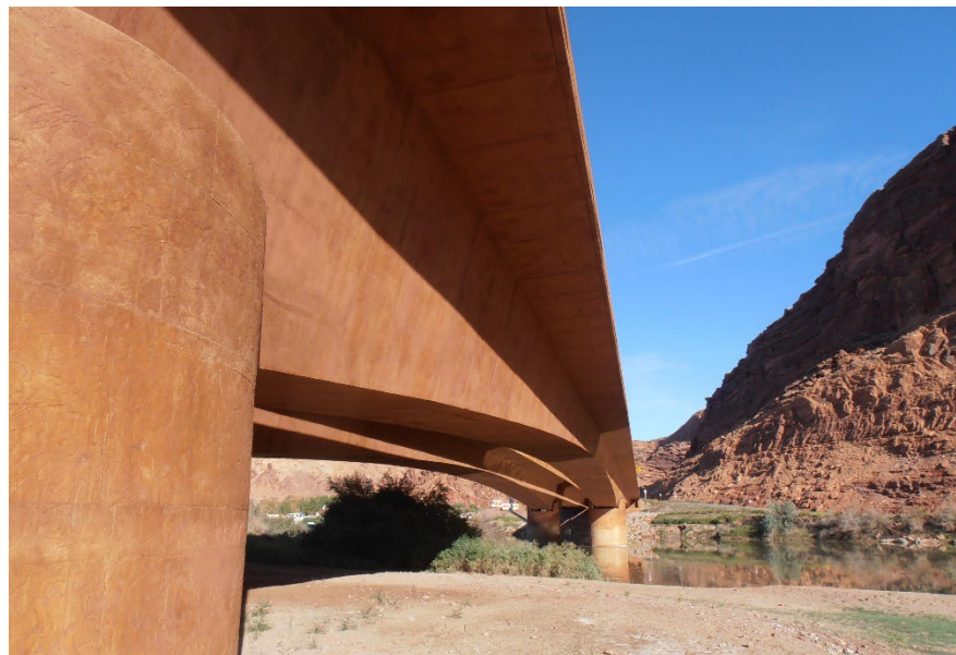
Figure 9.1.55 Cast-in-place Concrete Box Girder Bridge
