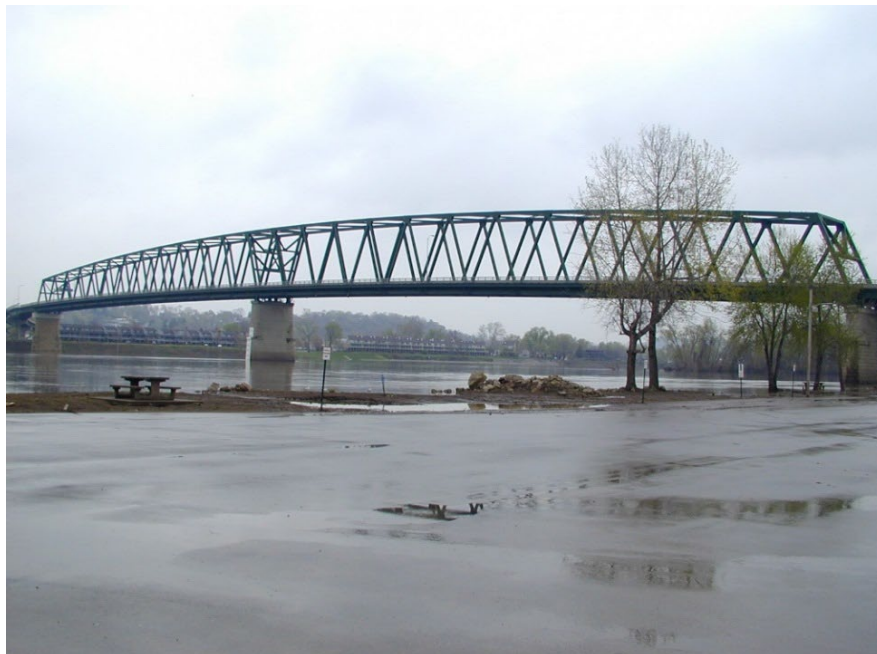
Figure 4.1.50 Through Truss Bridge
