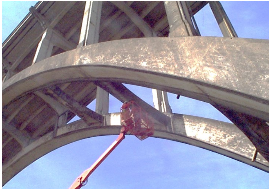
Figure 9.4.54 Inspection of Arch Strut (Secondary Member)
