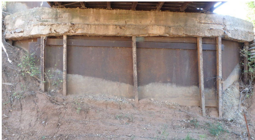
Figure 14.2.58 Stub Abutment on Piles with Piles Exposed
