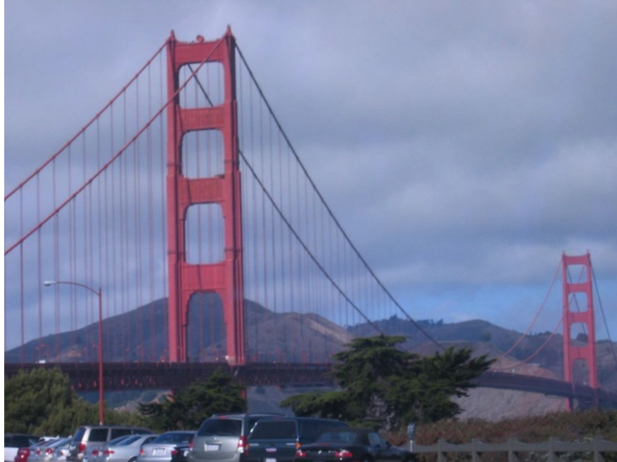
Figure 4.1.14 Cable-Supported Bridge: Suspension Cables and Hangers
