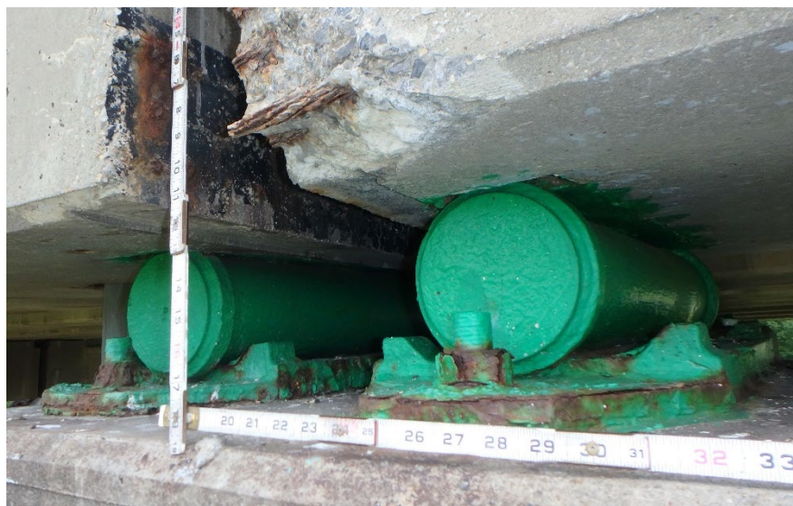
Figure 13.3.4 Single Roller Bearing
