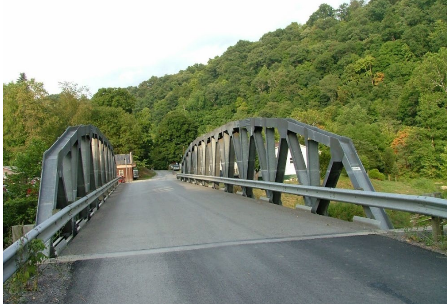
Figure 10.1.34 Single Span Camel Back Pratt Truss
