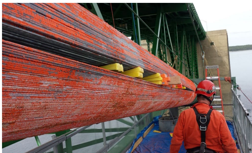
Figure 12.2.1 Inspection of Cable with Wedges
