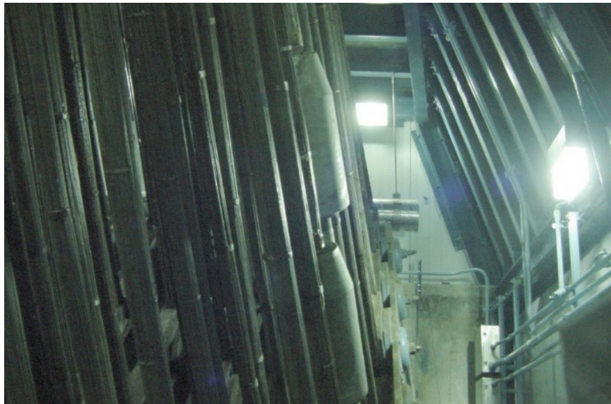
Figure 12.2.11 Chain Gallery (Anchor Vault) Interior
