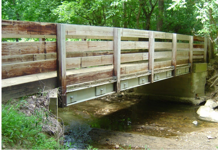
Figure 11.2.21 Stress-Laminated Timber Slab Bridge
