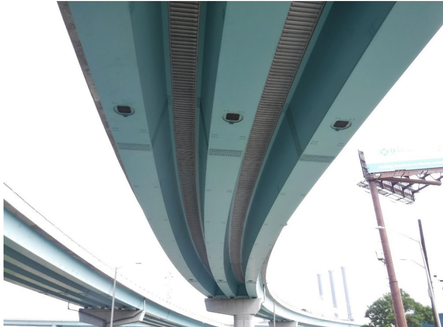
Figure 4.1.47 Steel Box Girder Bridge
