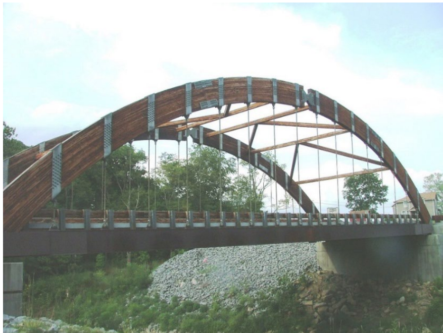
Figure 4.1.52 Through Arch Bridge
