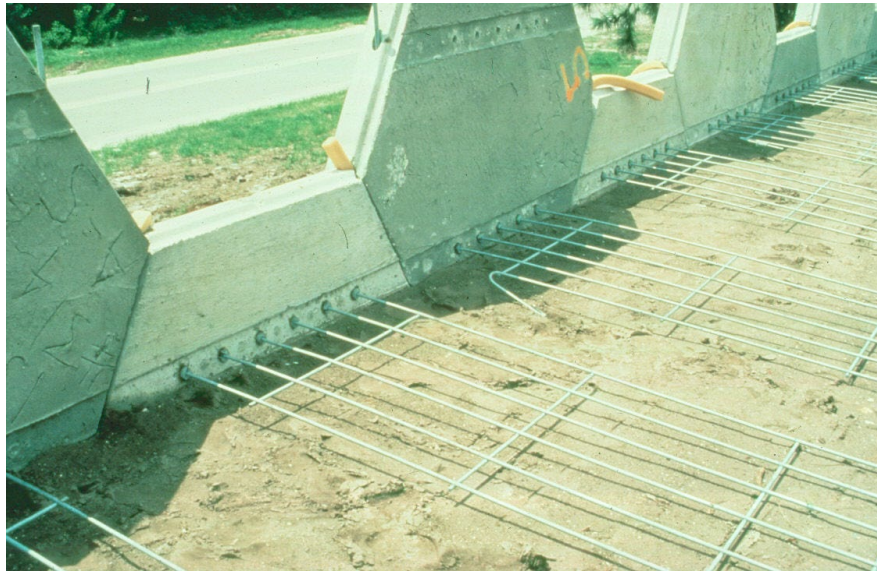
Figure 14.2.19 Mechanically Stabilized Earth Wall Under Construction
