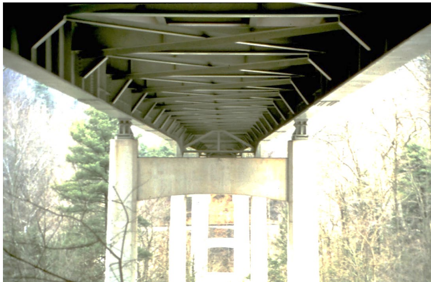
Figure 7.3.9 Nonredundant Two Girder Bridge
