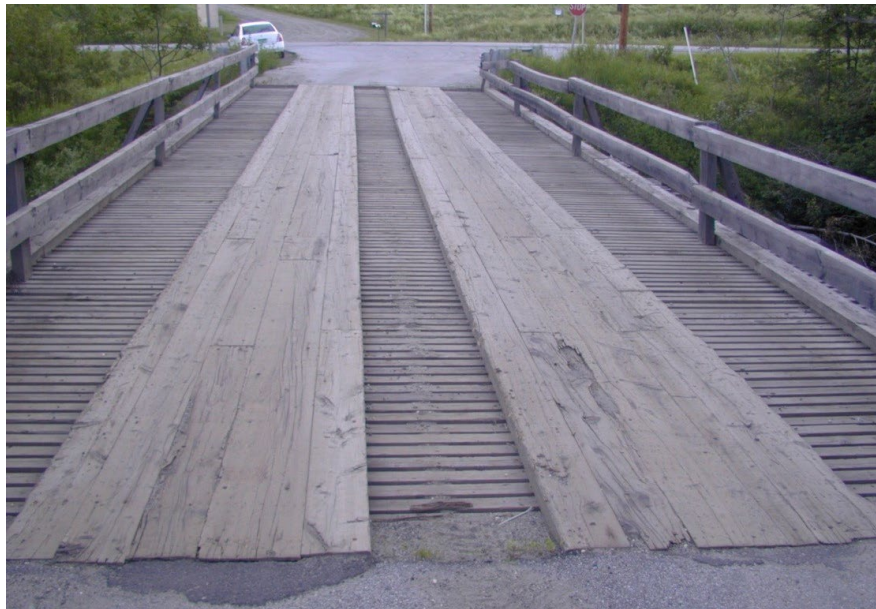
Figure 8.3.6 Timber Wearing Surface on a Timber Plank Deck
