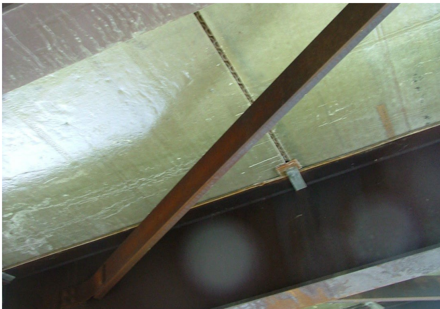
Figure 8.4.1 Fiber Reinforced polymer (FRP) Deck
