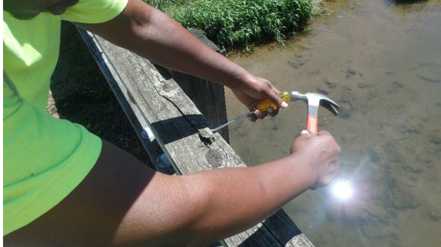
Figure 8.3.7 Inspector Probing Timber with a Pick
