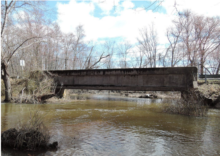
Figure 9.1.11 Concrete Through Girder Bridge
