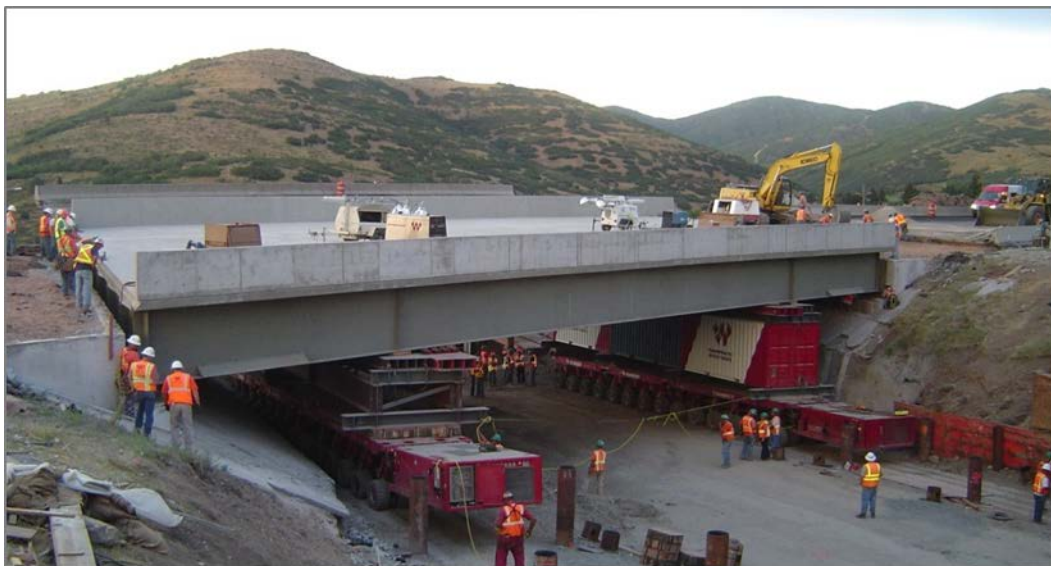
Figure 4.3.8-2. Actual SPMT Bridge Move.
