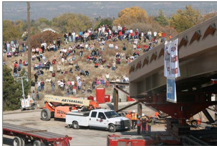
Figure 4.6.6.1-1. Photo from 4500 South showing the public watching the bridge move.
