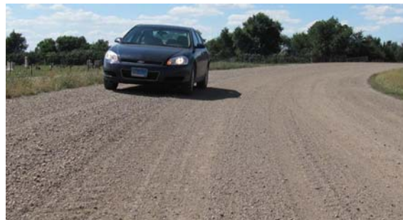
Figure 18. Photo. Super-elevation on sharp curve.
