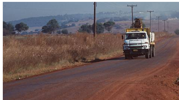
Figure 91. Photo. Road after treatment.
