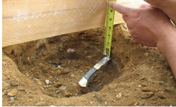
Figure 87. Photo. Checking gravel thickness.
