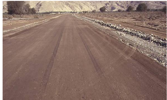
Figure 52. Photo. Electrochemical additive.
