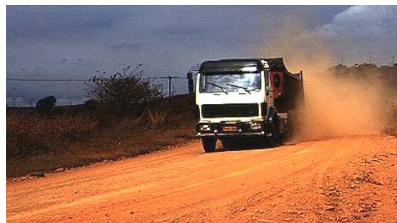
Figure 90. Photo. Road before treatment.
