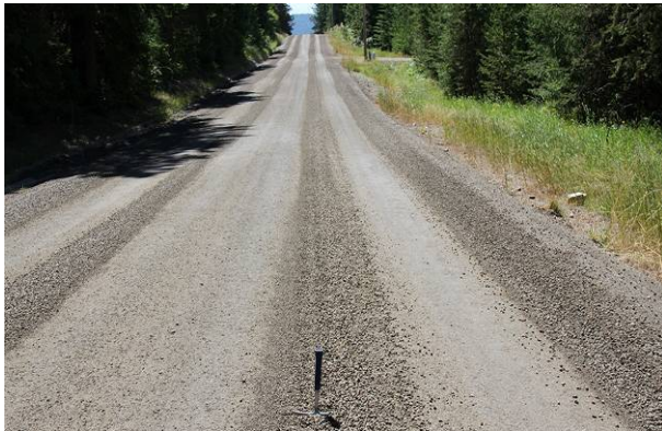
Figure 40. Photo. Raveling.
