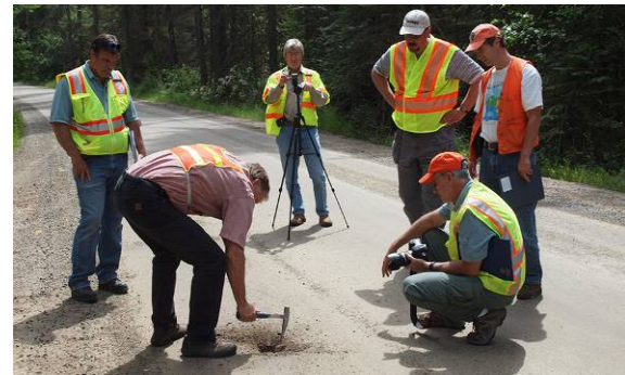
Figure 5. Photo. Evaluating the road.
