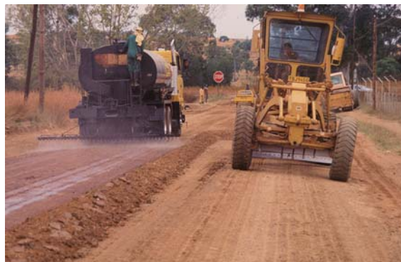
Figure 14. Photo. Mix-in treatment.
