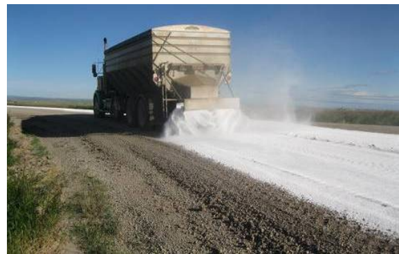
Figure 75. Photo. Flake application of calcium chloride.
