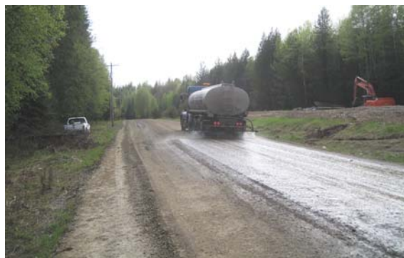
Figure 13. Photo. Spray-on treatment to well-prepared road.
