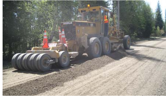
Figure 9. Photo. Grader maintenance.
