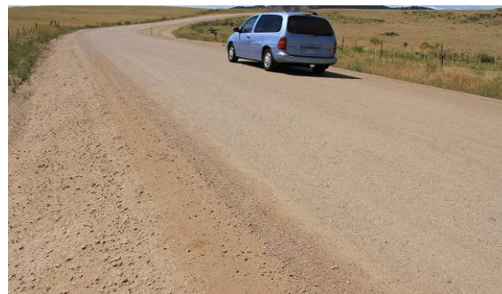
Figure 21. Photo. Road with good drainage.
