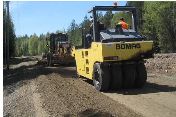
Figure 80. Photo. Compaction with rubber-tired roller.
