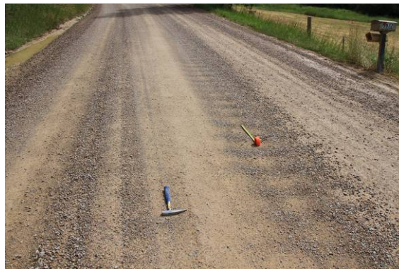
Figure 59. Photo. Chloride applied to poorly prepared road.
