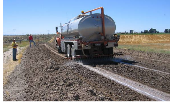
Figure 79. Photo. Spraying the additive.
