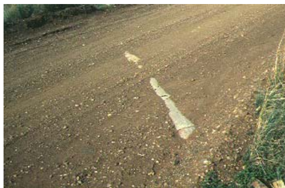
Figure 26. Photo. Road requires upgrade before treatment.
