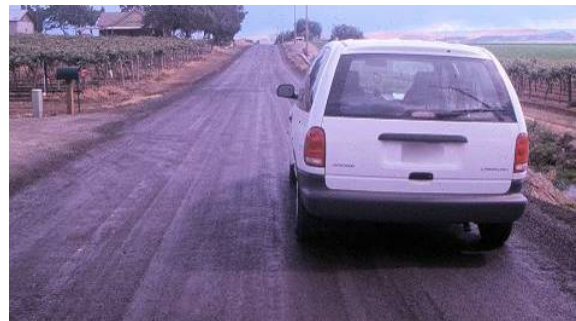
Figure 81. Photo. Completed road.
