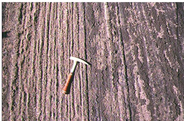
Figure 71. Photo. Poor penetration without pre-wetting.
