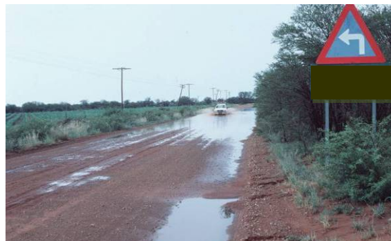
Figure 66. Photo. Road below natural ground level.
