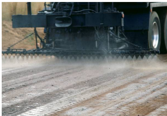
Figure 72. Photo. Penetration with pre-wetting.
