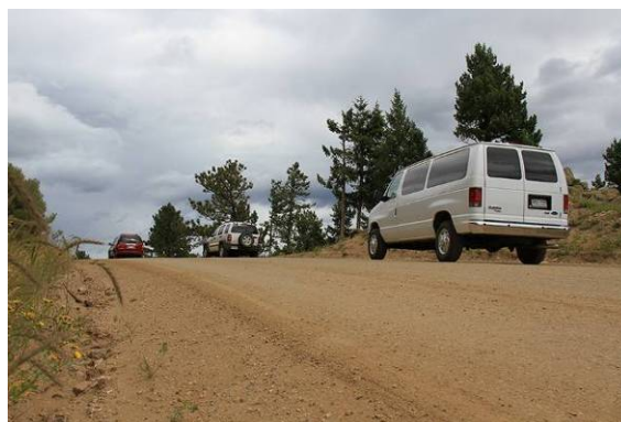
Figure 60. Photo. Good crown (4 to 6%).
