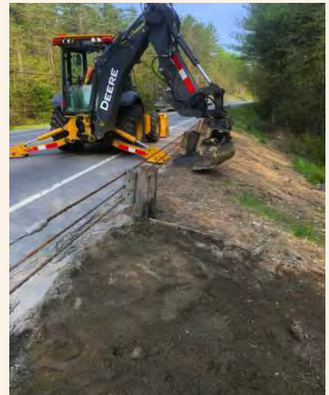
© 2023 New Hampshire Department of Transportation
