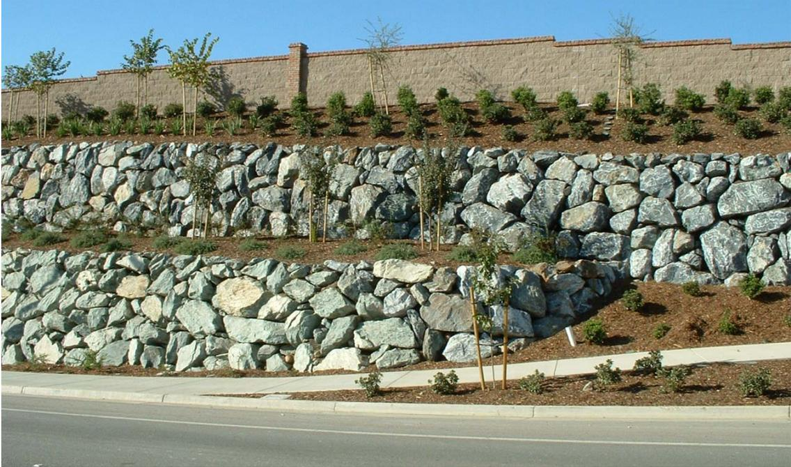
**Figure 74. Photograph. Example of proper layout, interlock, and chinking of variable shape and size rocks.**
