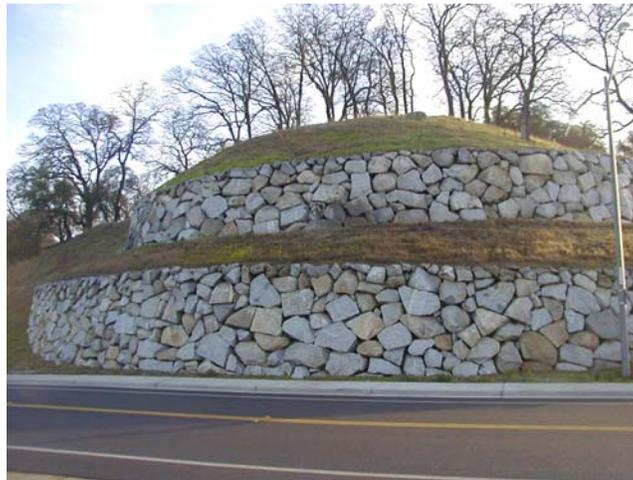
**Figure 21. Photograph. “Protecting” rockery used as a facing material for a two-tier, 7.6-m-high (25-ft-high) soil-nail wall in Rocklin, California (1999).**
