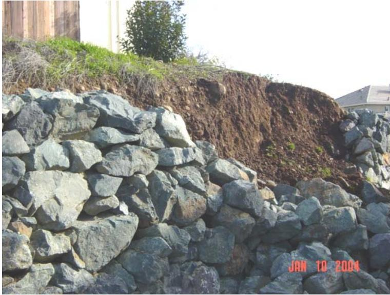
**Figure 1. Photograph. Failure of non-engineered rockery in El Dorado Hills, California, 2004.**
