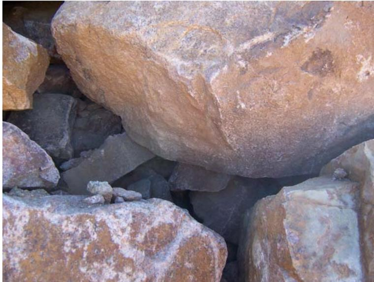
**Figure 69. Photograph. Example of improper rock bearing and lack of chinking.**
