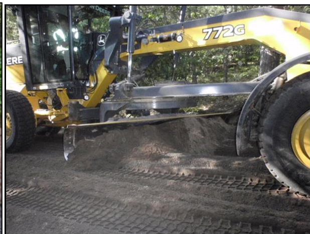
Road shaped with grader
