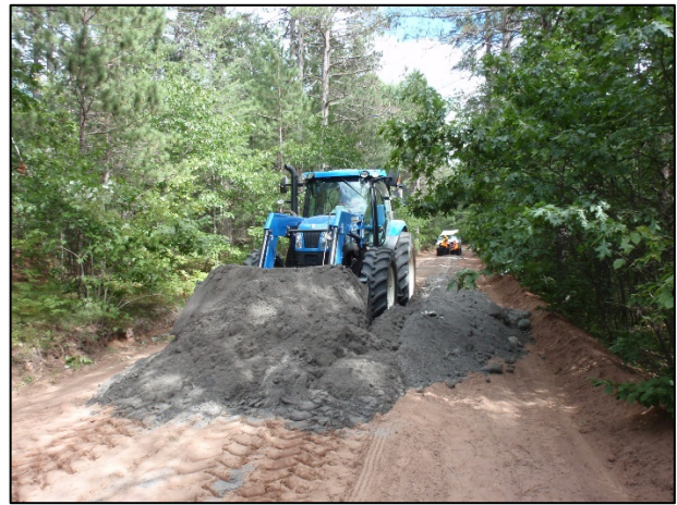
Ash spread on prepared subgrade
