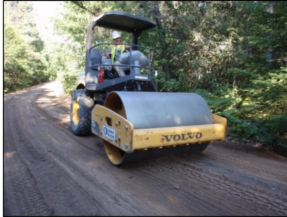
Compacting blended soil-ash mix
