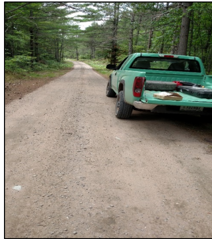
FR685 1 year after stabilization.
