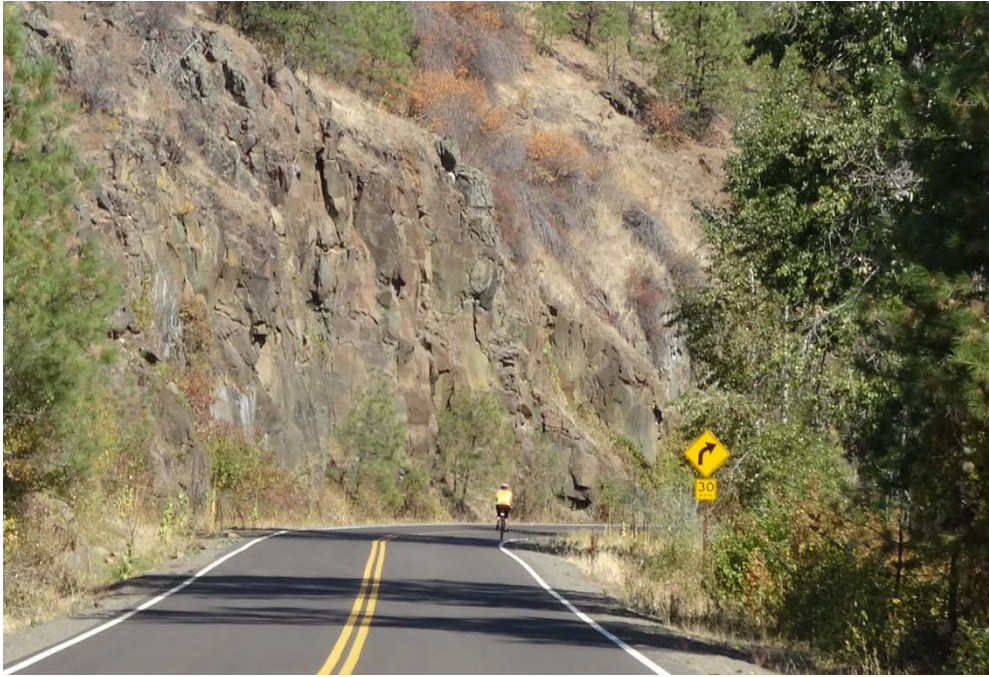
Figure 12: Photo. Curve warning sign with speed advisory plaque (WTI)
