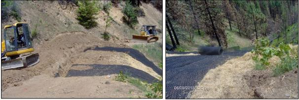
4. Backfill/compact anchor trench
