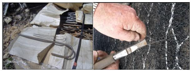
7. Anchor TRM to ground with stakes or rebar
