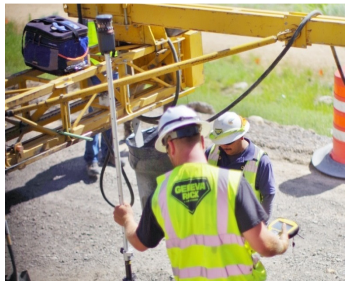
Figure 10: Real-time verification uses field survey equipment
