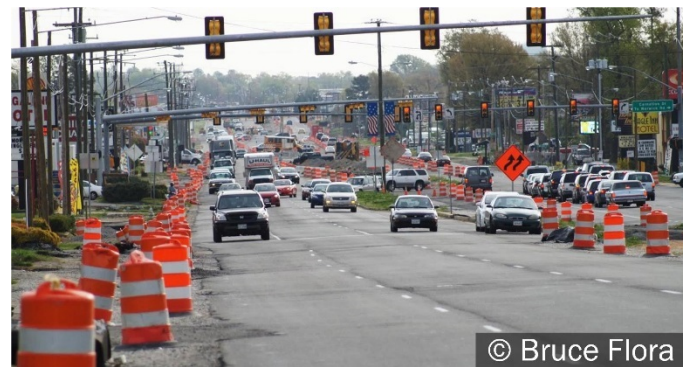
Figure 13: Traffic control installations can be documented quickly
