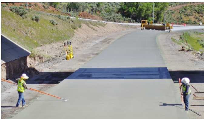
Figure 16: AMG improves access to the concrete paving work area
