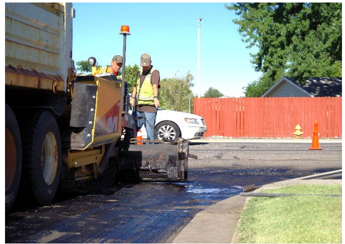
Figure 15: Asphalt mill-and-pave in an urban area without AMG
