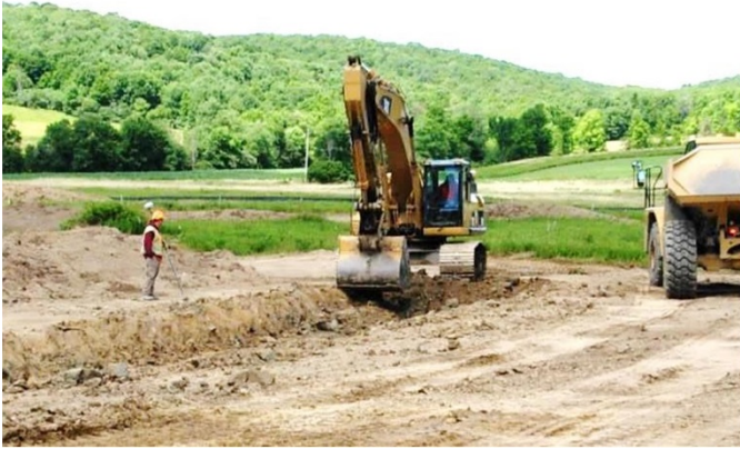
Figure 11: Inspector waits safely to take observations
