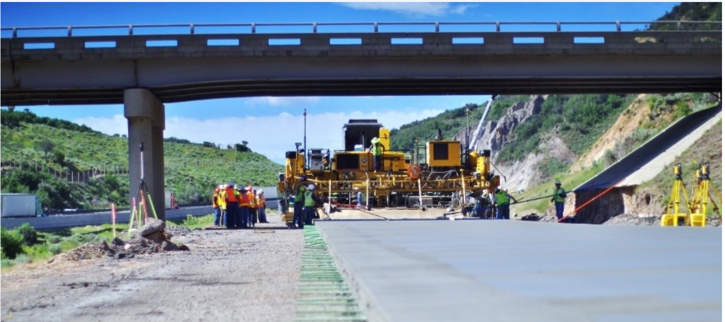
Figure 1: Automated Machine Guidance for concrete paving
