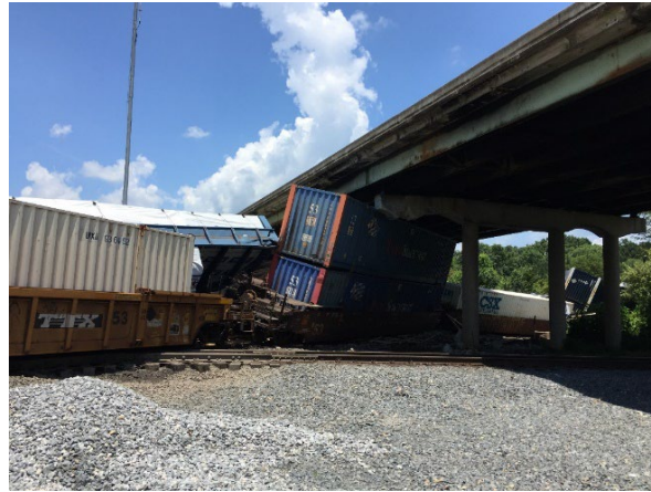
Collision beneath the U.S. Highway 59 overpass in Jefferson, Texas. Photo: TxDOT
