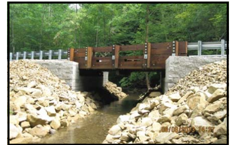
Figure 1—Riprap countermeasure field installation for a narrow bridge opening geometry.
