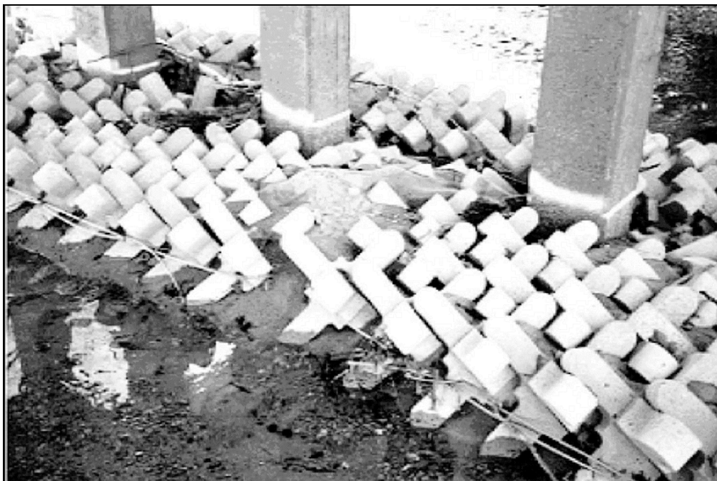
Figure 5.24. Installation of A-Jacks® modular units installed by Kentucky DOT for pier scour protection.
