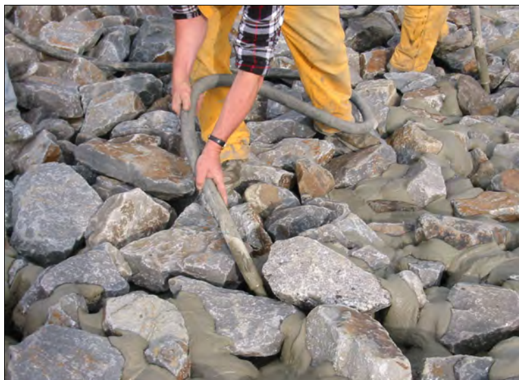
Figure 12.20. Grout placement by hand.
