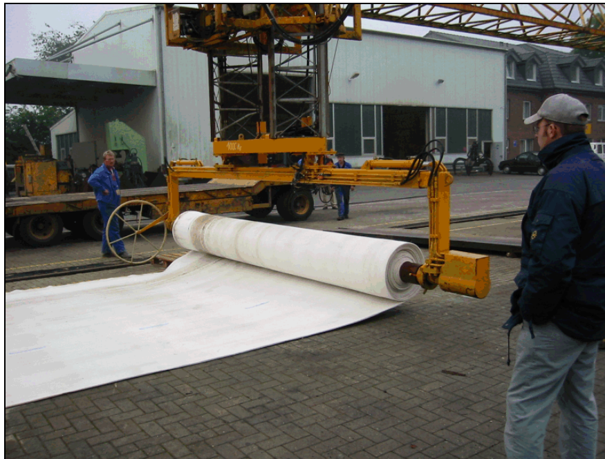
Figure 11.18. SandMat™ geocomposite blanket being unrolled. (photo from NCHRP Project 24-07(2), courtesy Colcrete – Von Essen Inc.)
