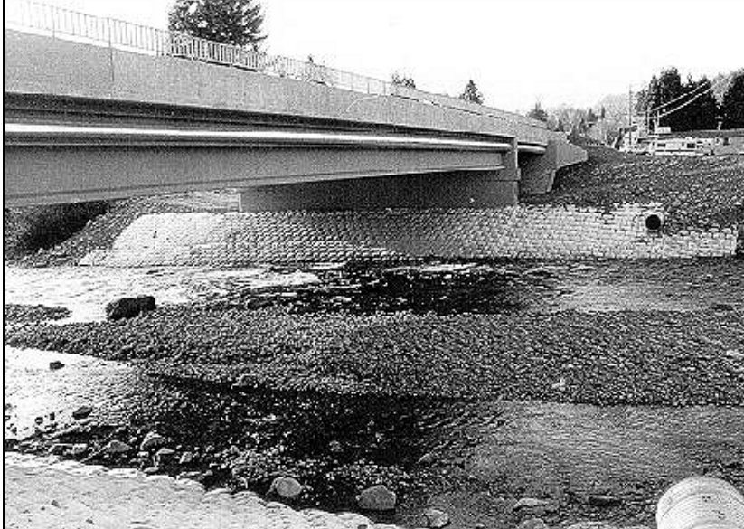
Figure 9.11. ABM installed on west bank of Salmon Creek (ODOT).
