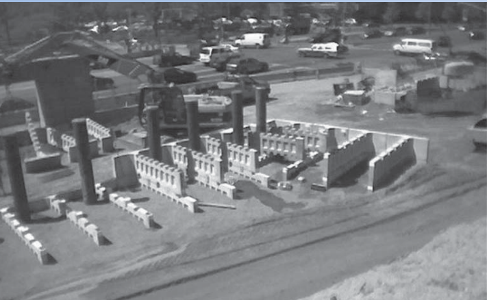
Precast T-walls also helped accelerate construction.
