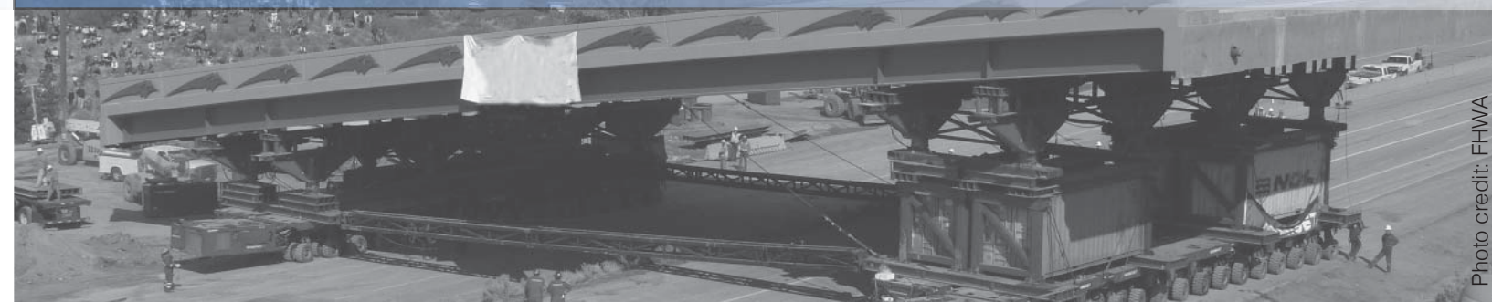
Crews used SPMTs to move the superstructure from the construction site to its final location over the interstate.
