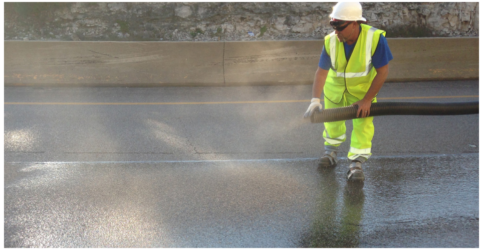
A worker, above, applies high-friction surface treatment to increase traction on a Missouri road segment.
