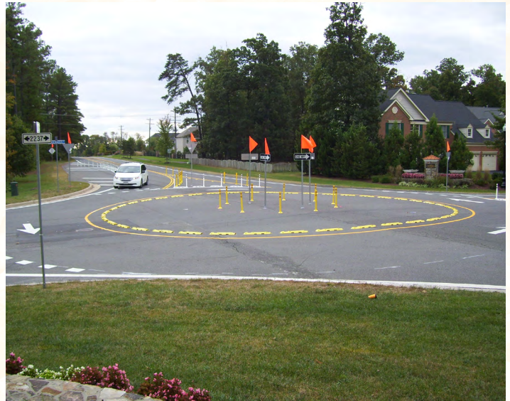
Credit: Virginia Department of Transportation
