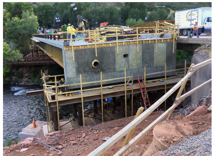
To reduce traffic disruption, crews in Glenwood Springs, CO, built a bridge on temporary supports before sliding it into place.
