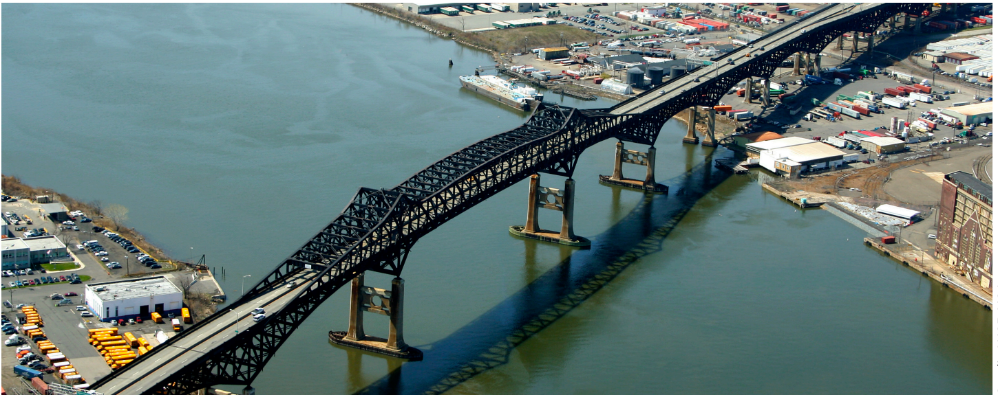
New Jersey's Pulaski Skyway deck replacement featured precast deck panels connected with UHPC, stainless steel rebar, and a polyester concrete overlay to maximize durability.
