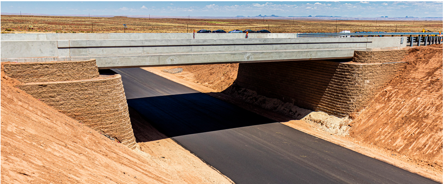
Credit: Arizona Department of Transportation
