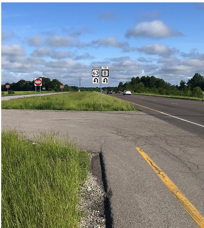
The Missouri Department of Transportation constructed a median U-turn to eliminate right-angle crashes at the intersection of U.S. 63 and Routes B/P in Clark.
