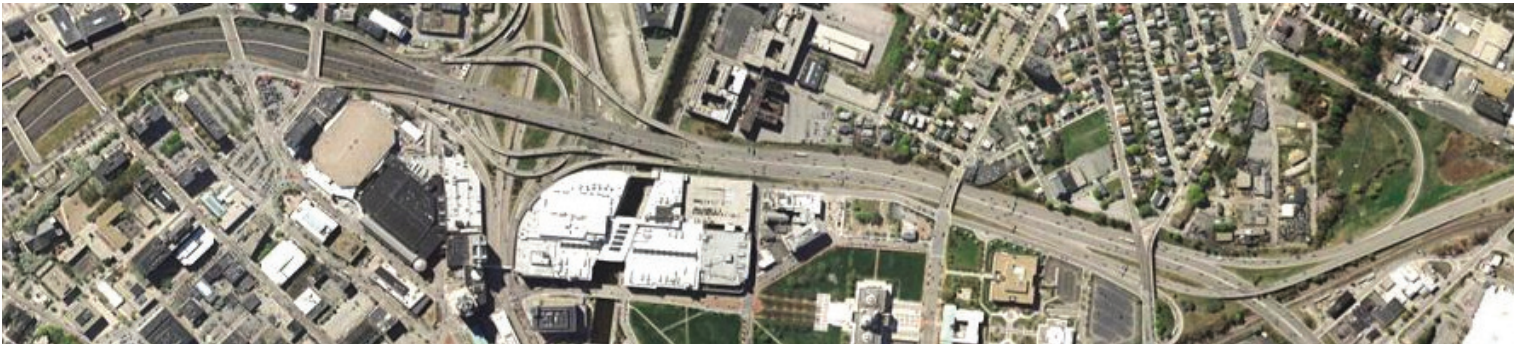
An aerial image of the I-95 Northbound Viaduct Replacement site in Providence, RI.
