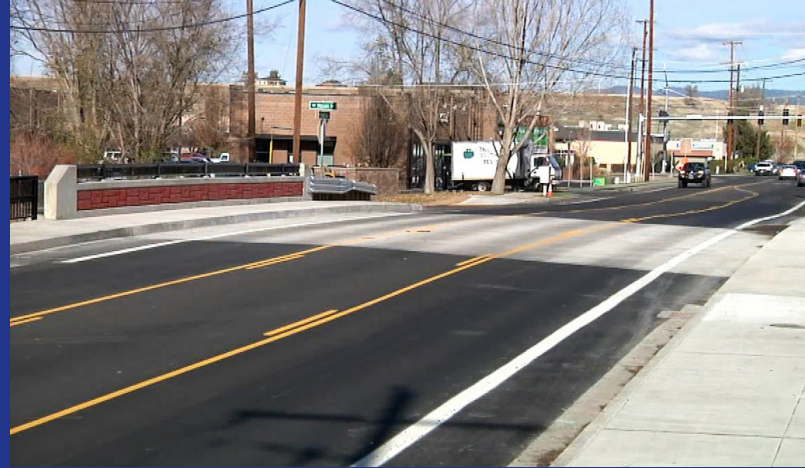
Figure 2: Recently reconstructed Ochoco Creek Bridge in Prineville, Oregon (Photo Credit: Oregon Department of Transportation)
