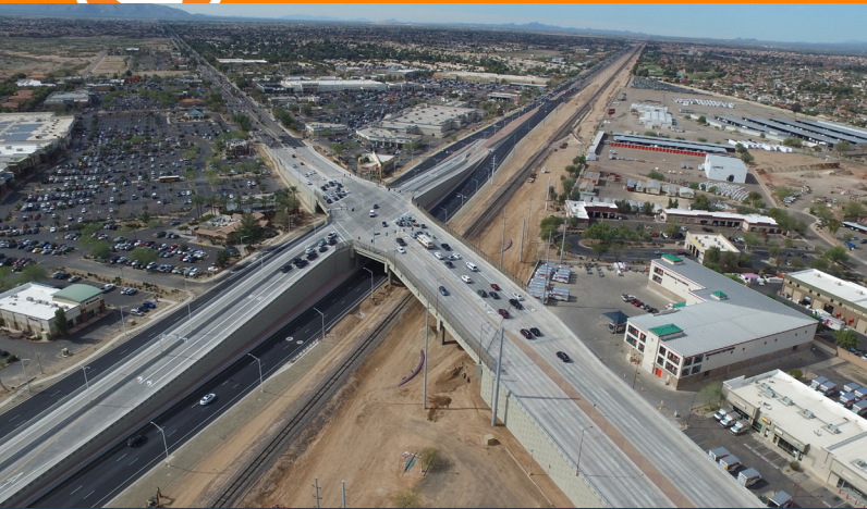
Figure 1: Newly constructed US-60/Bell Road Interchange in Surprise, Arizona (Photo Credit: City of Surprise)
