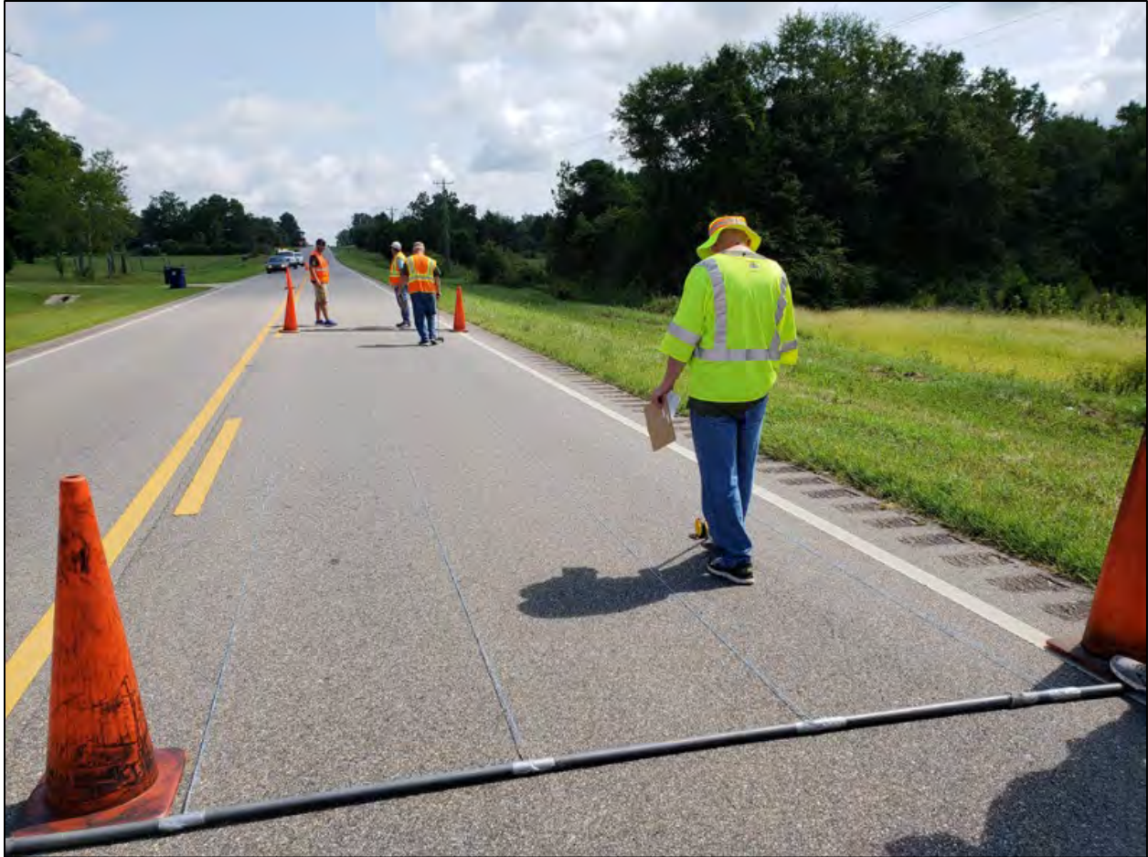
Figure 26. Photograph. A template can be used to increase the efficiency of wheel path layout.
