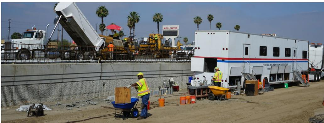
COVER IMAGE: FHWA Mobile Concrete Technology Center staff partnered with Caltrans in La Mirada, CA, to implement PEM principles into specifications. Caltrans reported reduced costs and improved test results. (Source: FHWA)
