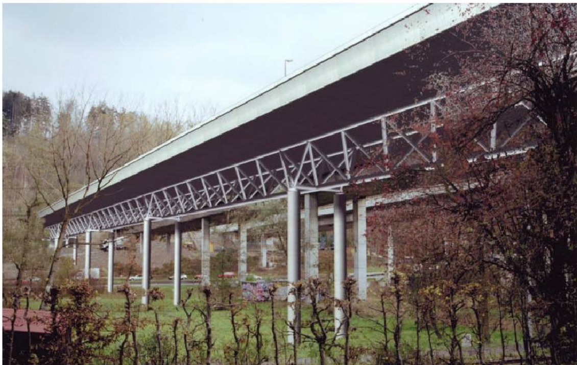
Figure 2.32 (Cont.): Completed Lully Viaduct Bridge – Swiss Highway A1 Source: http://www.dic-ing.ch/data/lully.pdf
