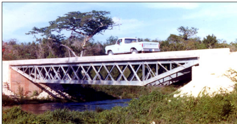
Figure 2.40: Steel Under-Truss Bridge, Belize, Central America
