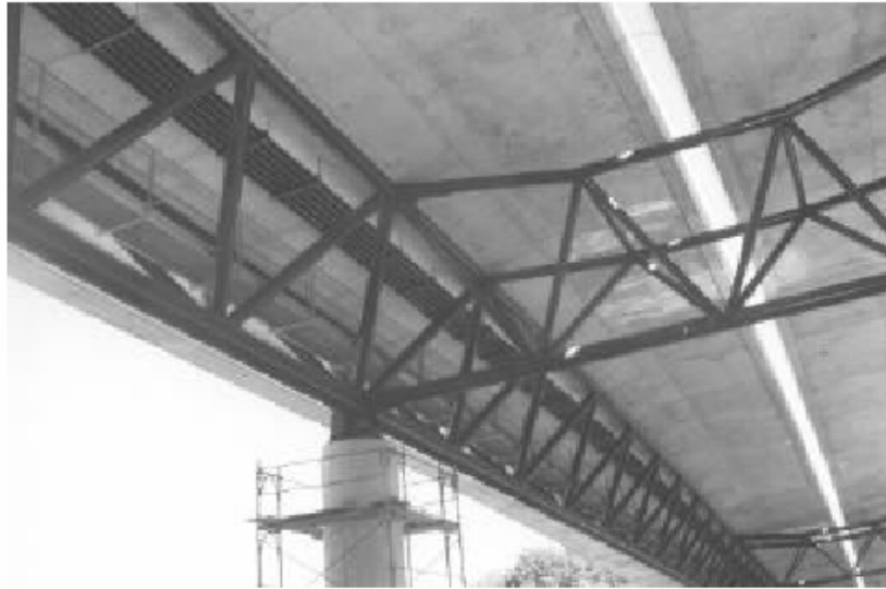
Figure 2.32 (Cont.): View of Bridge During Construction Source: http://www.dic-ing.ch/data/lully.pdf
