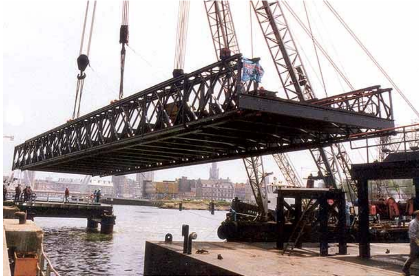
Figure 2.15: Janson HPB During Erection Source: www.jansonbridging.com
