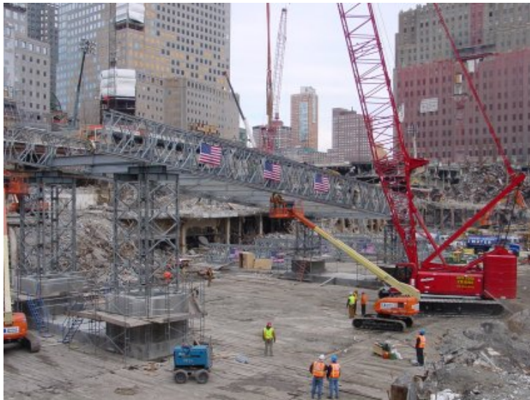
Figure 2.9: Erection of the Acrow 700XS Bridge @ Ground Zero in New York
