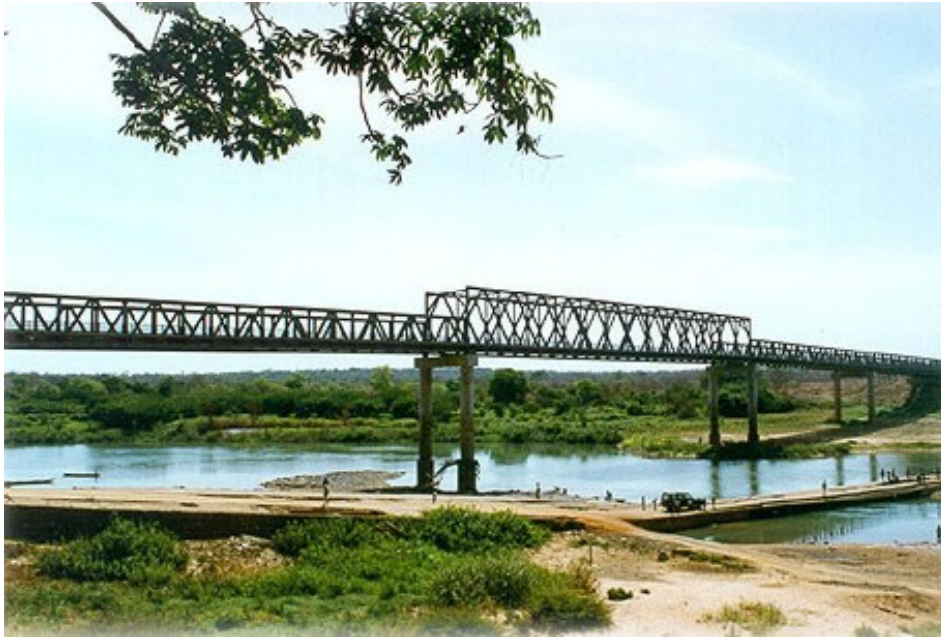
Figure 2.14: Mabey and Johnson Bridge
