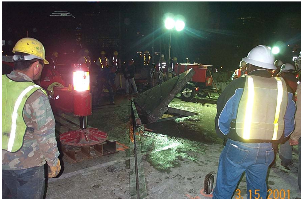
Figure 2.22: Saw Cutting and Removing Existing Concrete Deck
