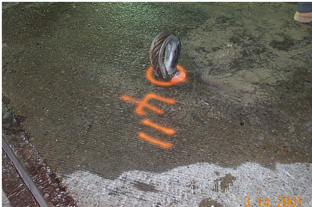
Figure 2.21: Drilling and Installing Lifting Cables
