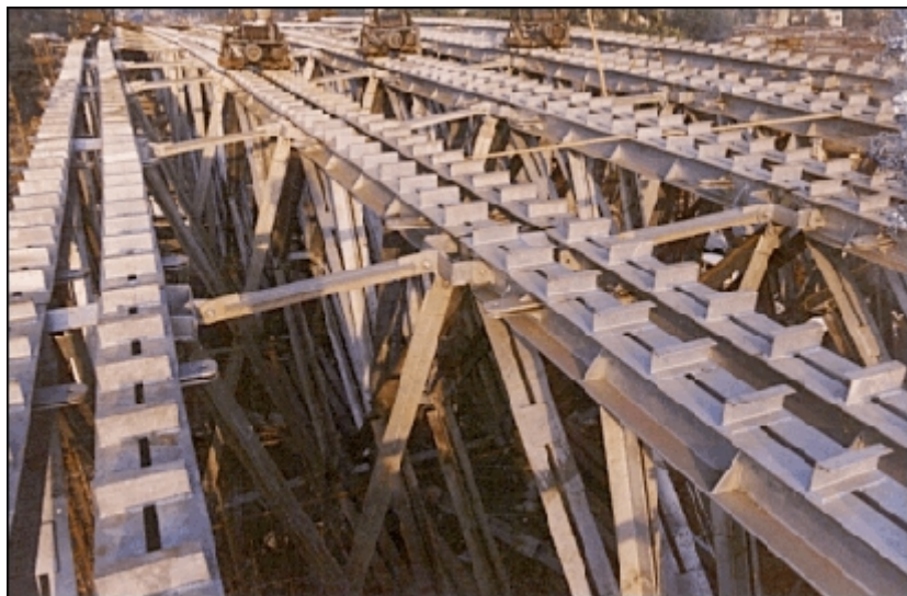
Figure 2.18: Quadricon Bridge System Source: www.quadricon.com
