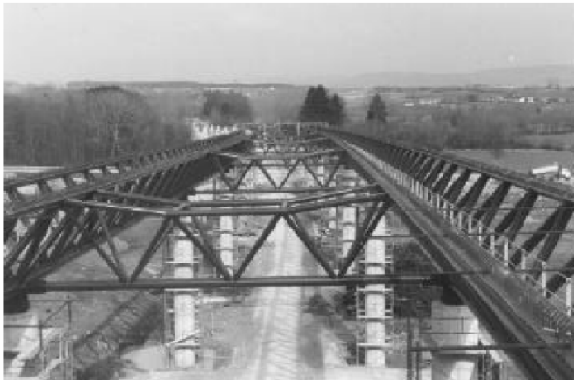
Figure 2.32: Longitudinal View During Construction Source: http://www.dic-ing.ch/data/lully.pdf
