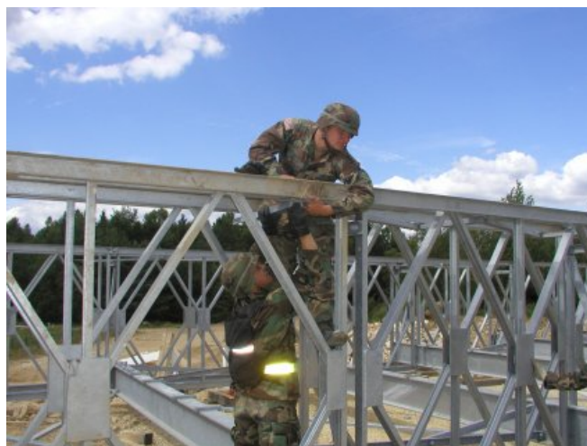
Figure 2.6: Hand Assembly of Bailey M2 Bridge
