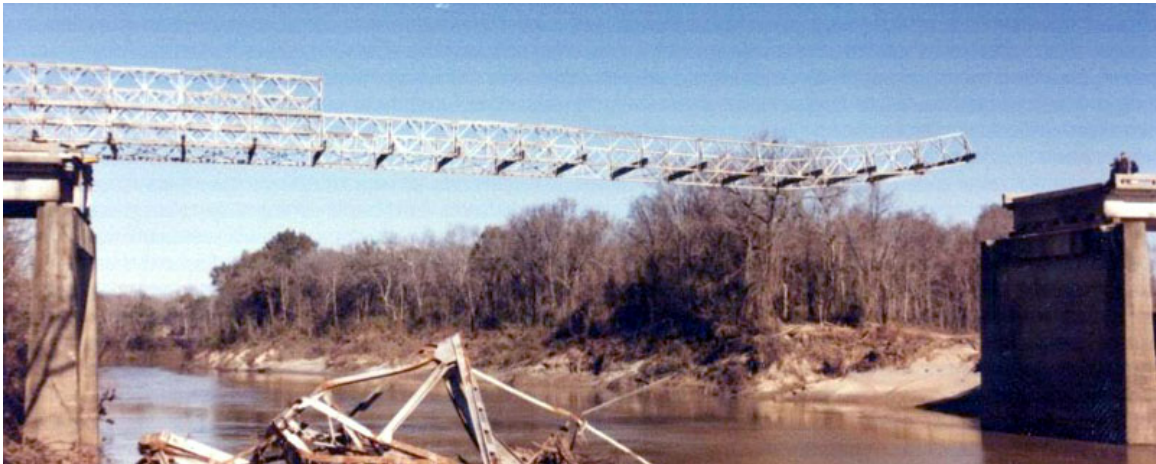
Figure 2.7: Full Cantilever Launching of a Bailey Bridge
