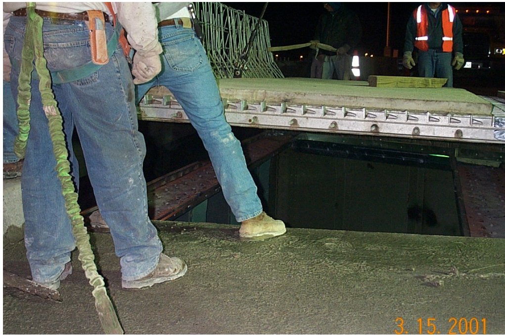
Figure 2.23: Placement of New Concrete Filled Grid Deck
