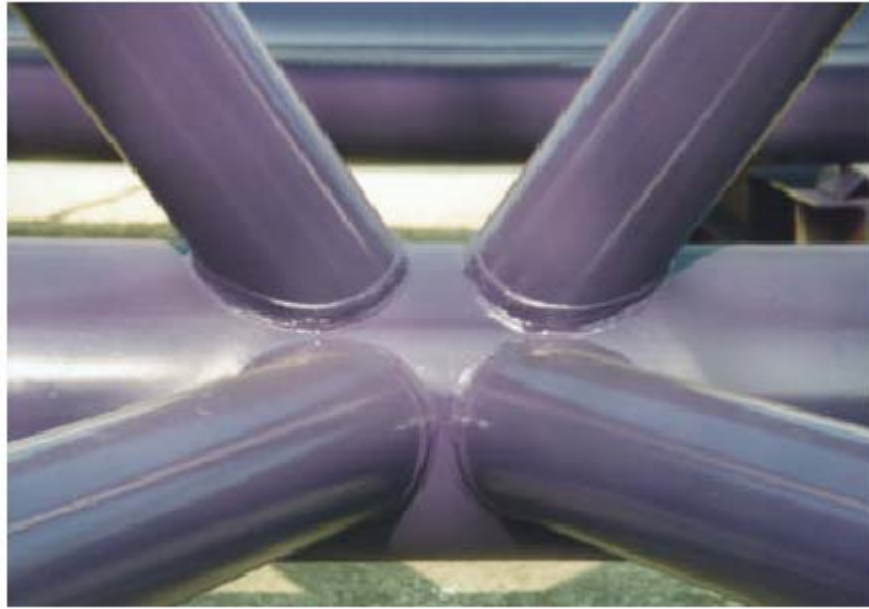
Figure 2.31: Bottom Chord to Diagonals Joint Connection Detail Source: http://www.dic-ing.ch/data/lully.pdf
