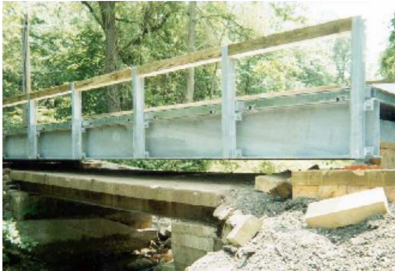
Figure 2.19: Longitudinal Beam Replacement Photo
