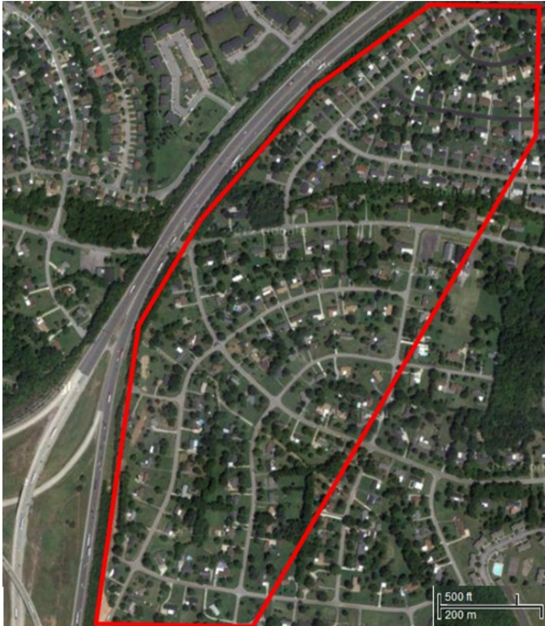
Figure 21. Study Area A: Ten-lane highway with dense development close to the highway.
