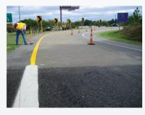
FIGURE 2: HFST at horizontal curve
