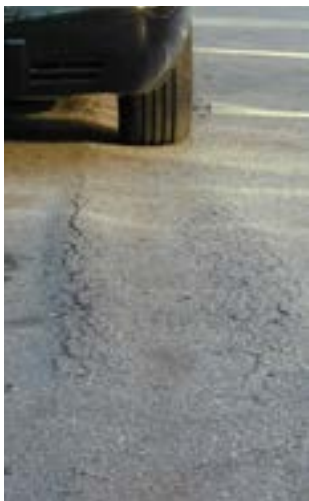
Inadequate design, selection, testing, and performance in asphalt binders can lead to pavement distress like the rutting shown here. Source: APTech.
