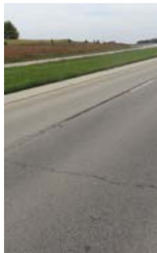
Increasing the use of performance-based asphalt binders can help minimize premature pavement distress like this transverse cracking. Source: APTech.
