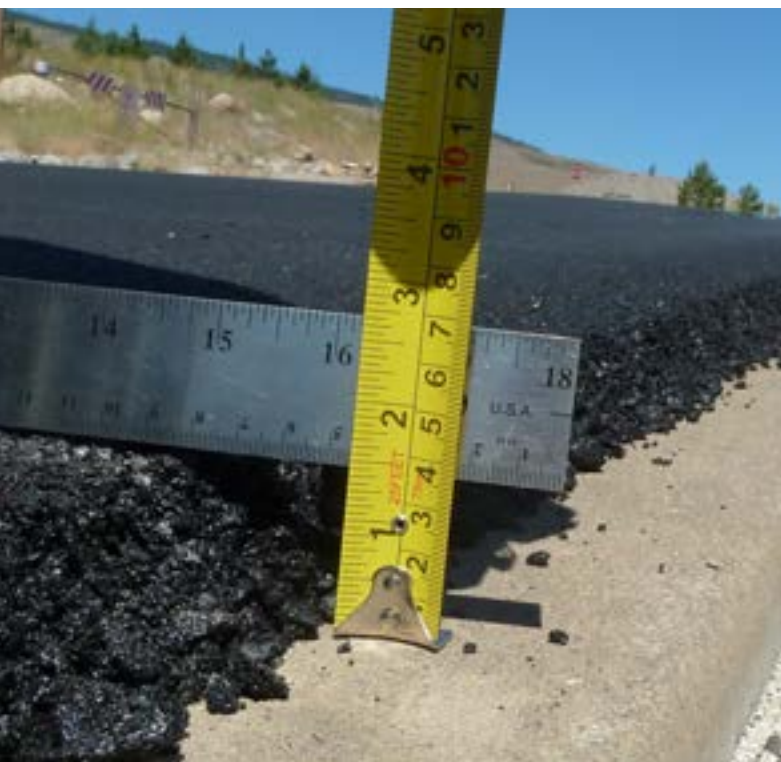
Thin asphalt overlays commonly measure 1.5 inches or less, like this dense-graded asphalt overlay in Reno, NV. Source: Applied Pavement Technology, Inc.
