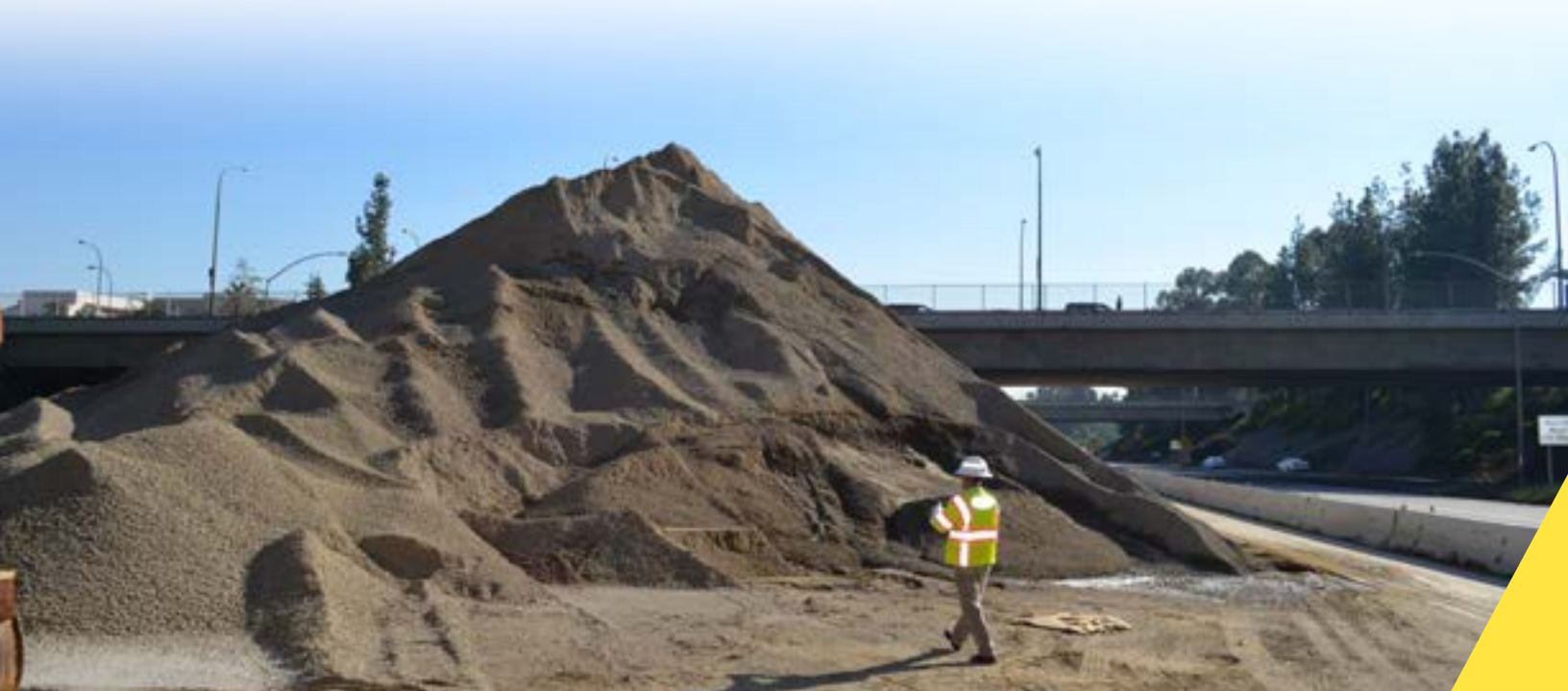
(Below) This stockpile of RCA beside a road is ready for reuse. Source: APTEch.
