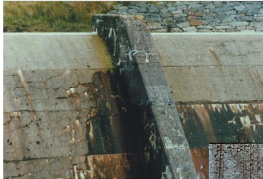
Dam constructed with low-alkali cement
