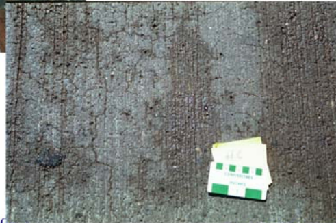
Pavement constructed with low-alkali cement
